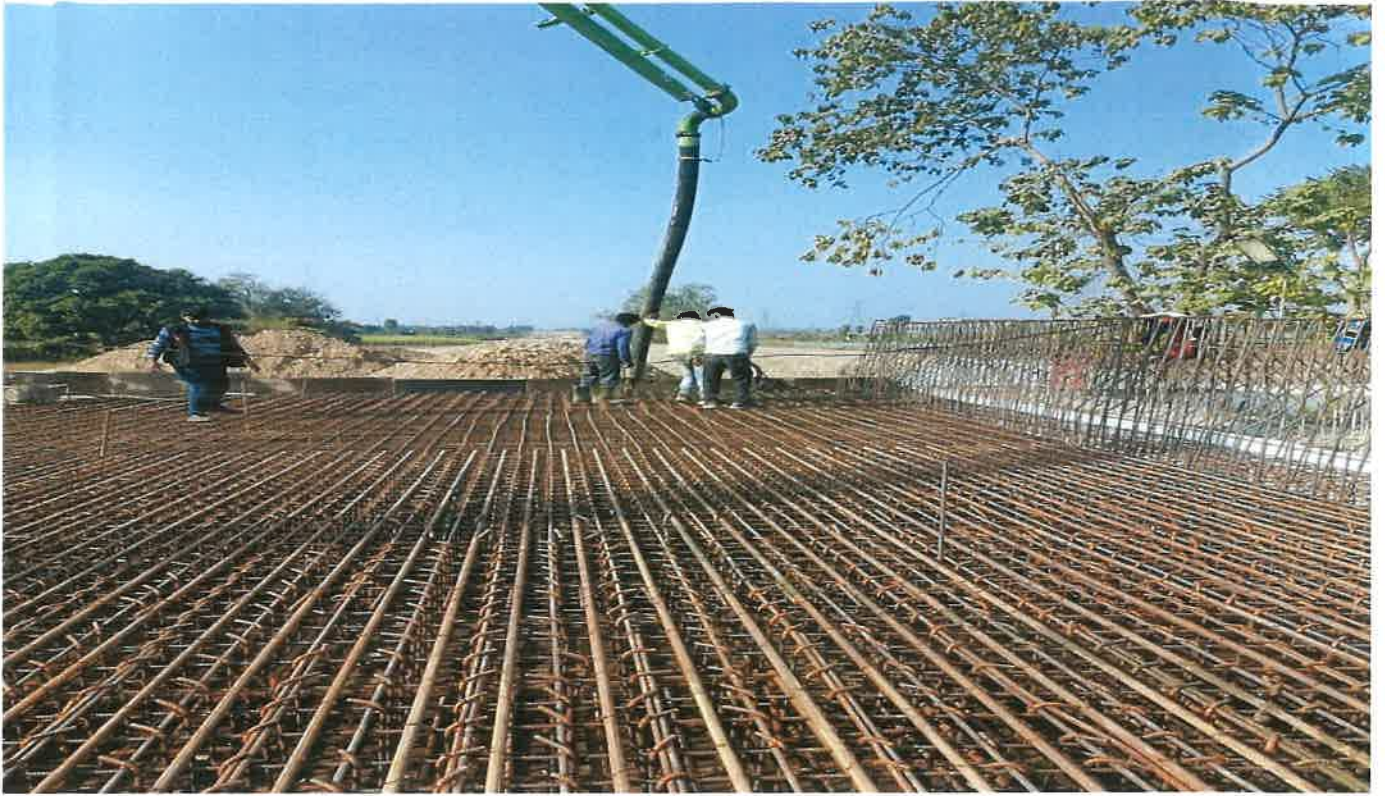
MNB Slab Concrete Pouring Work in Progress at Ch. 25+320
