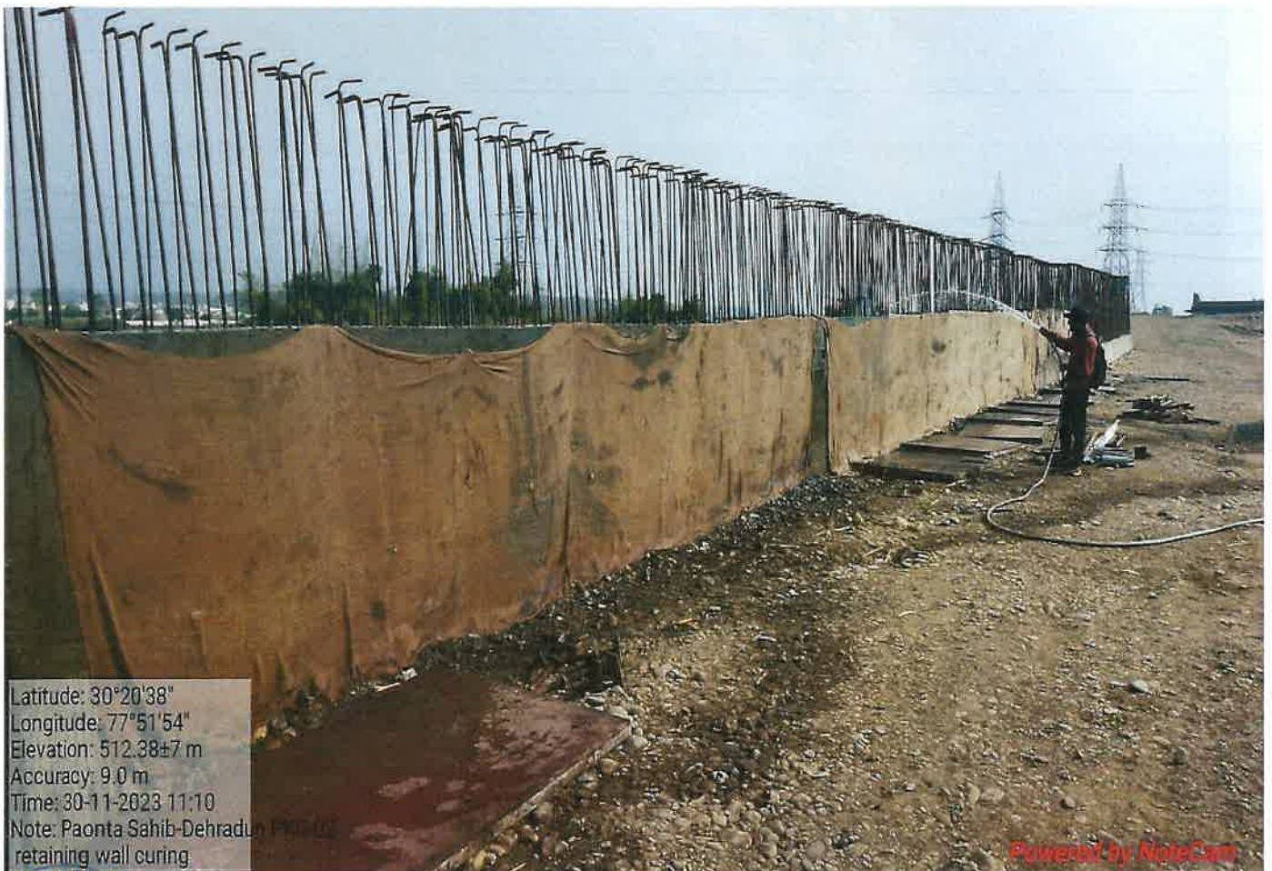
Retaining Wall Curing Work in Progress at Ch. 30+110
