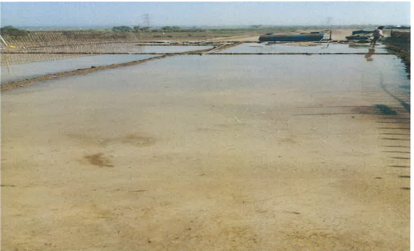
MNB Top Slab Curing Work in Progress at Ch. 19+297
