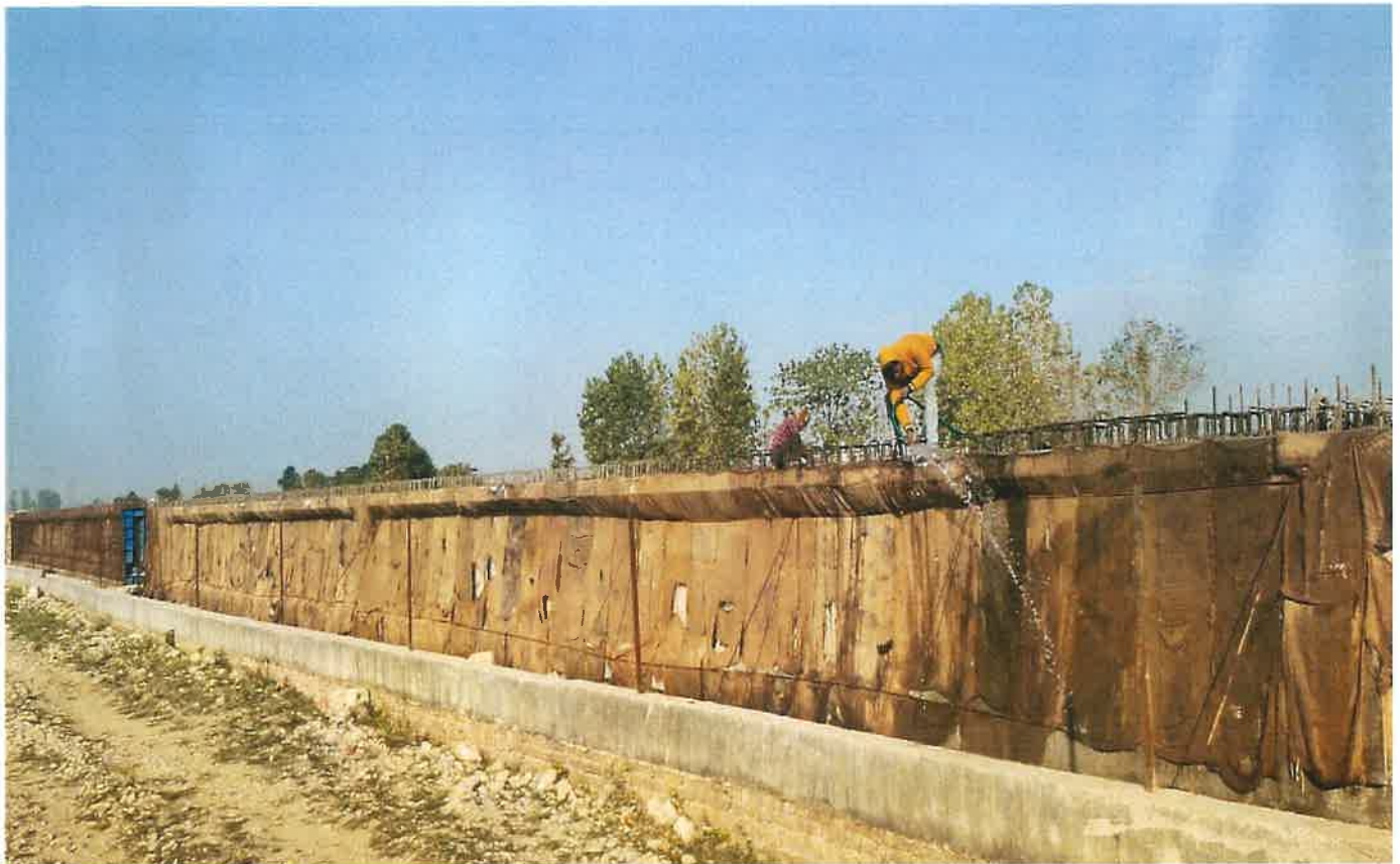
MJB Girder Curing Work in Progress at Ch. 33+033
