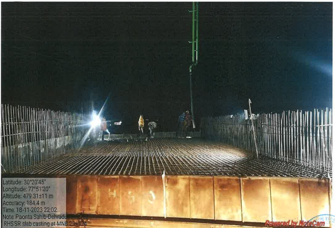
MNB Slab Concrete Pouring Work in Progress at Ch. 29+174
