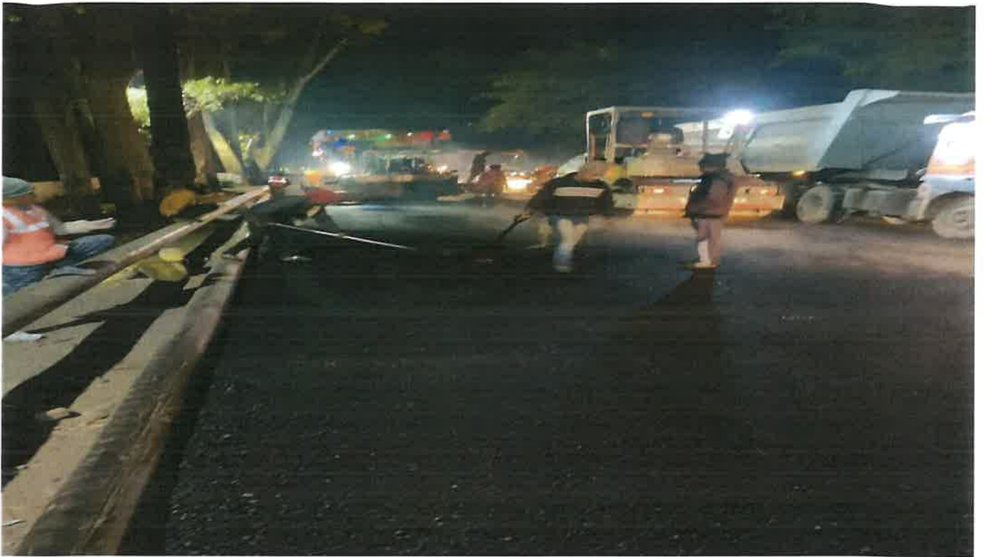
DBM Laying Work in Progress at Ch. 43+605 to 44+730
