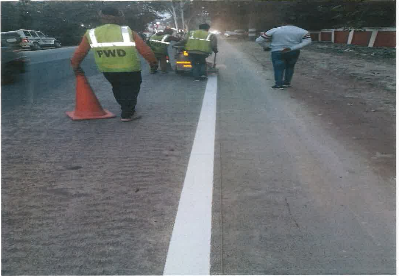
Thermoplastic Road Marking Work in Progress at Ch. 44+800
