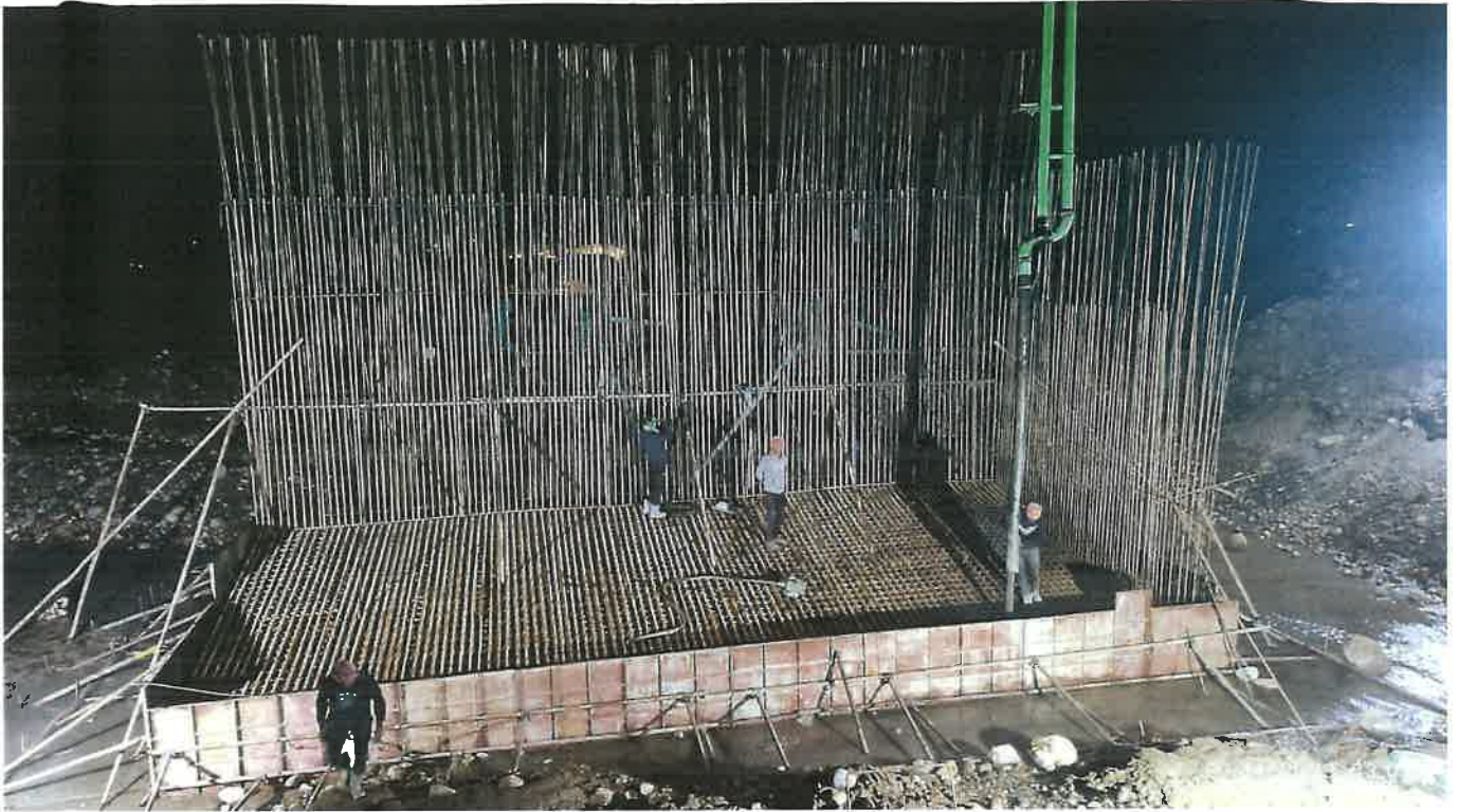
MJB Abutment Foundation Concreting Work in Progress at Ch. 33+033
