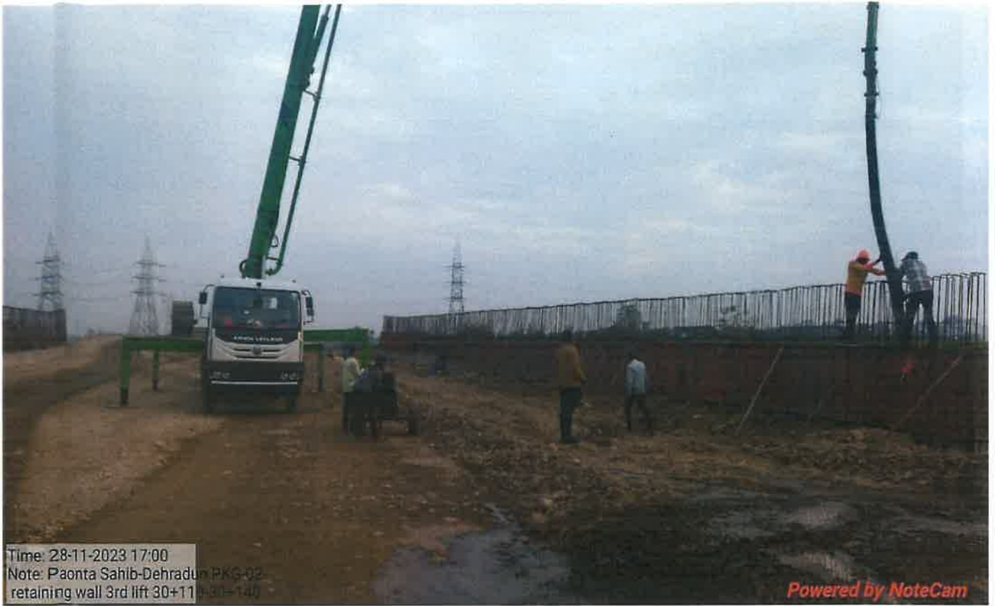
Retaining Wall Concreting Work in Progress at Ch. 30+140
