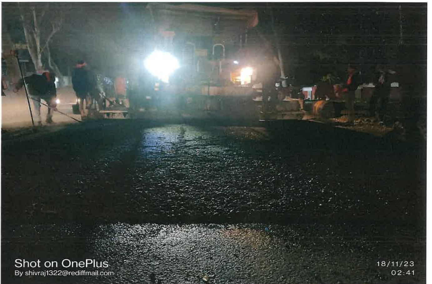
DBM Laying Work in Progress at Ch. 44+260 to 44+500
