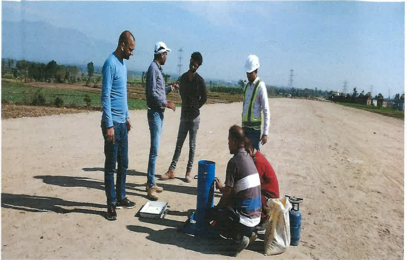
Sub-Grade Top Layer FDD Testing at Ch. 19+500
