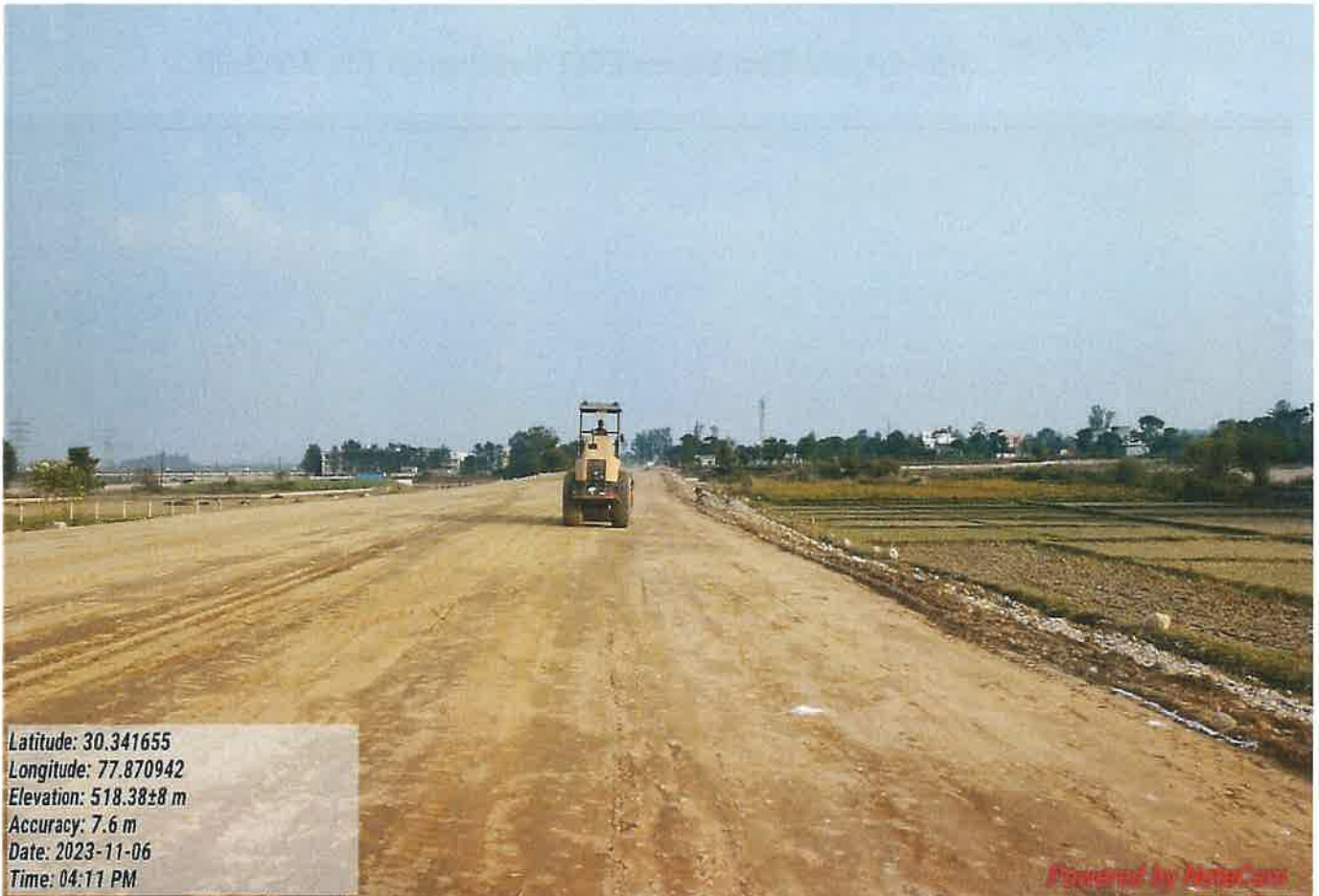
Sub-Grade Top Layer Rolling Work in Progress at Ch. 30+600
