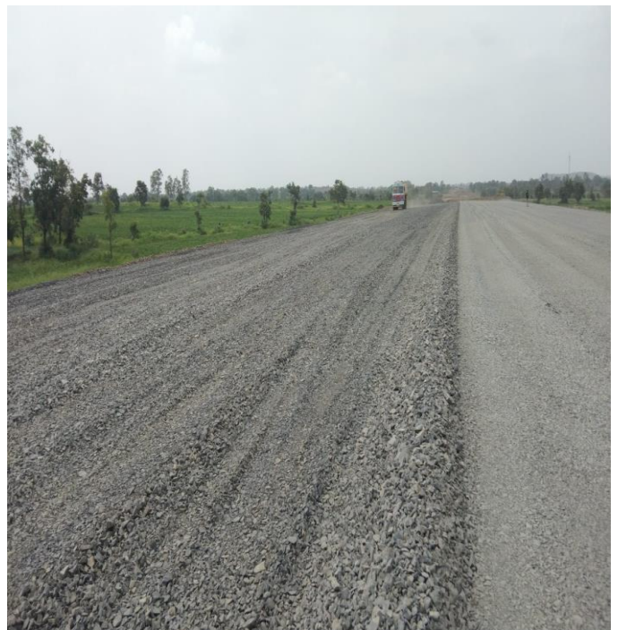
GSB WIP at Ch- 119+940 to 120+140 RHS
