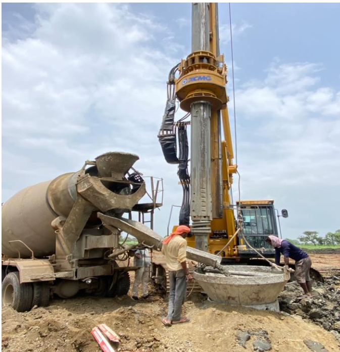
ROB at Ch- 127+207
