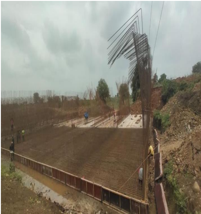
MJB Raft Reinforcement at Ch- 113+817
