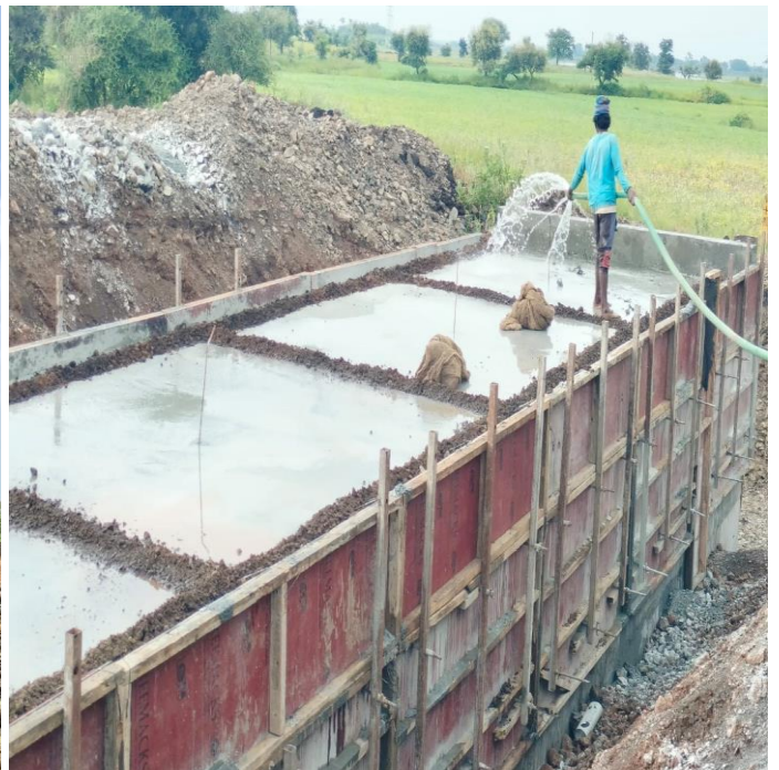
Box Culvert Slab Curing WIP at Ch- 166+400
