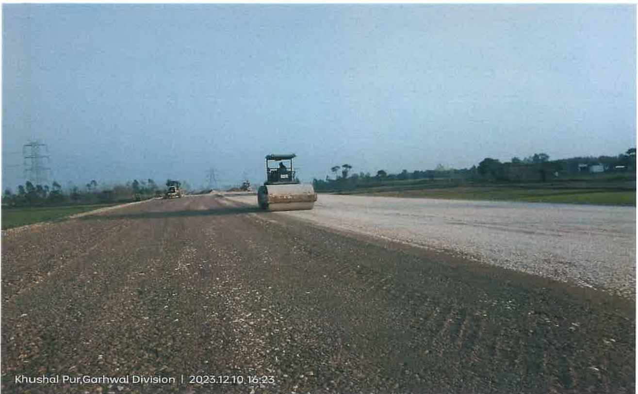
GSB Bed Rolling Work in Progress at Ch. 19+900
