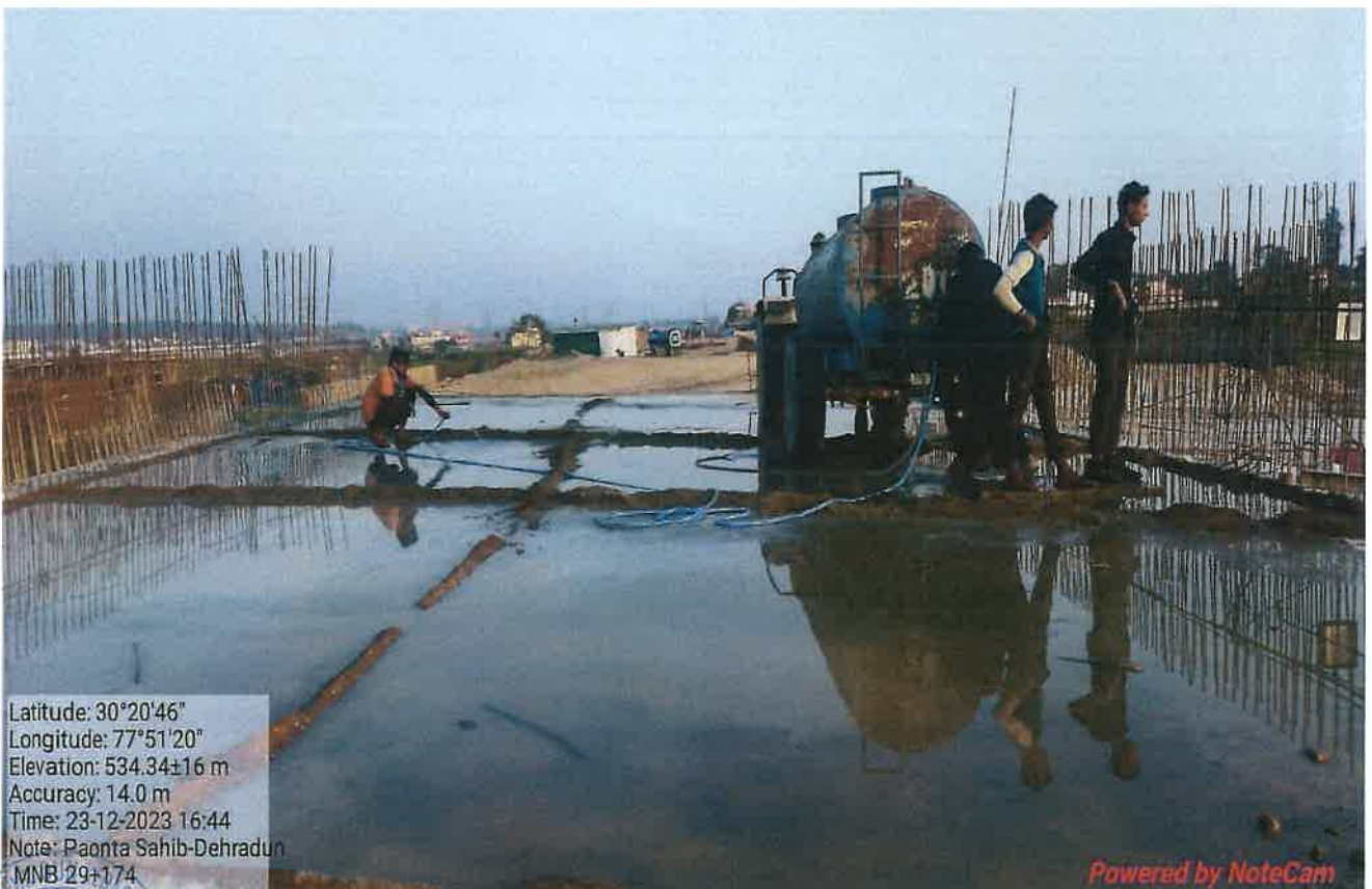
MNB Slab Curing Work in Progress at Ch. 29+174
