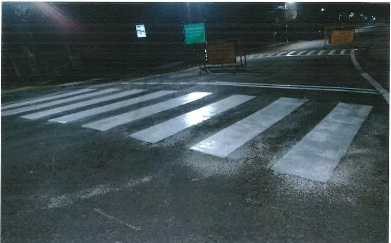
Junction Pedestrian Crossing Marking at Ch. 42+200
