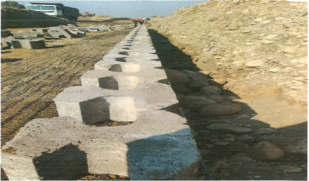
RE Block Erection Work in Progress at Ch. 31+500
