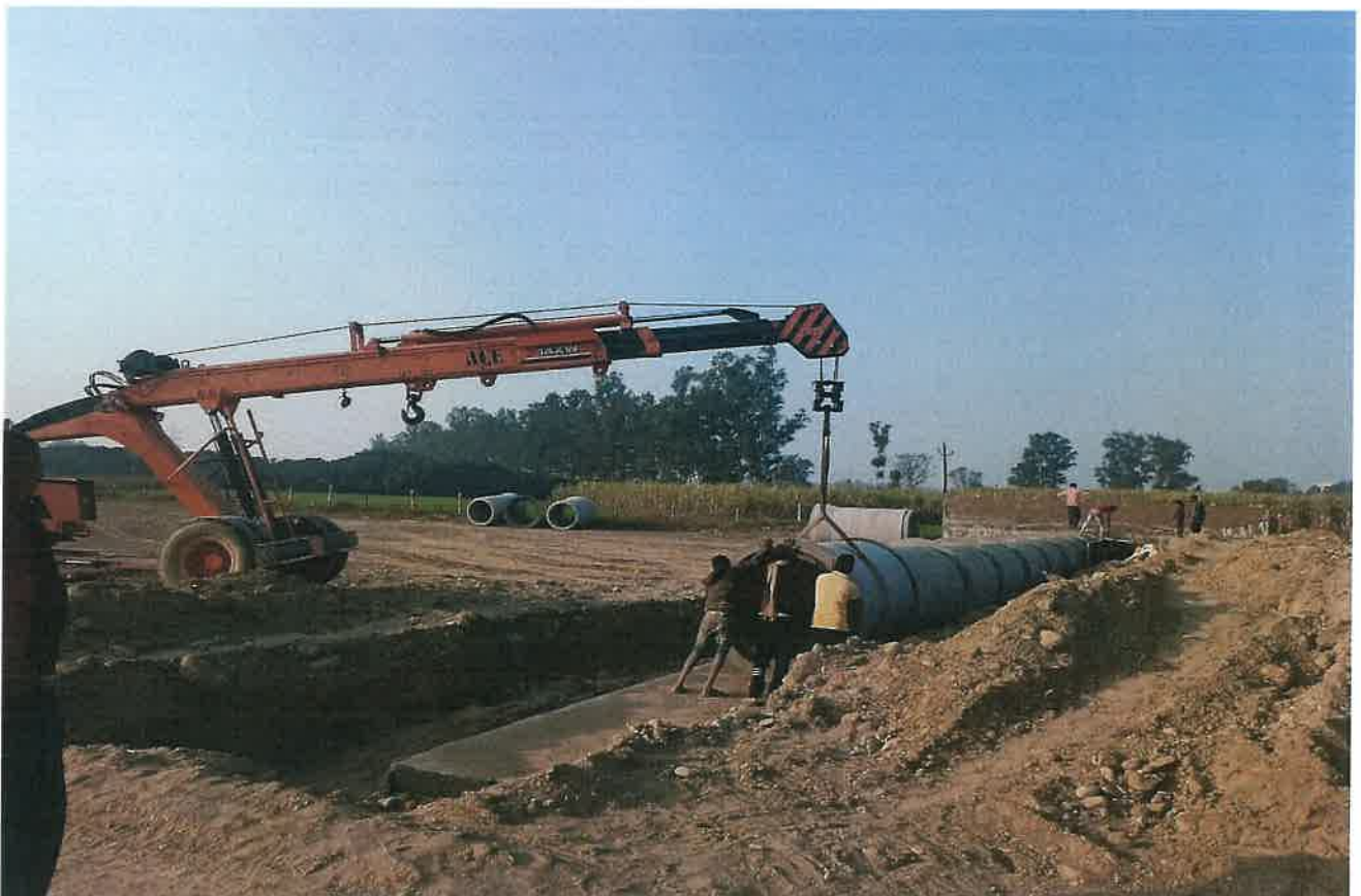
Hume Pipe Laying of HPC Work in Progress at Ch.33+600
