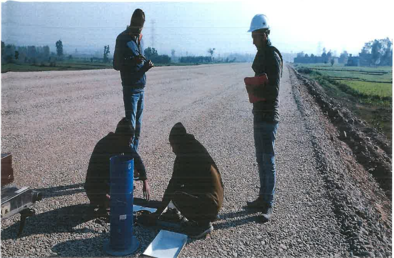
FDD Checking on GSB Top Layer at Ch.19+350
