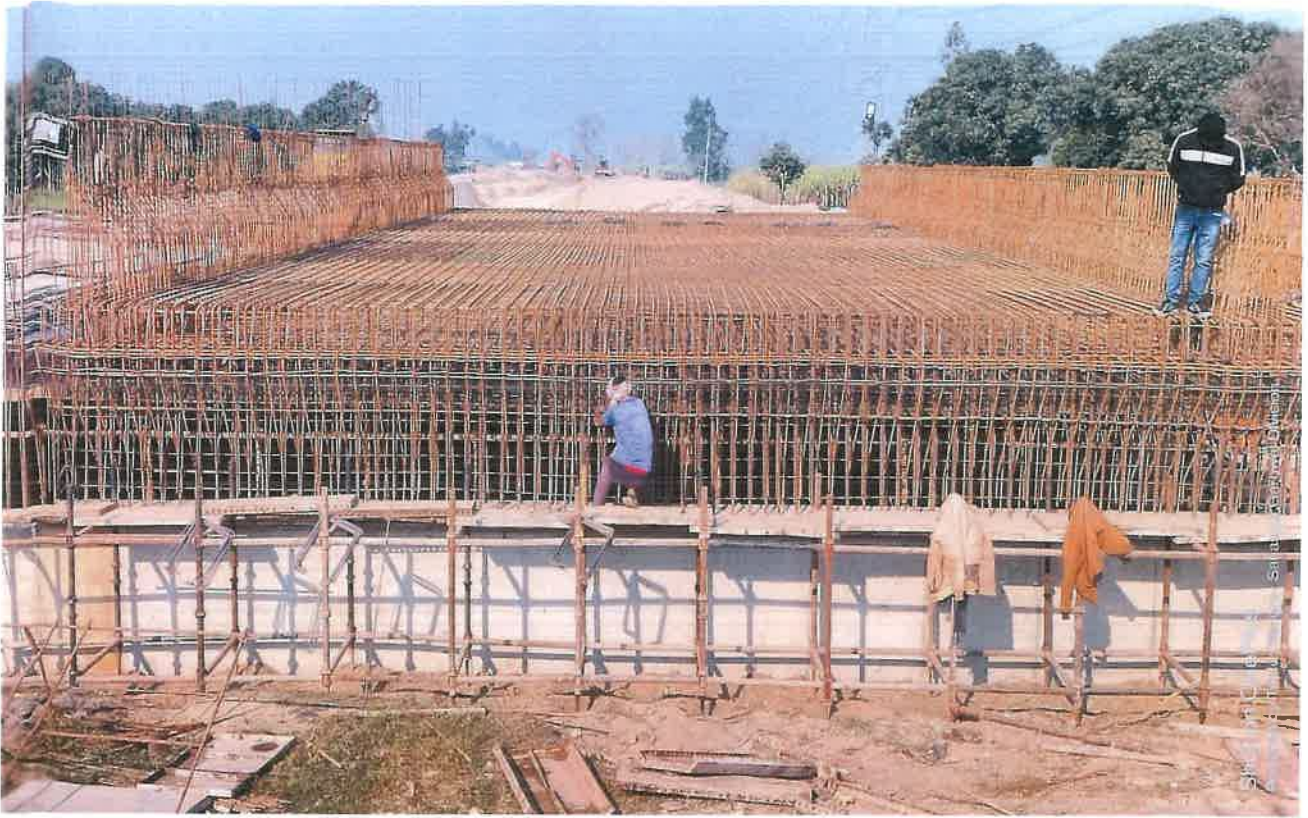
MNB Slab Reinforcement Work in Progress at Ch. 22+973
