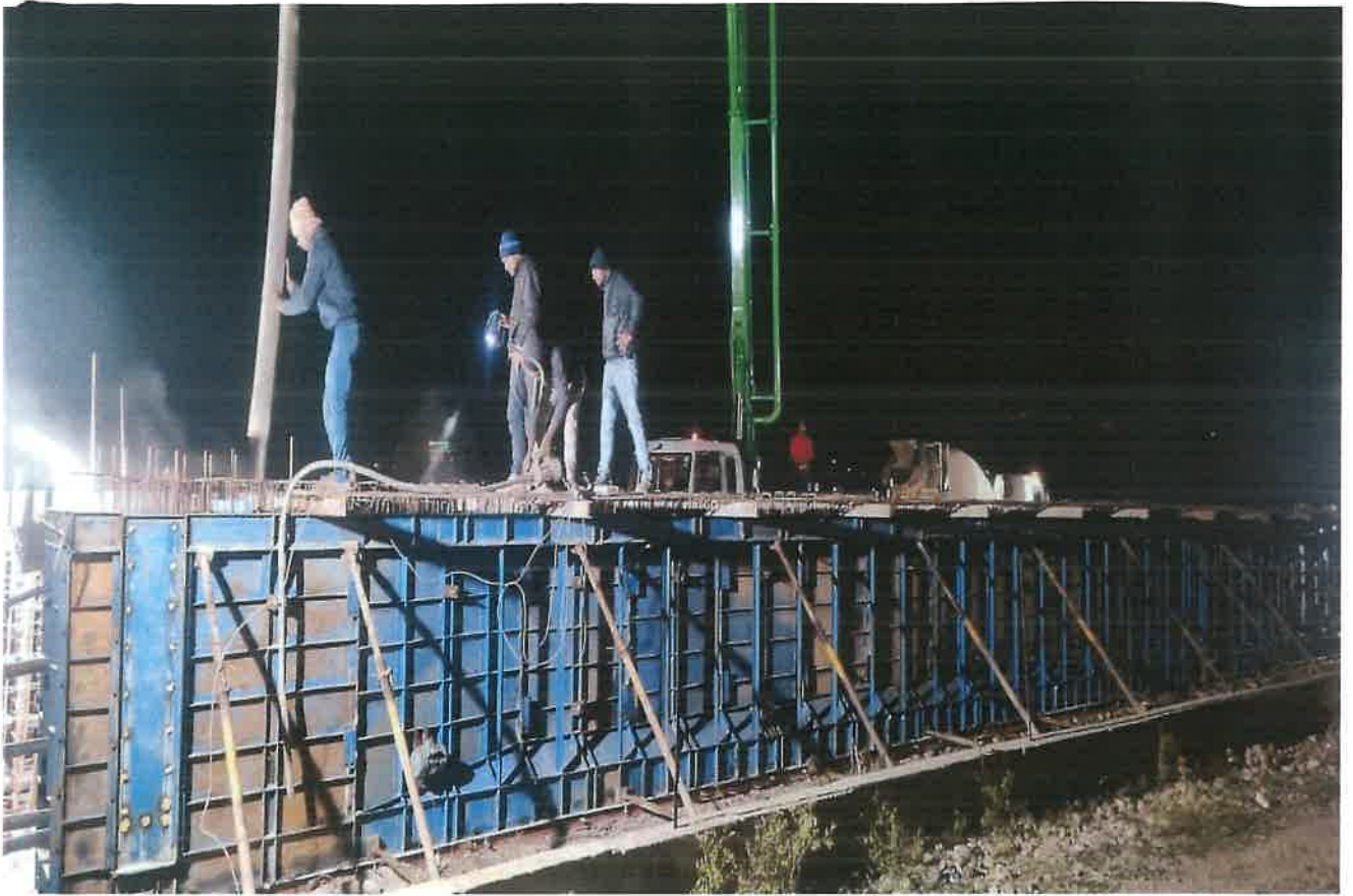
MJB Girder Concrete Work in Progress at Ch. 33+033
