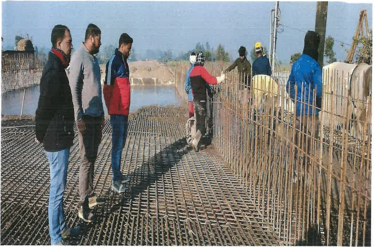
MNB Slab Casting Work in Progress at Ch. 27+741
