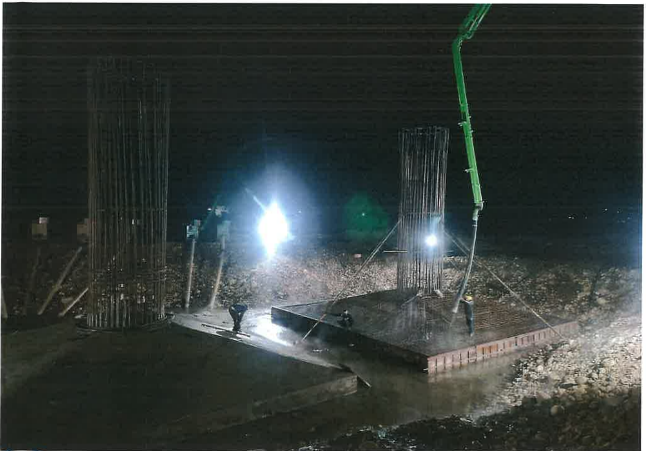
MJB Foundation Concreting Work in Progress at Ch. 33+033
