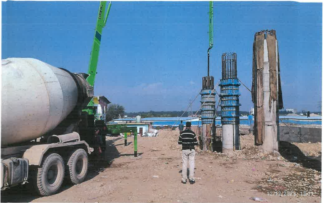
VUP Abutment Shaft Concrete Work in Progress at Ch. 31+678
