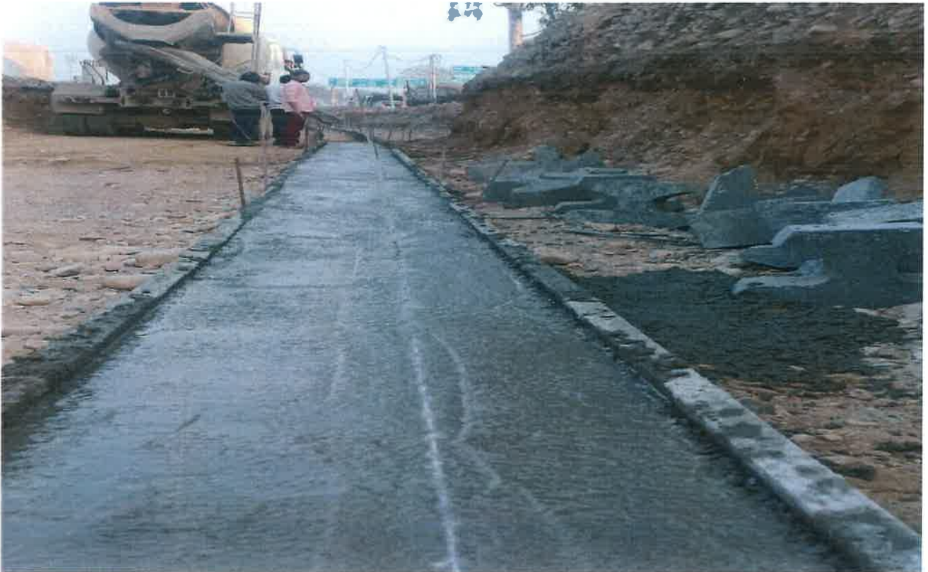
RE Wall Bed PCC Work in Progress at Ch. 31+540
