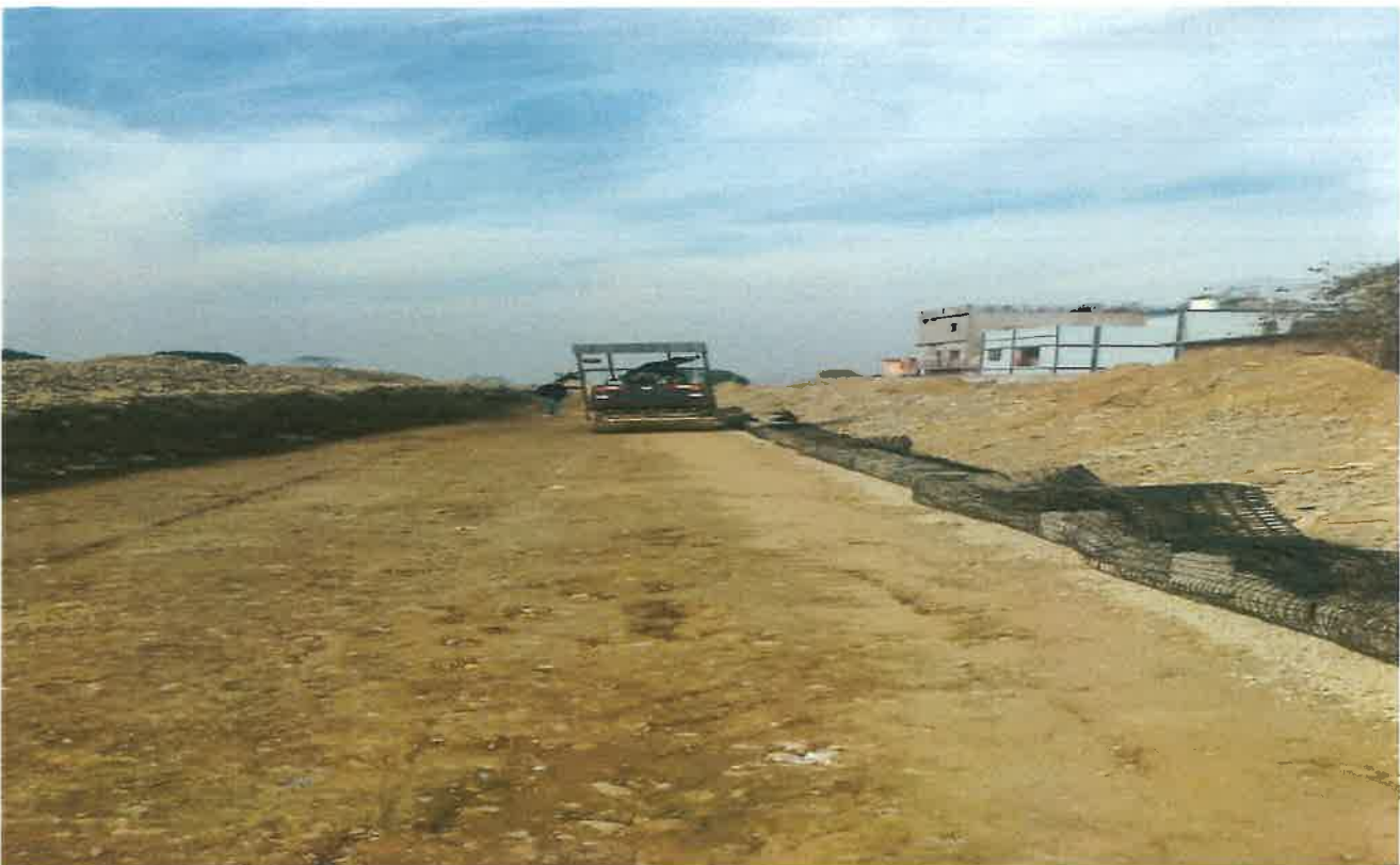
RE Wall Bed Compaction Work in Progress at Ch. 31+320
