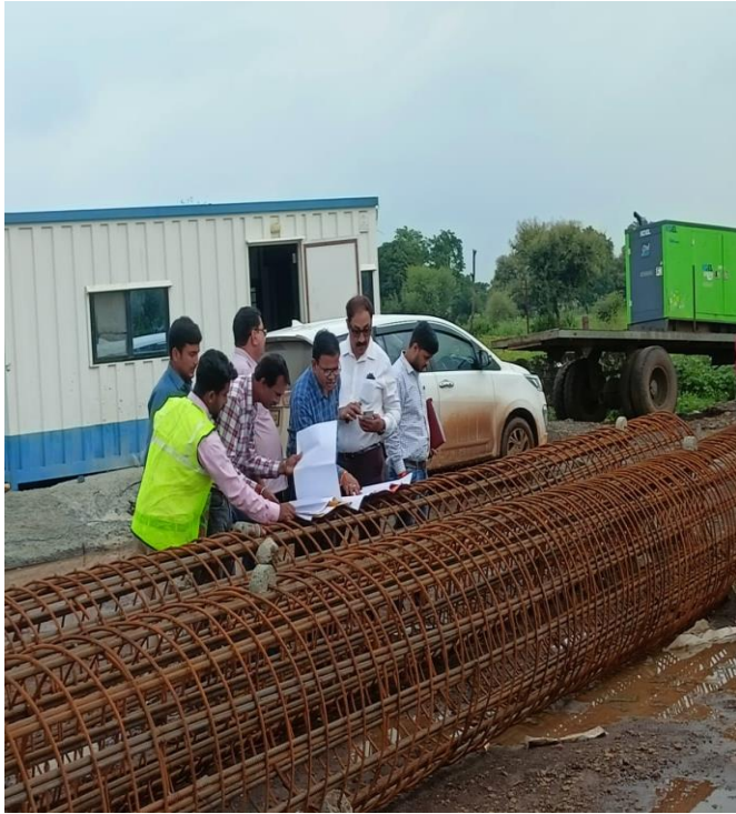
CH:- 127+197 ROB PILE REINFORCEMENT CHECKING
