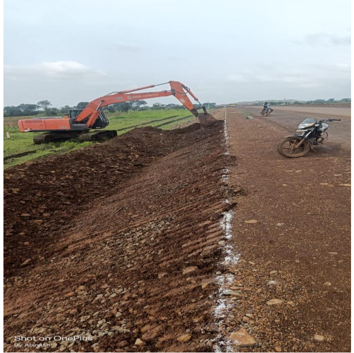
CH:- 110+100 to 110+200 SLOPE CUTTING WIP (LHS)
