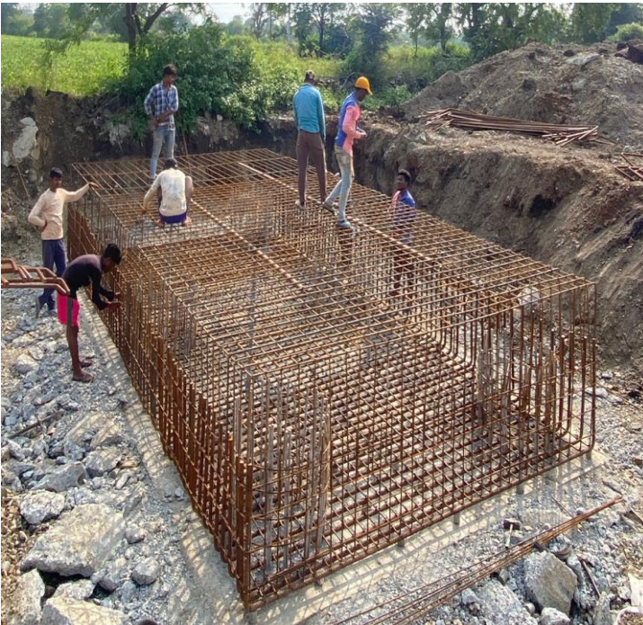
CH:- 127+197 ROB PILE CAP REINFORCEMENT WIP
