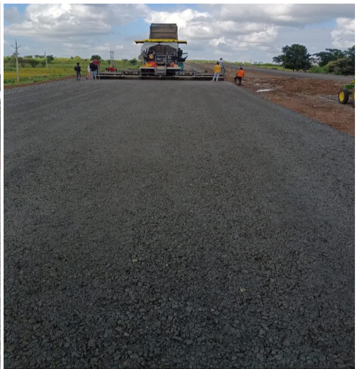
CH:- 105+600 to 106+000 WMM TOP LAYING
