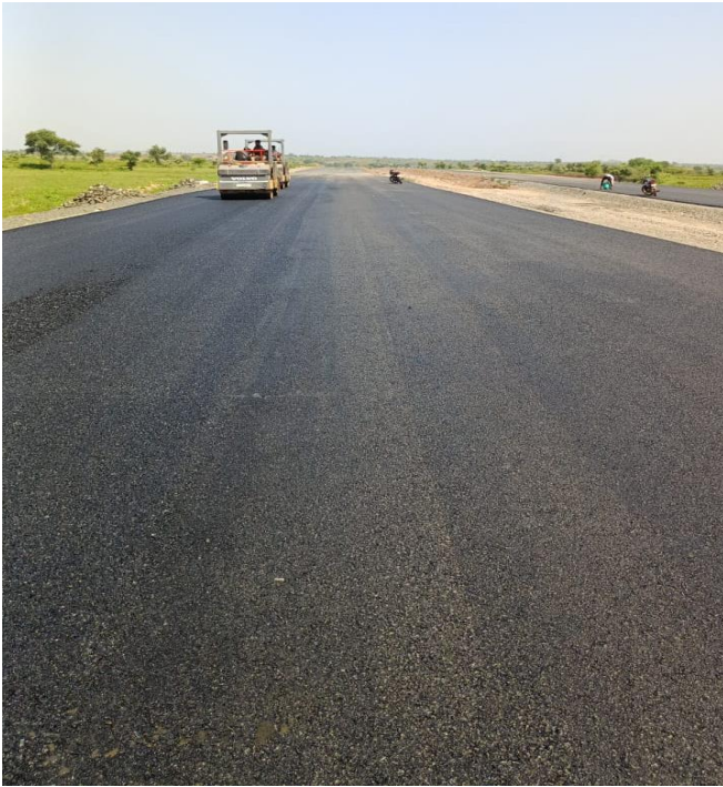
DBM Laying at 115+000 to 115+280
