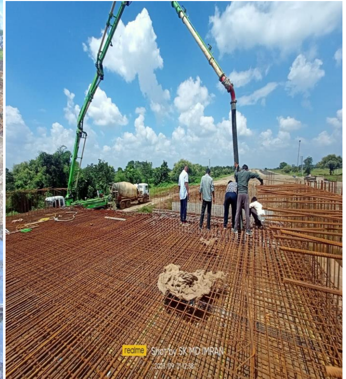
CH:- 99+592 MNB FINAL LIFT WALL CONNCRETE POURING
