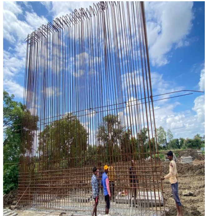
CH:- 127+197 ROB PIER-1 REINFORCEMENT BINDING WIP (LHS)
