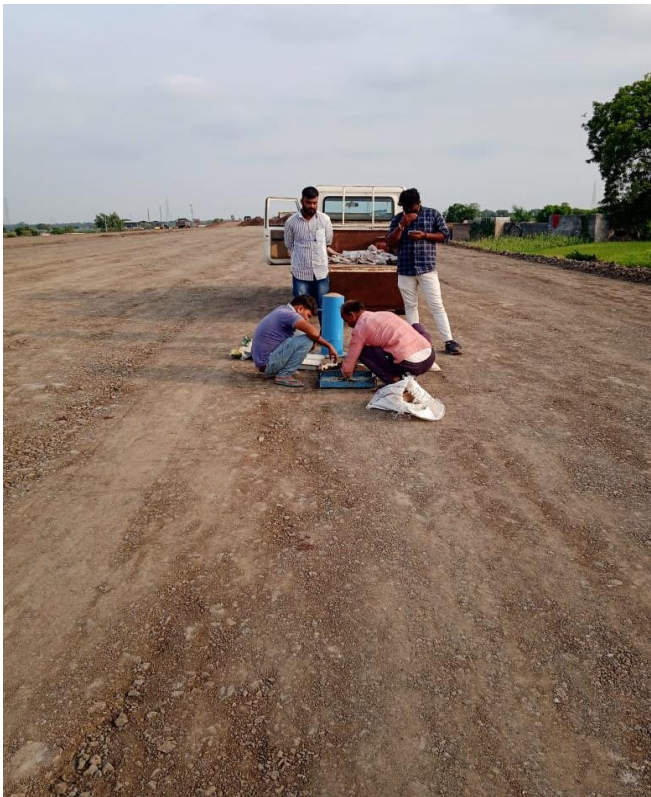
CH:- 110+900 to 111+080 SG TOP FDD CHECKING
