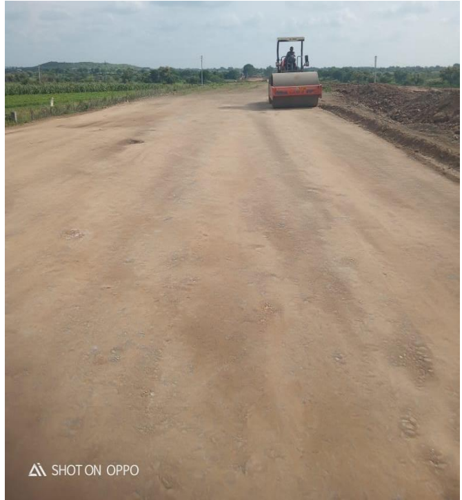
CH:- 114+200 to 114+250 EMBANKMENT 3RD LAYER ROLLING
