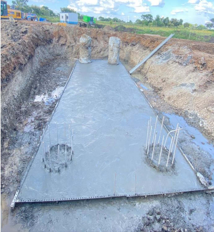
CH:- 127+197 ROB ABUTMENT PILE CAP PCC WIP
