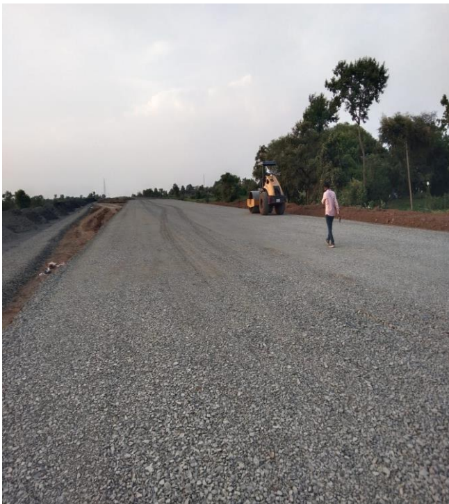
GSB WIP at Ch- 108+250
