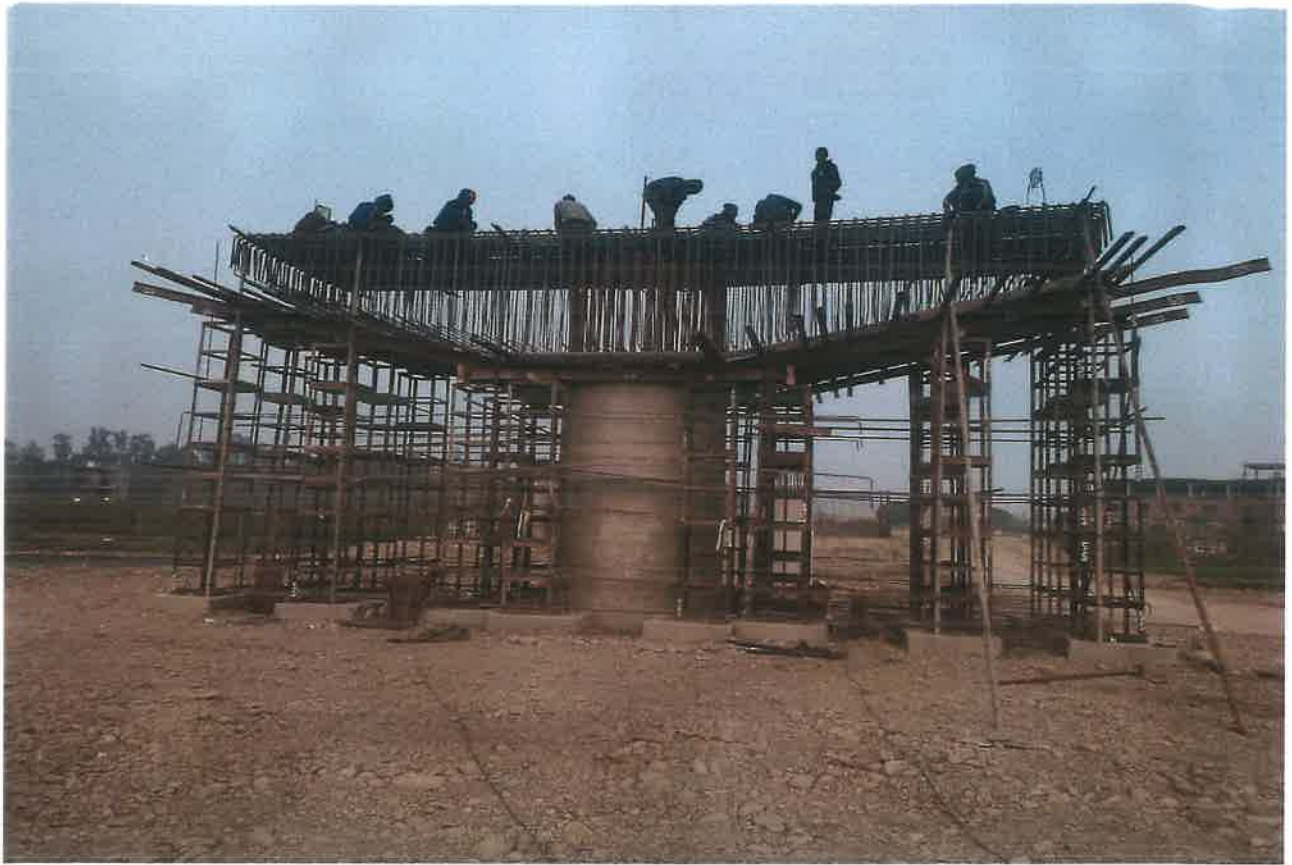
MJB Pier Cap Reinforcement Binding Work in Progress at Ch. 33+033
