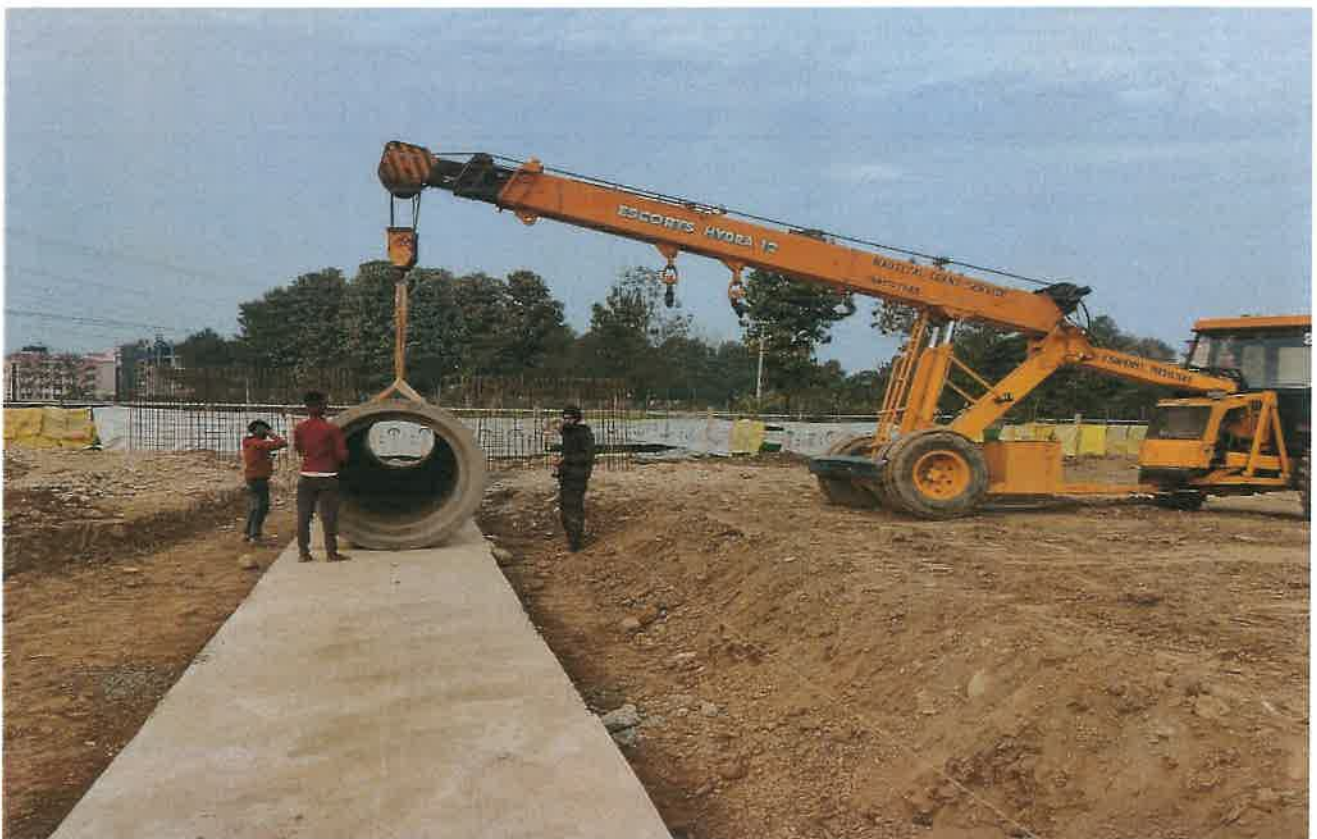
HPC Pipe Laying Work in Progress at Ch. 39+219
