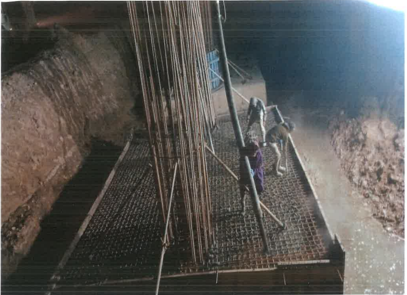
VUP Raft Casting Work in Progress at Ch. 22+598
