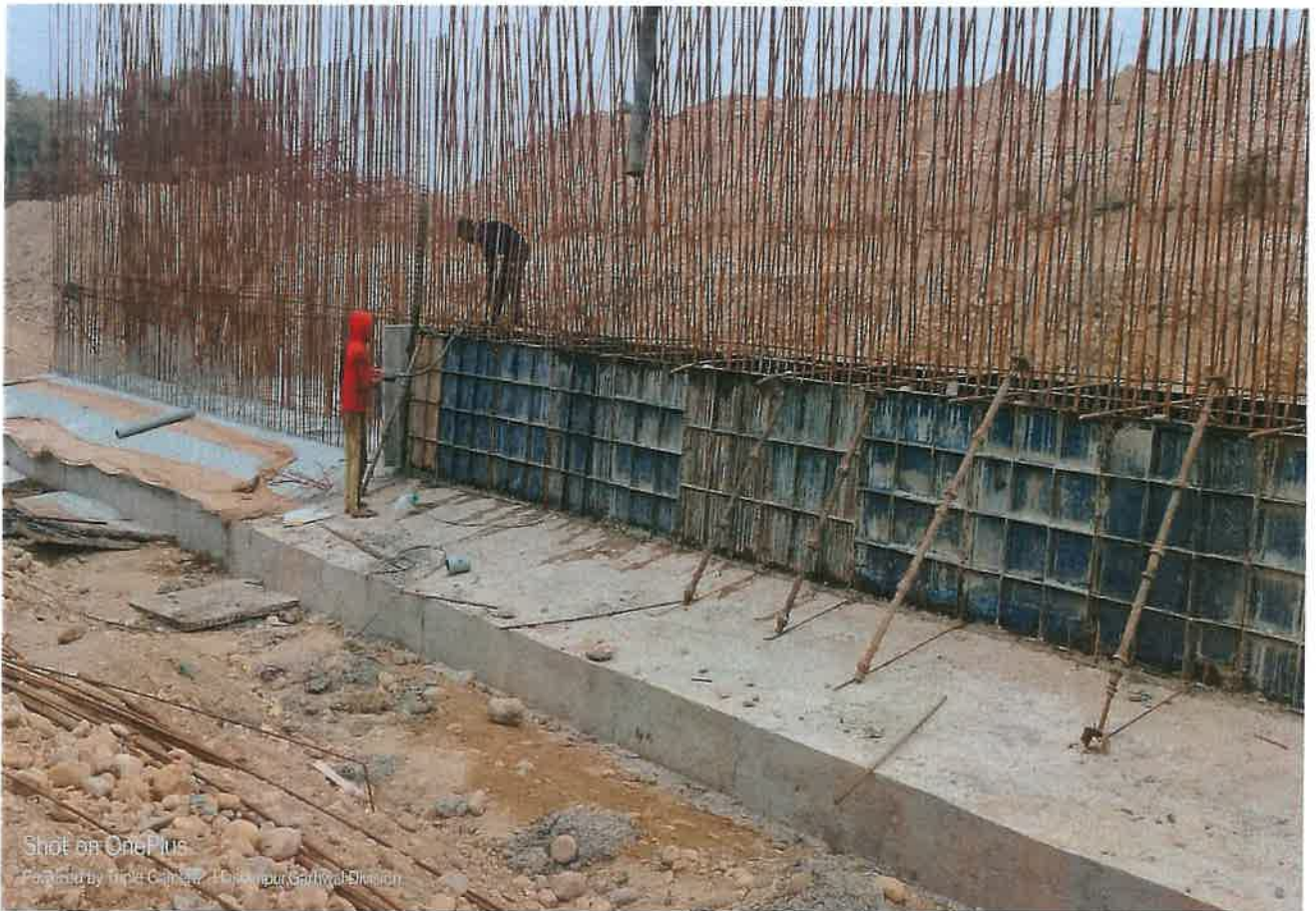
MNB Wall Shuttering Work in Progress at Ch. 28+122
