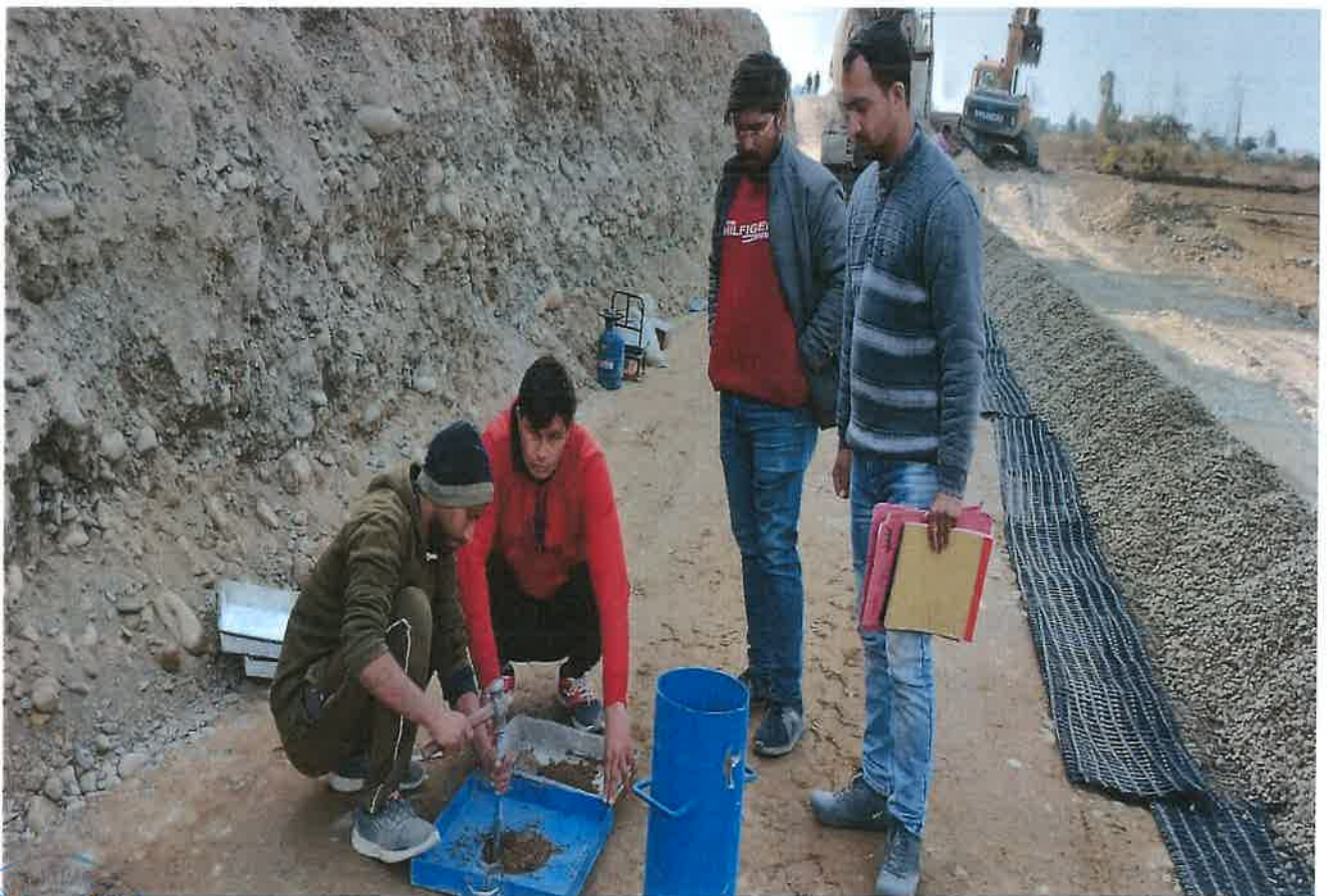
FDD Checking of RE Wall Backfill at Ch. 30+200
