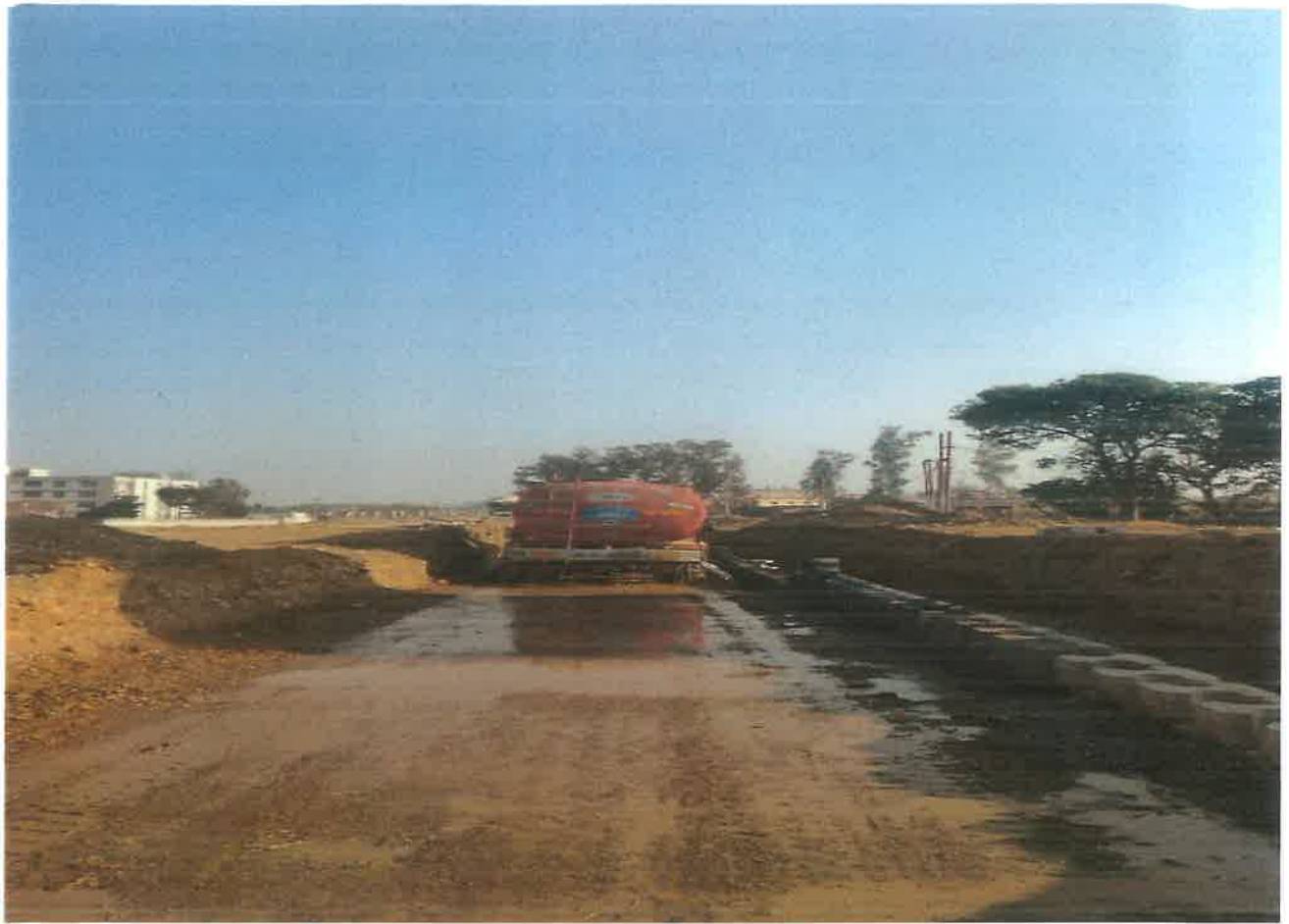
Water Spreading on RE Wall Backfill Bed at Ch. 31+500
