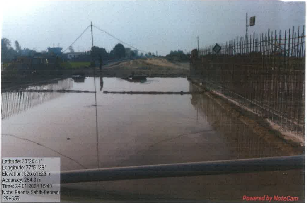
MNB Slab Curing Work in Progress at Ch. 29+659
