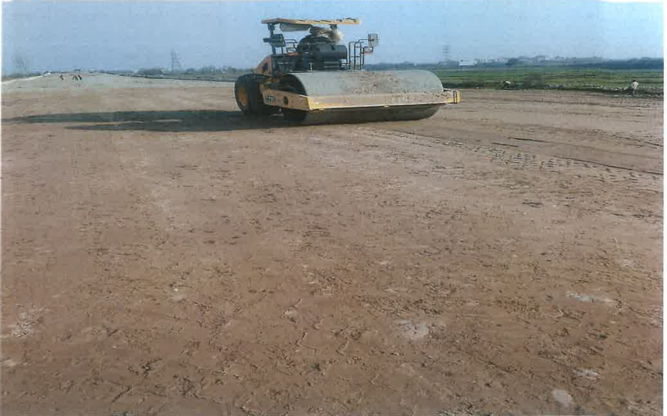
Sub Grade Top Rolling Work in Progress at Ch.29+700
