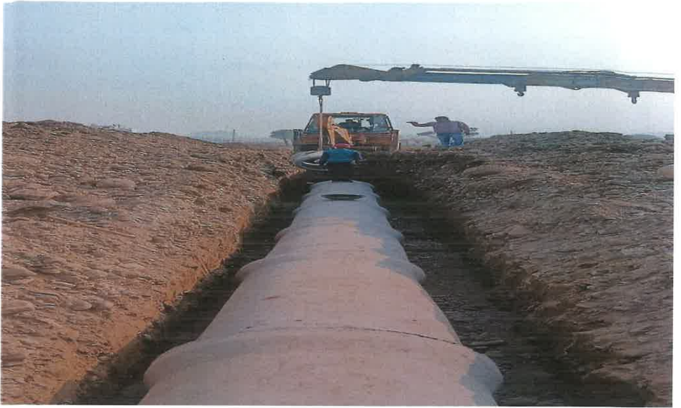
Utility Pipe Laying at Ch. 33+400
