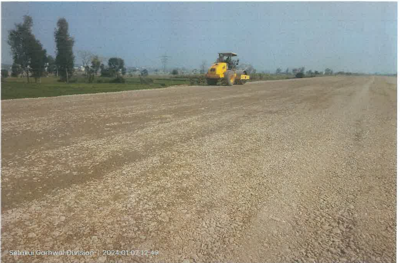
GSB Bed Rolling Work in Progress at Ch. 27+200
