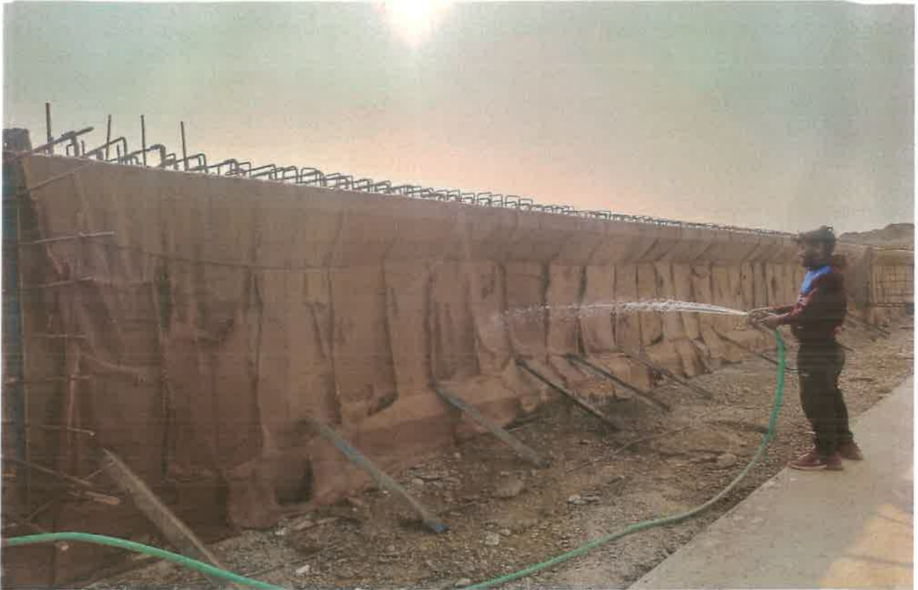
MJB Abutment Girder Curing Work in Progress Ch. 33+033
