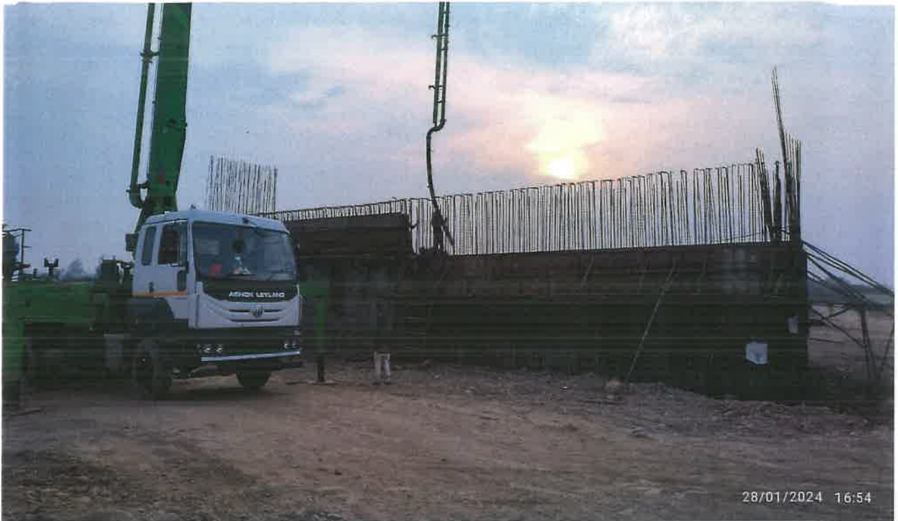
MJB Abutment Wall Casting Work in Progress at Ch. 33+033
