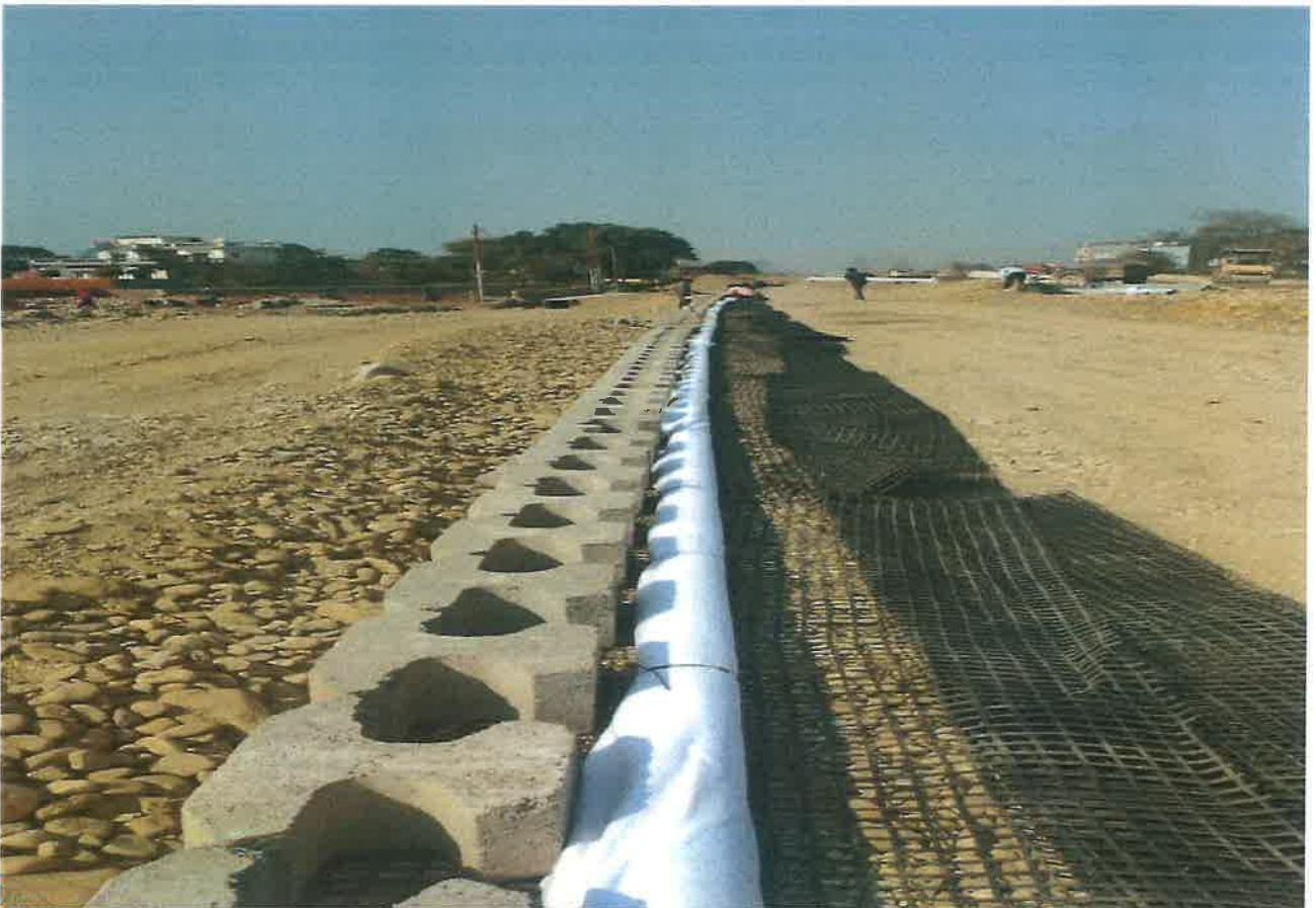
PVC Pipe Laying for Drainage Work in RE Wall
