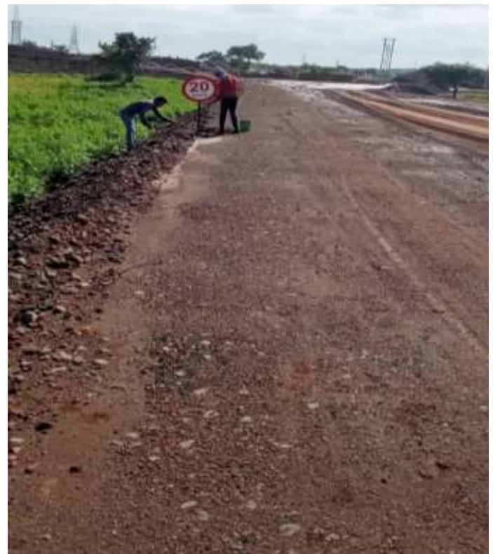
CH:- 109+750 SPEED LIMIT BOARD INSTALLATION
