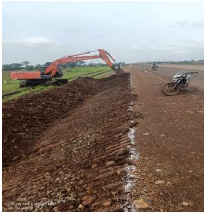
CH:- 110+100 to 110+200 SLOPE CUTTING WIP (LHS)
