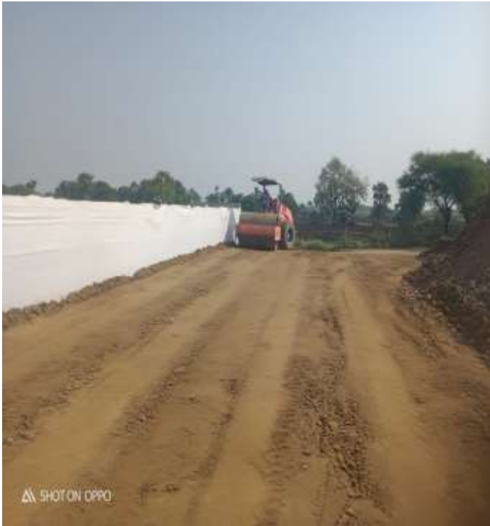
CH. 123+400 BACKFILLING WORK IN PROGRESS
