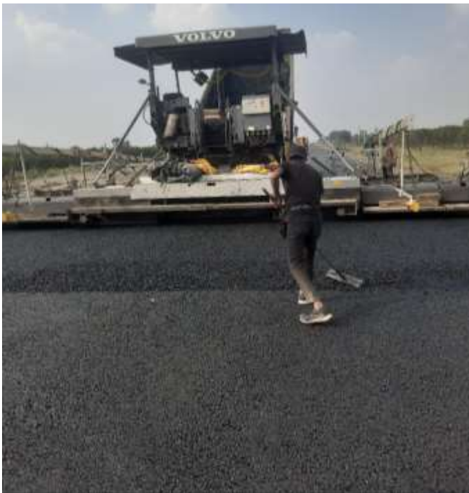
CH. 101+700 DBM LAYING WORK IN PROGRESS
