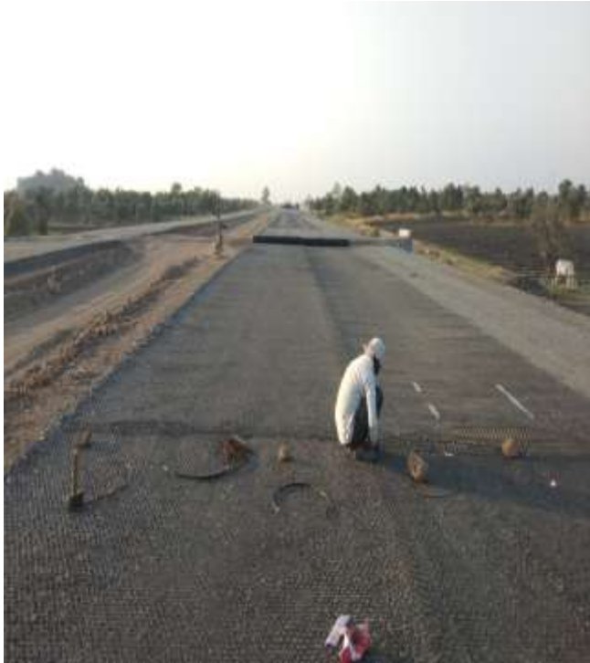
Ch.96+140 to Ch.96+430 GEOGRID LAYING WORK IN PROGRESS
