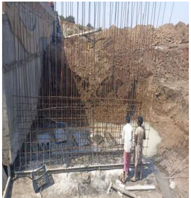
CH. 104+251 RETAINING WALL STEEL BINDING WORK IN PROGRESS
