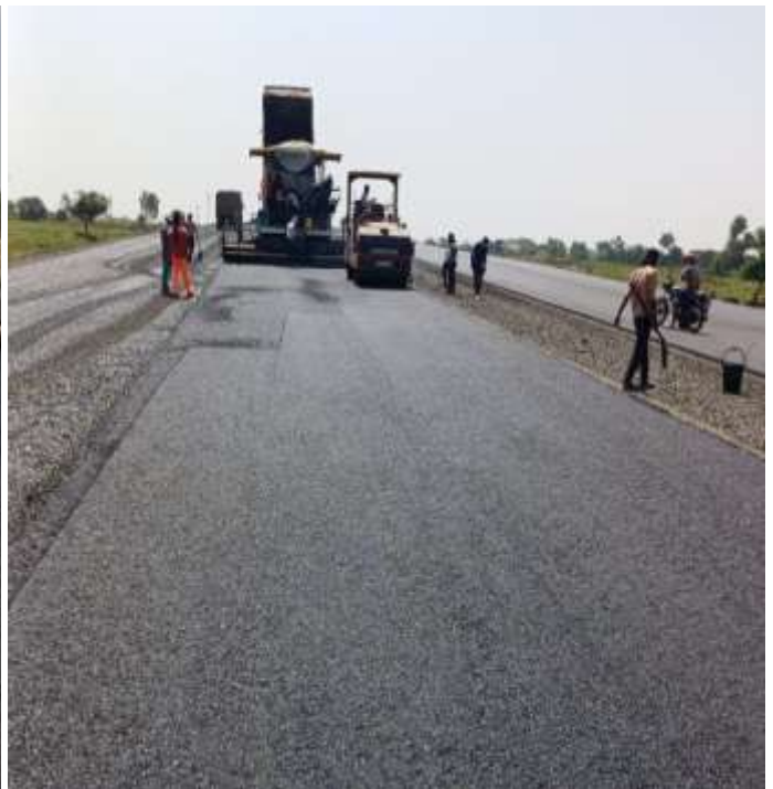
DBM LAYING AT CH. 114+240 TO CH.114+600
