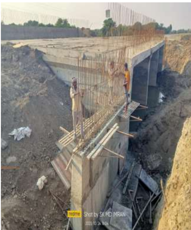
Ch.98+600 MINOR BRIDGE RETAINING WALL CASTING
