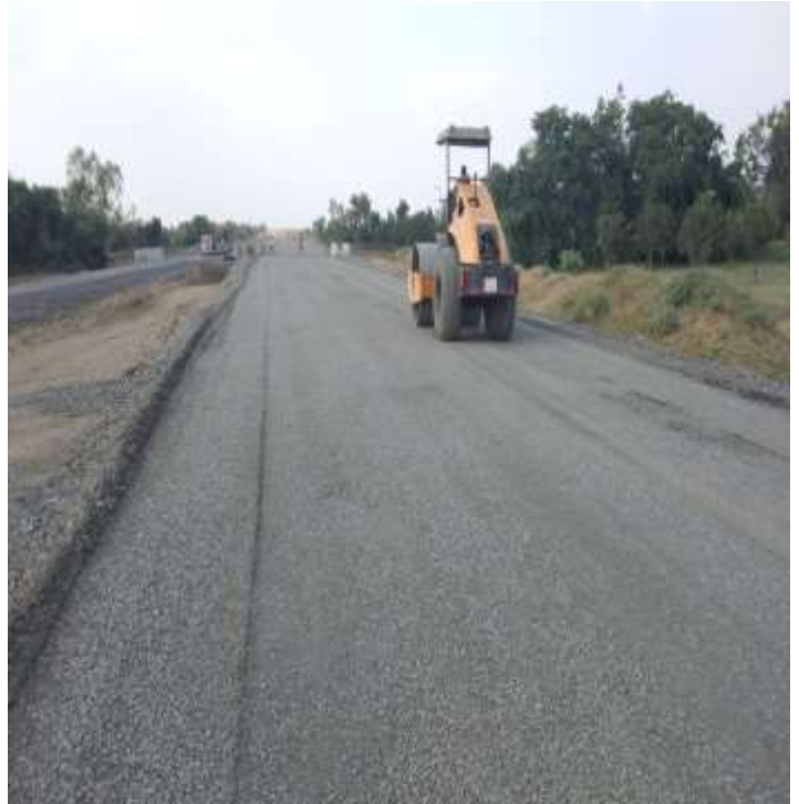
CH. 99+230 TO CH.99+330 WMM LAYING WORK IN PROGRESS
