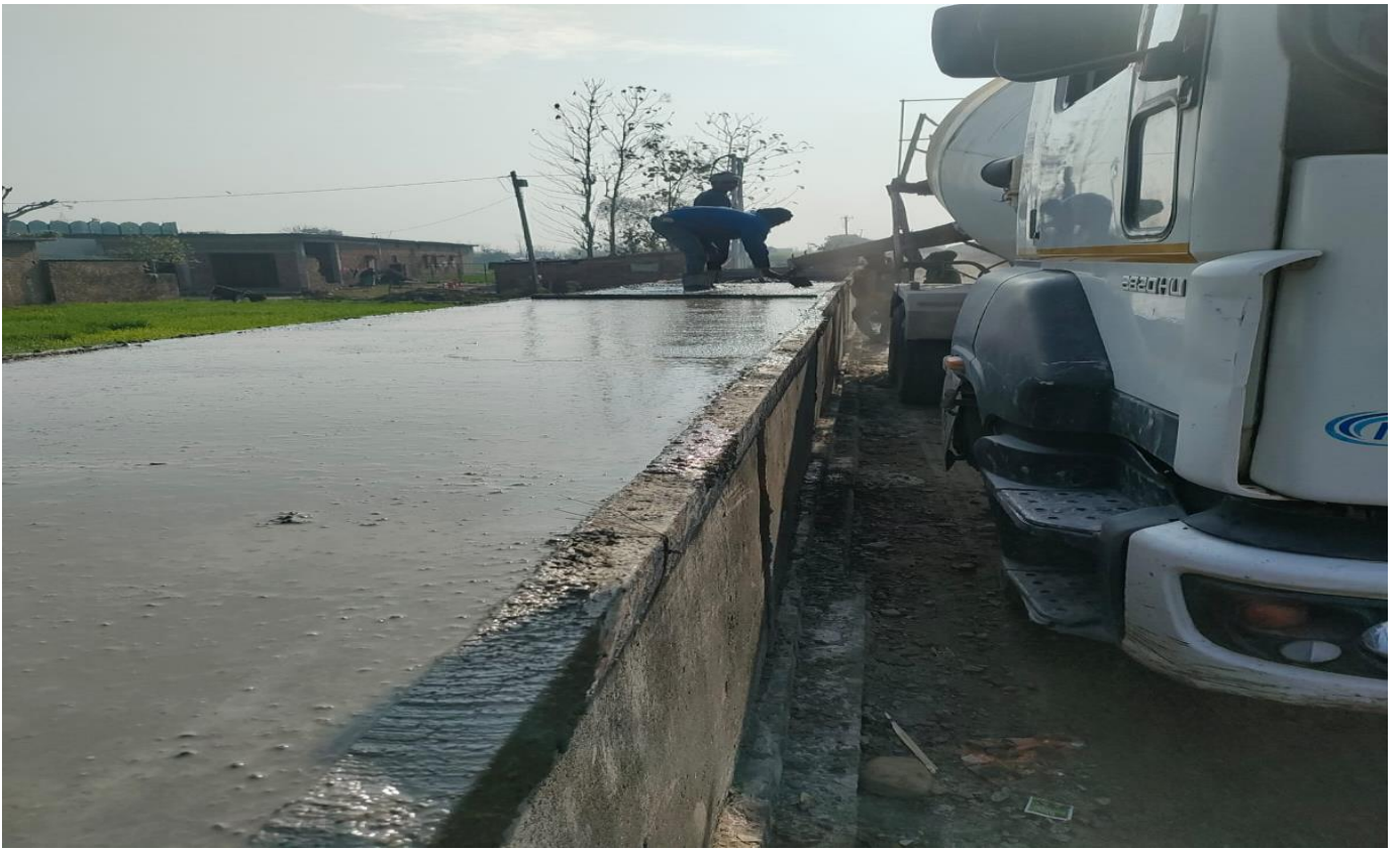
Drain Slab Pouring Work in Progress at Ch. 28+430
