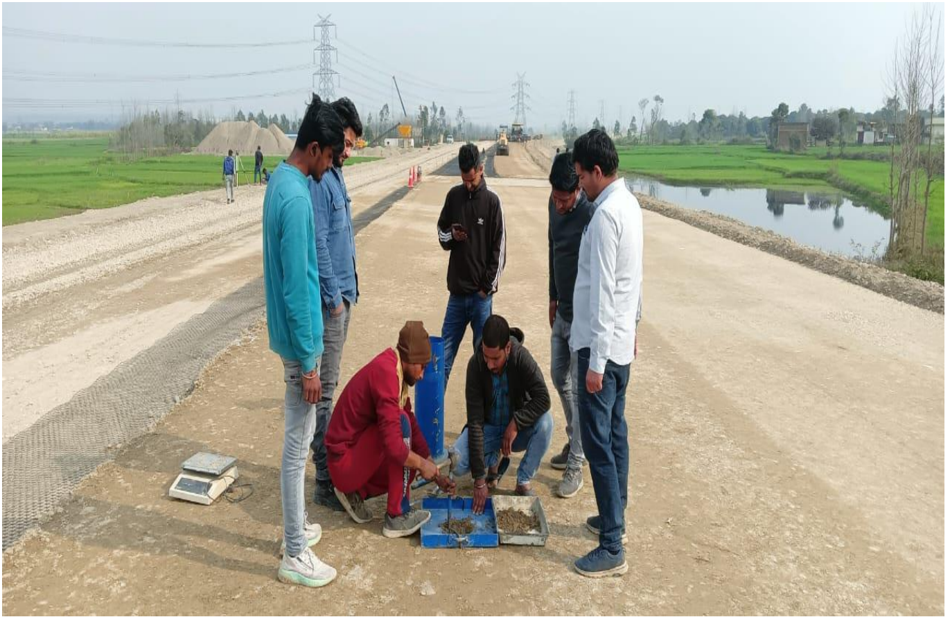
FDD Checking on WMM Top Layer at Ch.19+850
