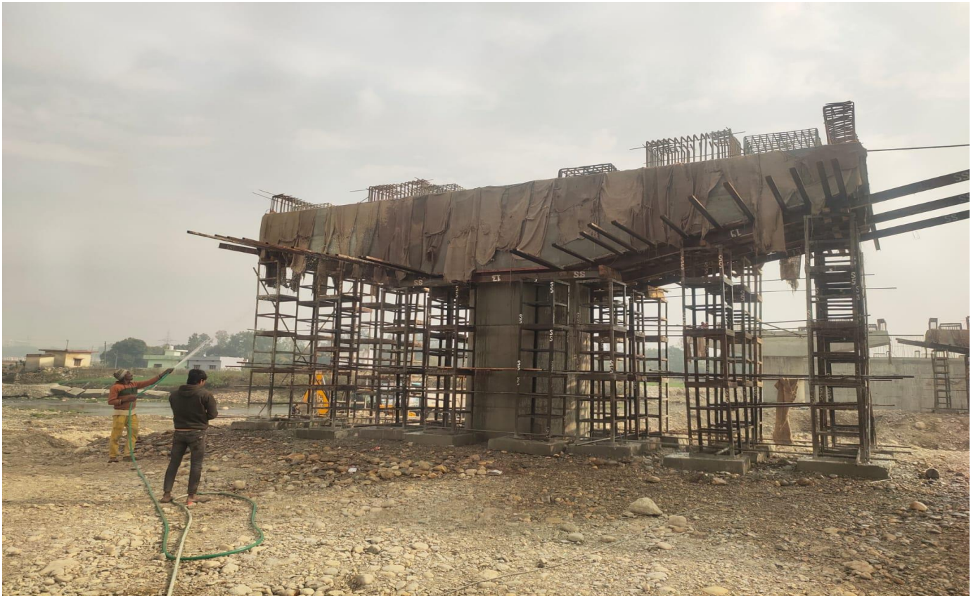
MJB Pier Cap Curing Work in Progress
