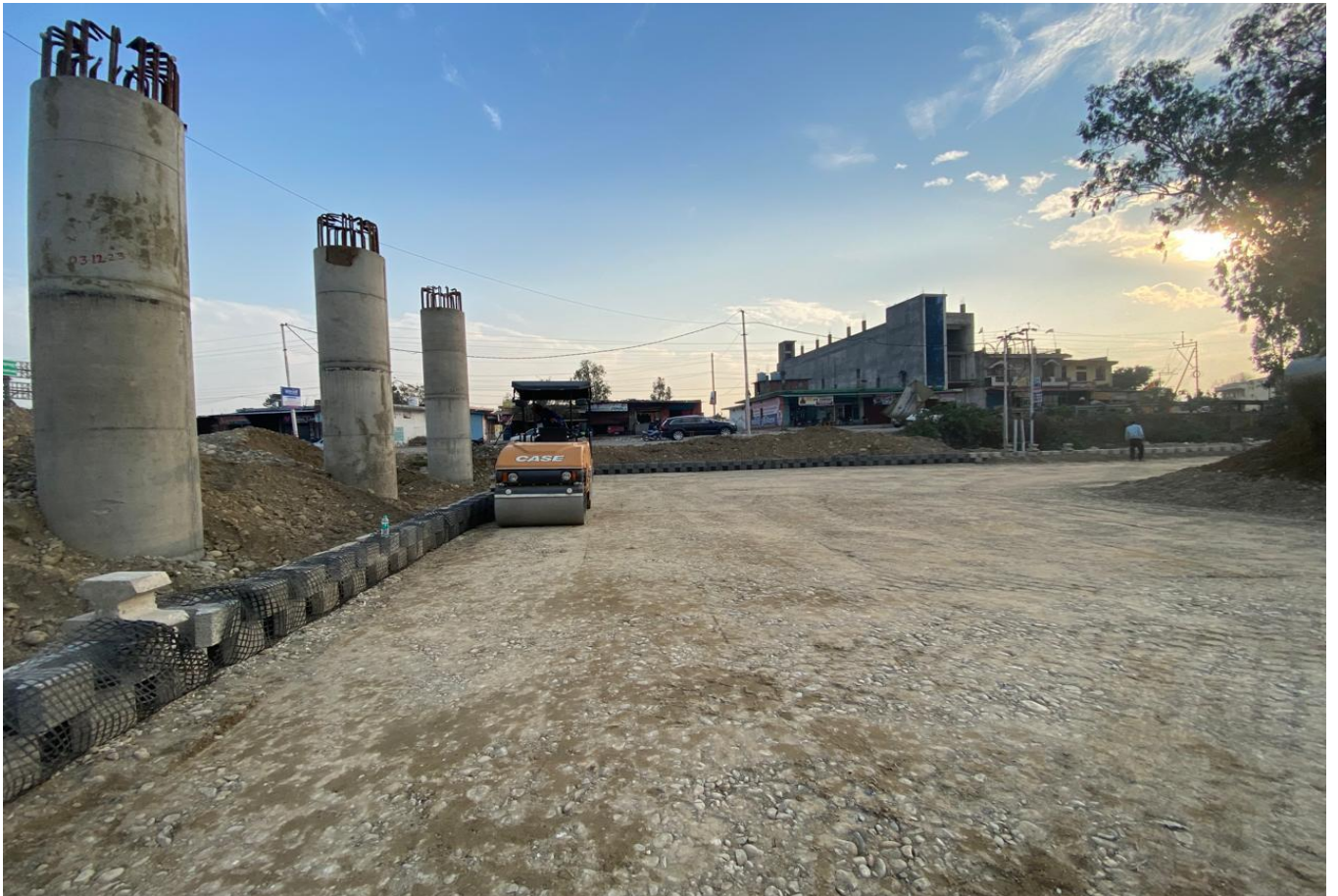
RE Wall Back Fill Material Rolling Work in Progress at Ch. 31+600
