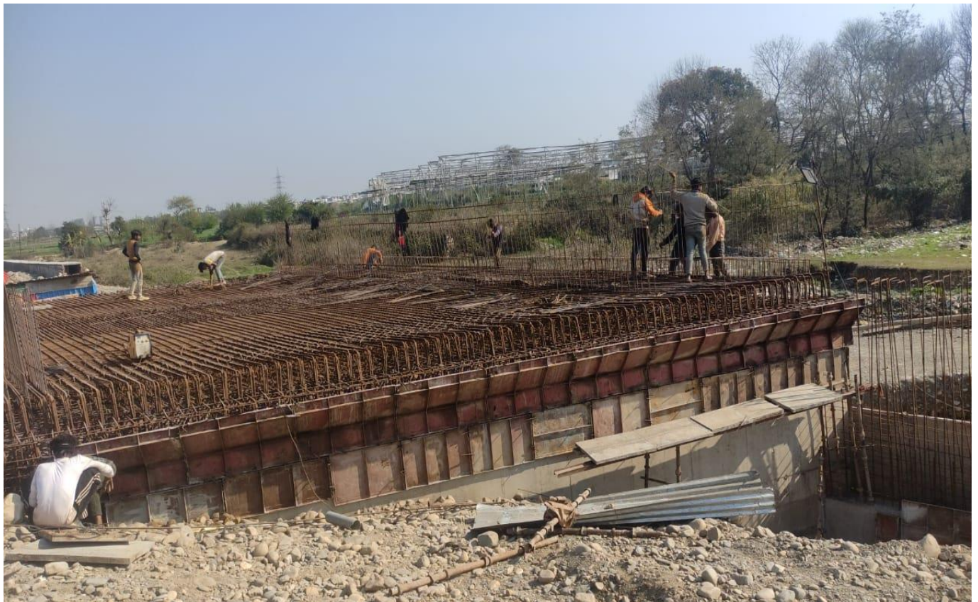
MNB Slab Reinforcement Work in Progress at Ch. 29+659
