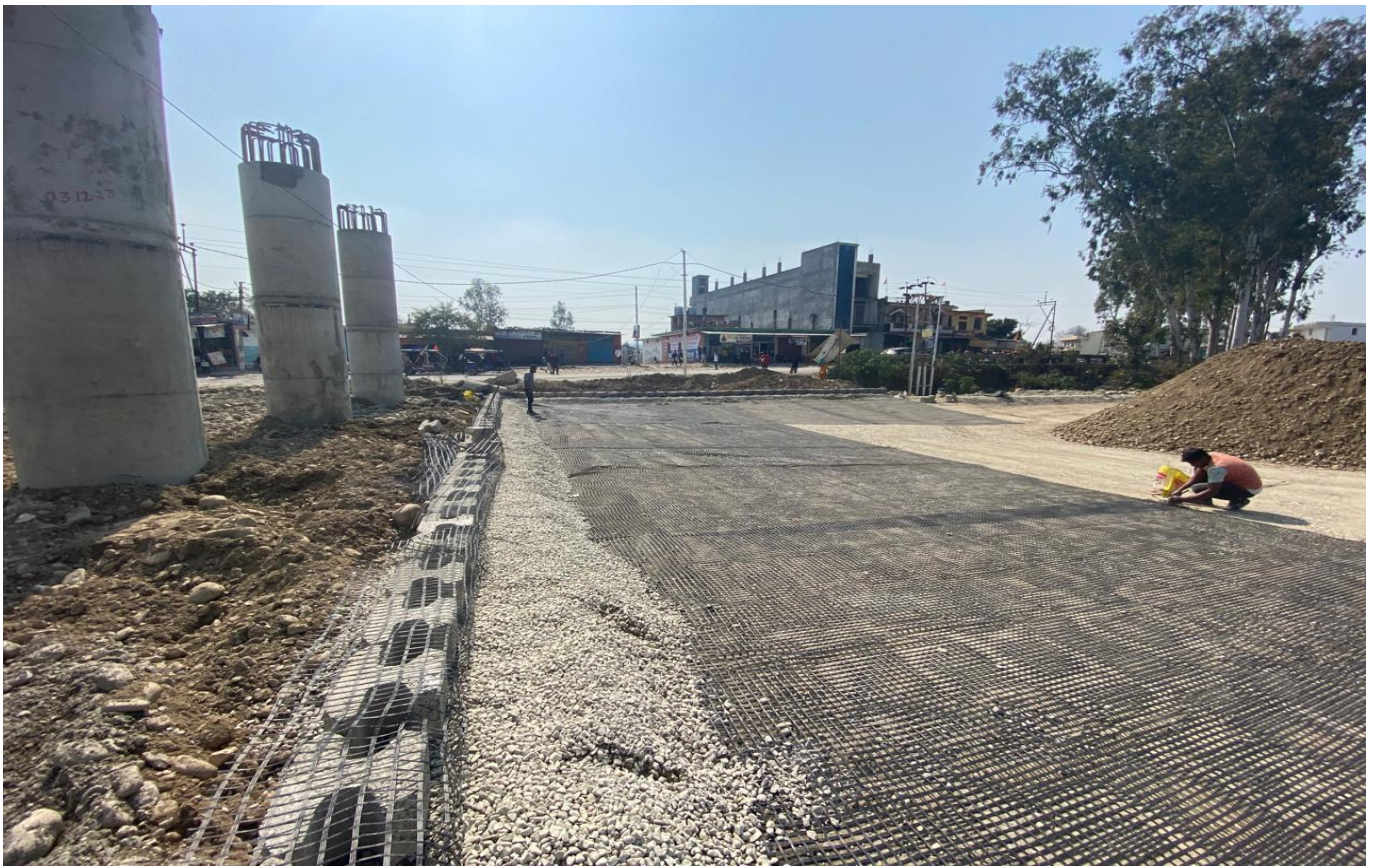
RE Block Erection and Geogrid Laying work in Progress at Ch. 31+650
