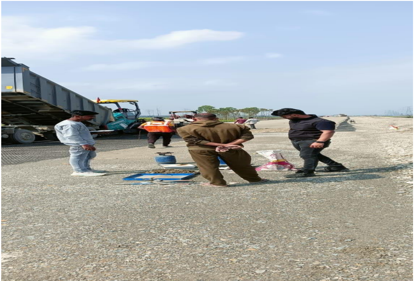
FDD Checking on GSB Top Layer at Ch.22+100
