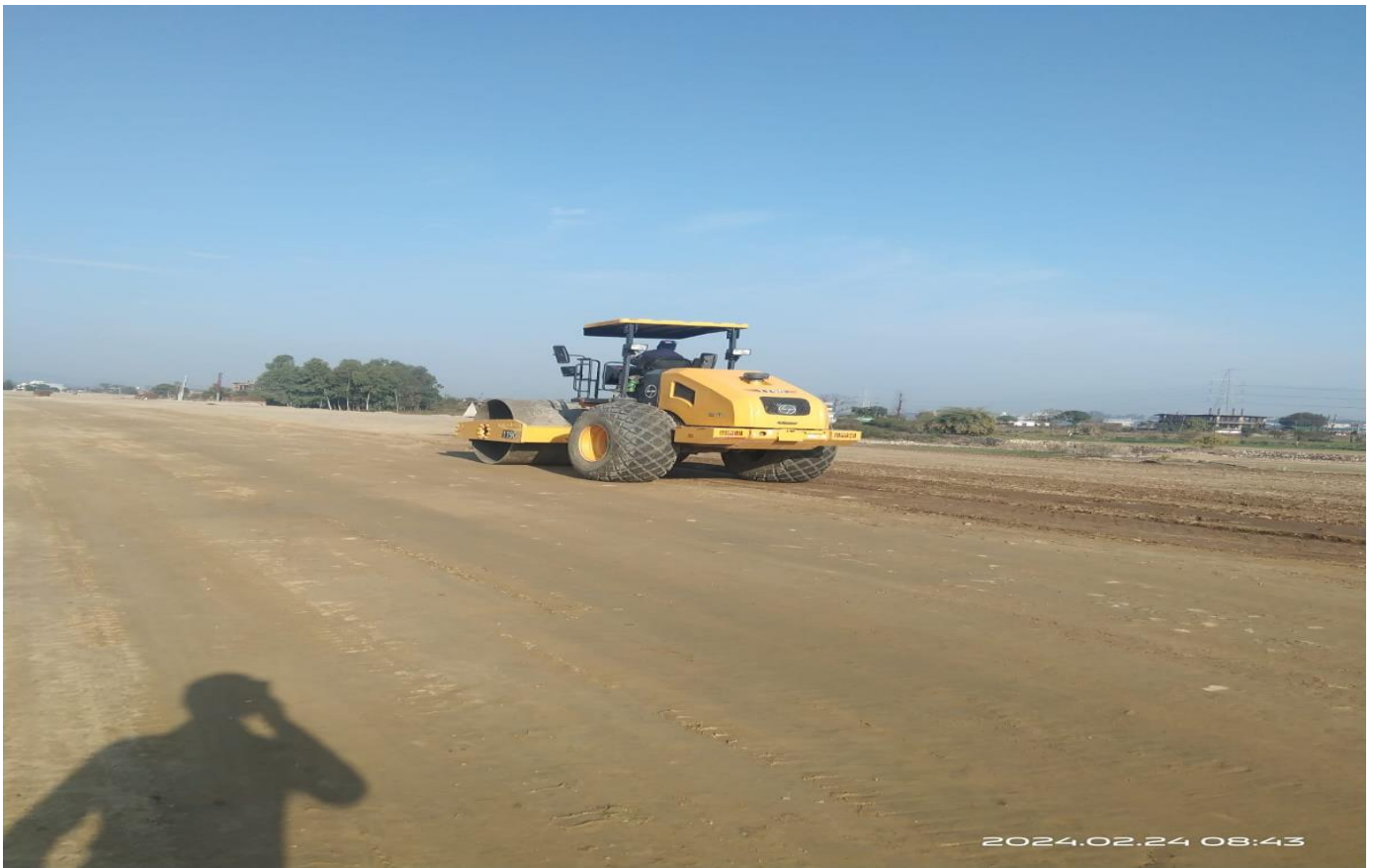
Sub Grade Top Rolling Work in Progress at Ch.29+350
