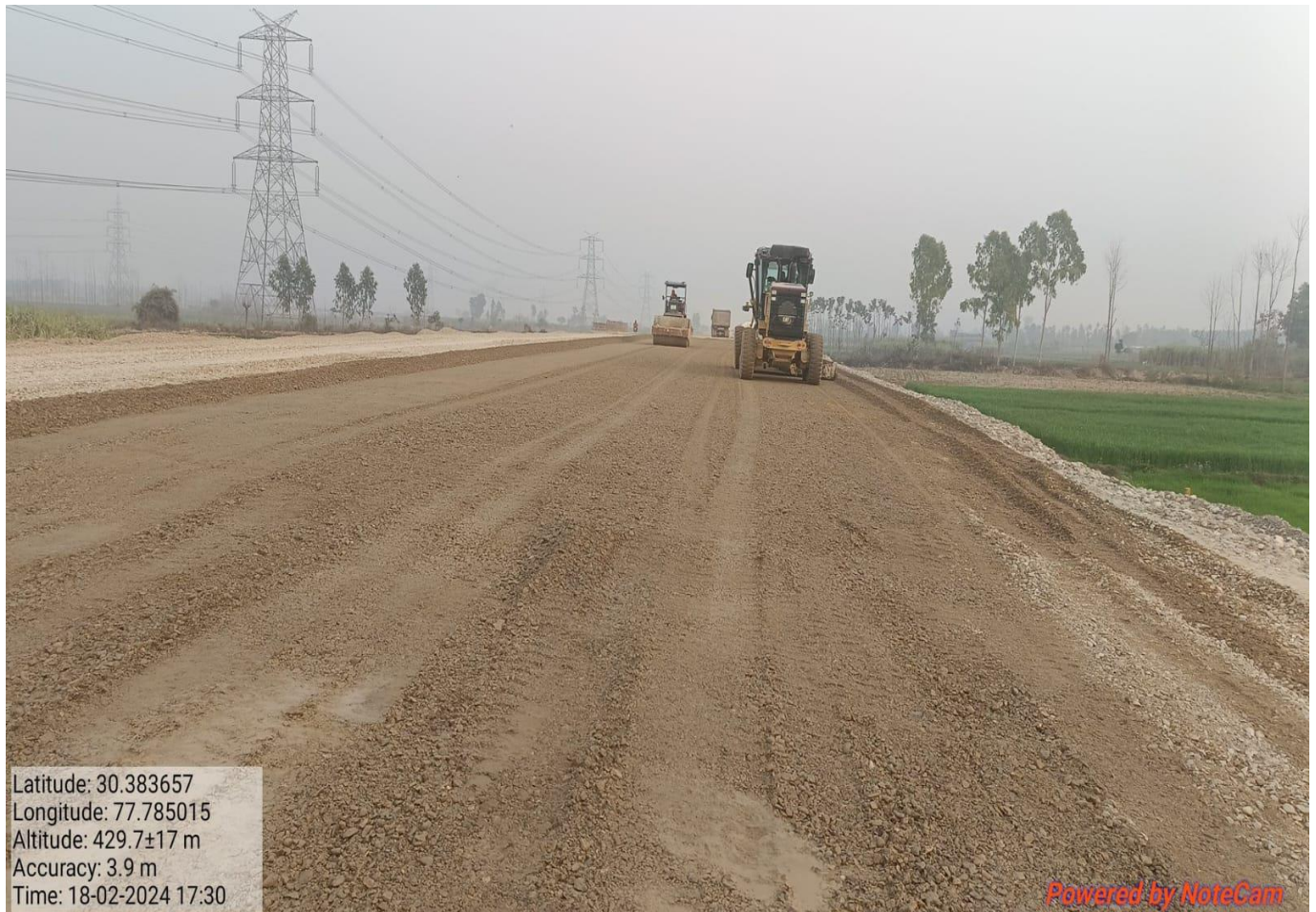
GSB Top Layer Rolling Work in Progress at Ch. 21+700
