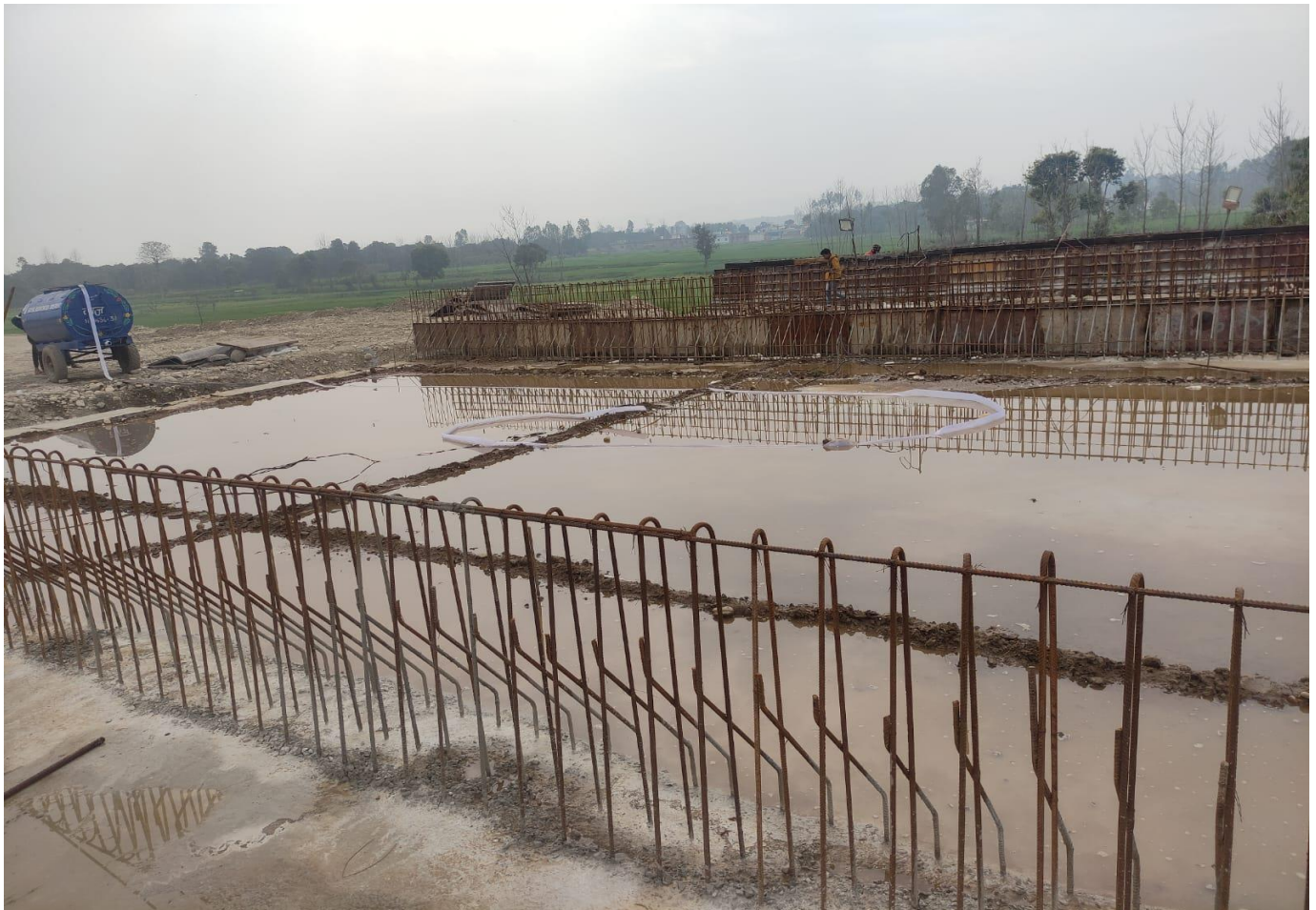
MNB Slab Curing Work in Progress at Ch. 20+163
