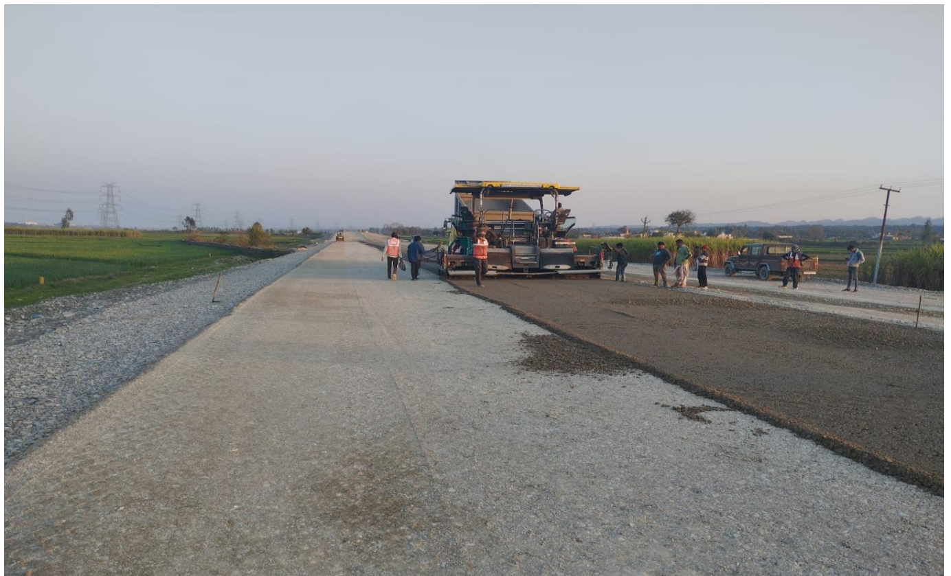
WMM Laying Work in Progress at Ch.23550
