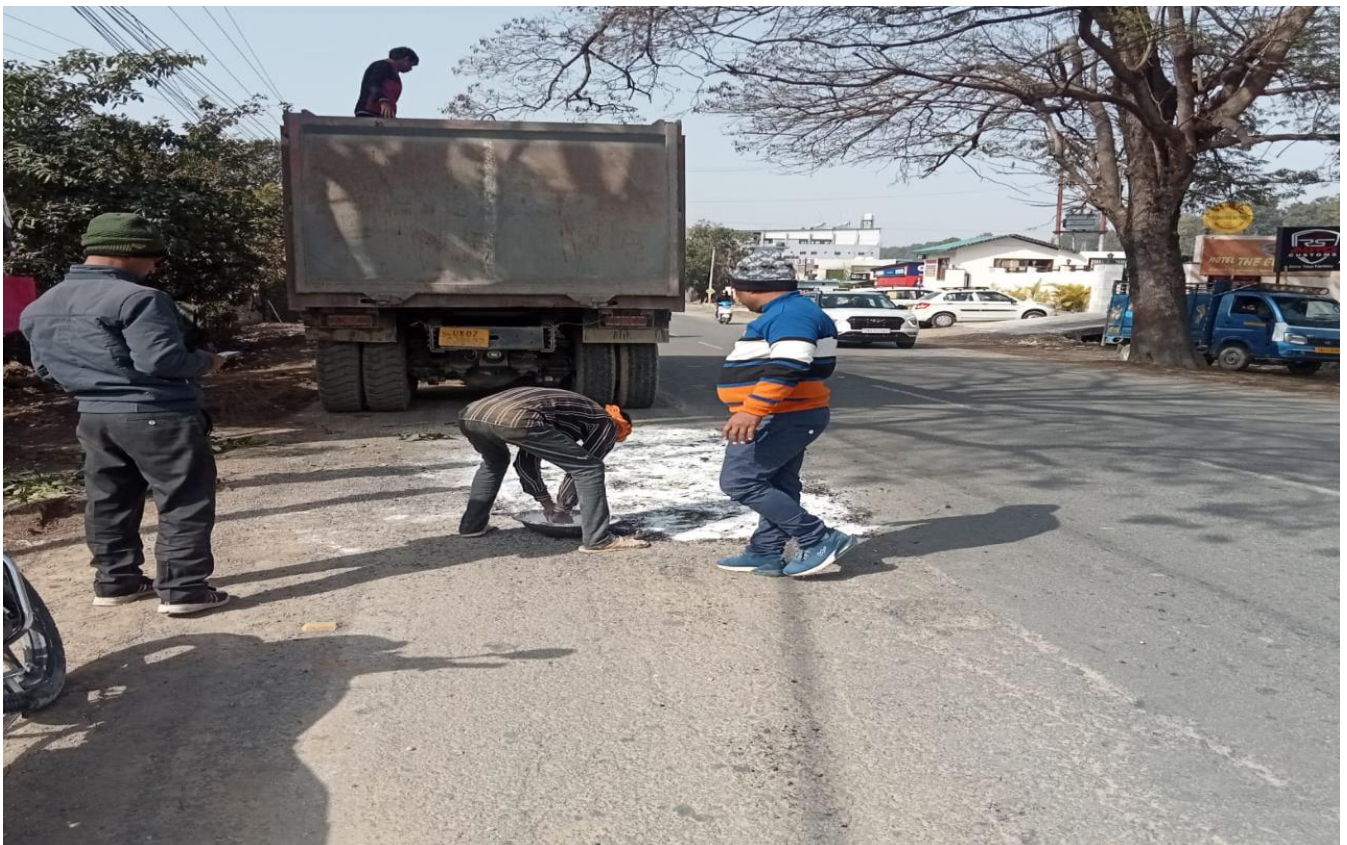
Patch Repairing work is going on at Ch 43+550
