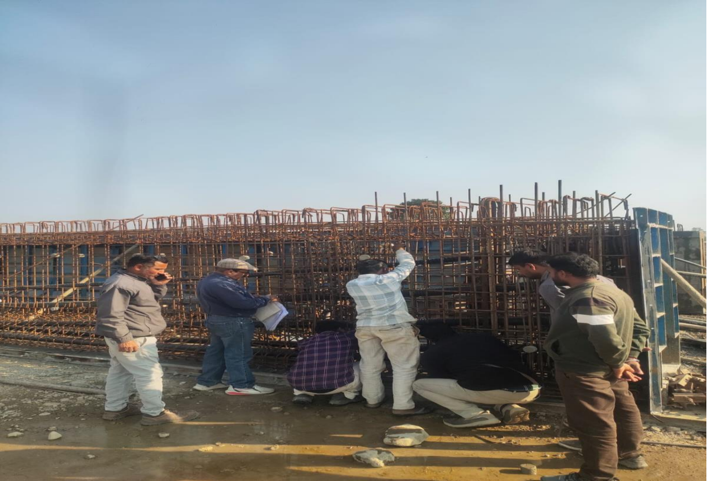
33+033 MJB Girder Profile Checking by BE Sir
