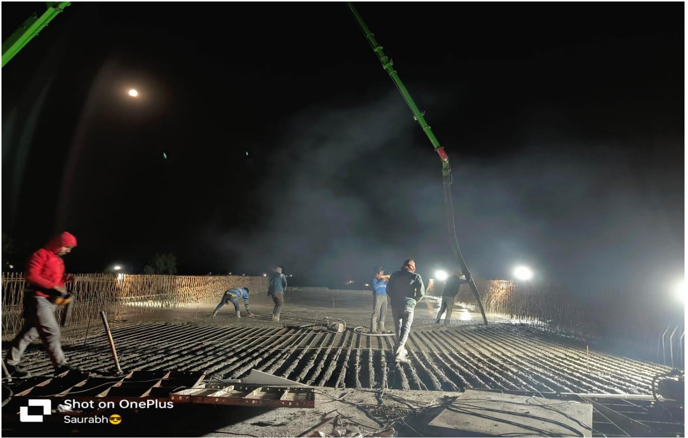
MNB Slab Concrete Pouring Work in Progress at Ch. 28+222
