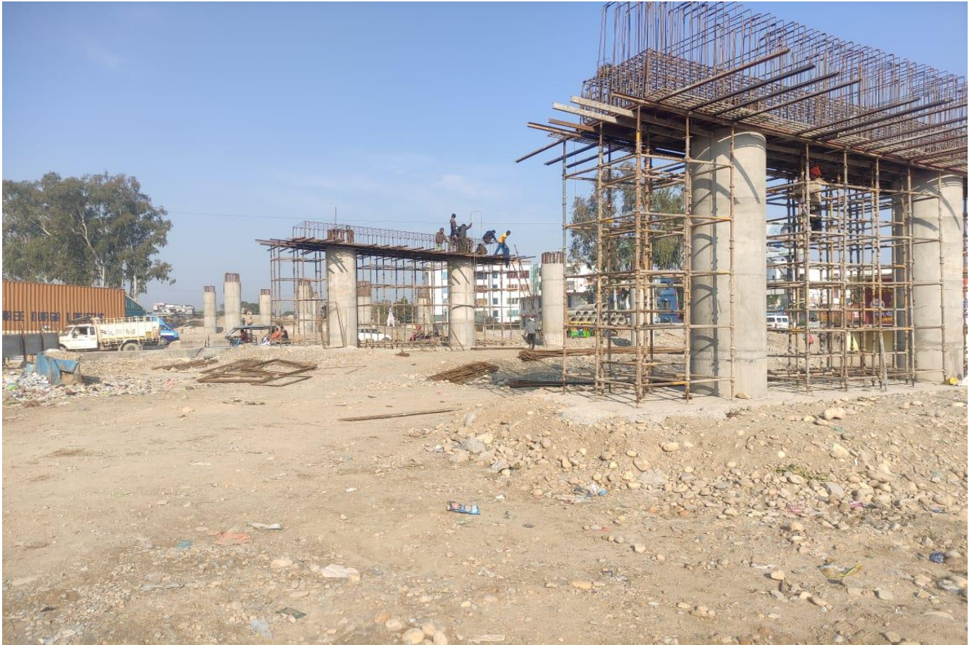
VUP Pier Cap Reinforcement Binding Work in Progress at Ch. 31+691
