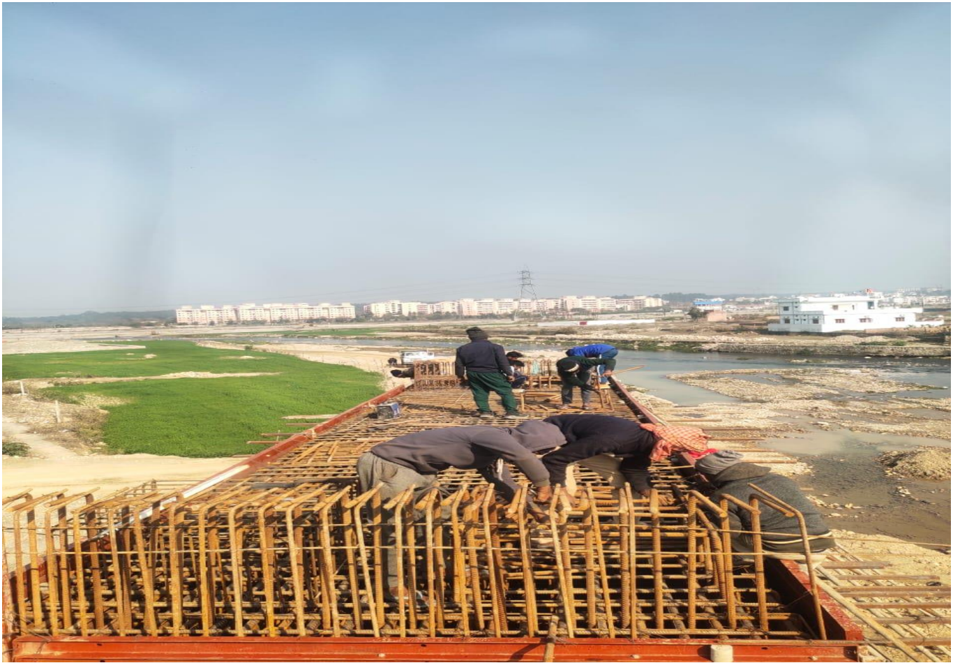
MJB Pier Cap Pedestal & Seismic Restrainer Reinforcement Binding work in Progress
