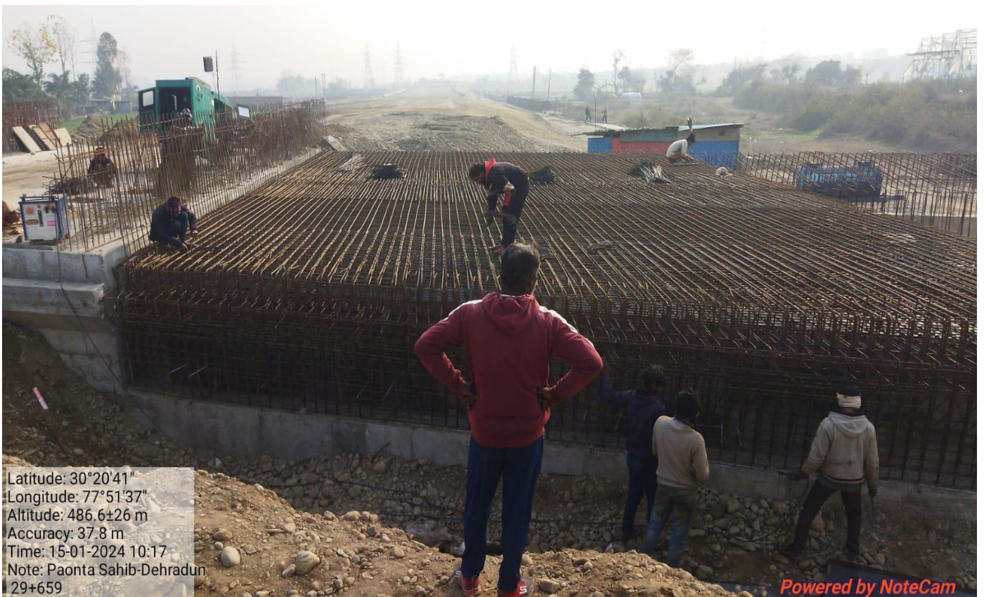
MNB Slab Curing Work in Progress at Ch. 29+659
