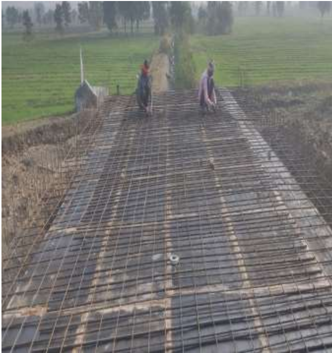
CH.120+150 SLAB REINFORCEMENT WORK IN PROGRESS
