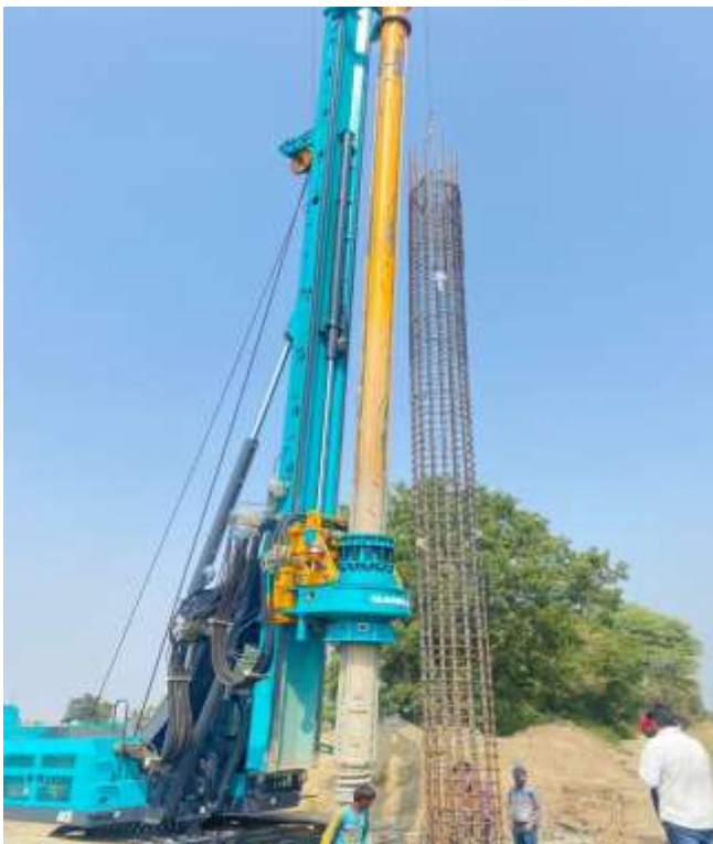
ROB PILE CAGING WORK IN PROGRESS
