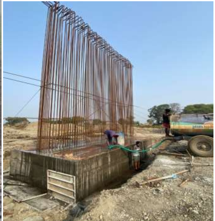
ROB P4 PILE CAP CURING WORK IN PROGRESS (RHS)
