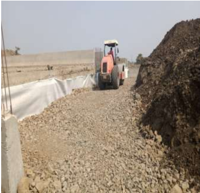
MNB BACKFILLING WORK IN PROGRESS
