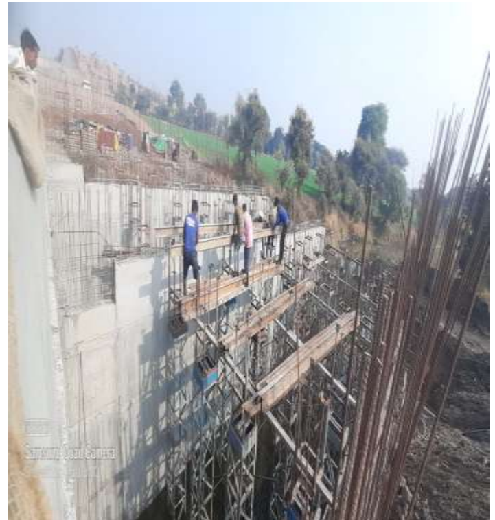
CH.116+595 SLAB STAGGING WORK IN PROGRESS
