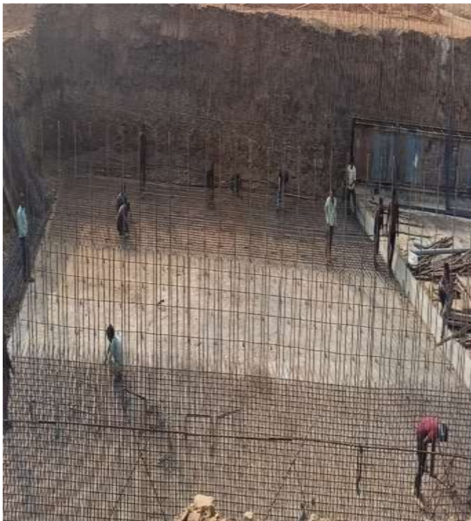
CH. 109+670 LVUP RAFT RENINFORCEMENT WORK IN PROGRESS
