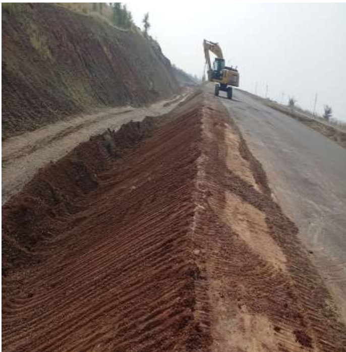
CH. 107+370 SLOPE CUTTING WORK IN PROGRESS
