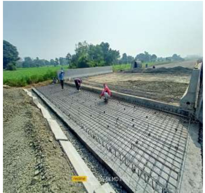
CH. 99+345 APPROACH SLAB WORK IN PROGRESS
