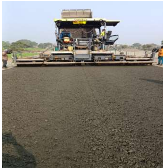
CH. 116+220 WMM TOP LAYING (LHS)
