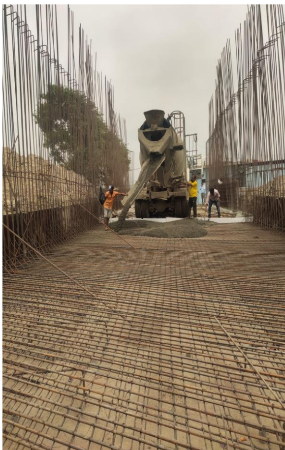
Box Culvert Raft Concrete Pouring Work in Progress at Ch. 31+370
