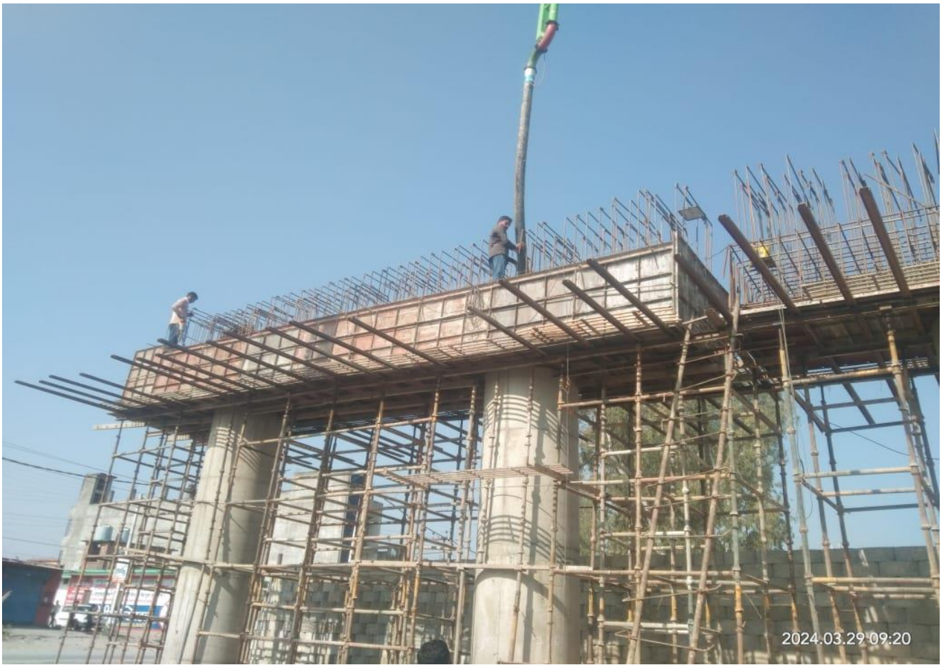
VUP Pier Cap Concrete Pouring Work in Progress at Ch. 31+691
