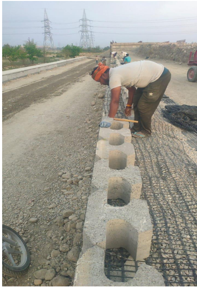
RE Block Erection Work in Progress at Ch. 30+200
