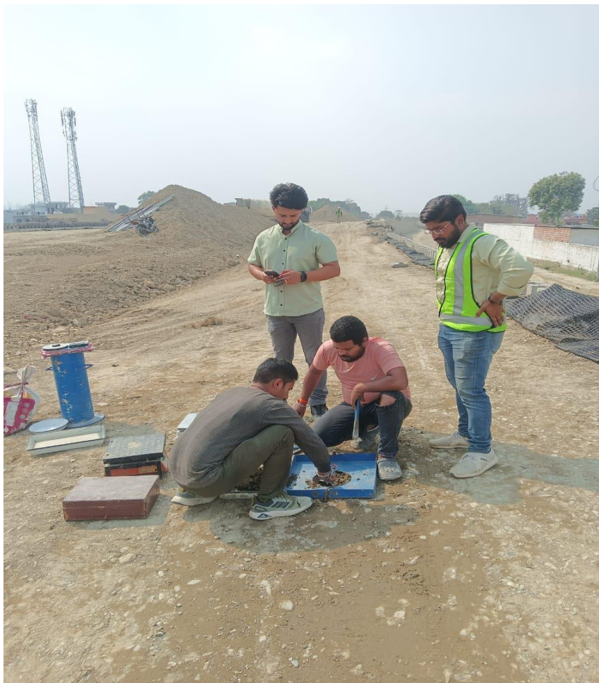
FDD Checking on RE Wall Back Fill Bed at Ch. 31+400
