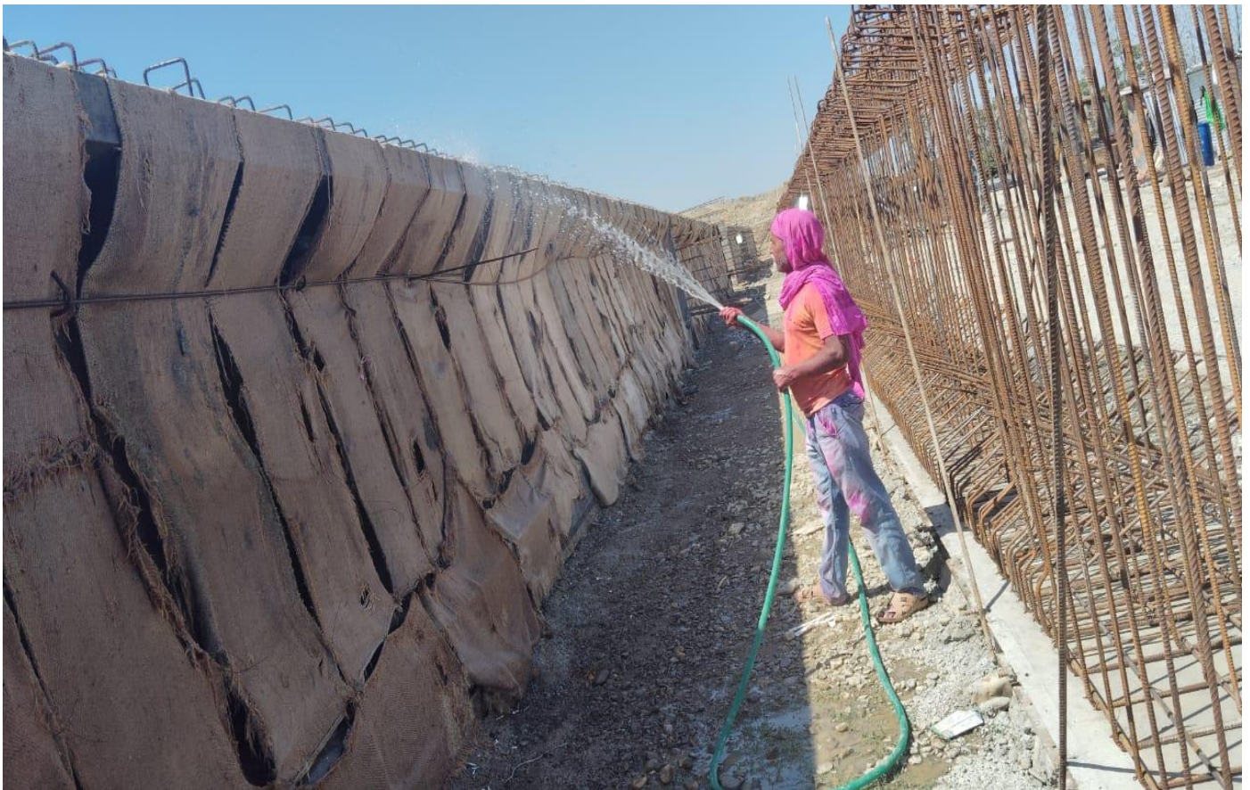
MJB Girder Curing Work in Progress
