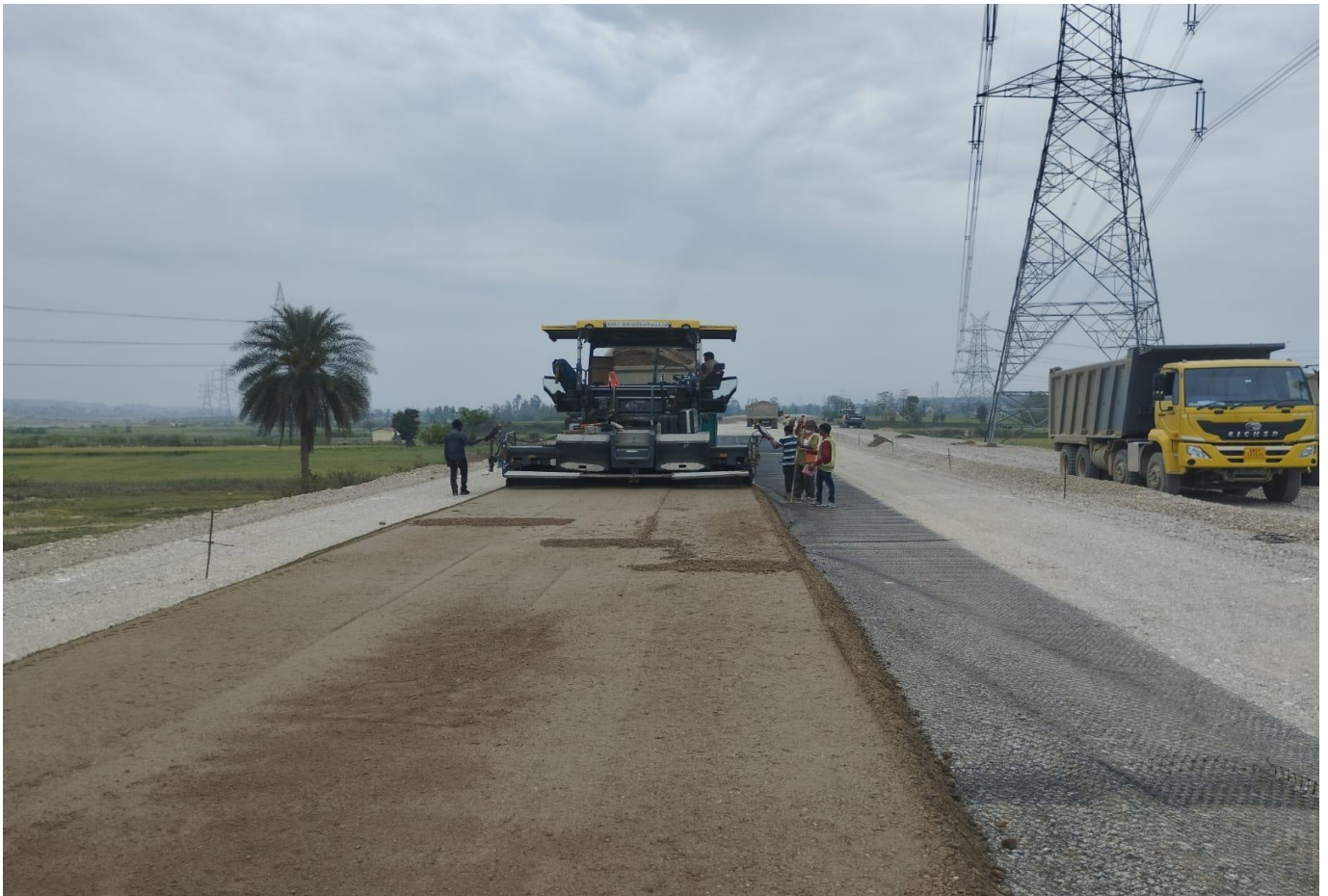
WMM Laying Work in Progress at Ch. 26+300
