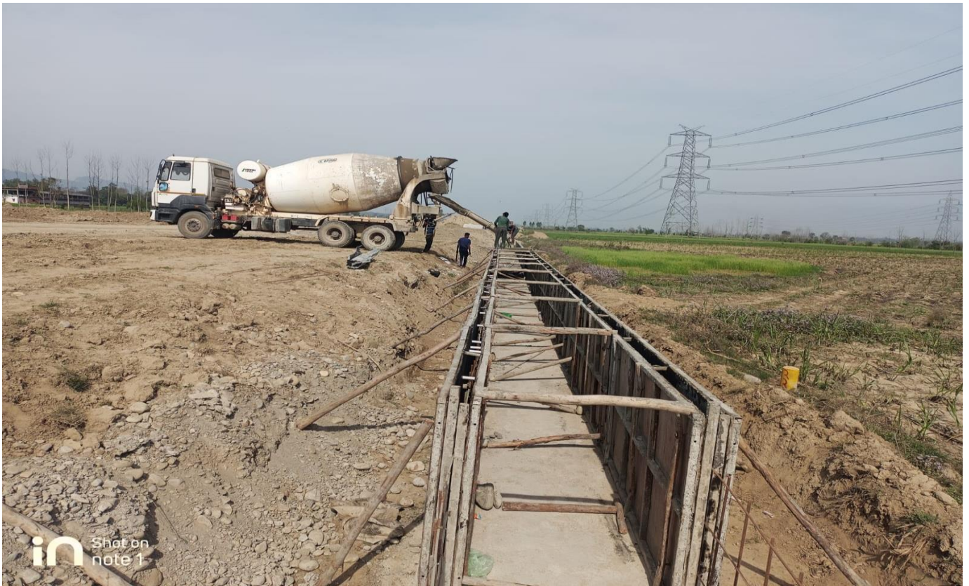
Drain Wall Pouring Work in Progress at Ch. 22+500
