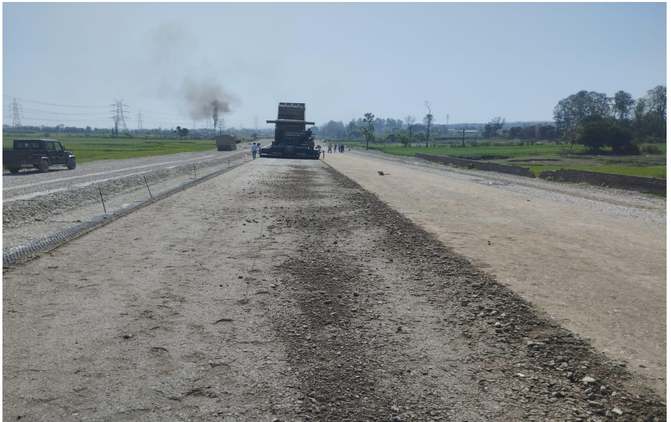
WMM Laying Work in Progress at Ch.24+750
