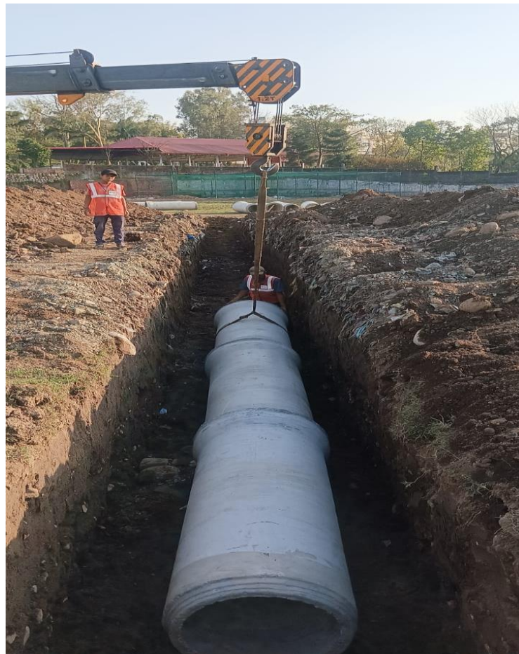
Utility Pipe Laying at Ch. 39+350
