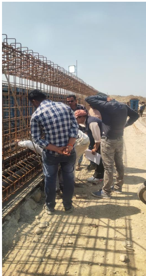
33+033 MJB Girder Profile Checking by BE Sir
