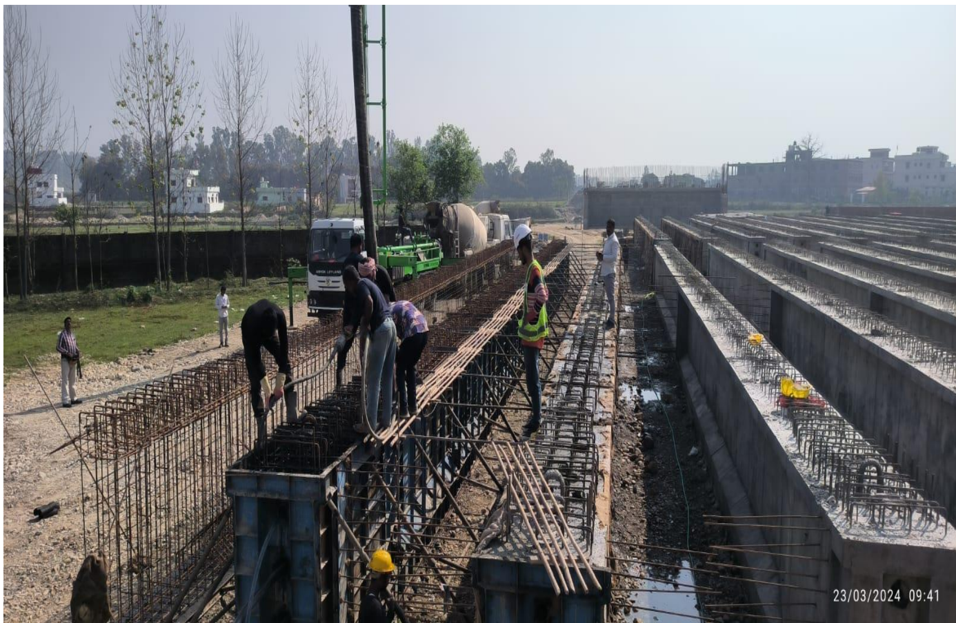
MJB Girder Concrete Pouring Work in Progress Ch. 33+033
