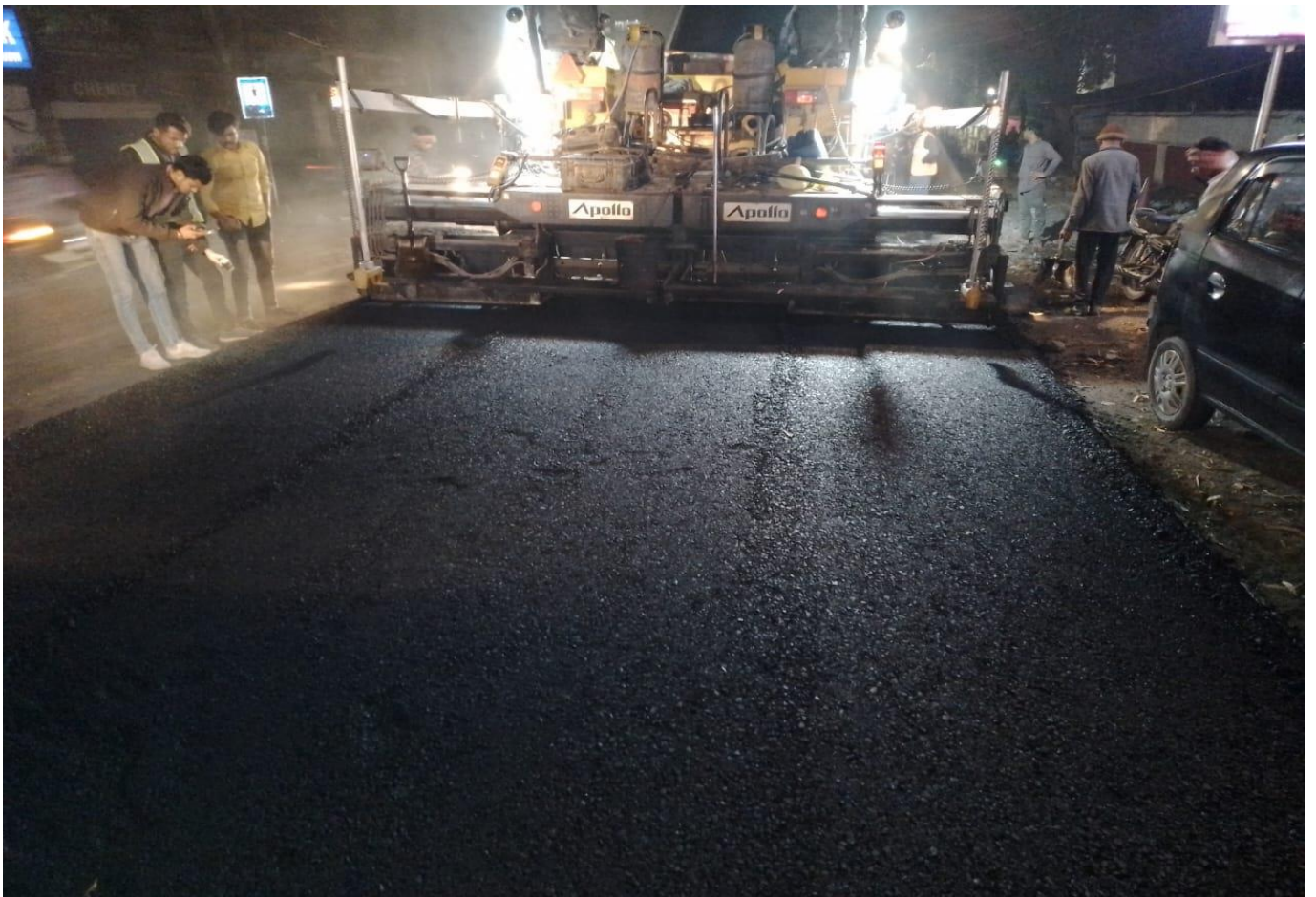
DBM Laying Work in Progress at Ch. 43+300
