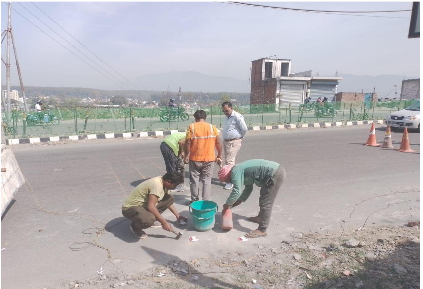
Road Stud Installation Work in Progress at Ch. 40+100
