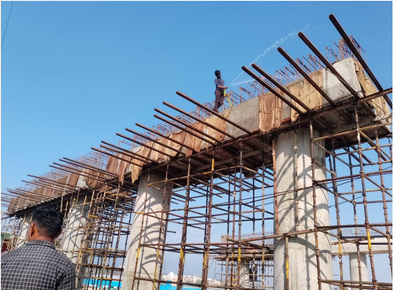
VUP Pier Cap Curing Work in Progress at Ch. 31+691
