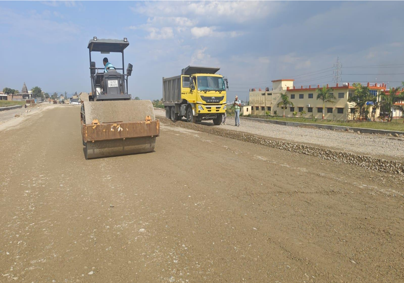
GSB Top Rolling Work in Progress at Ch.29+700
