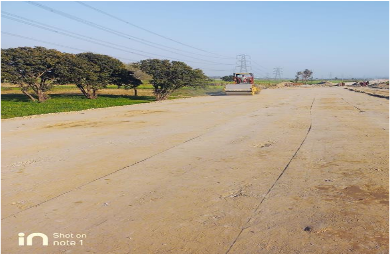
Sub Grade Top Rolling Work in Progress at Ch.22+860
