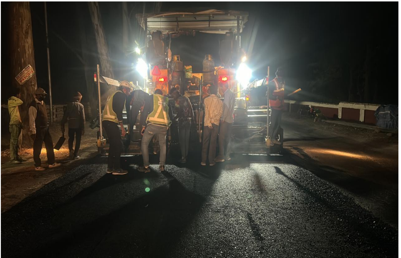
DBM Laying Work in Progress at Ch. 43+600
