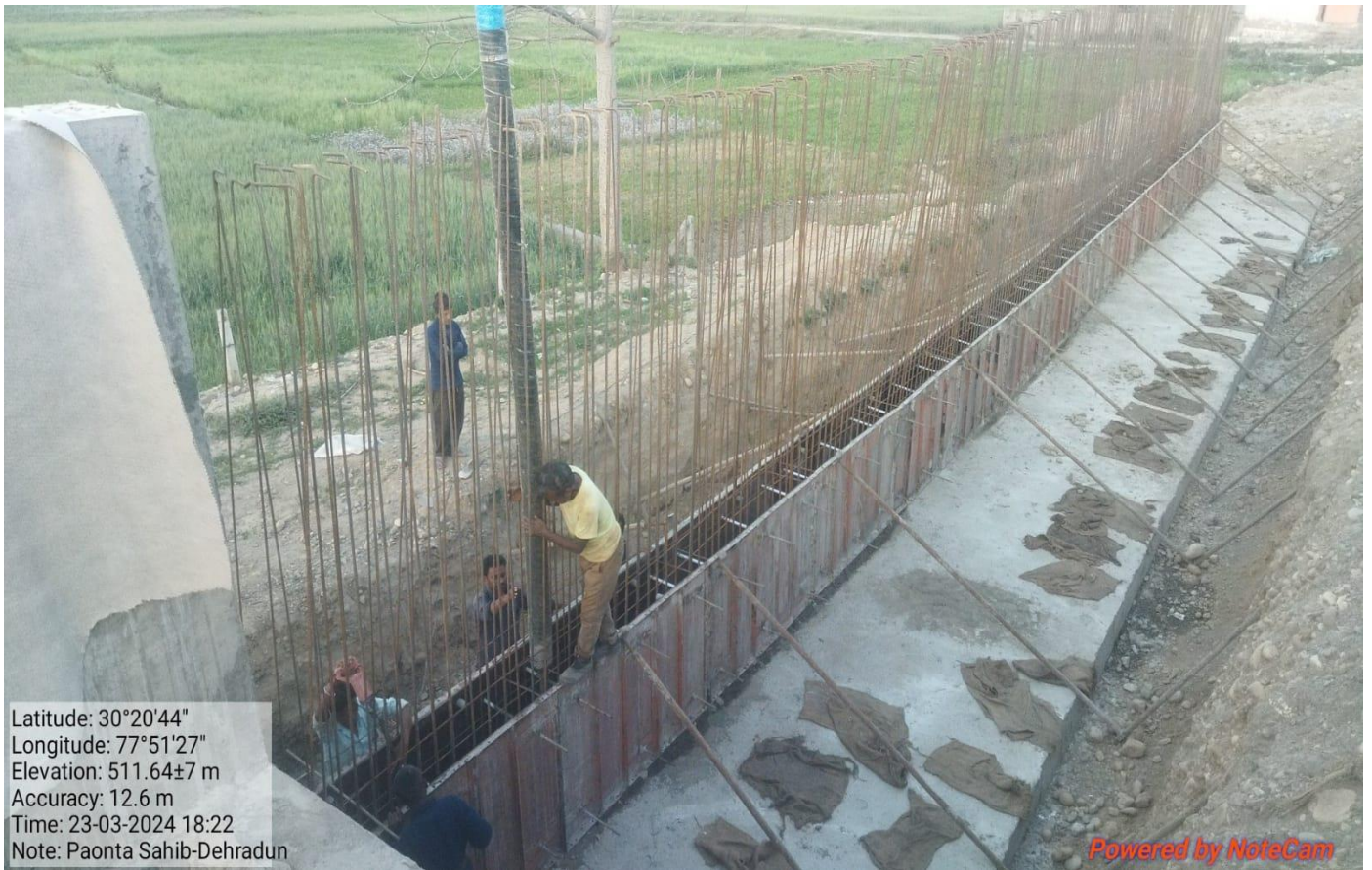
Retaining Wall Concrete Pouring Work in Progress at Ch. 29+360
