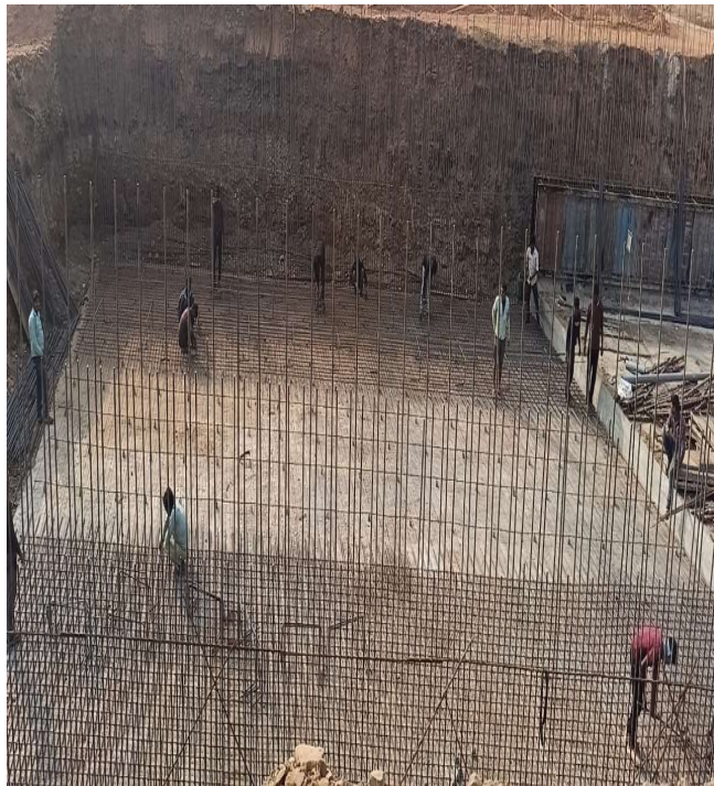
CH. 109+670 LVUP RAFT REINFORCEMENT WORK IN PROGRESS
