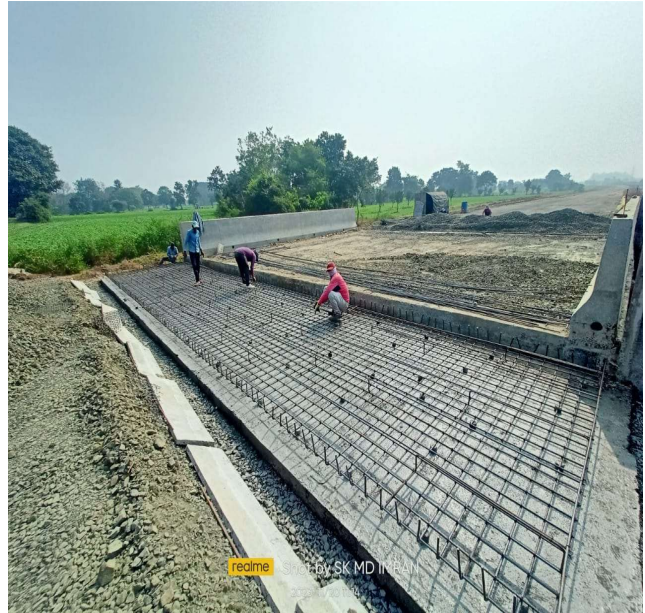
CH. 99+345 APPROACH SLAB WORK IN PROGRESS
