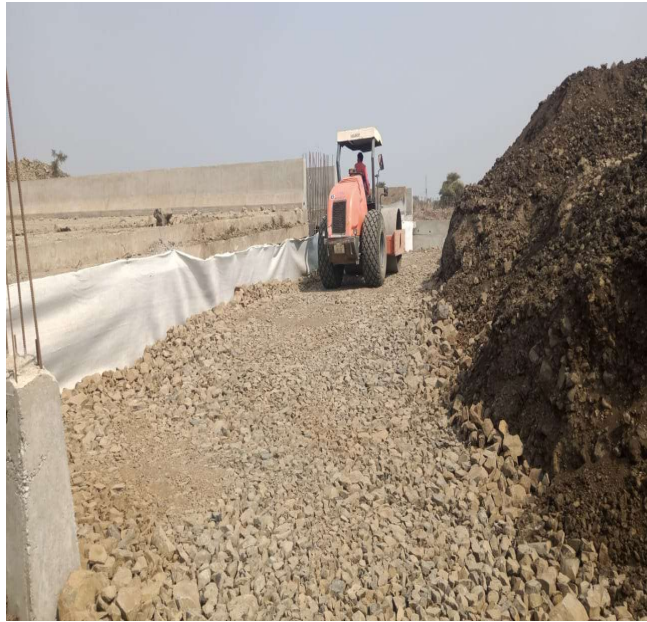
MNB BACKFILLING WORK IN PROGRESS
