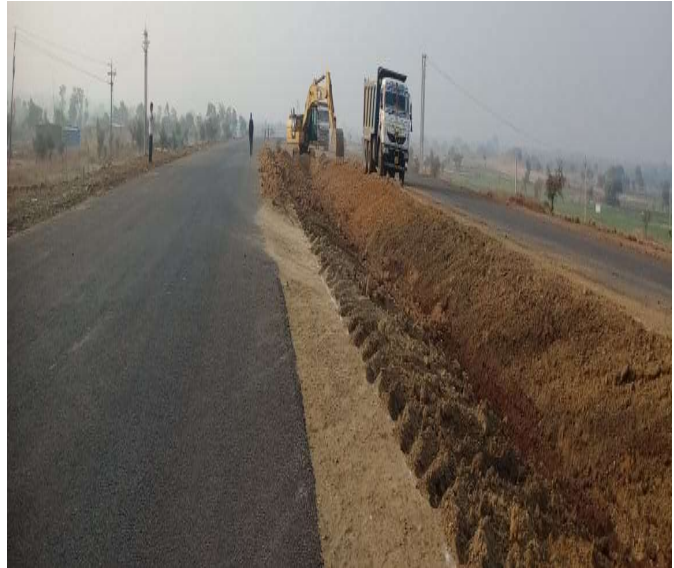
CH.97+700 to CH.98+200 MEDIAN SLOPE CUTTING WORK IN PROGRESS
