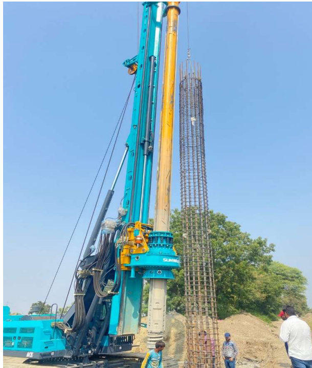
ROB PILE CAGING WORK IN PROGRESS
