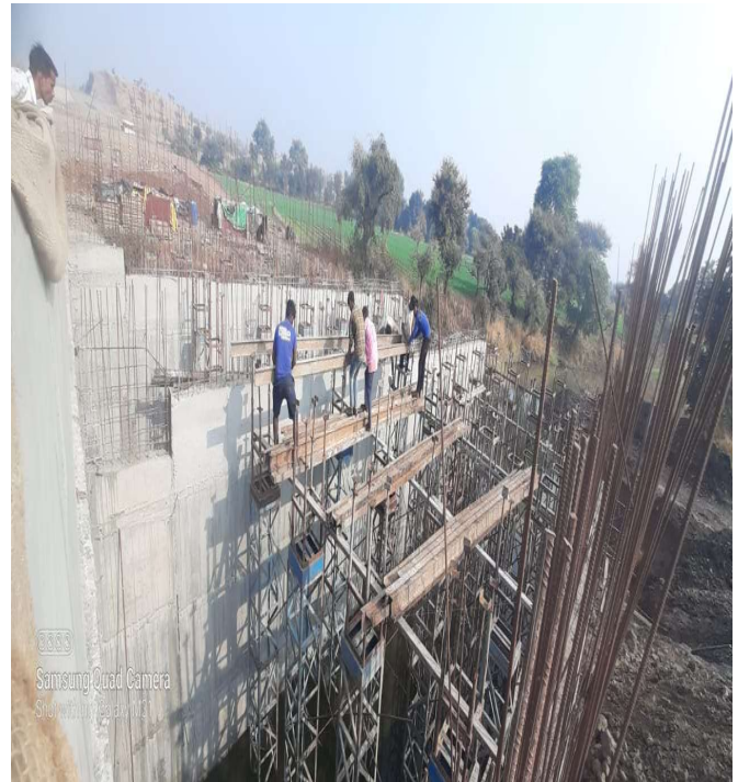
CH.116+595 SLAB STAGING WORK IN PROGRESS
