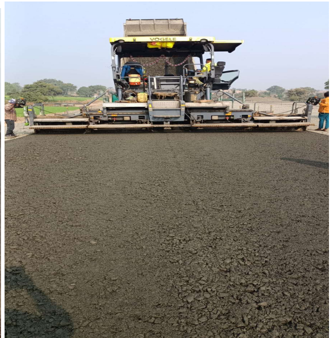
CH. 116+220 WMM TOP LAYING (LHS)
