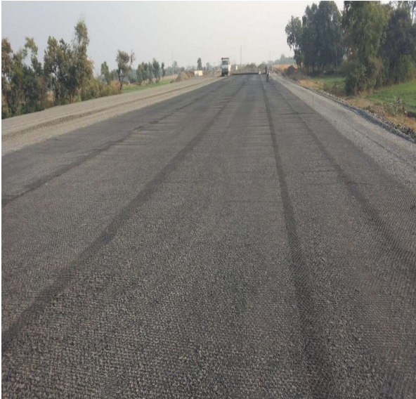
CH.119+380 to CH.119+550 GEOGRID LAYING WORK IN PROGRESS
