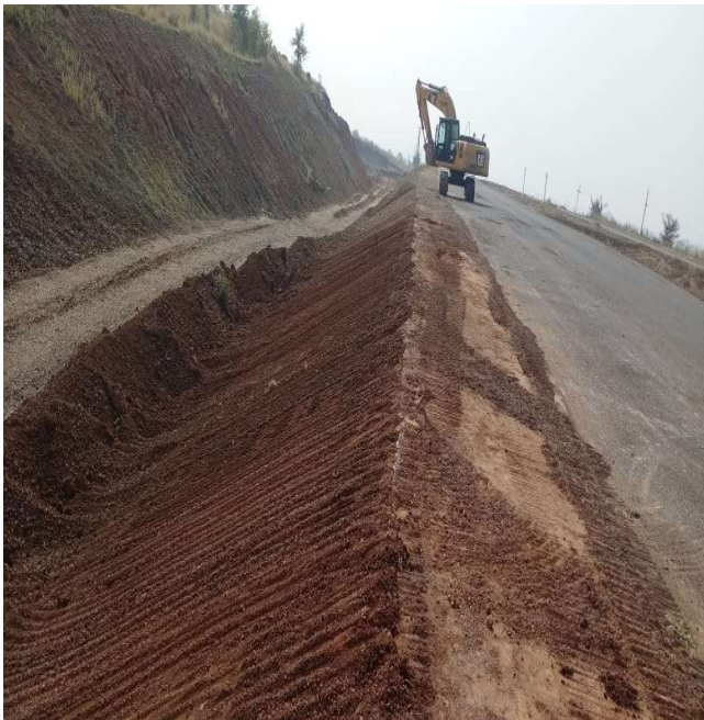
CH. 107+370 SLOPE CUTTING WORK IN PROGRESS
