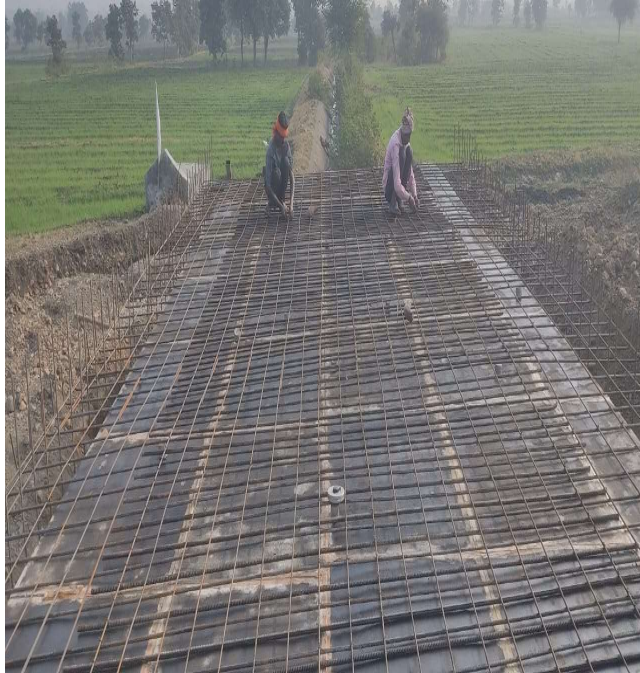
CH.120+150 SLAB REINFORCEMENT WORK IN PROGRESS
