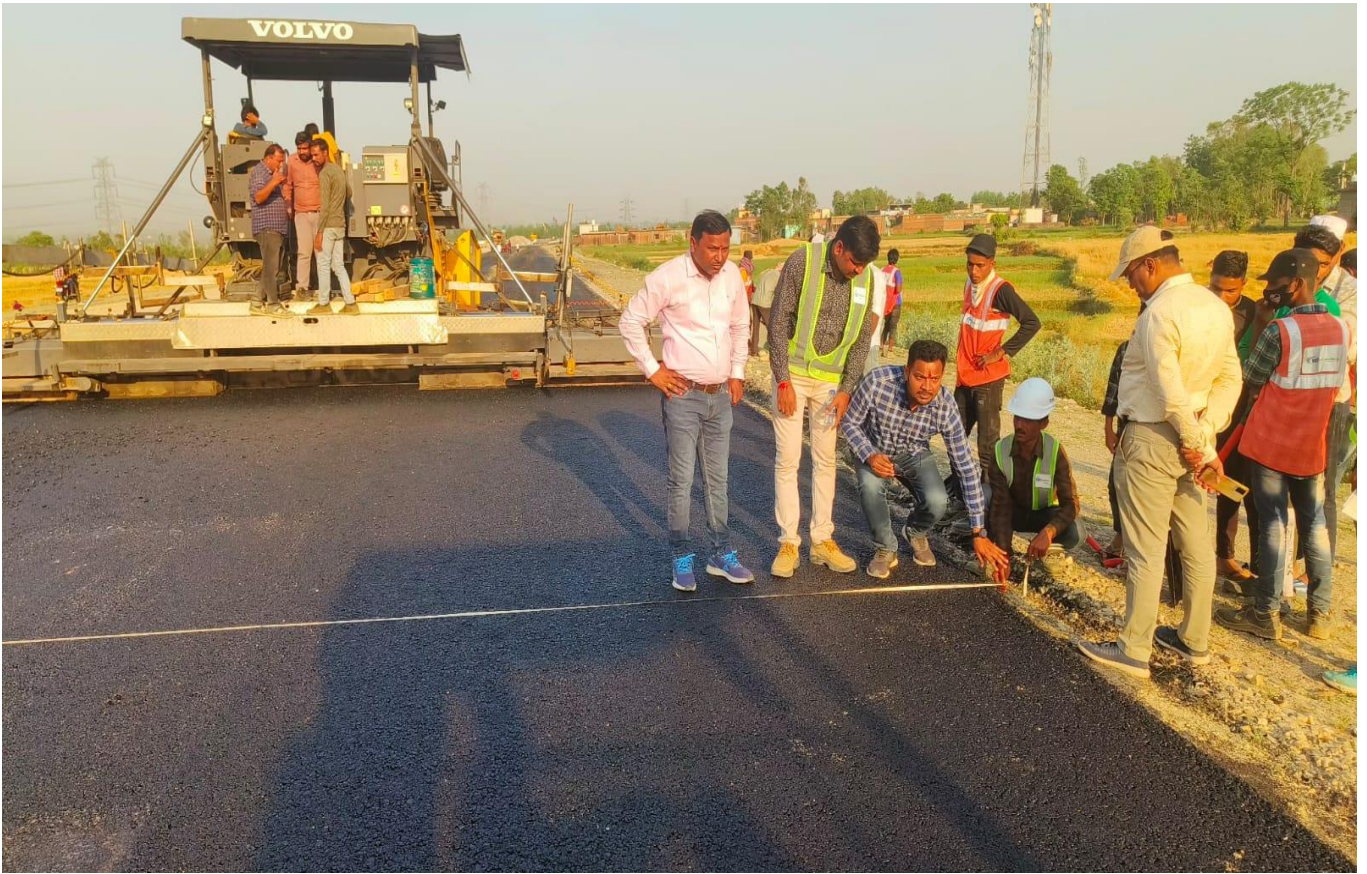
DBM Width & Thickness Checking with IE Team at Ch. 19+350
