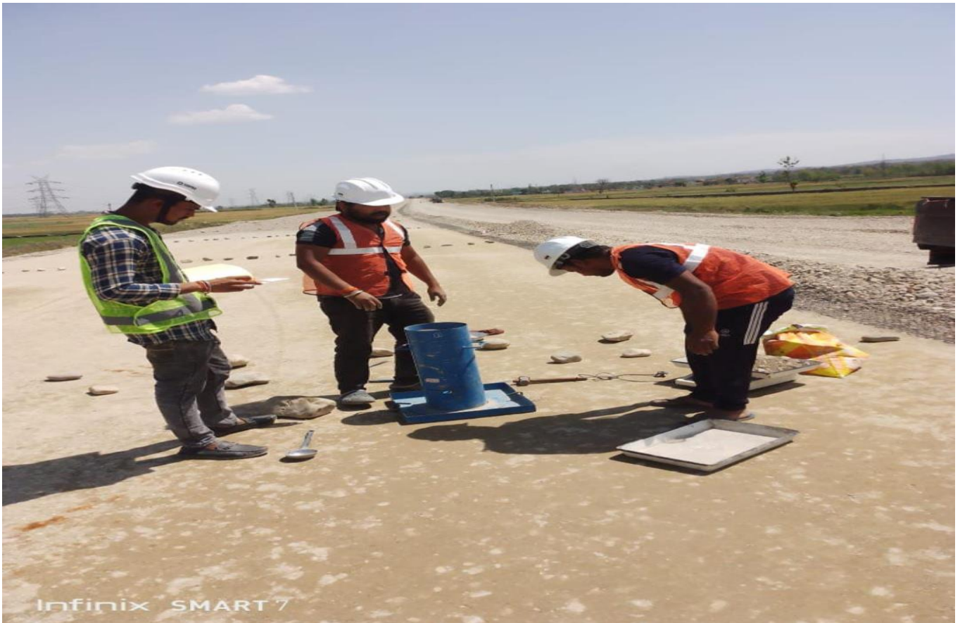
FDD Checking of WMM Top at Ch. 23+000
