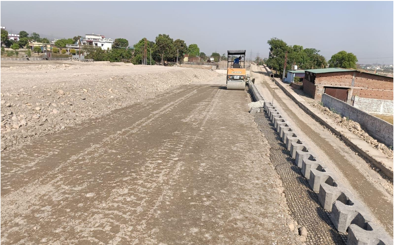
RE Wall Backfill Rolling Work in Progress at Ch -31+400 to 31+500 LHS
