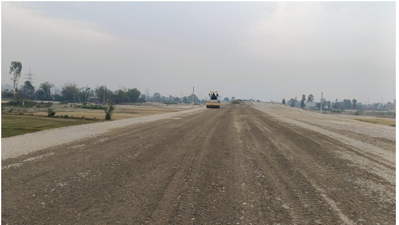
GSB Top Rolling Work in Progress at Ch. 28+100
