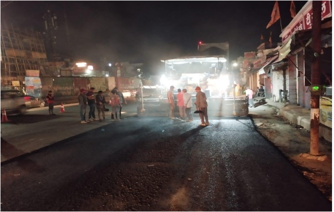
DBM Laying Work in Progress at Ch. 40+500
