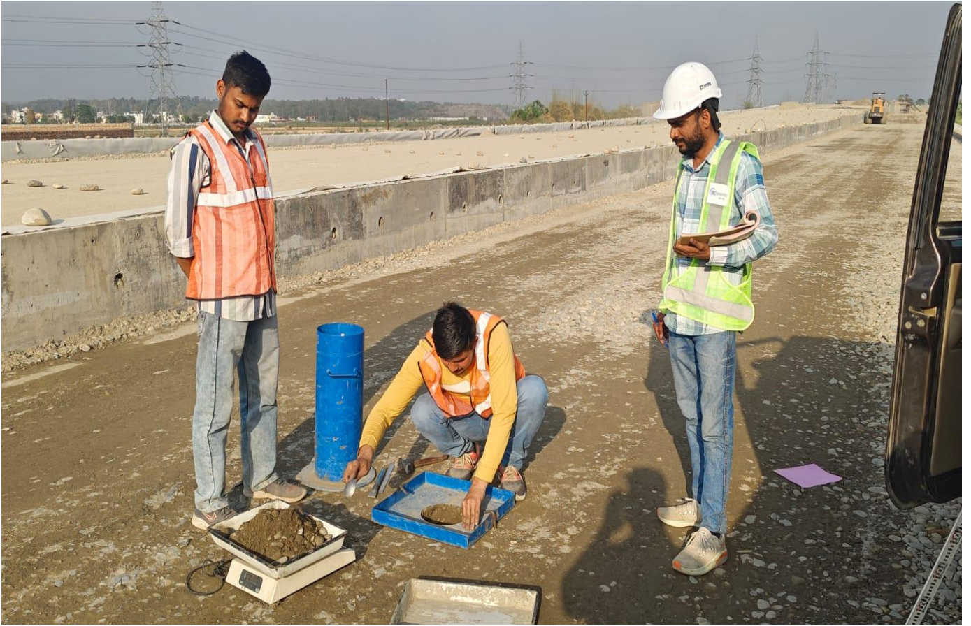
FDD Checking of Service Road GSB Top at Ch 29+820 to 30+000
