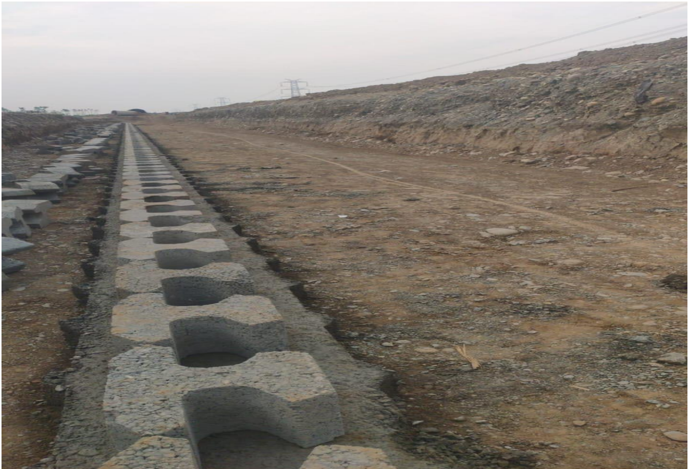
RE Wall Erection Work in Progress at Ch. 22+200
