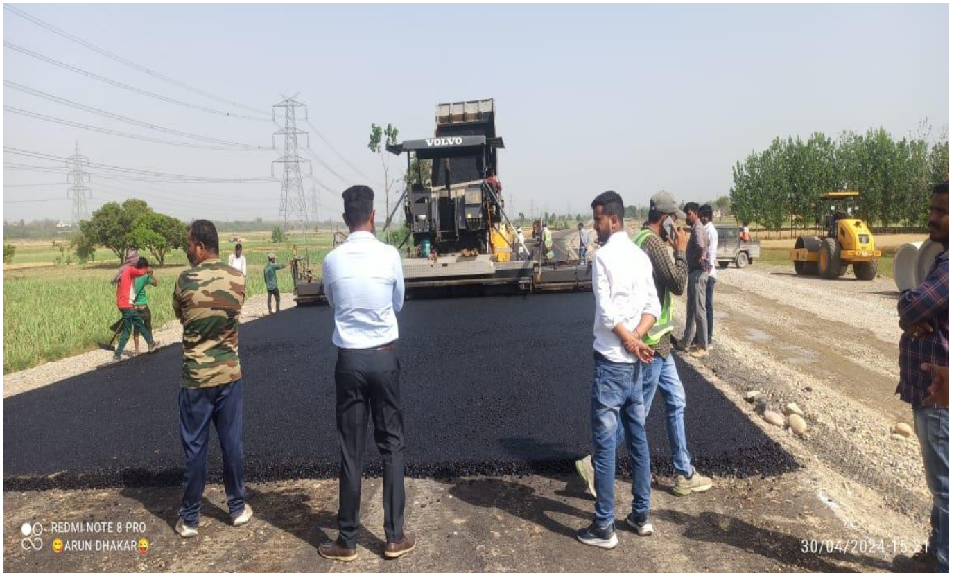
DBM Laying Work in Progress at Ch. 23+000
