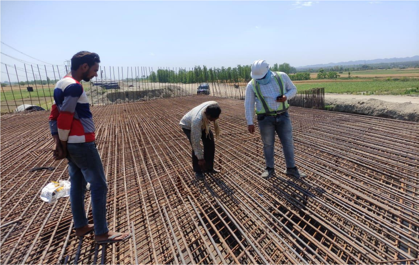
MNB Top Slab Reinforcement Binding Work in Progress at Ch. 20+820
