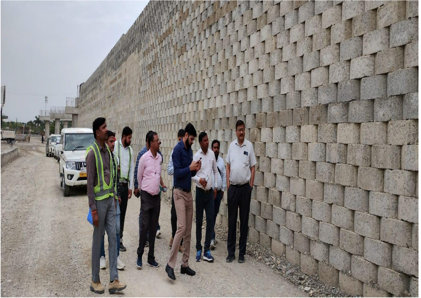
NHAI and IE Team Site Visit at Ch. 31+678
