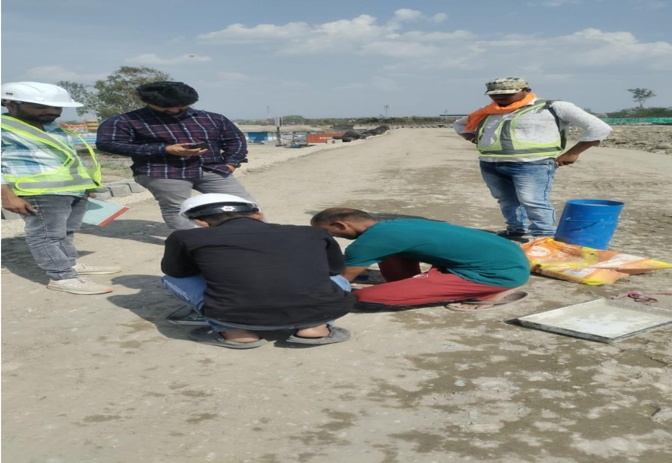
FDD Checking on RE Wall Back Fill Bed at Ch. 31+550
