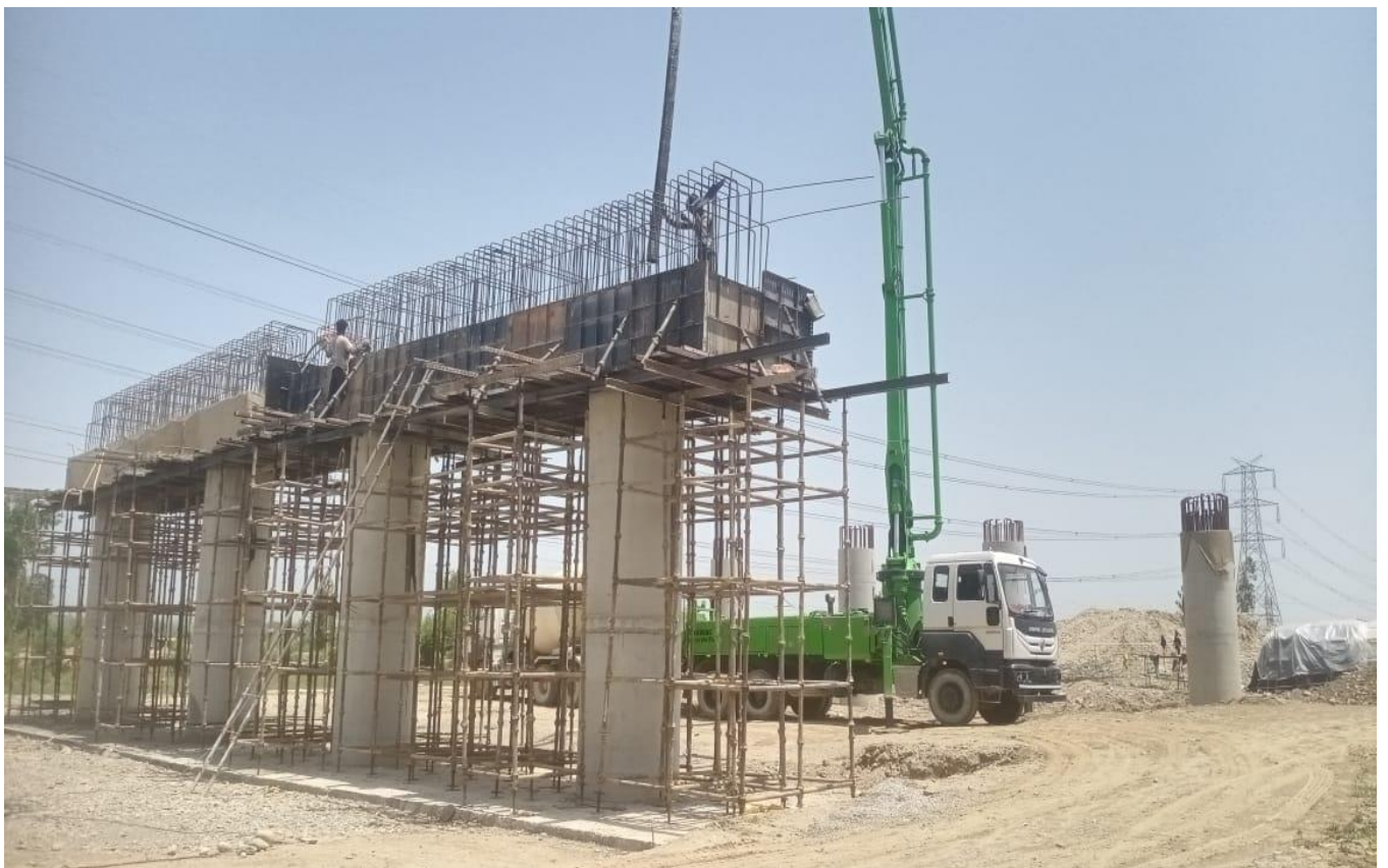
VUP Pier Cap Concrete Pouring Work in Progress at Ch. 22+598
