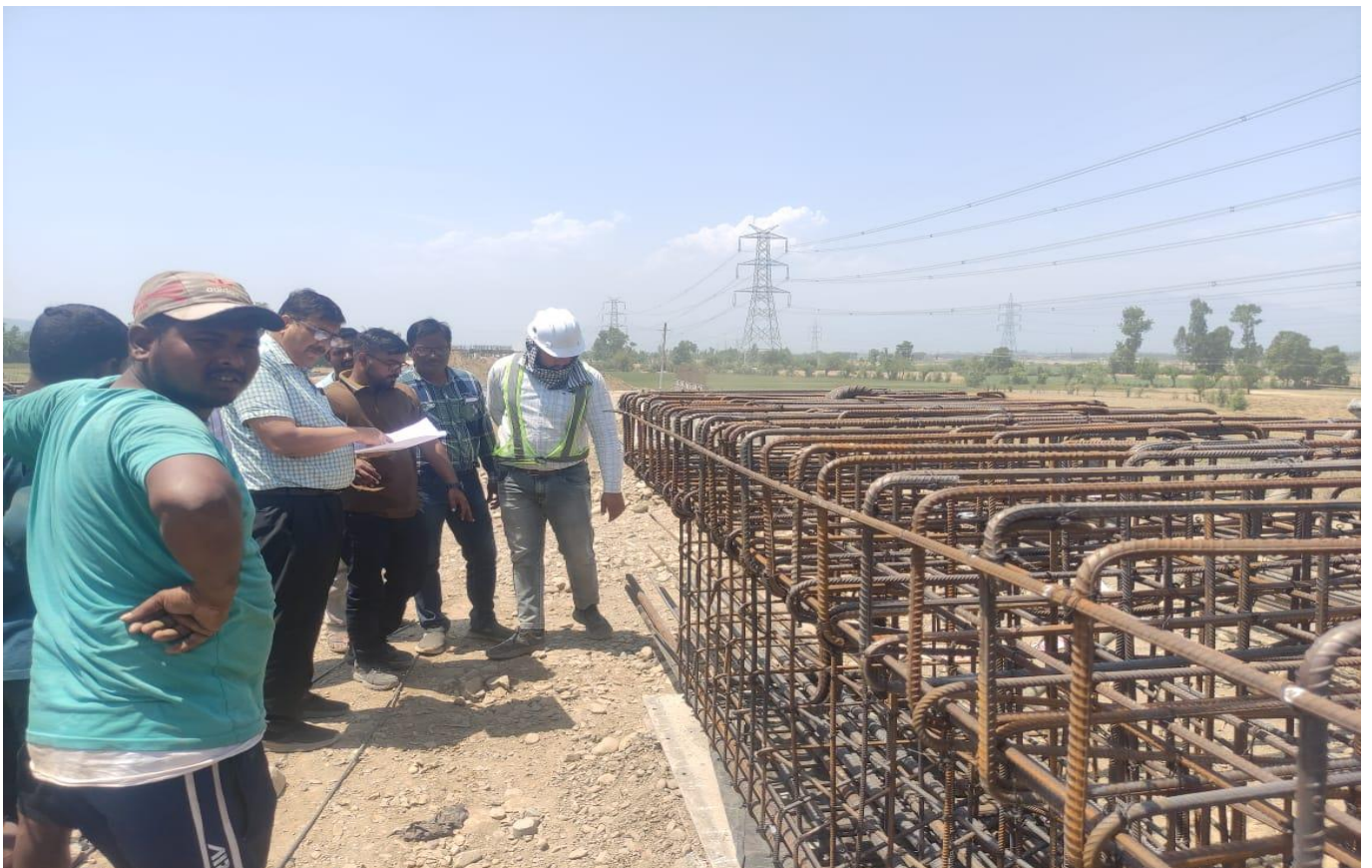
VUP Girder Reinforcement Checking by TL Sir & ABE Sir
