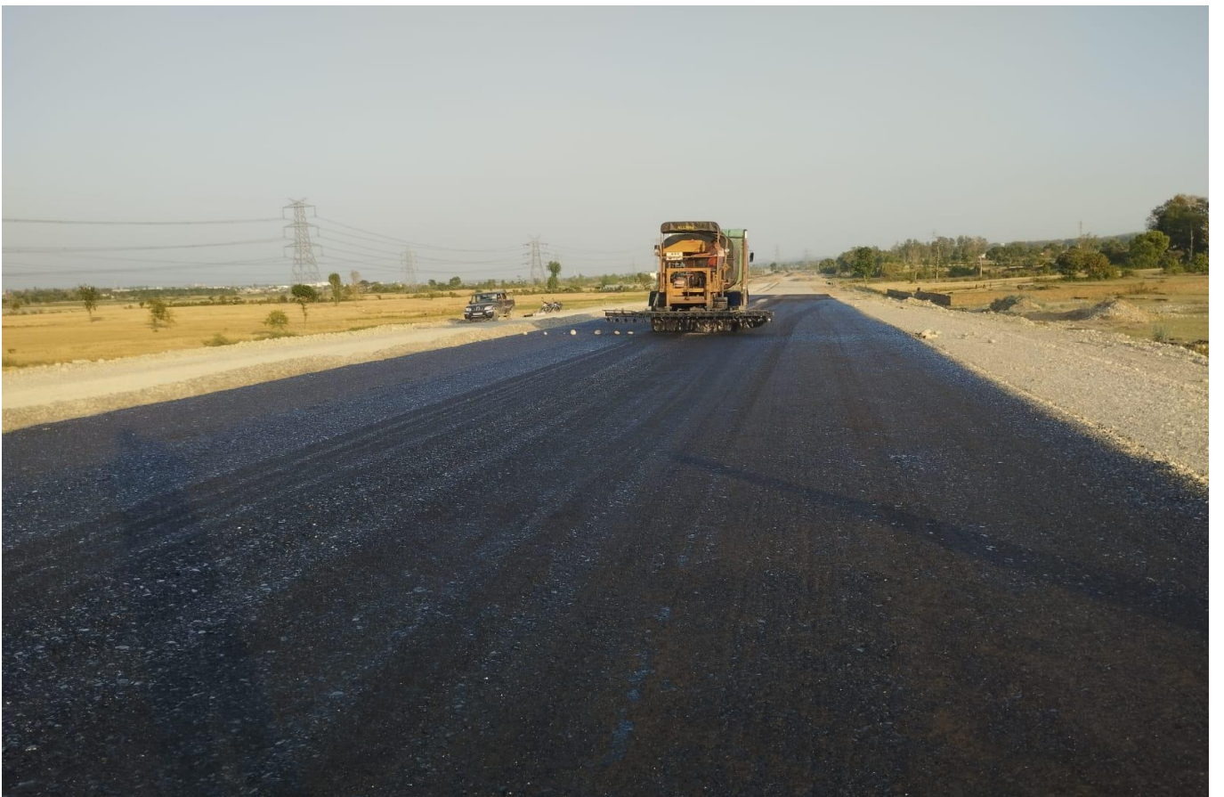
Prime Coat Spraying Work in Progress at Ch 24+200
