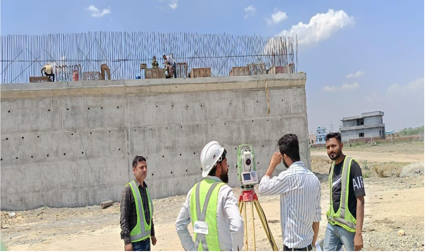
MJB Abutment Pedestal Layout & Level Checking by SE sir
