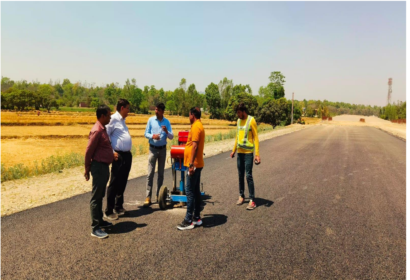
DBM Core Cutting Going on at Ch. 19+400
