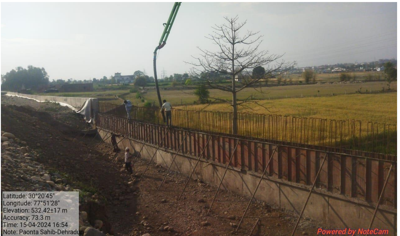
Retaining Wall Concrete Pouring Work in Progress from Ch-29+360 to 29+390
