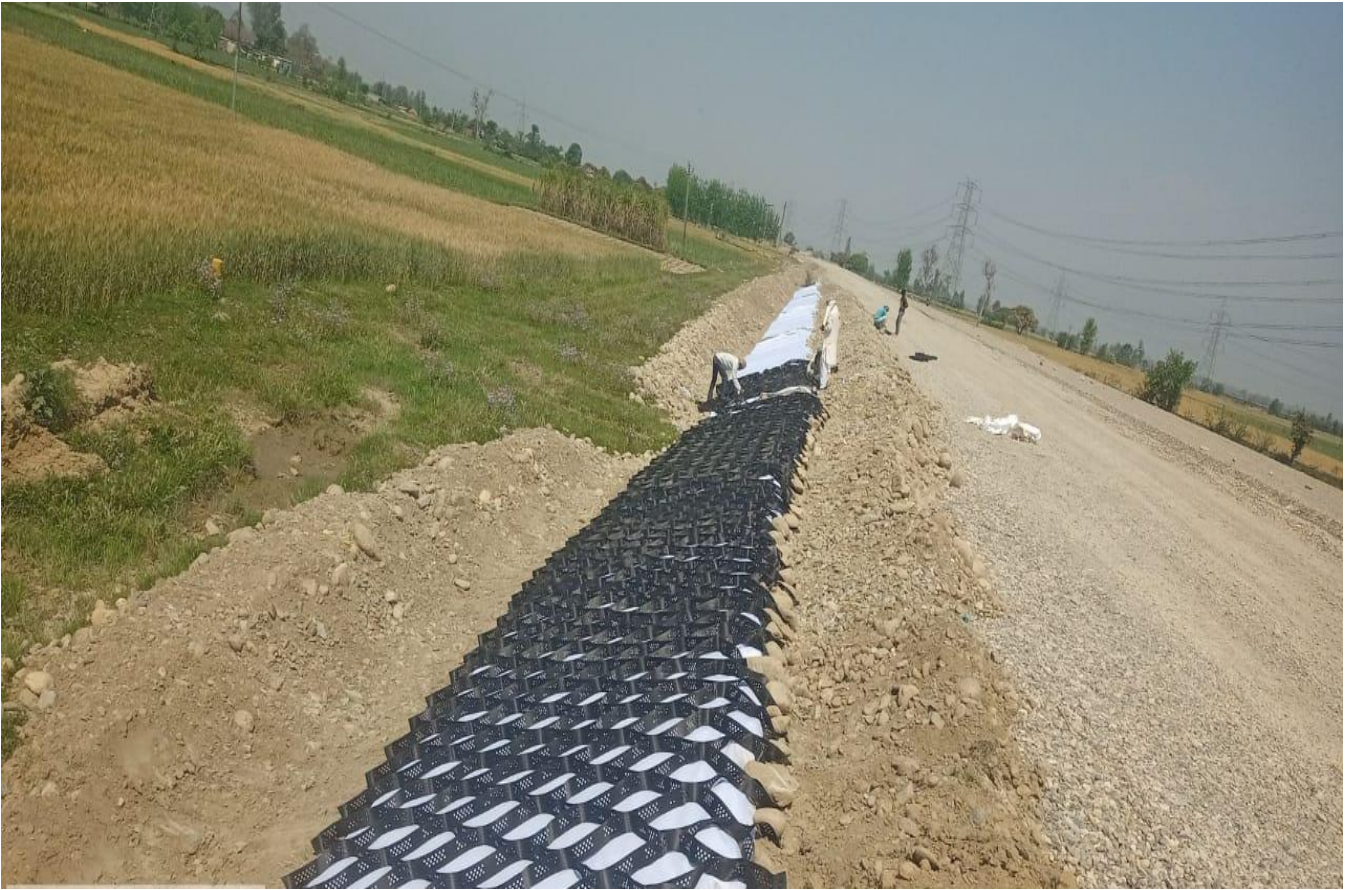
Geo Cell Laying Work in Progress for Slope Protection at Ch-23+650
