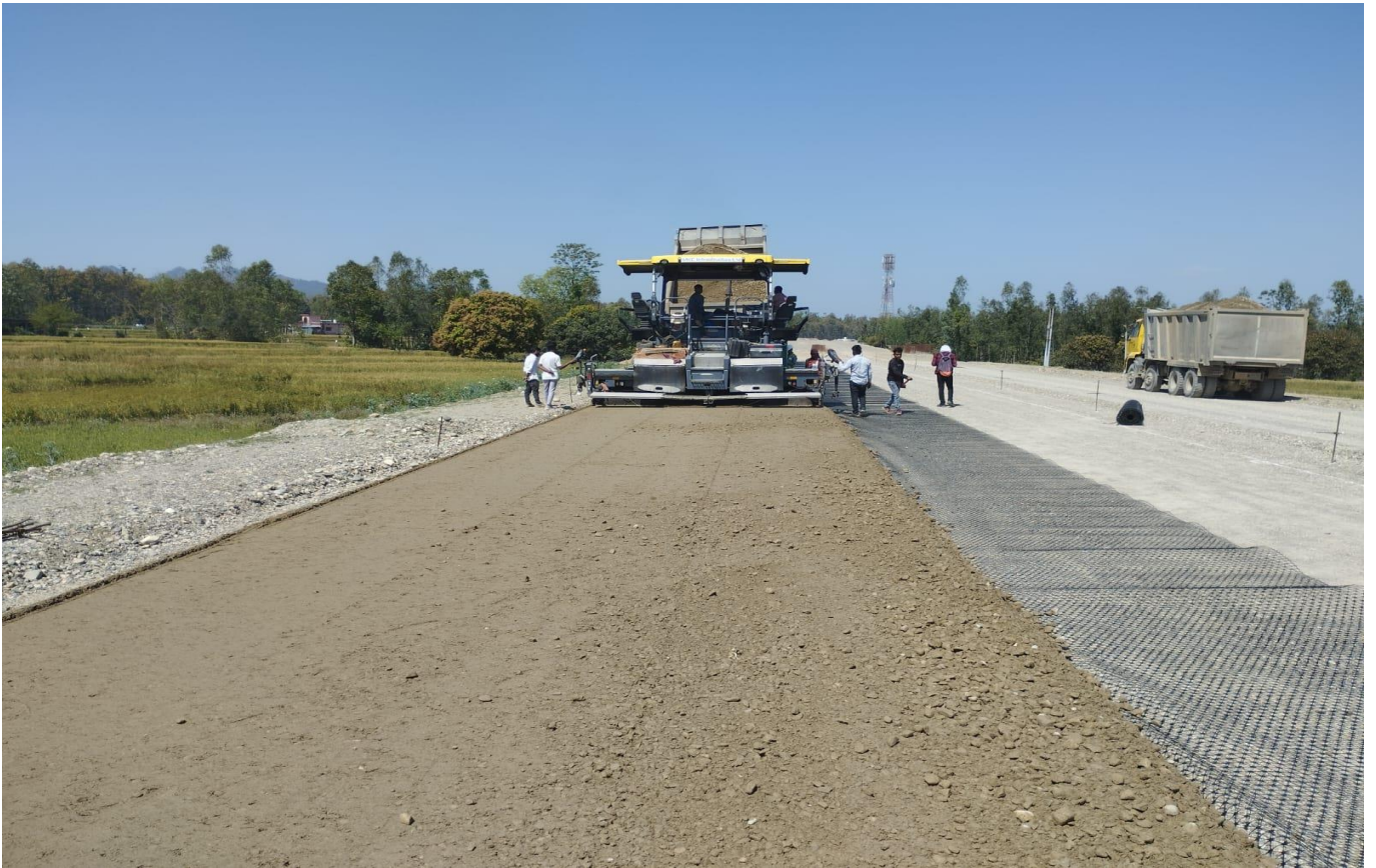
WMM Laying Work in Progress at Ch. 19+400
