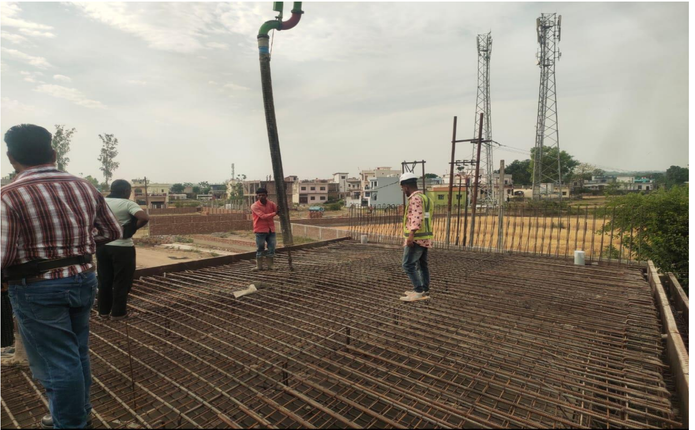
Box Culvert Slab Pouring Work in Progress at Ch. 31+370
