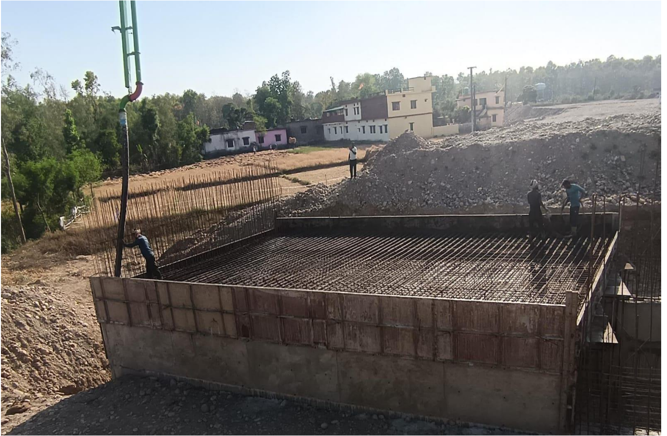
Box Culvert Top Slab Concrete Pouring Work in Progress at Ch. 19+080
