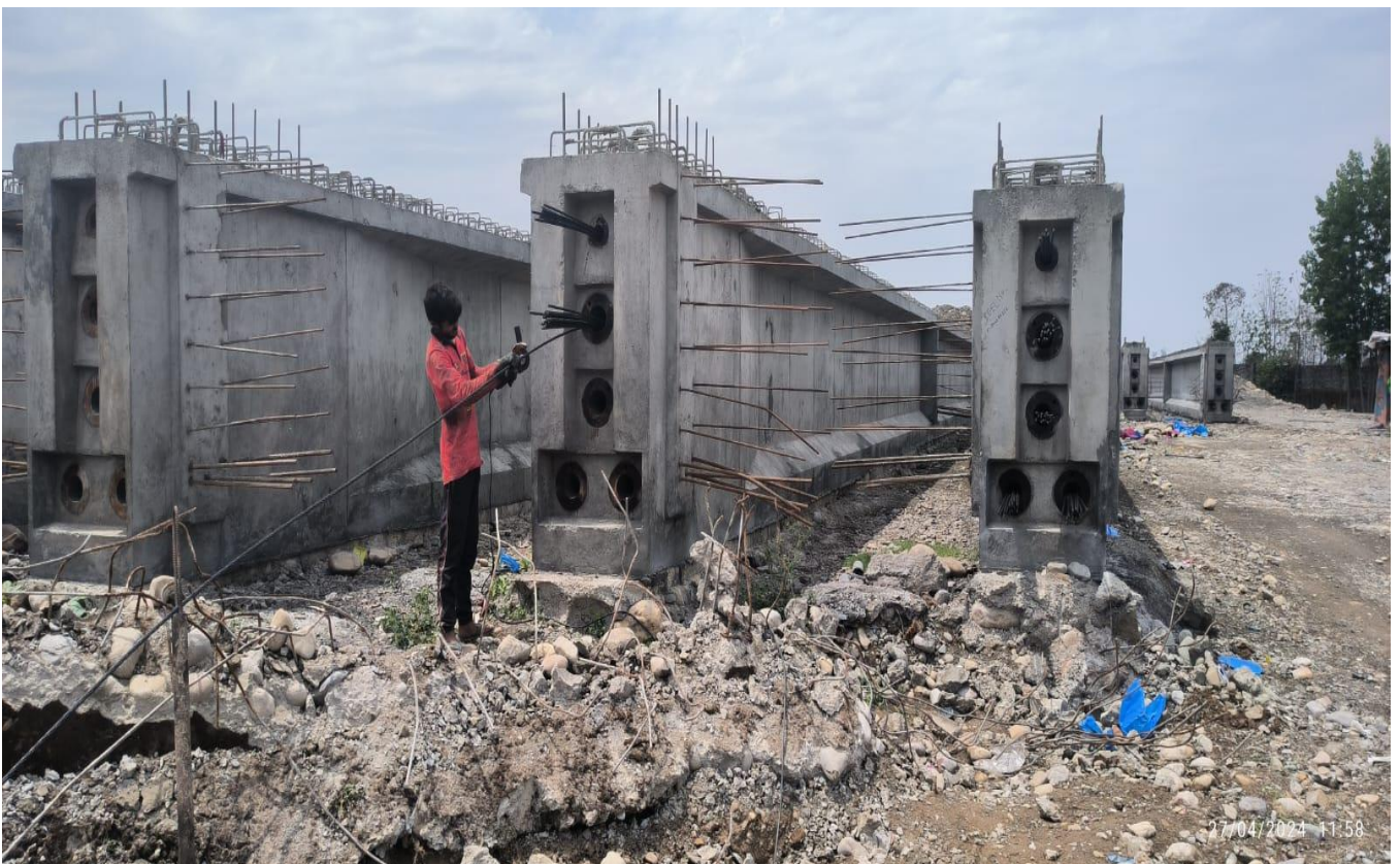
MJB LRPC Threading Work in Progress at Ch. 33+033
