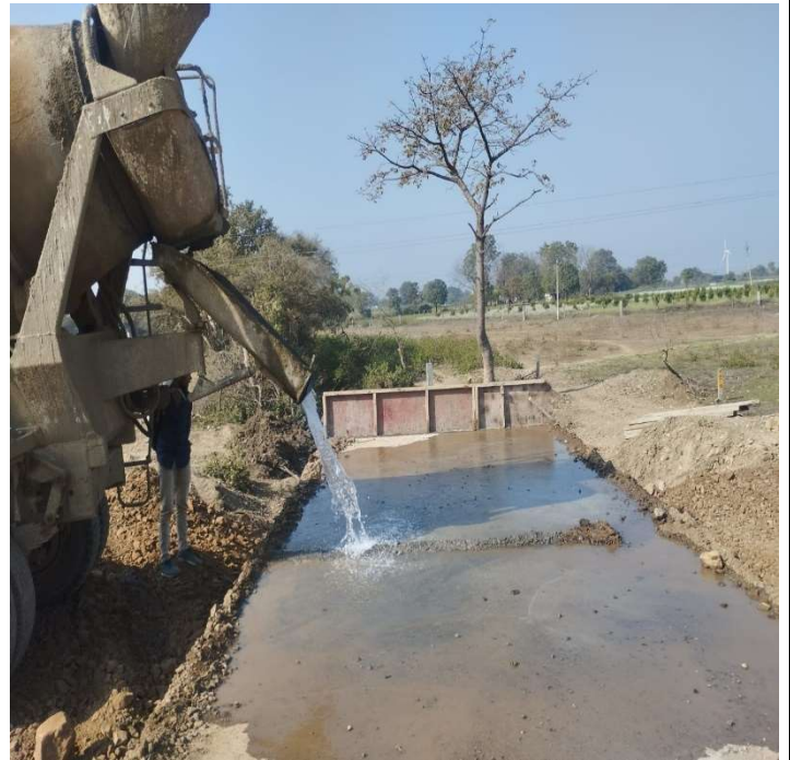
Curing work is in progress @Ch 126+388 BC
