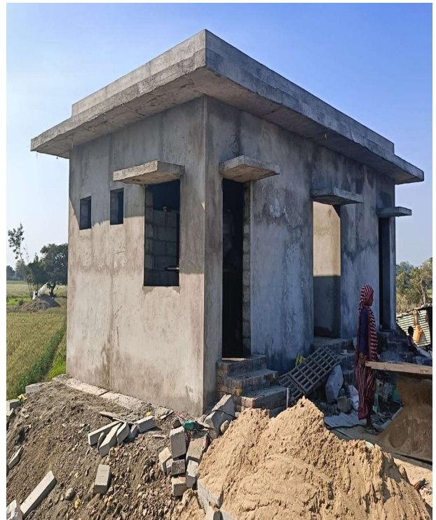
TOILET BLOCK WORK IN PROGRESS
