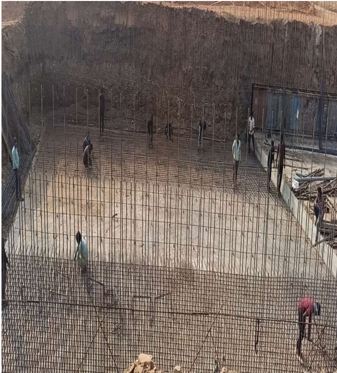
CH. 109+670 LVUP RAFT RENINFORCEMENT WORK IN PROGRESS
