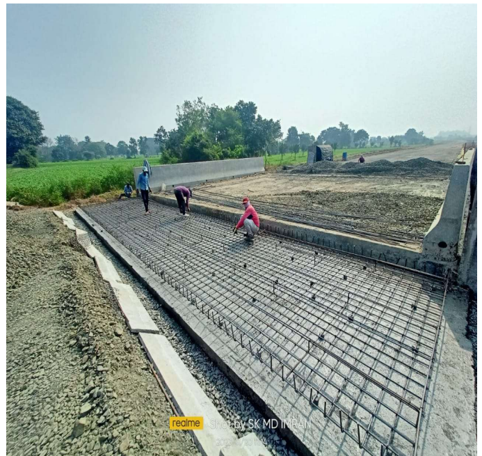
CH. 99+345 APPROACH SLAB WORK IN PROGRESS
