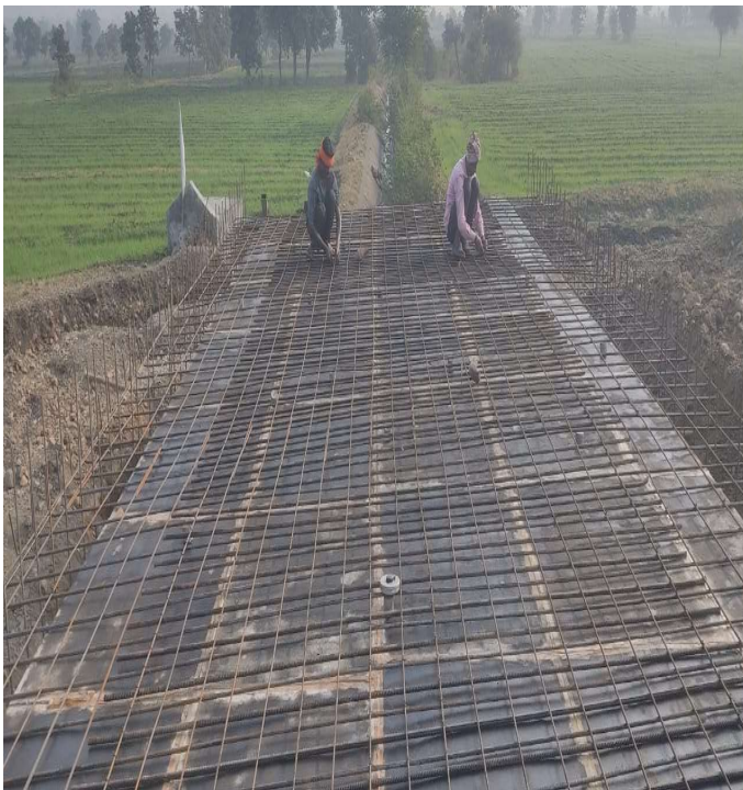
CH. 109+670 LVUP RAFT RENINFORCEMENT WORK IN PROGRESS
