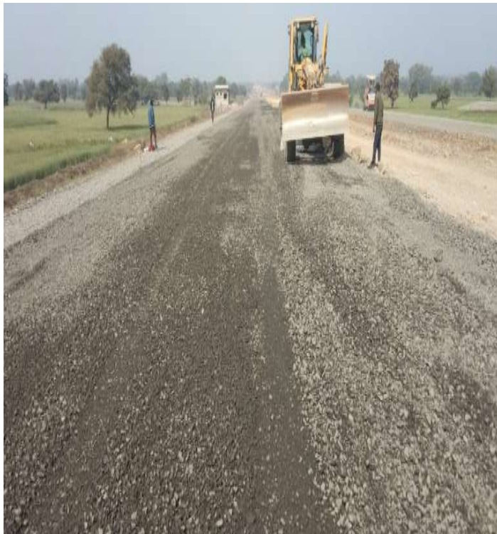
WMM 1ST LAYER WORK IN PROGRESS @ Ch.93+040
