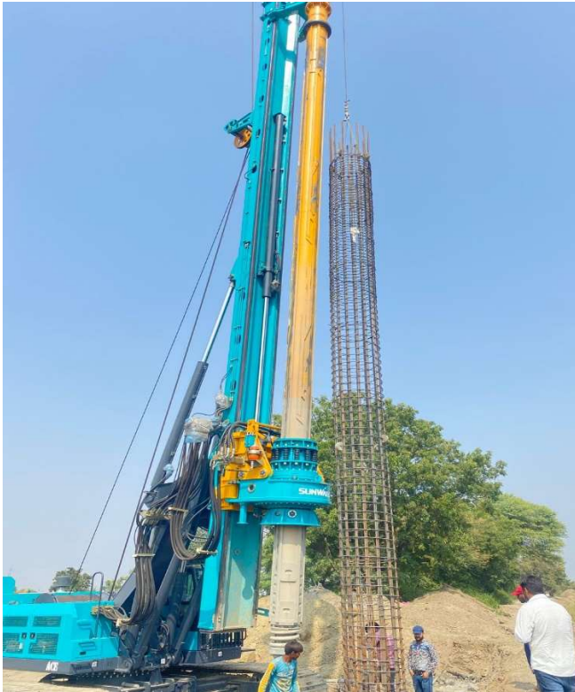
ROB PILE CAGING WORK IN PROGRESS
