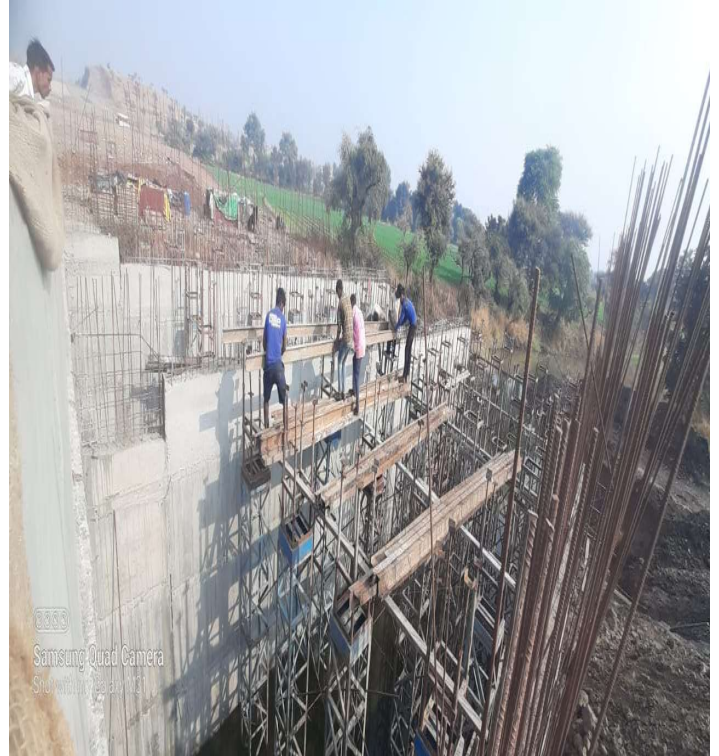
CH.116+595 SLAB STAGGING WORK IN PROGRESS
