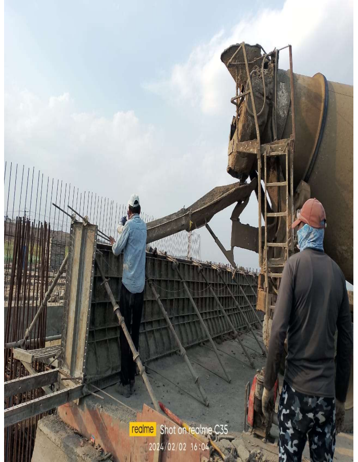
Ch 114+901 lvup RHS median side crash barrier
