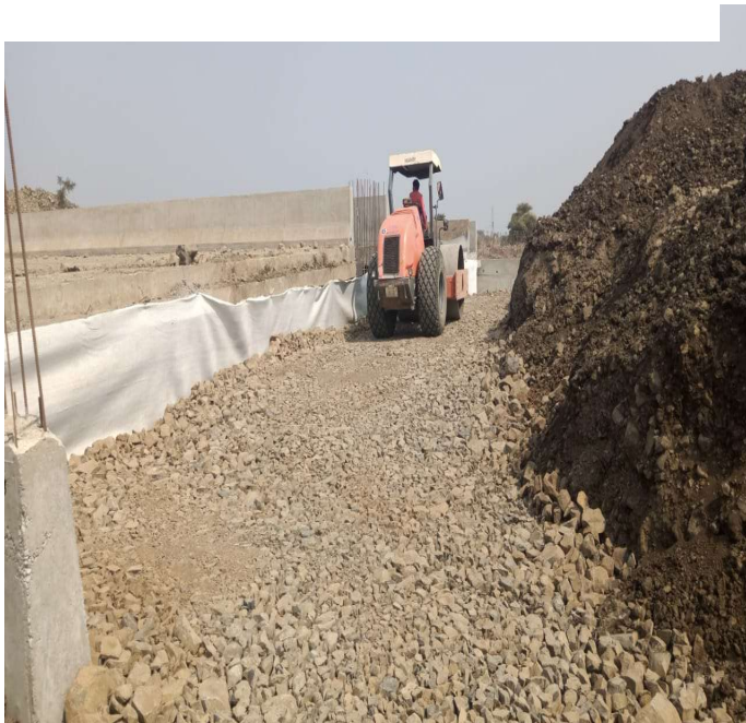
MNB BACKFILLING WORK IN PROGRESS
