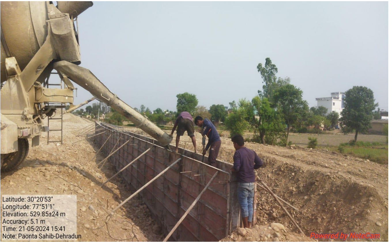
Retaining Wall Concrete Pouring Work in Progress at Ch. 28+600
