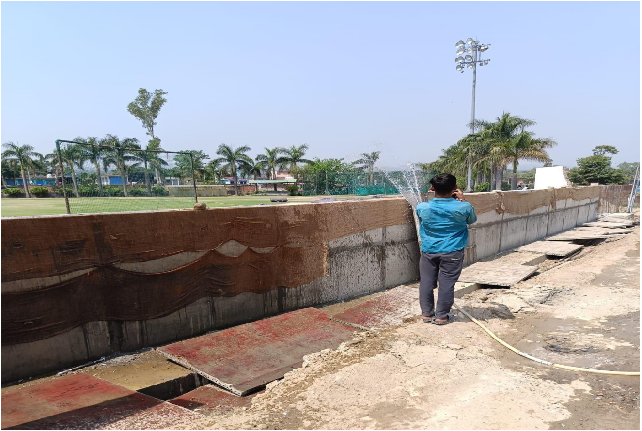
Toe Wall Curing Work in Progress at Ch. 31+960
