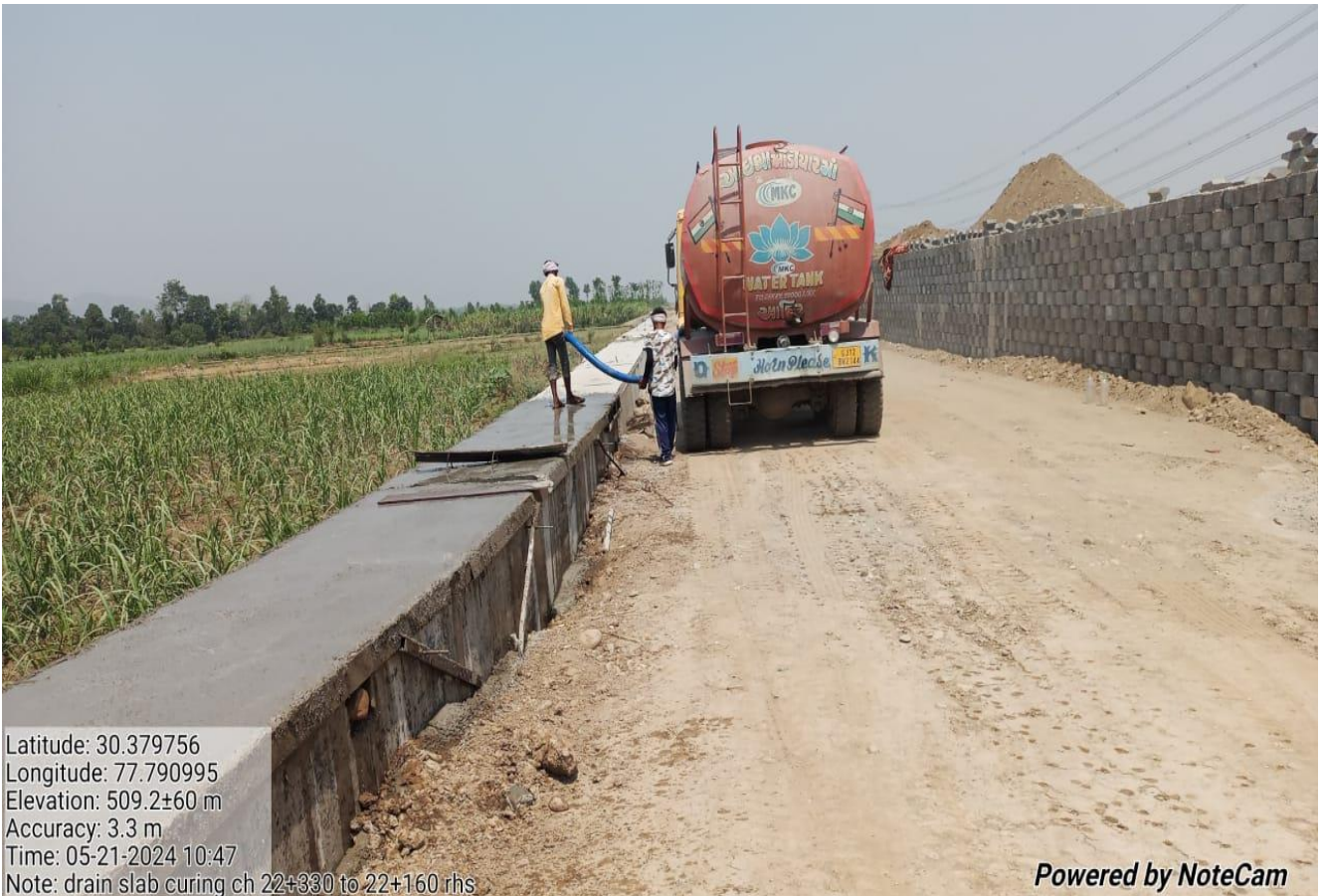
Drain Slab Curing Work in Progress at Ch 22+160 to 22+330
