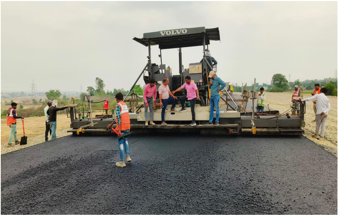
DBM Laying Continue Checked by IE Team at Ch 26+580
