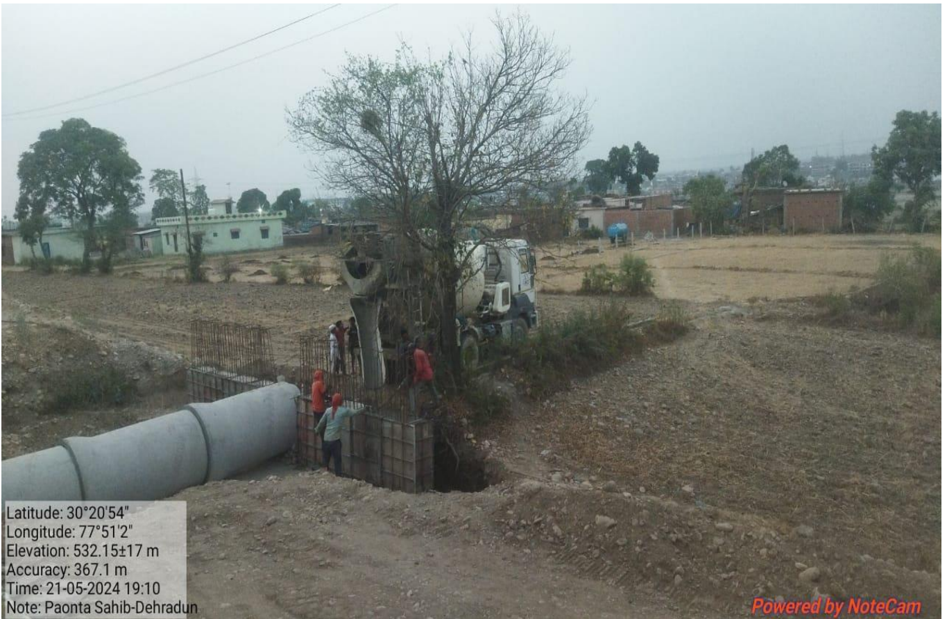
HPC Retaining Wall Pouring Work in Progress at Ch. 28+581
