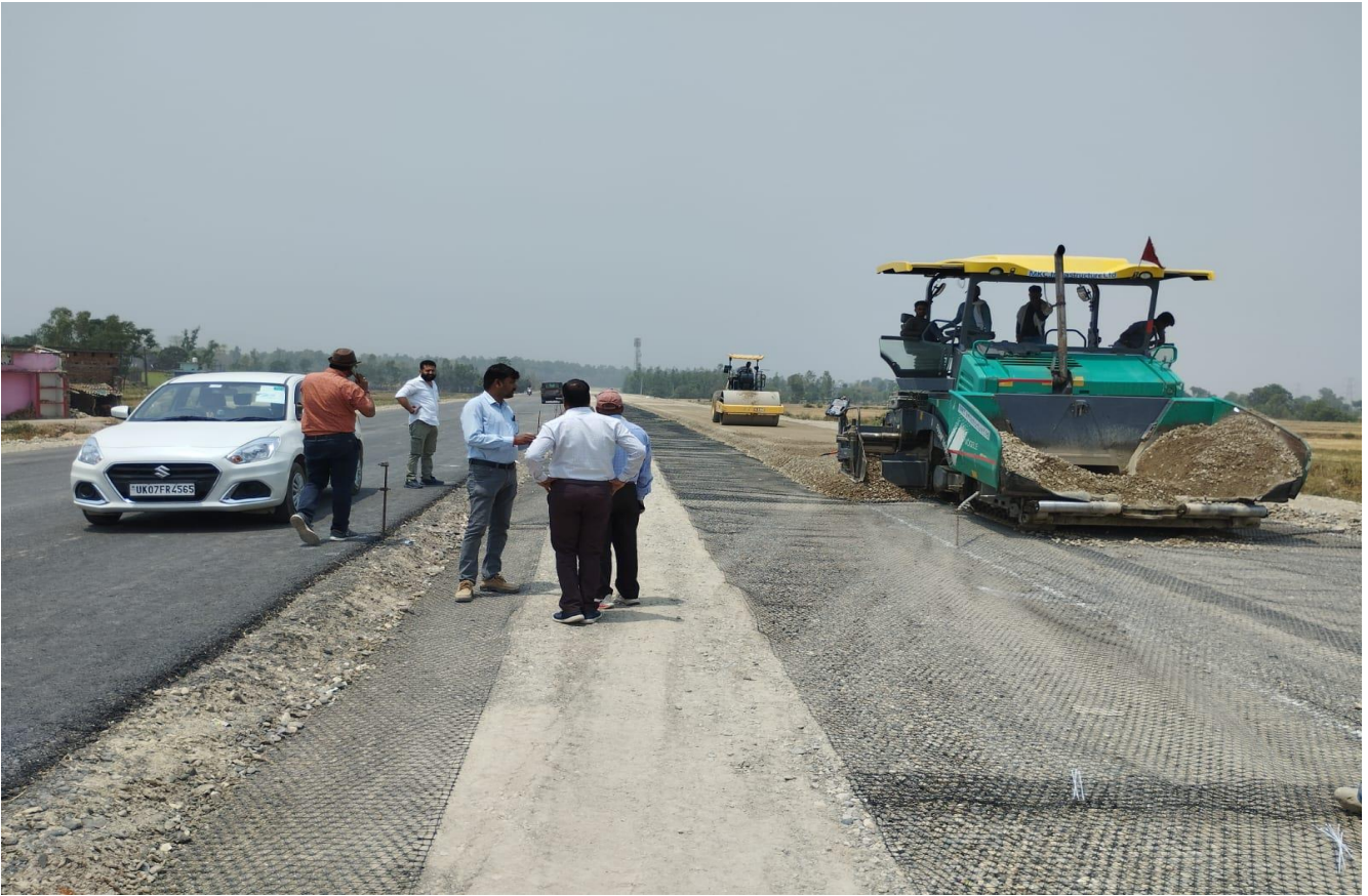
Site Inspection by RE Sir and IE Team
