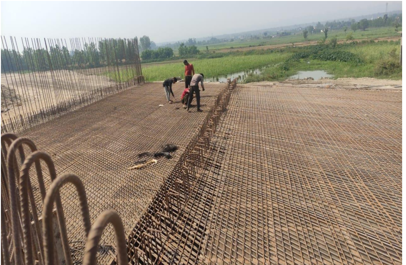
MNB Slab Reinforcement Binding Work in Progress at Ch. 20+820
