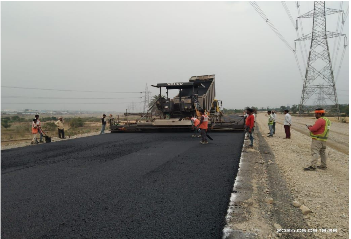
DBM Laying Work in Progress at Ch. 26+400
