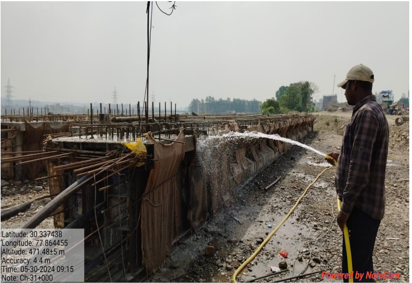
PSC Girder Curing Work in Progress at Ch. 31+000
