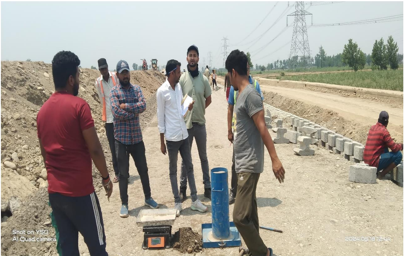
FDD Checking of Backfilling of RE Wall at Ch. 22+300
