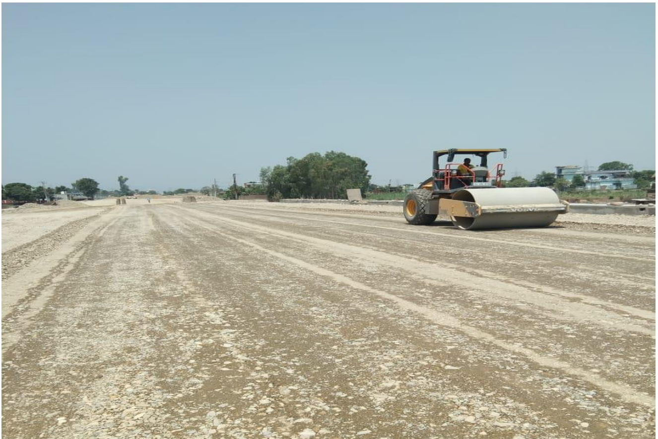
GSB Top Rolling Work in Progress at Ch. 29+250
