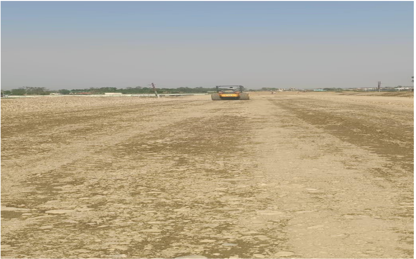
Sub Grade Top Rolling Work in Progress at Ch. 33+320 to 33520 (LHS)
