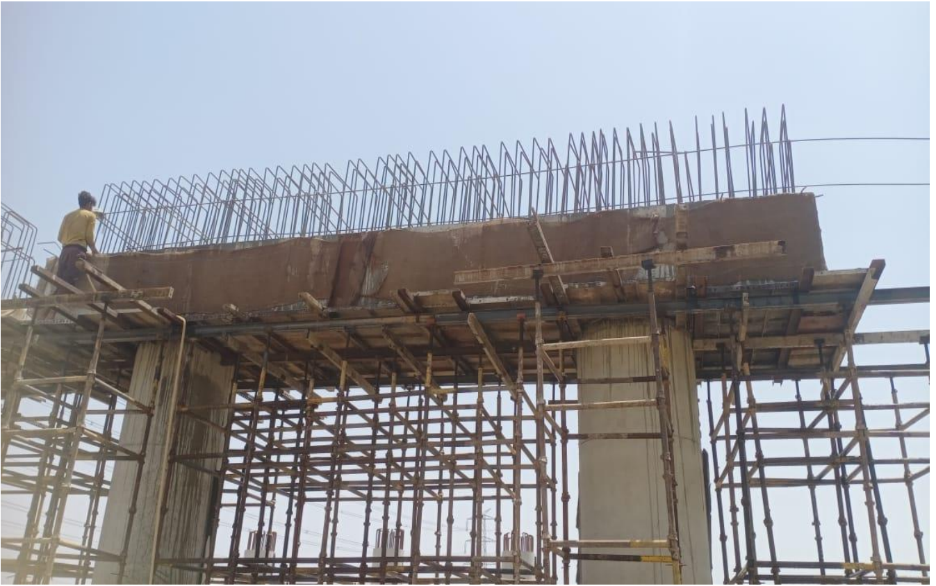
VUP Pier Cap Curing Work in Progress at Ch. 22+598
