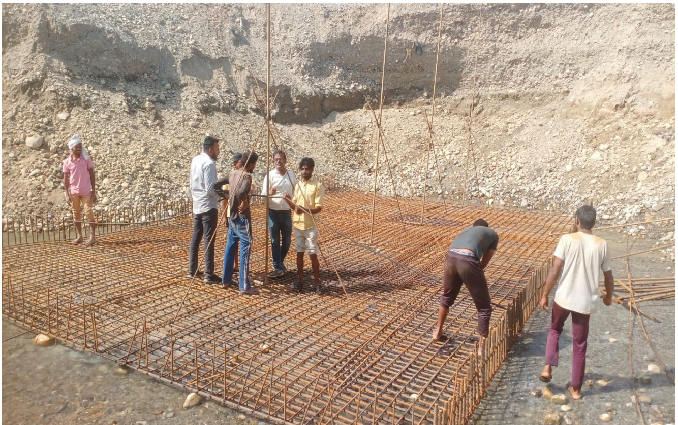
MNB Abutment Raft Reinforcement Binding Work in Progress at Ch. 21+610
