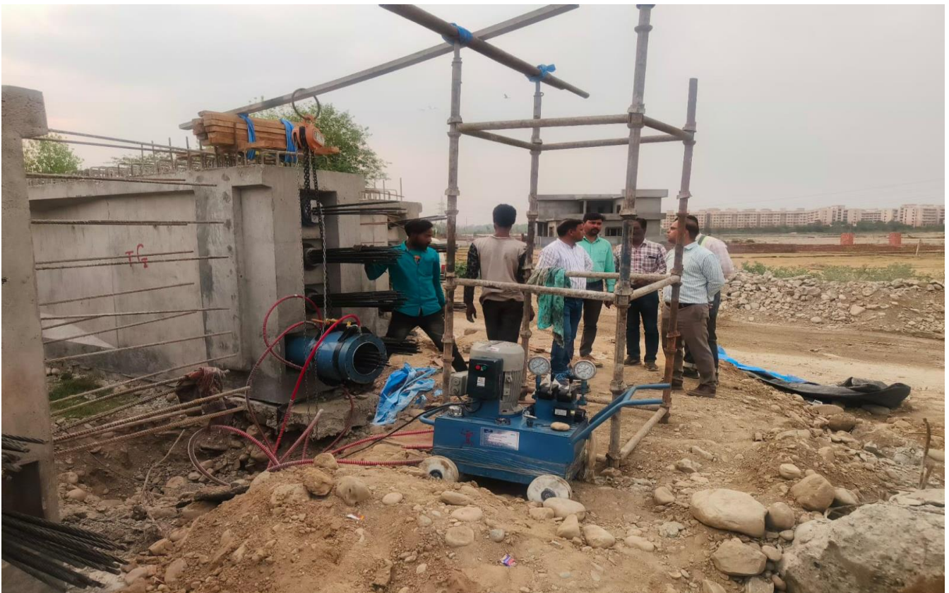
MJB PSC Girder Stressing Work in Progress at Ch. 33+033
