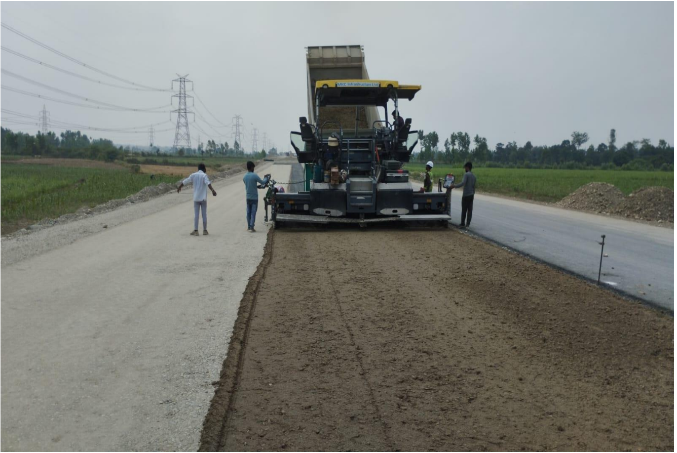
WMM Laying Work in Progress at Ch. 21+400
