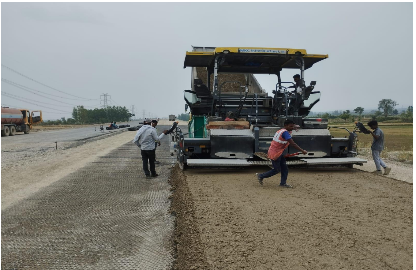
WMM Laying Work in Progress at Ch 20+500 to 20+720(RHS)
