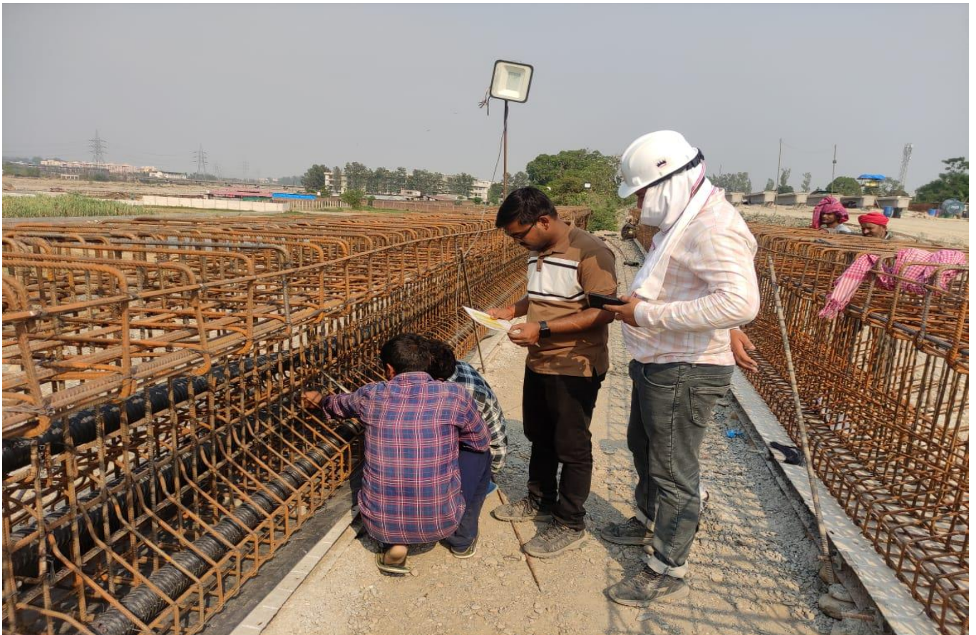
VUP PSC Girder Reinforcement & Profile Checking by ABE Sir at Ch. 31+691
