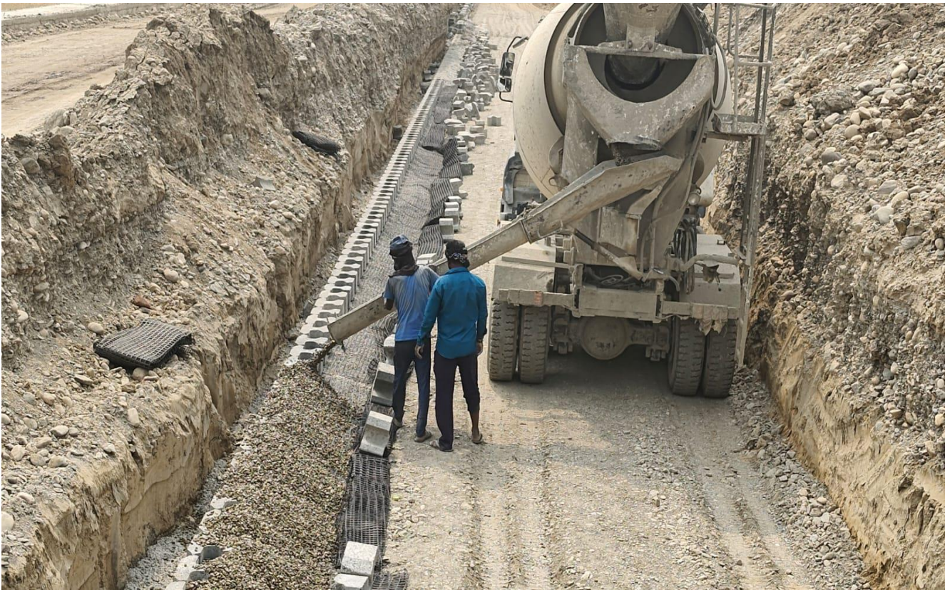
Filter media pouring work is in progress at ch 22+350 to 22+450 (LHS)
