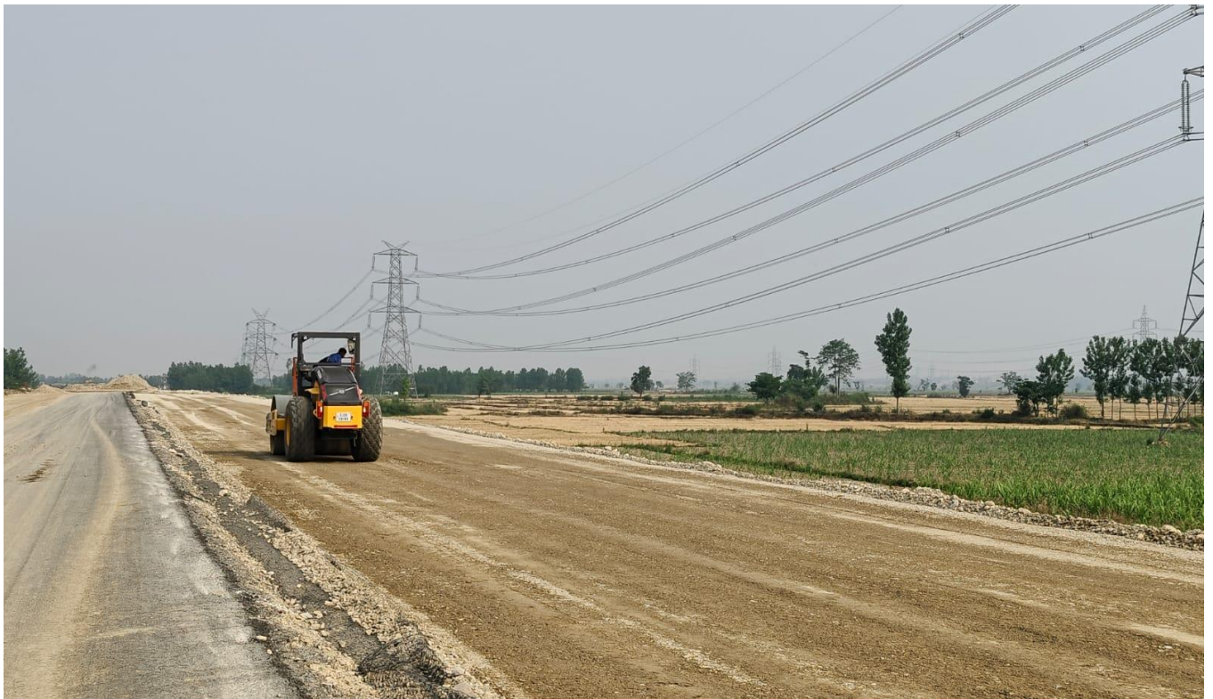
GSB Top Rolling Work in Progress at Ch. 21+300 to 21+500 (LHS)
