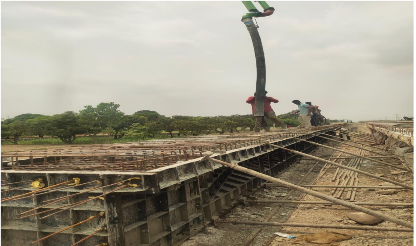
VUP RCC Girder Casting Work in Progress Ch. 22+598
