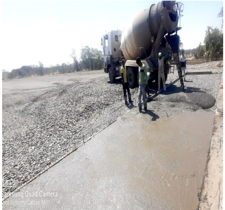
Ch.119+903 SVUP RHS Approach Slab Work in progress.
