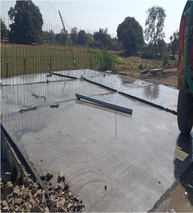
Top slab curing work is in progress @ Ch 125+281 MNB(RHS)
