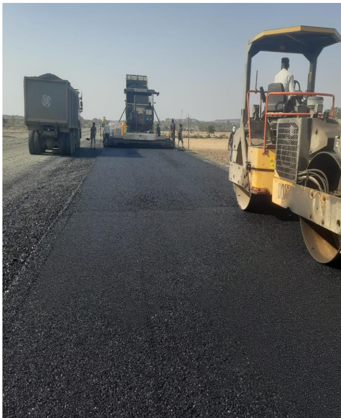
DBM laying work in progress at Ch 119+930 to 120+590
