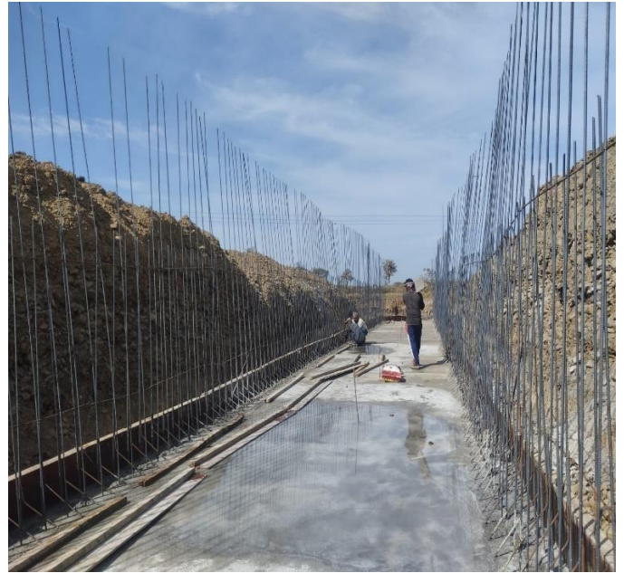
Bottom Haunch shuttering work is in progress
