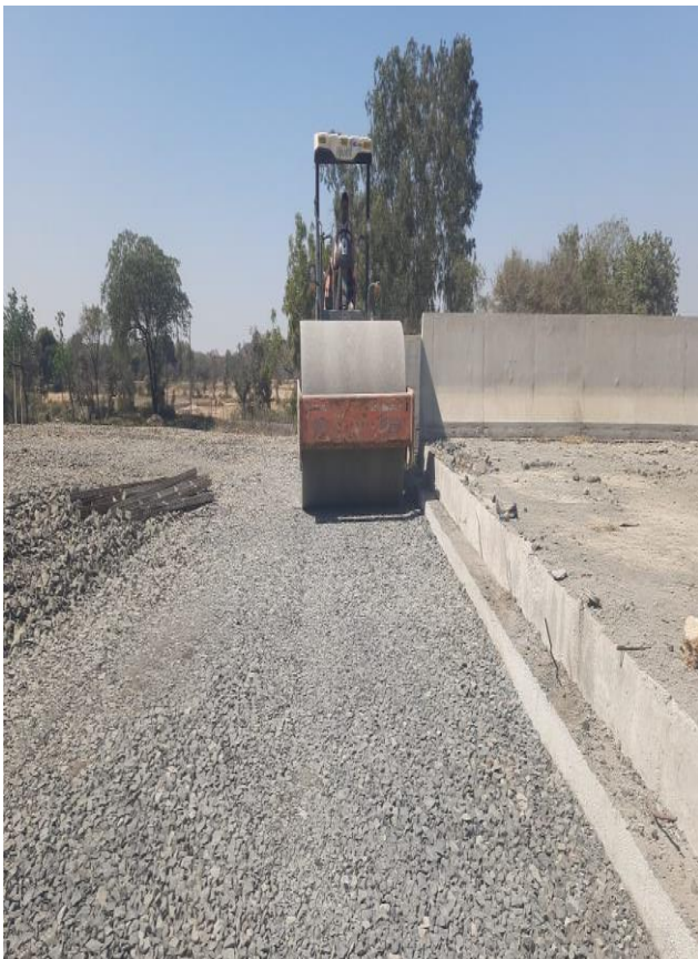
Ch.119+903 SVUP RHS Approach Slab Bed Rolling.
