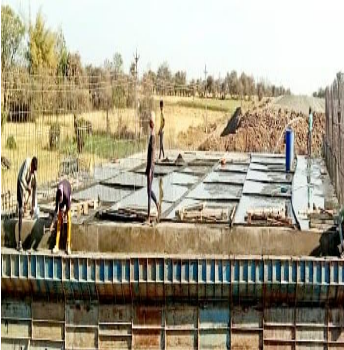
Ch.120+682 MNB RHS Span Top Slab Curing Continue.
