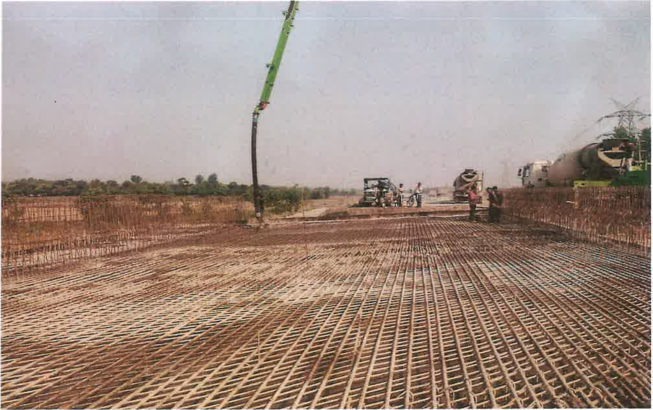
MNB Slab Concrete Pouring Work in Progress at Ch. 20+820
