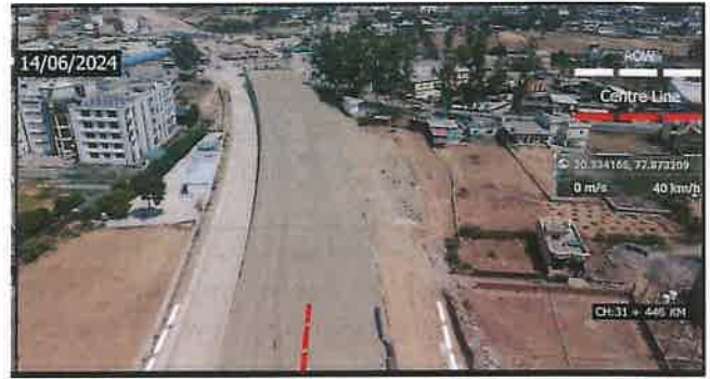
Ch. 31400 to 31480 RHS , Drain & Service Road Work
