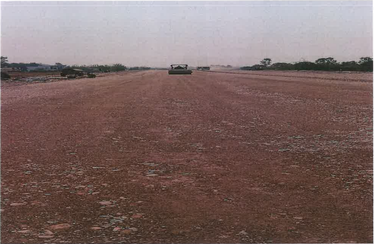
GSB Top Rolling Work in Progress at Ch. 32+060 to 32280
