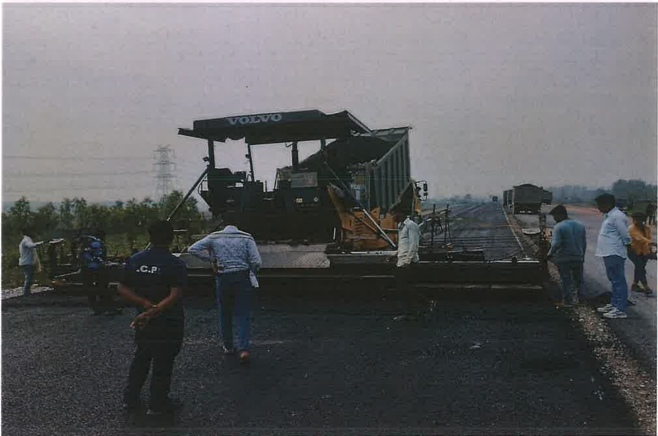
DBM Laying Work in Progress at Ch. 24+150 to 24+800 LHS
