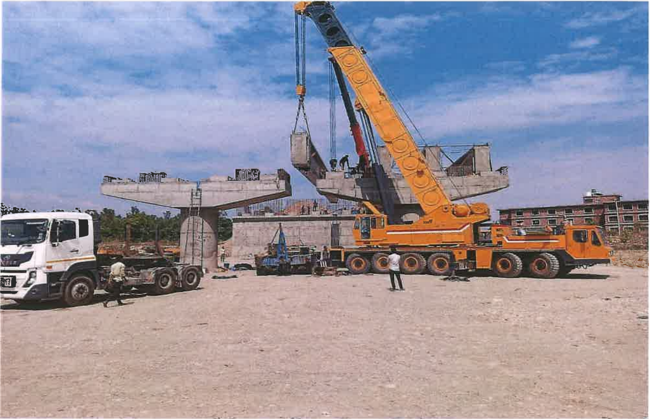
MJB Girder Launching Work in Progress at Ch. 33+033
