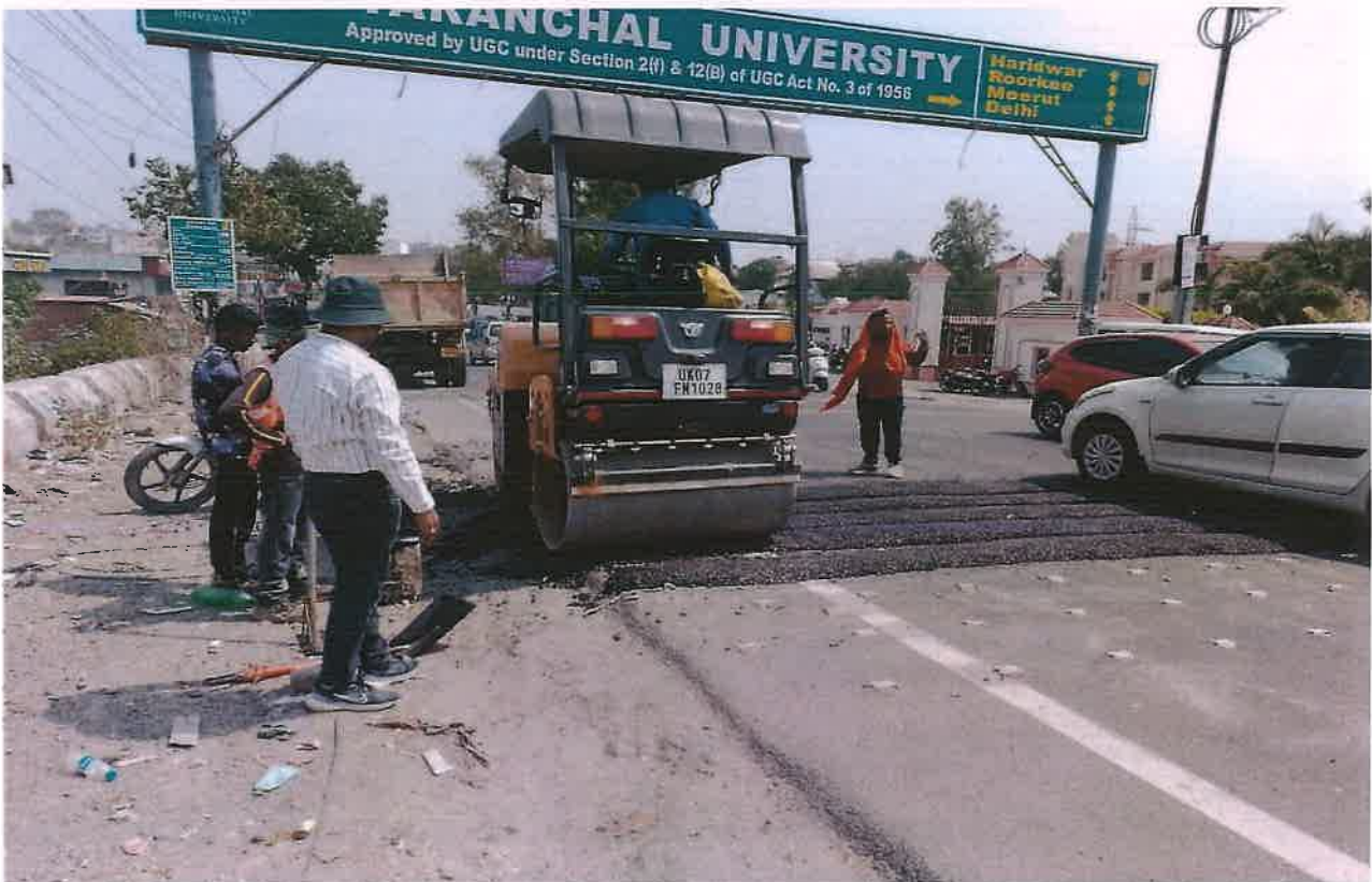
Speed Breaker Making Work in Progress at Black spots
