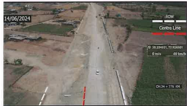
Ch. 34520 to 34770 LHS, MCW & Service Road Work
