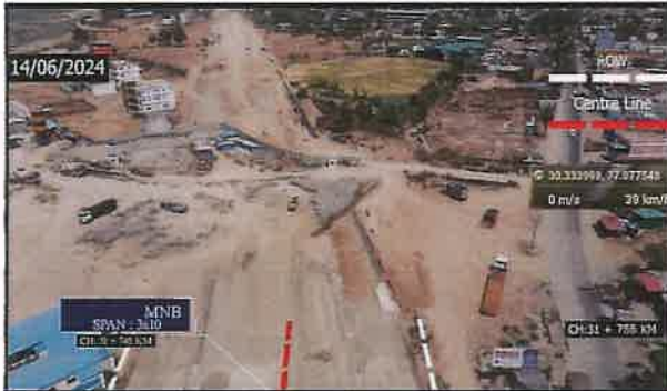
Ch. 31770 to 31850 BHS, Highway Work
