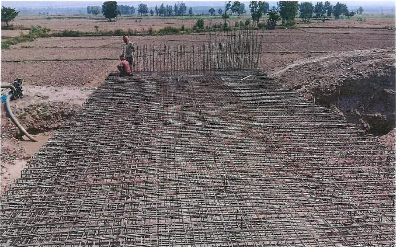
Box Culvert Slab Reinforcement Binding Work in Progress at Ch 21+283
