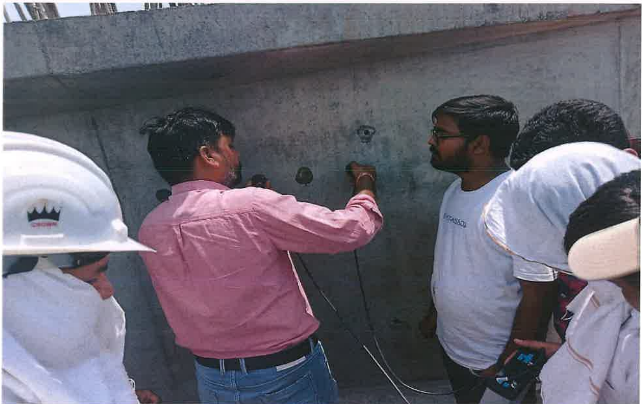
MJB Girder NDT Testing at Ch. 33+033
