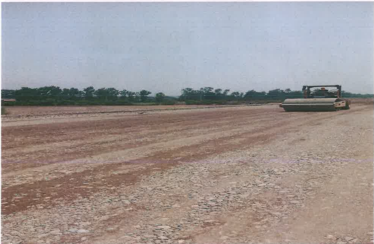
GSB Top Rolling Work in Progress at Ch. 33+700 to 33+950
