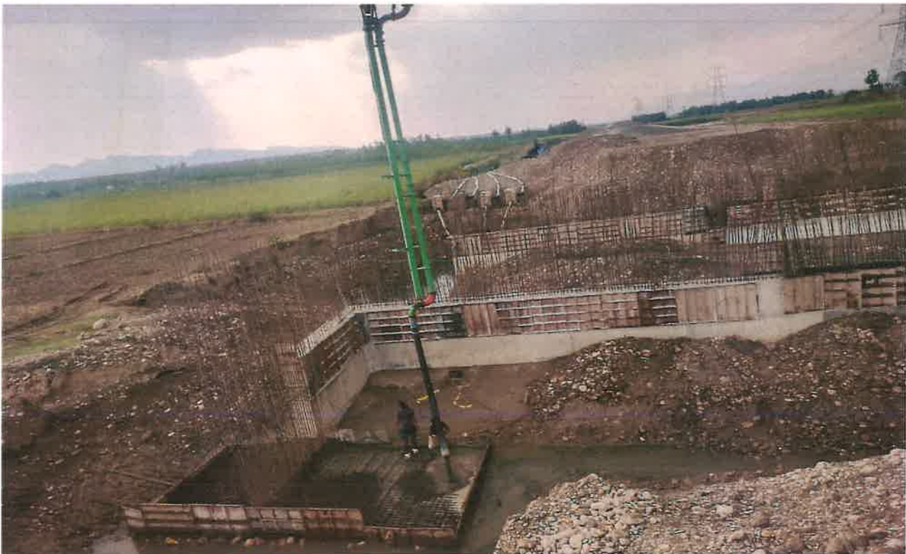
MNB Retaining Wall Raft Concrete Pouring Work in Progress at Ch. 21+610
