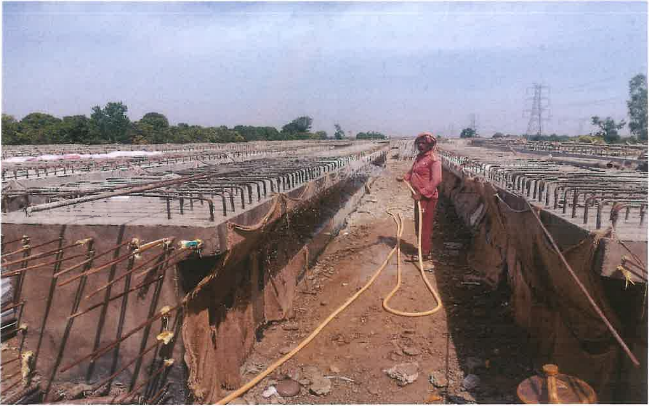
RCC Girder Curing Work in Progress at Ch. 22+598
