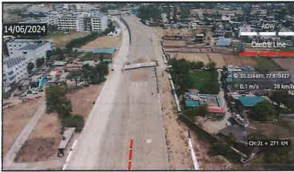
Ch. 31280 to 31300 RHS , Drain & Service Road Work
