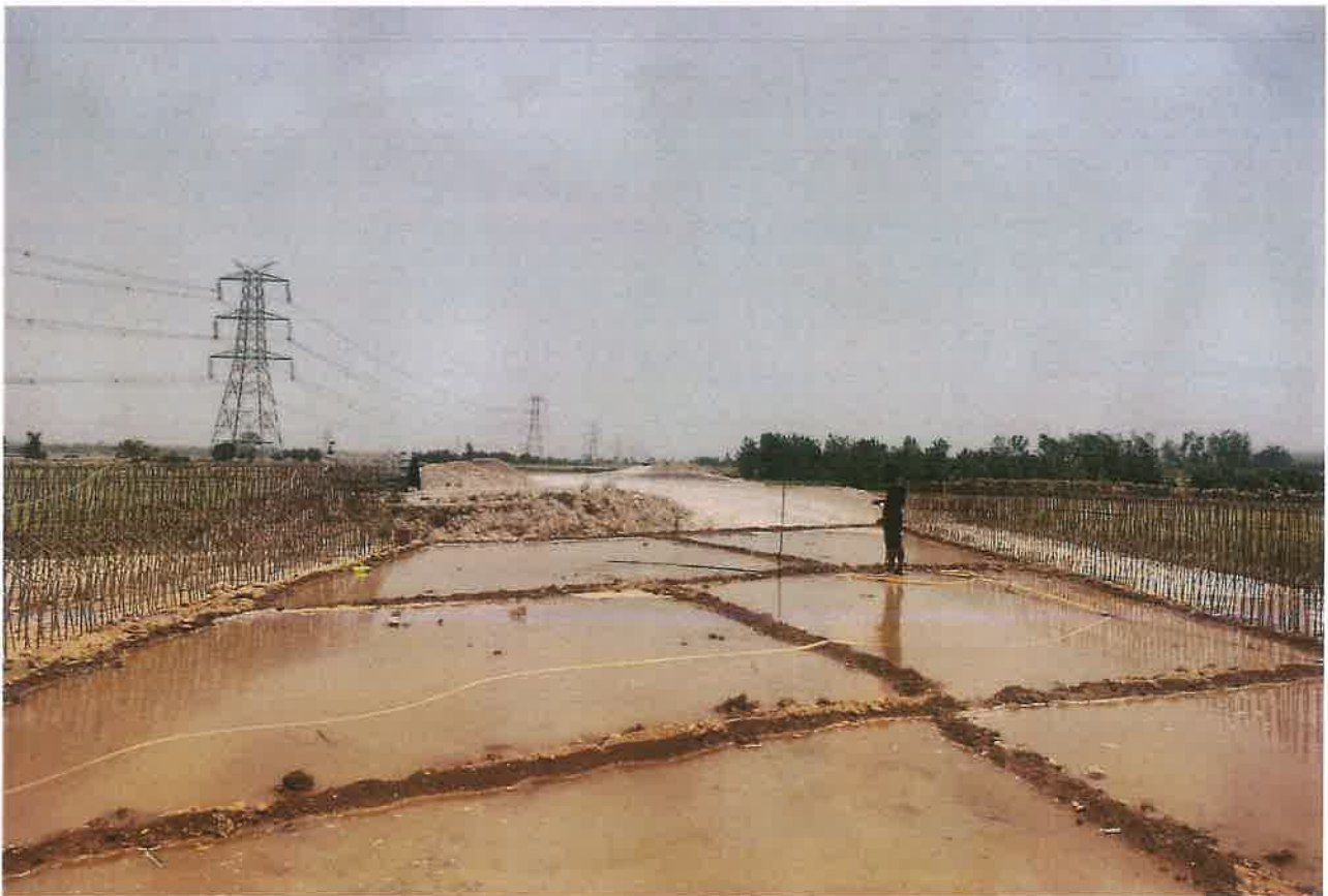
MNB Slab Curing Work in Progress at Ch 20+820
