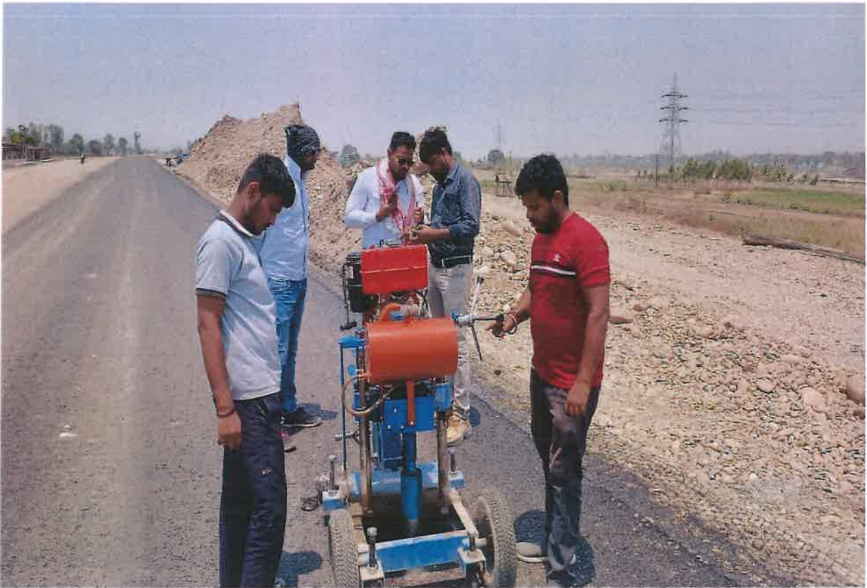
DBM Core Cutting & Thickness Checking with IE Team at Ch. 29+420 RHS
