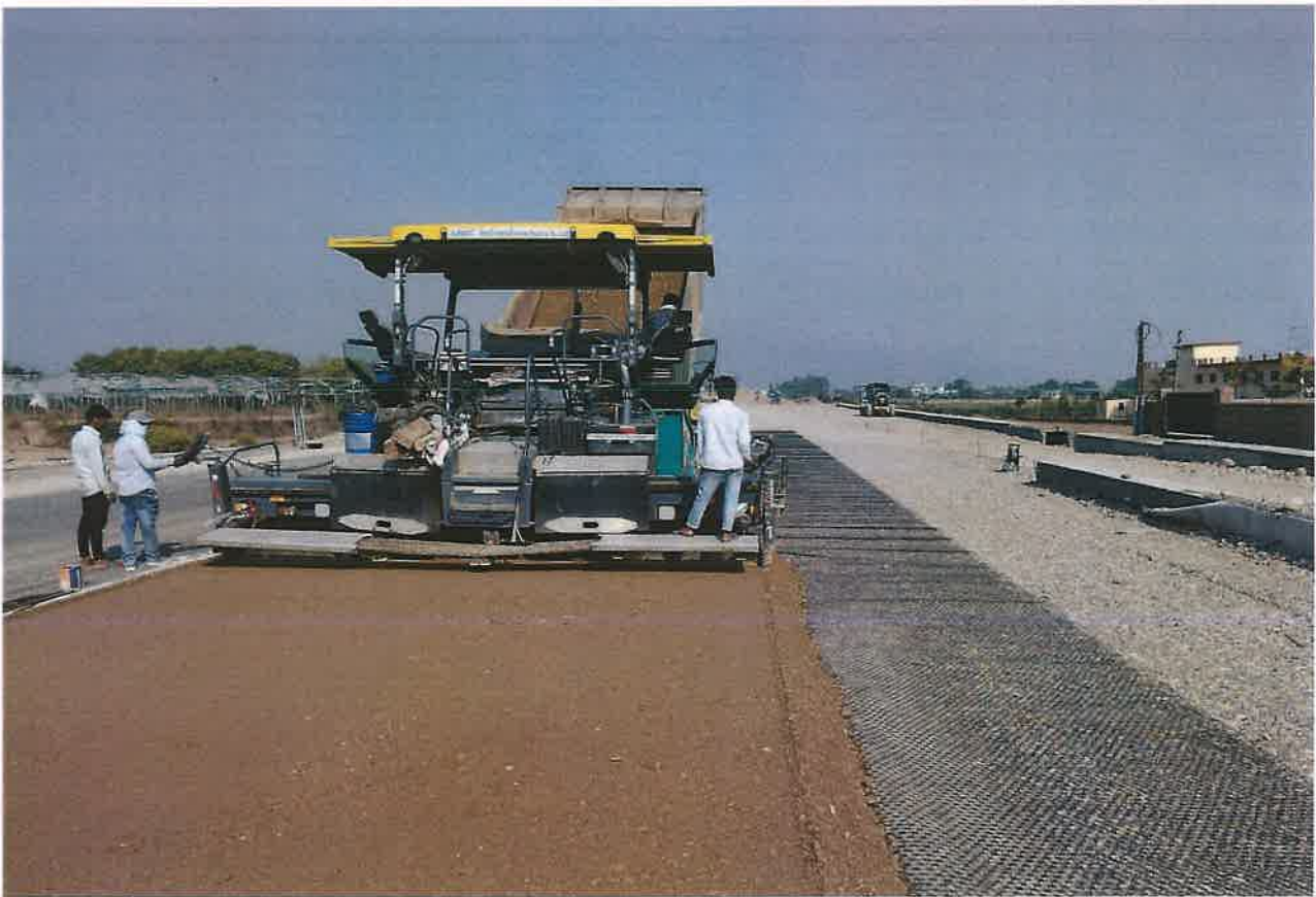
WMM Laying Work in Progress at Ch 29+700 to 29+950 (RHS)
