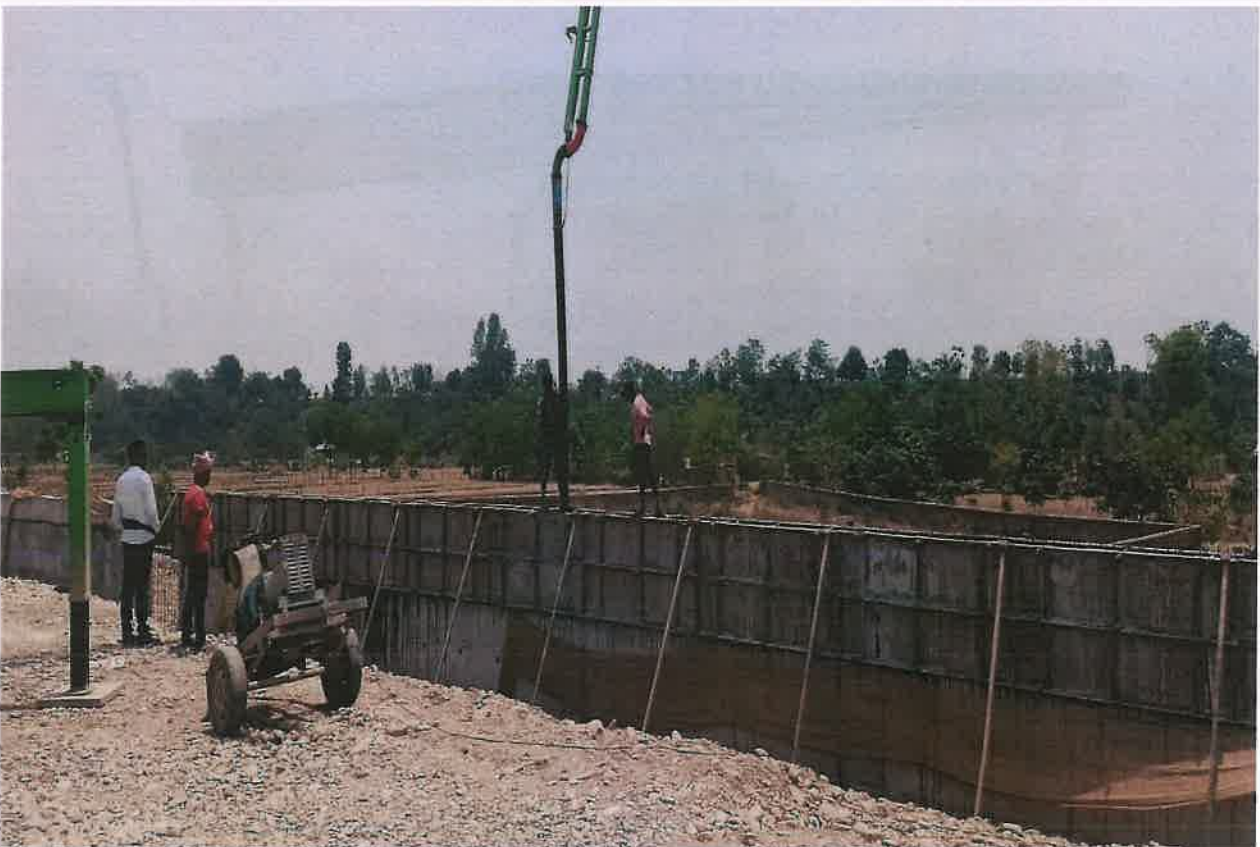
Retaining Wall Pouring Work in Progress at Ch. 35+400 RHS
