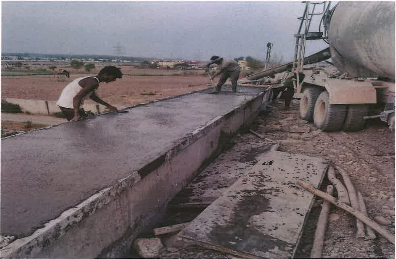
Drain Slab Casting Work in Progress at Ch. 29+410 LHS
