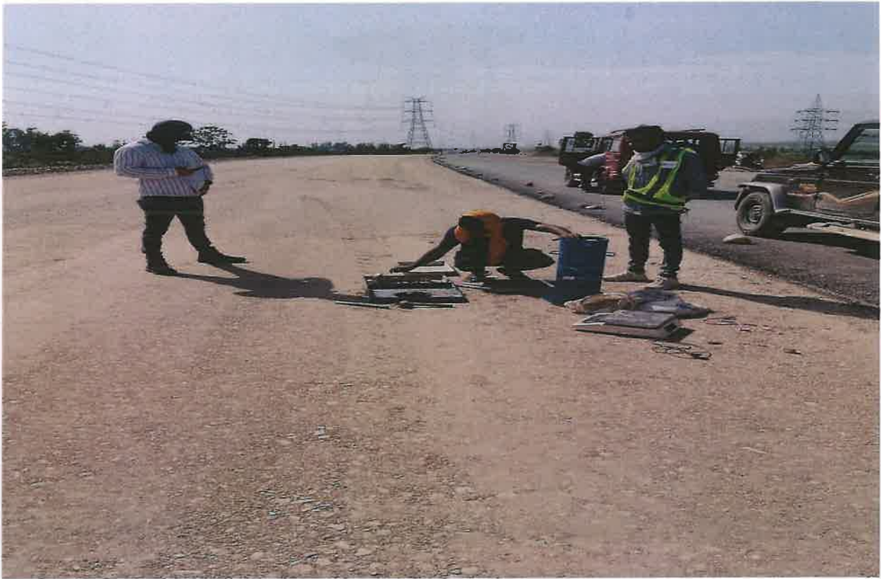
FDD Checking on WMM Top Layer at Ch. 26+500 to 26+950 RHS
