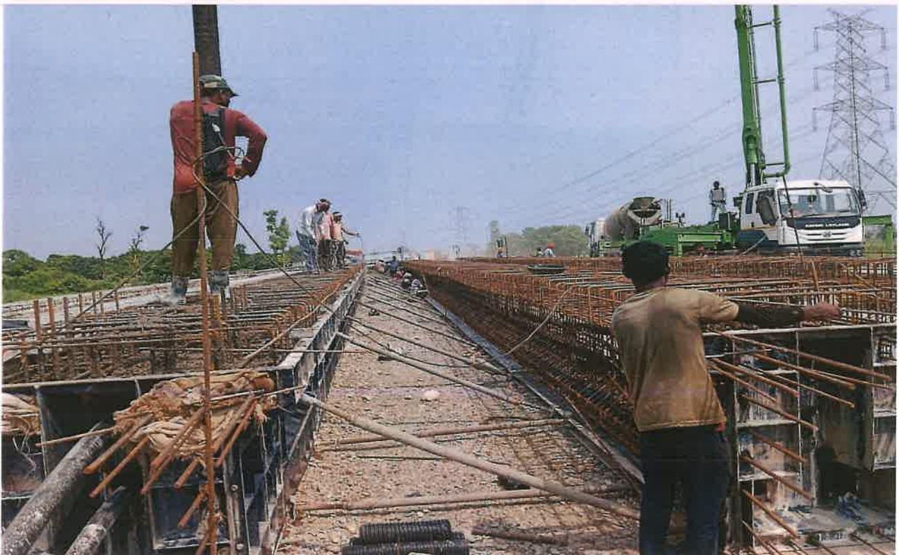
VUP PSC Girder Casting Work in Progress Ch. 22+598
