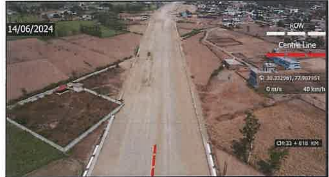
Ch. 33650 to 33680 LHS, Drain & Service Road Work
