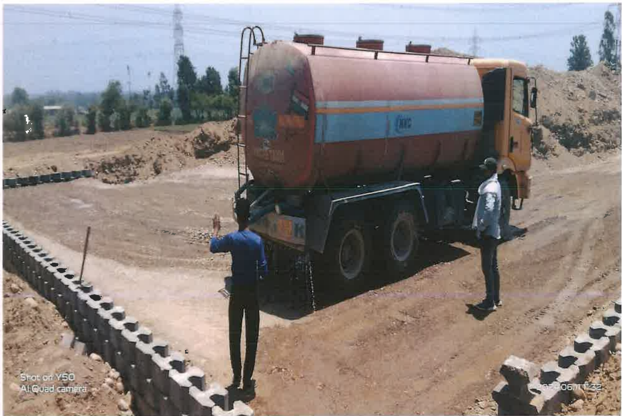
Watering of RE Wall Closing Wall at ch-22+630
