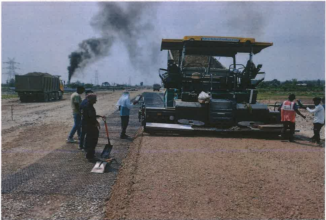
WMM Laying Work in Progress at Ch 24+800 to 25+050 (RHS)
