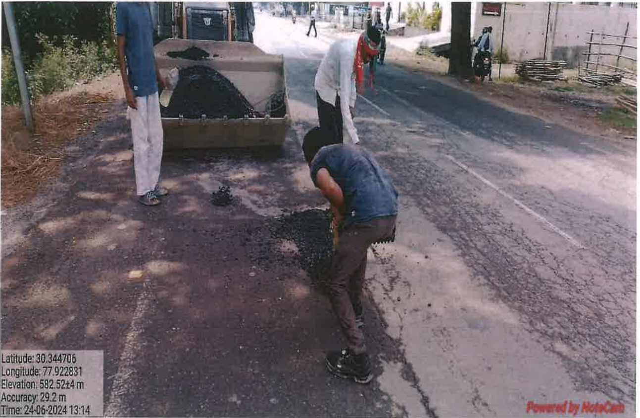
Existing road maintenance Work in Progress at Jhajhra
