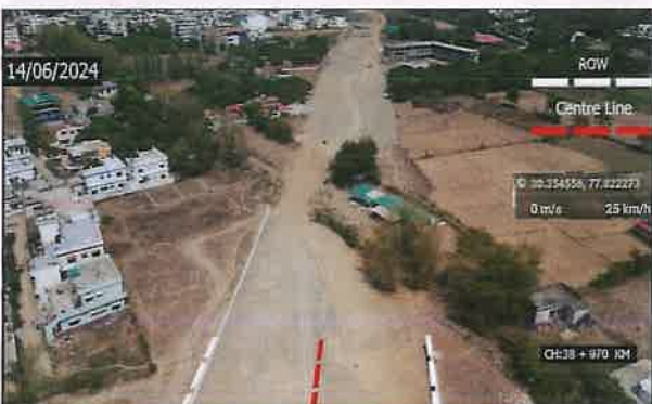
Ch. 39000 to 39120 BHS, Highway Work
