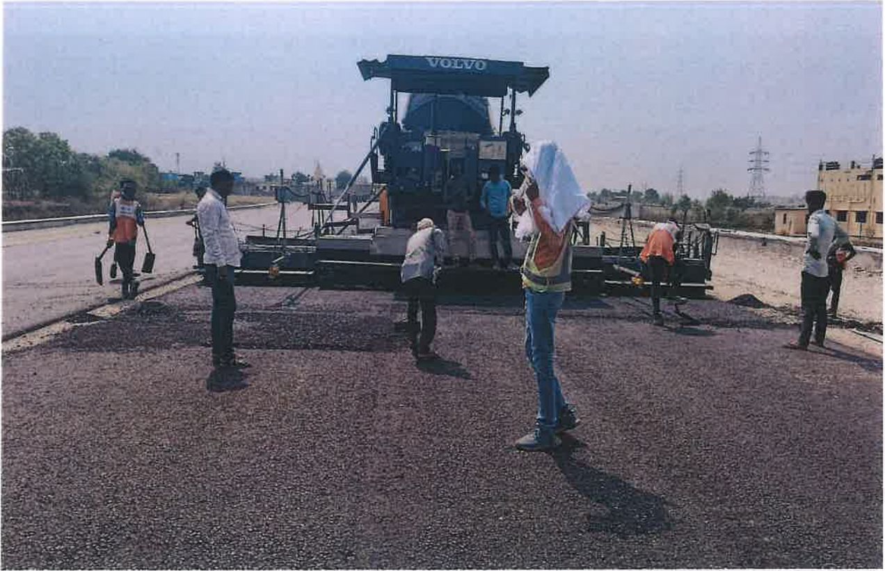
DBM Laying Work in Progress at Ch 29+680 to 29780
