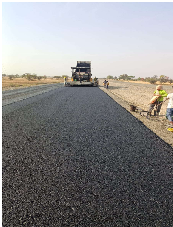
DBM laying Ch 128670 to 129660 LHS
