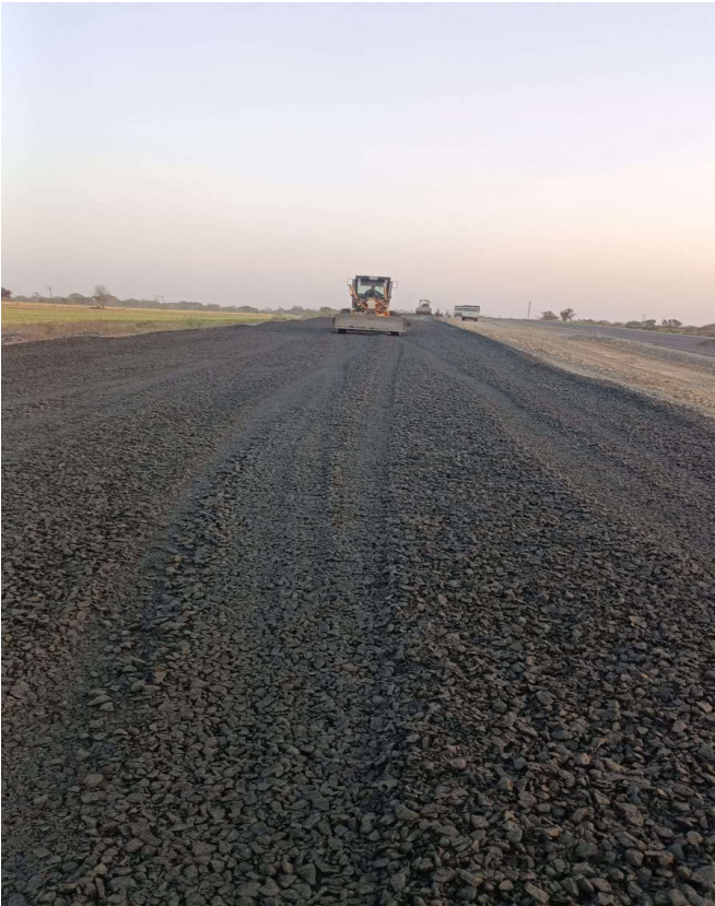
Wmm top laying work in progress LHS at ch 100240 to 100580 RHS
