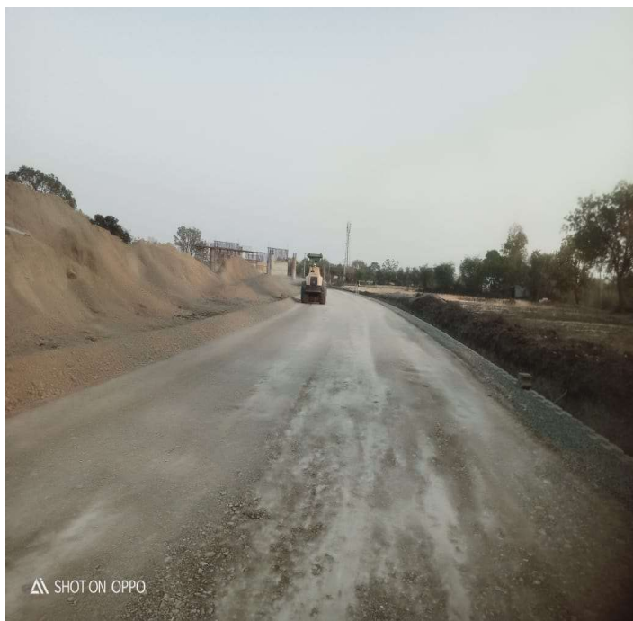
ROB Re block A2 side rolling work in progress Ch 112+840 to Ch. 112+980 BHS
