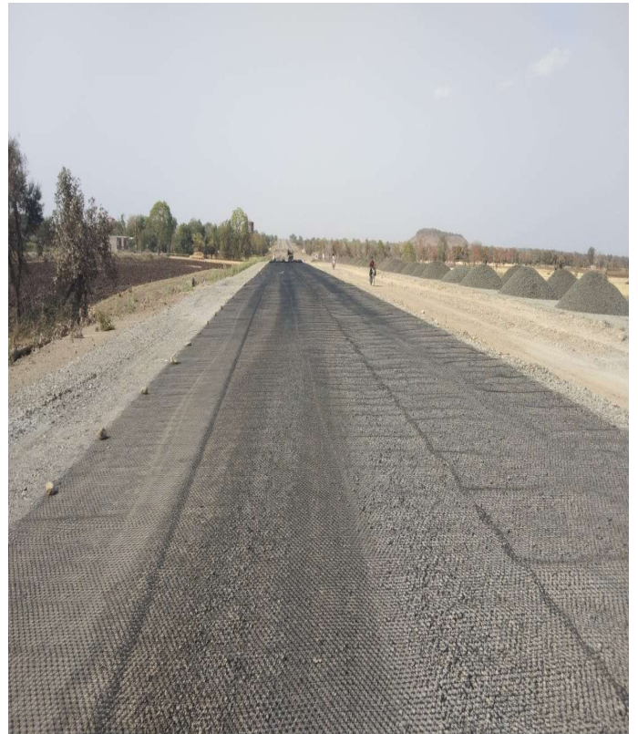
Geo grid laying work in progress Ch 100240 to 100580
