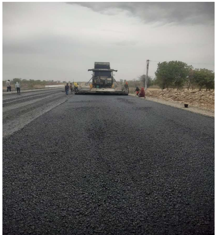
Dbm top laying at ch 113+540 to 113+720 rhs
