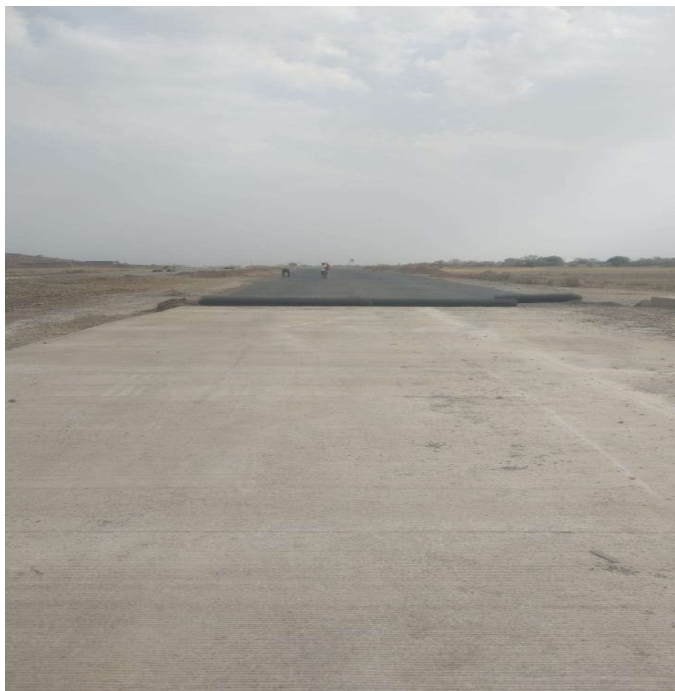
Geo grid laying work in progress
