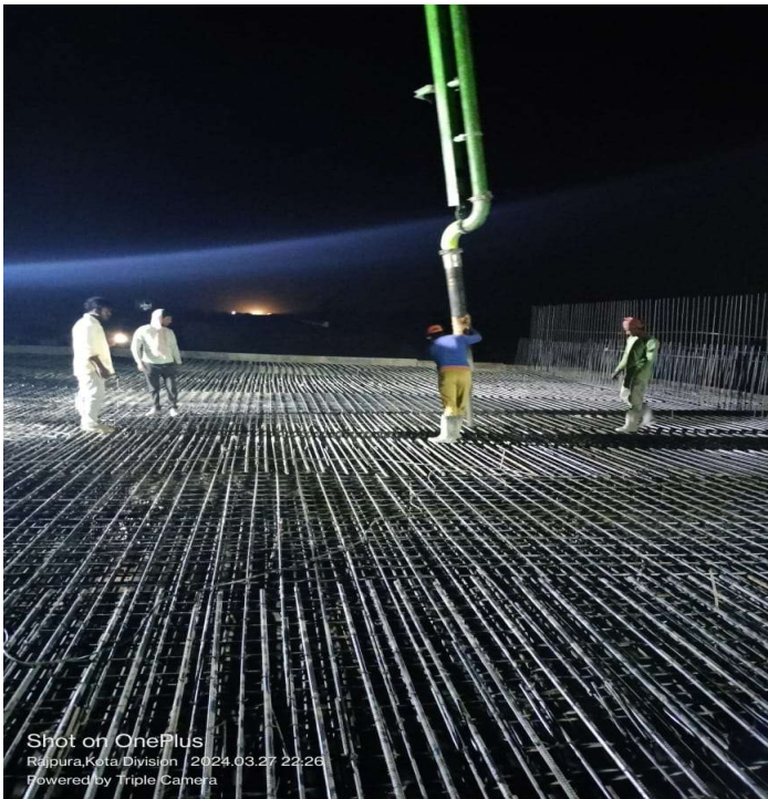
MNB RHS SLAB CONCRETE POURING START 90+028
