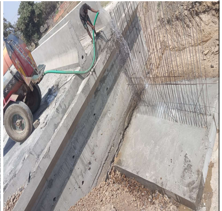
Retaining wall bottom Raft curing work is in progress @Ch 125+281 MNB
