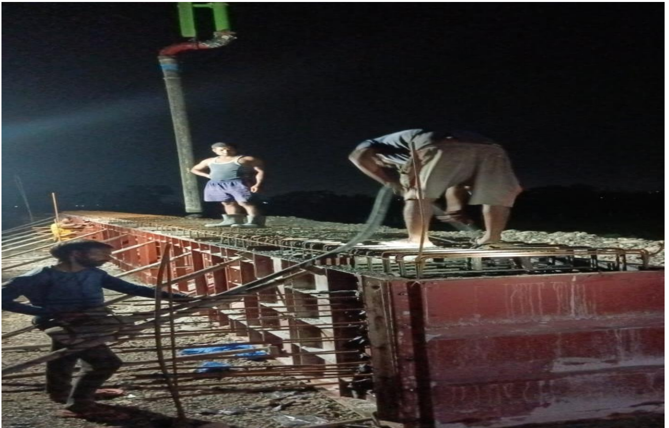
VUP RCC Girder Casting Work in Progress at Ch. 31+000
