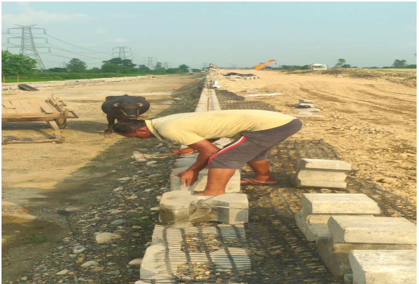
RE Wall Erection Work in Progress at Ch-22+170 LHS
