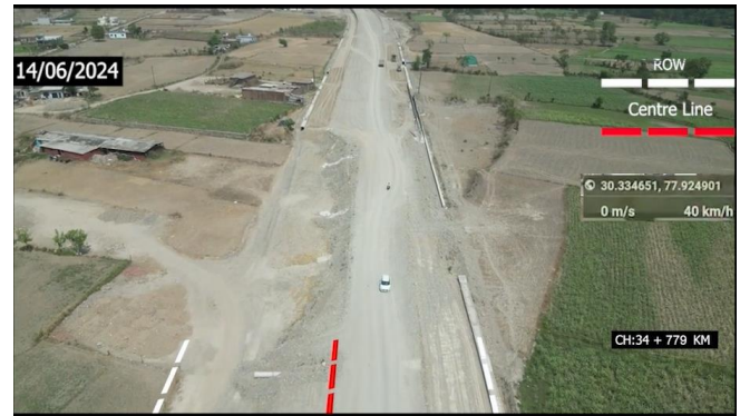
Ch. 34520 to 34770 LHS, MCW & Service Road Work
