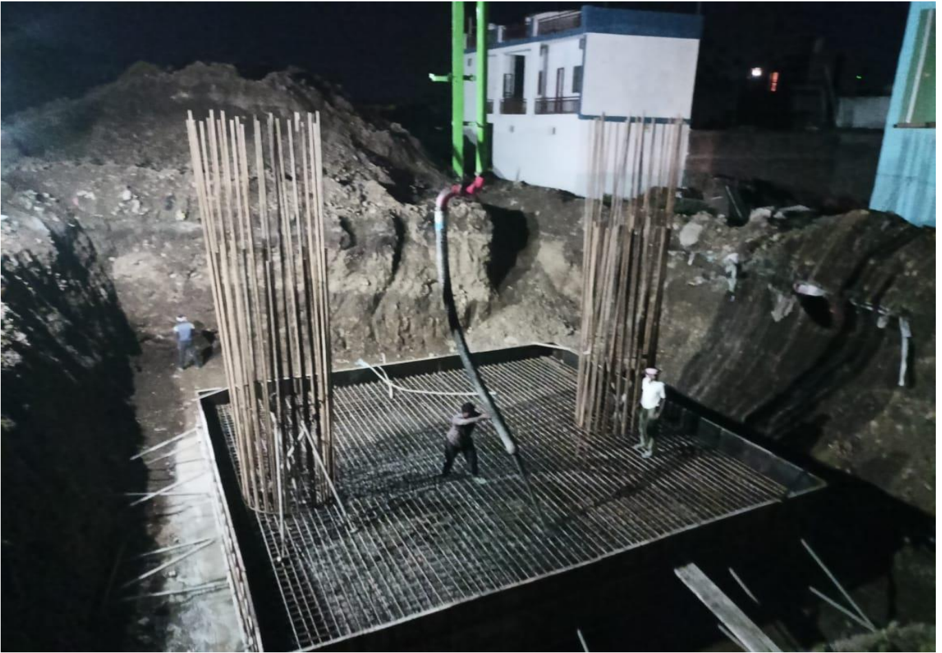
VUP A1 Abutment Foundation Casting Work in Progress at Ch. 40+063
