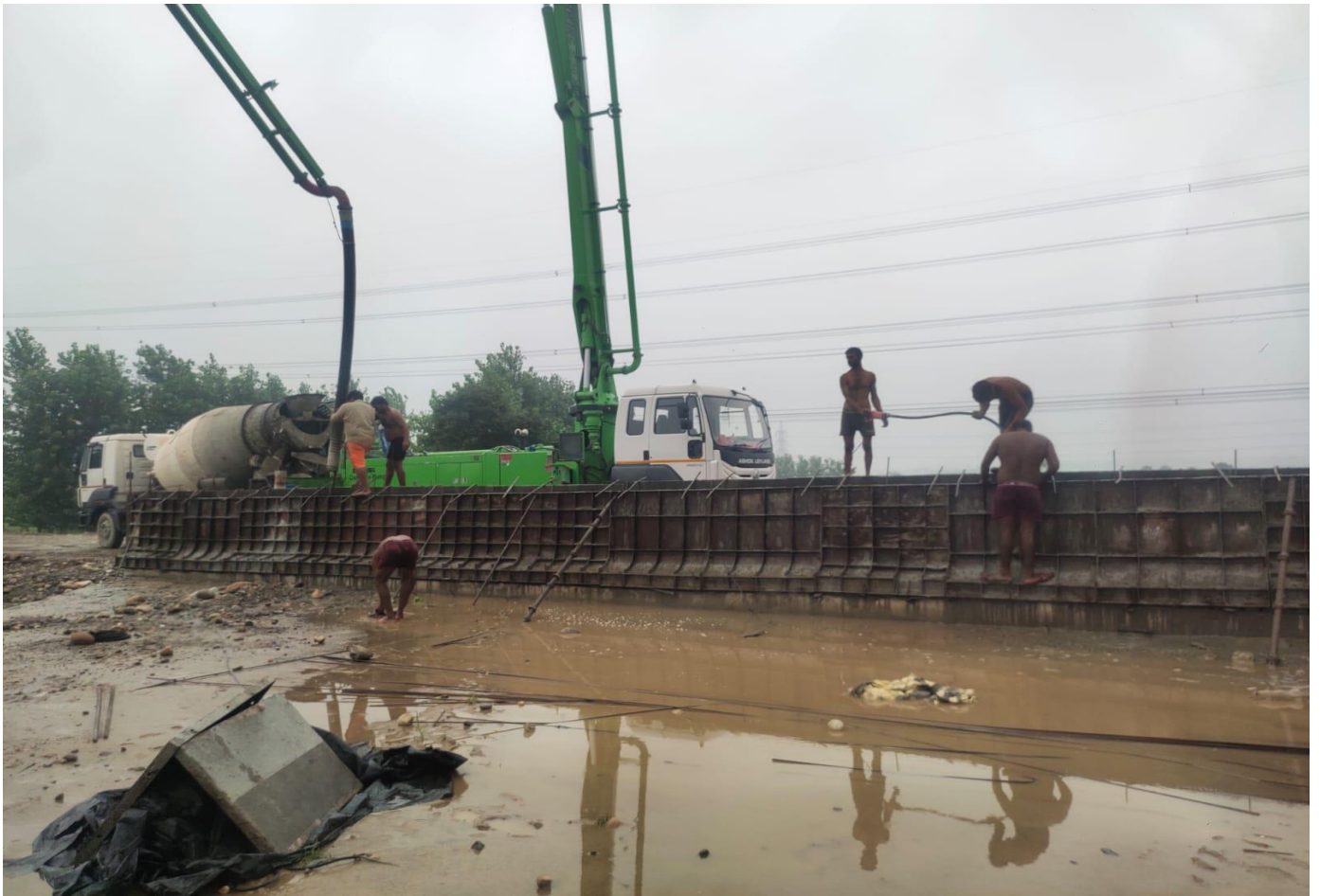
MNB Crash Barrier Casting Work in Progress at Ch. 20+820
