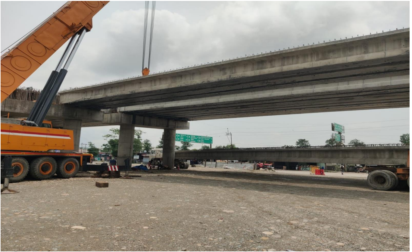
VUP Girder Launching Work in Progress at Ch. 31+691
