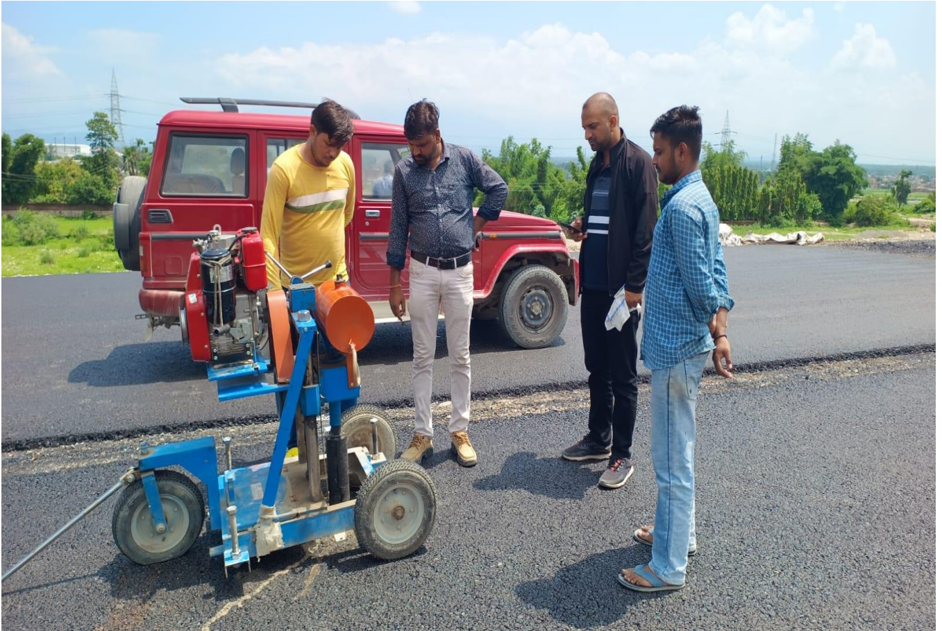
DBM Core Cutting & Thickness Checking with AQME sir.
