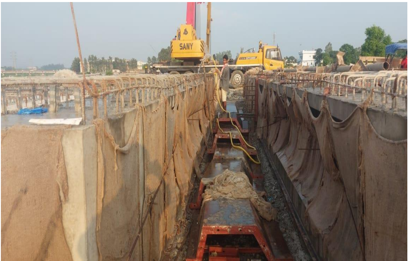
RCC Girder Curing Work in Progress at Ch. 31+000
