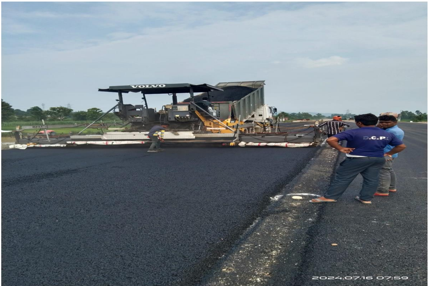
DBM Laying Work in Progress at Ch. 27+800 to 28+080
