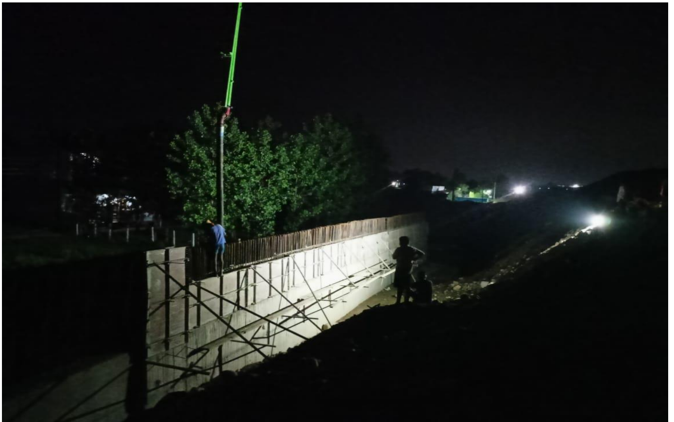
Retaining Wall Pouring Work in Progress at Ch. 32+350 LHS
