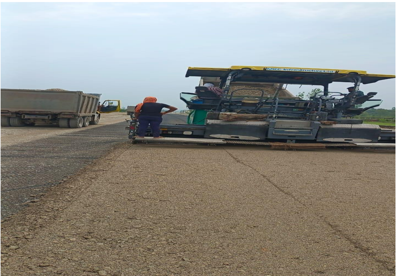
WMM Laying Work in Progress at Ch 35+950 (RHS)
