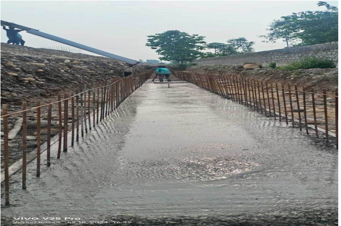
Drain Raft Casting Work in Progress at Ch. 32+520 to 32+560 LHS
