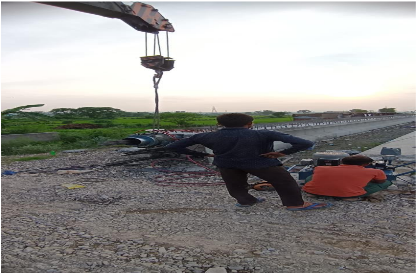
PSC Girder Stressing Work in Progress of VUP CH. 31+691
