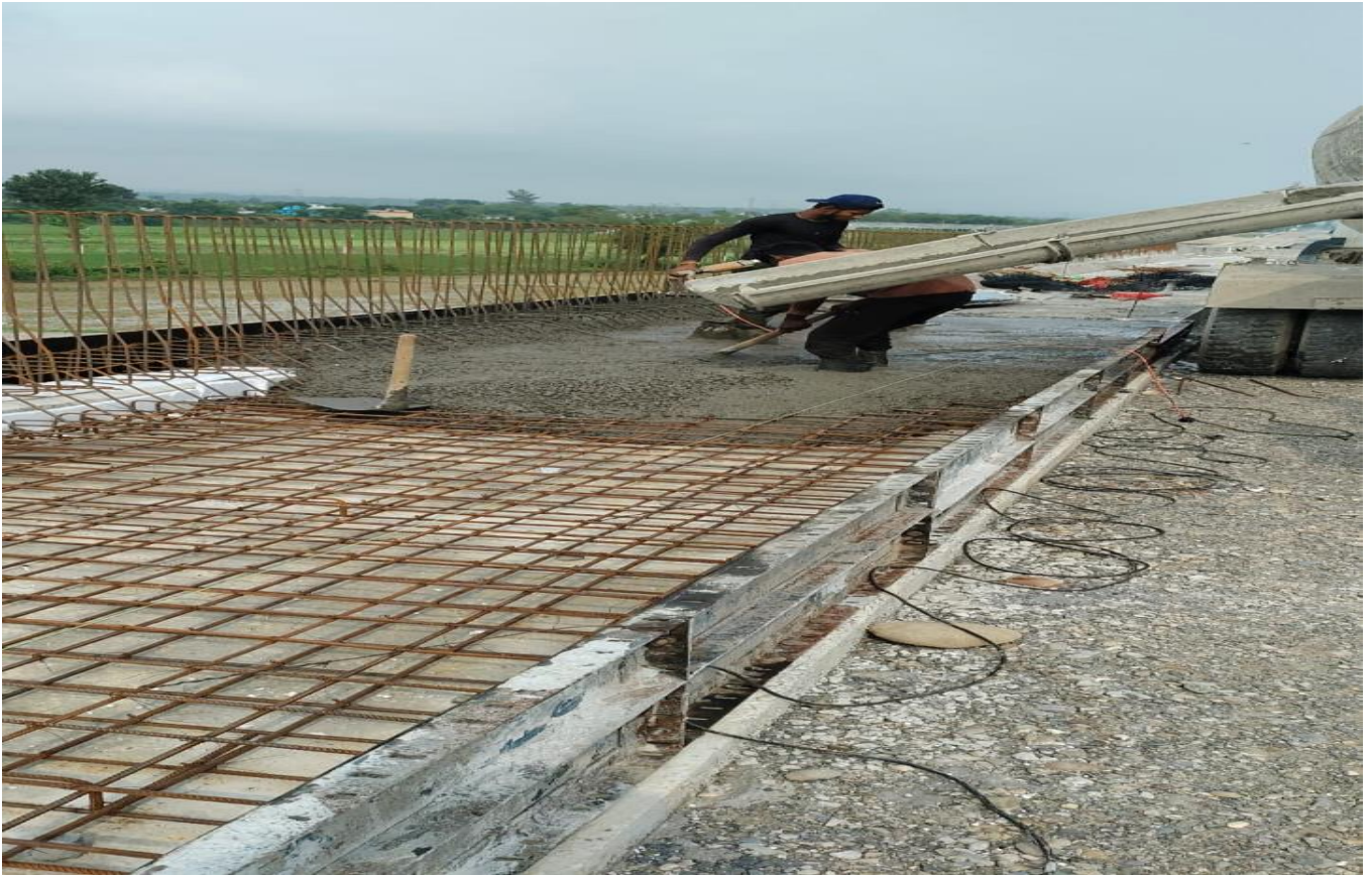
Friction Slab Casting Work in Progress at Ch. 30+200 to 30+220
