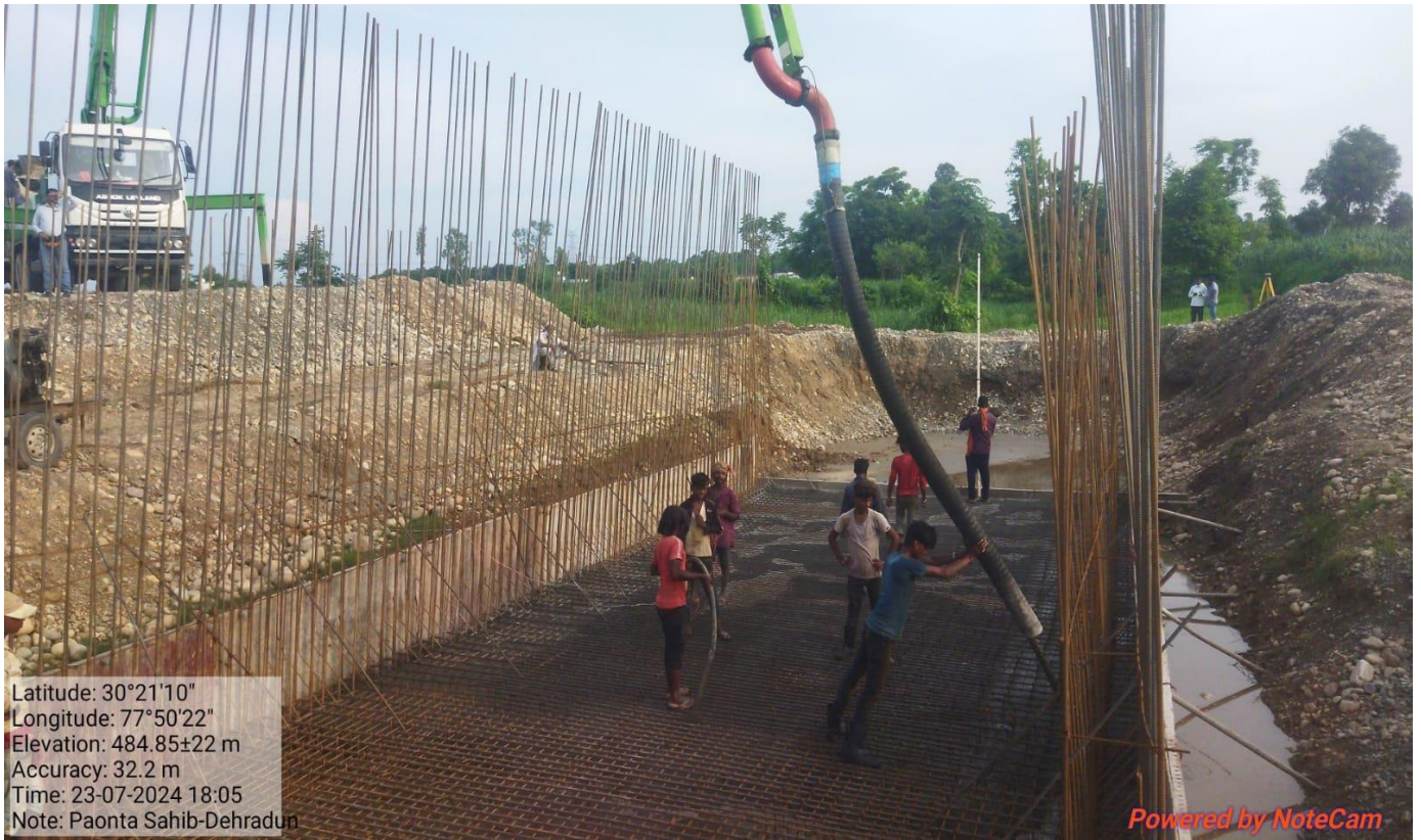
Box Culvert Raft Concrete Pouring Work in Progress at Ch. 27+400
