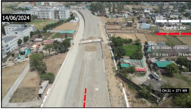
Ch. 31280 to 31300 RHS , Drain & Service Road Work
