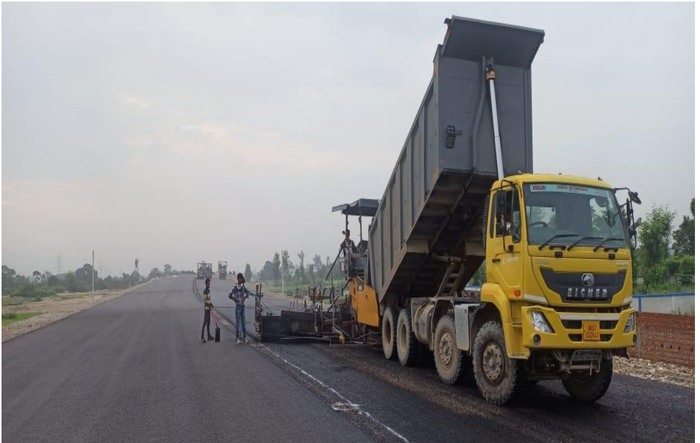
DBM Laying Work in Progress at Ch 27+810 to 28+090
