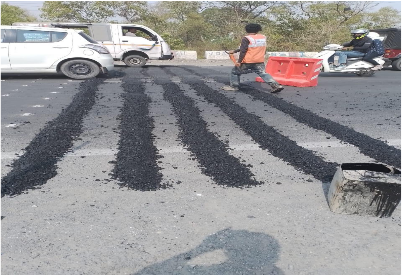
Speed Breaker Making Work in Progress at Black spots
