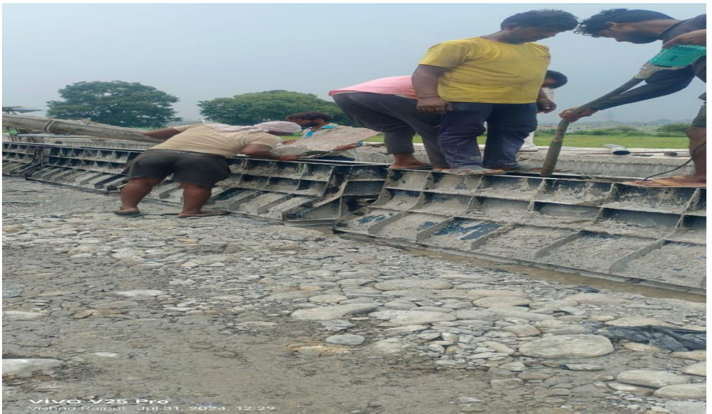
New Jersey Crash Barrier Casting Work in Progress at Ch. 32+200
