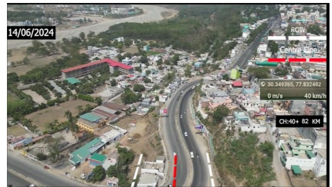
Ch. 40100 to 40350 LHS , Highway Work
