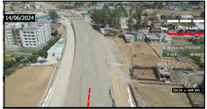
Ch. 31400 to 31480 RHS , Drain & Service Road Work
