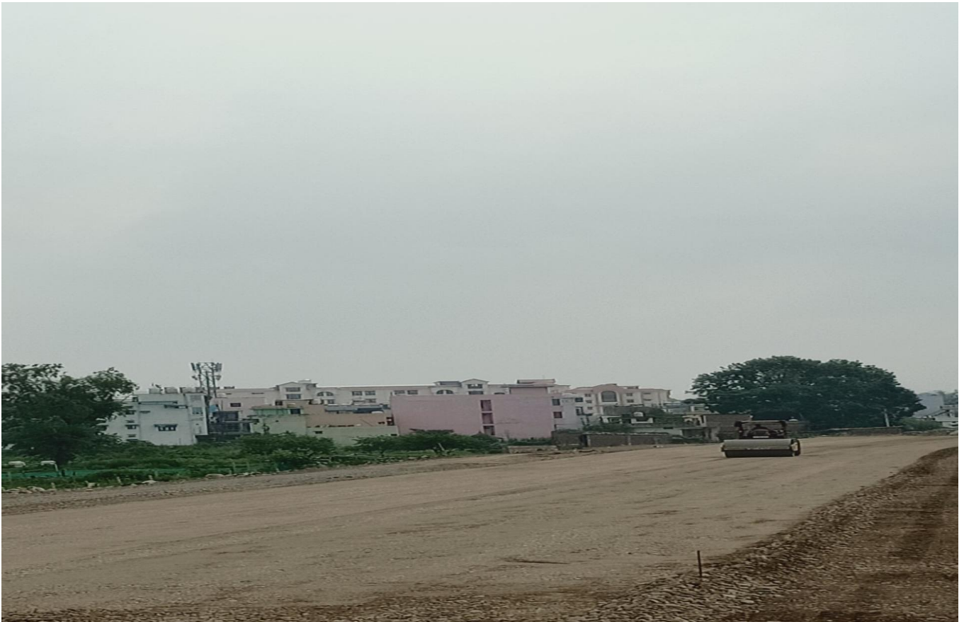
GSB Top Rolling Work in Progress at Ch. 38+600 to 38+780
