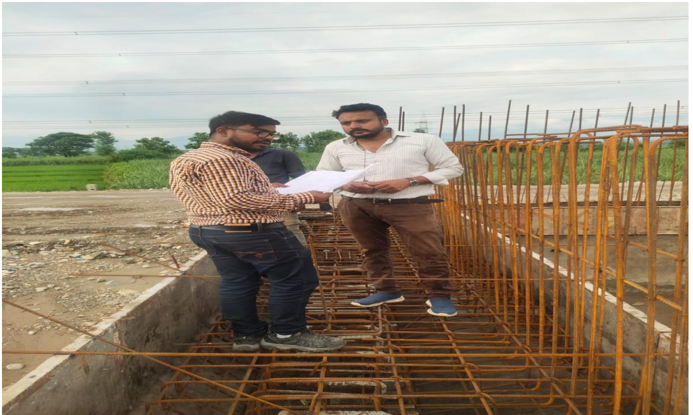
MNB Abutment Cap Reinforcement Checking by ABE Sir at Ch. 21+610
