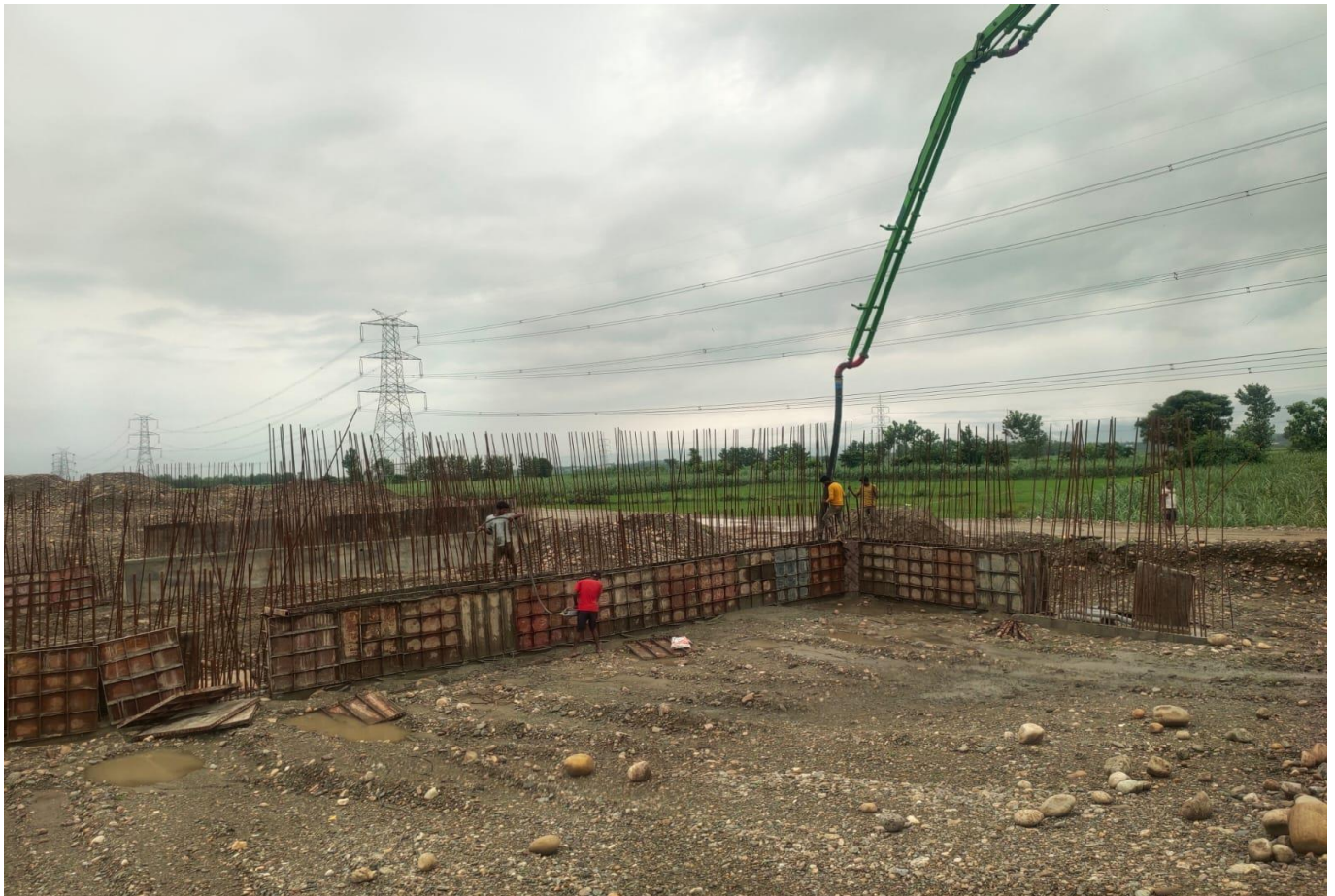
MNB Abutment Wall Concrete Pouring Work in Progress at Ch 21+610
