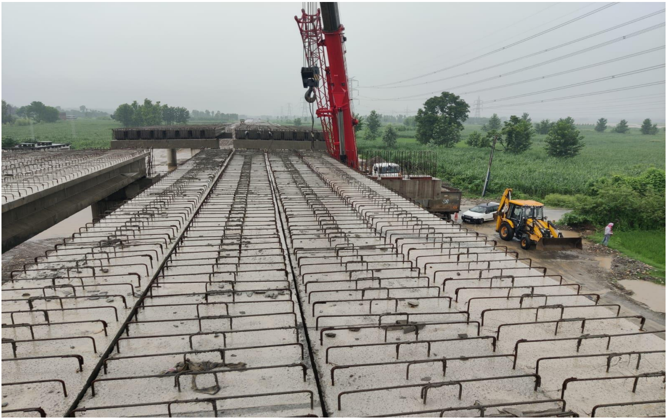
VUP Girder Launching Work in Progress at Ch. 22+598
