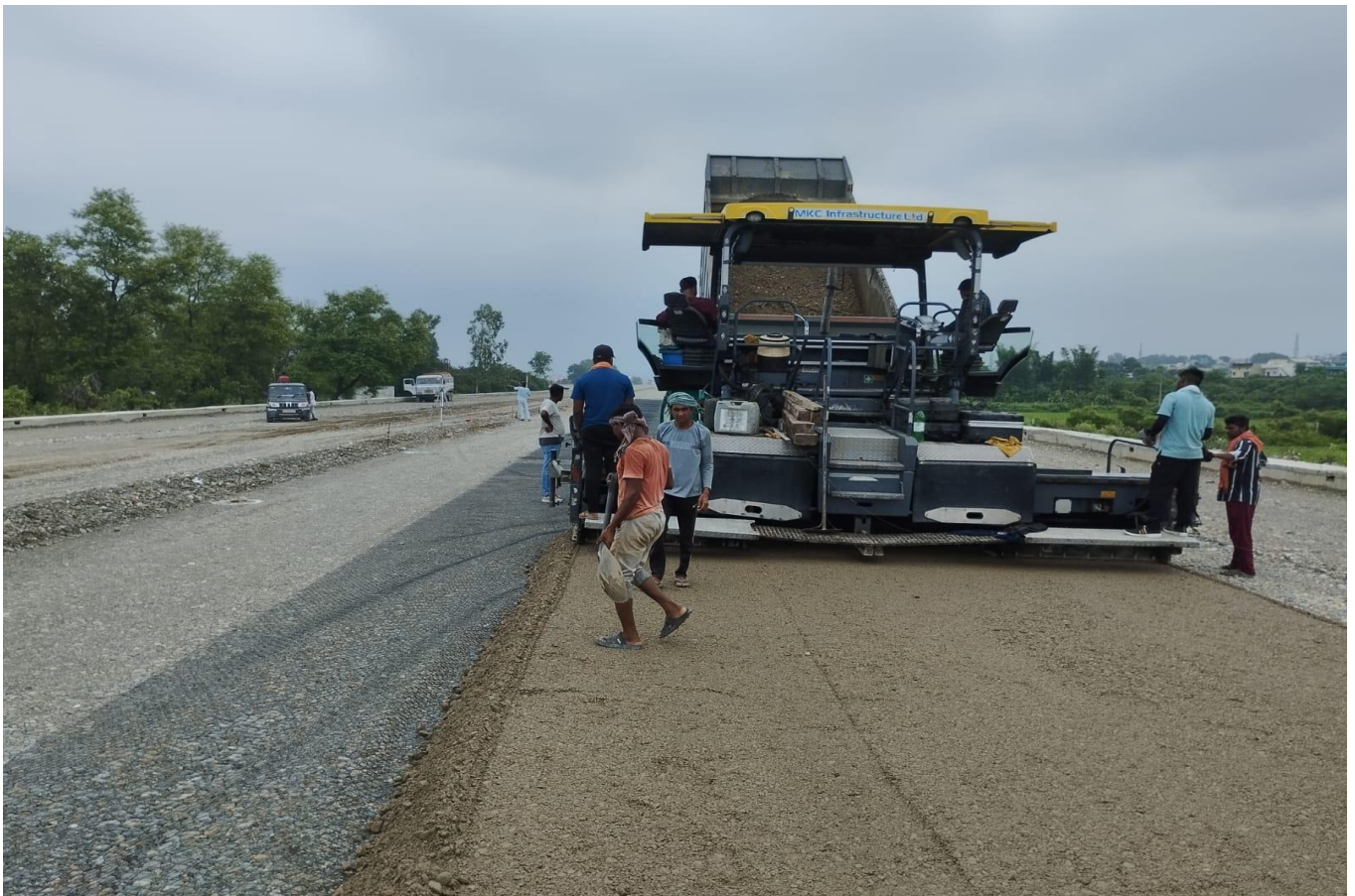
WMM Laying Work in Progress at Ch 37+020 to 37+300 (RHS)
