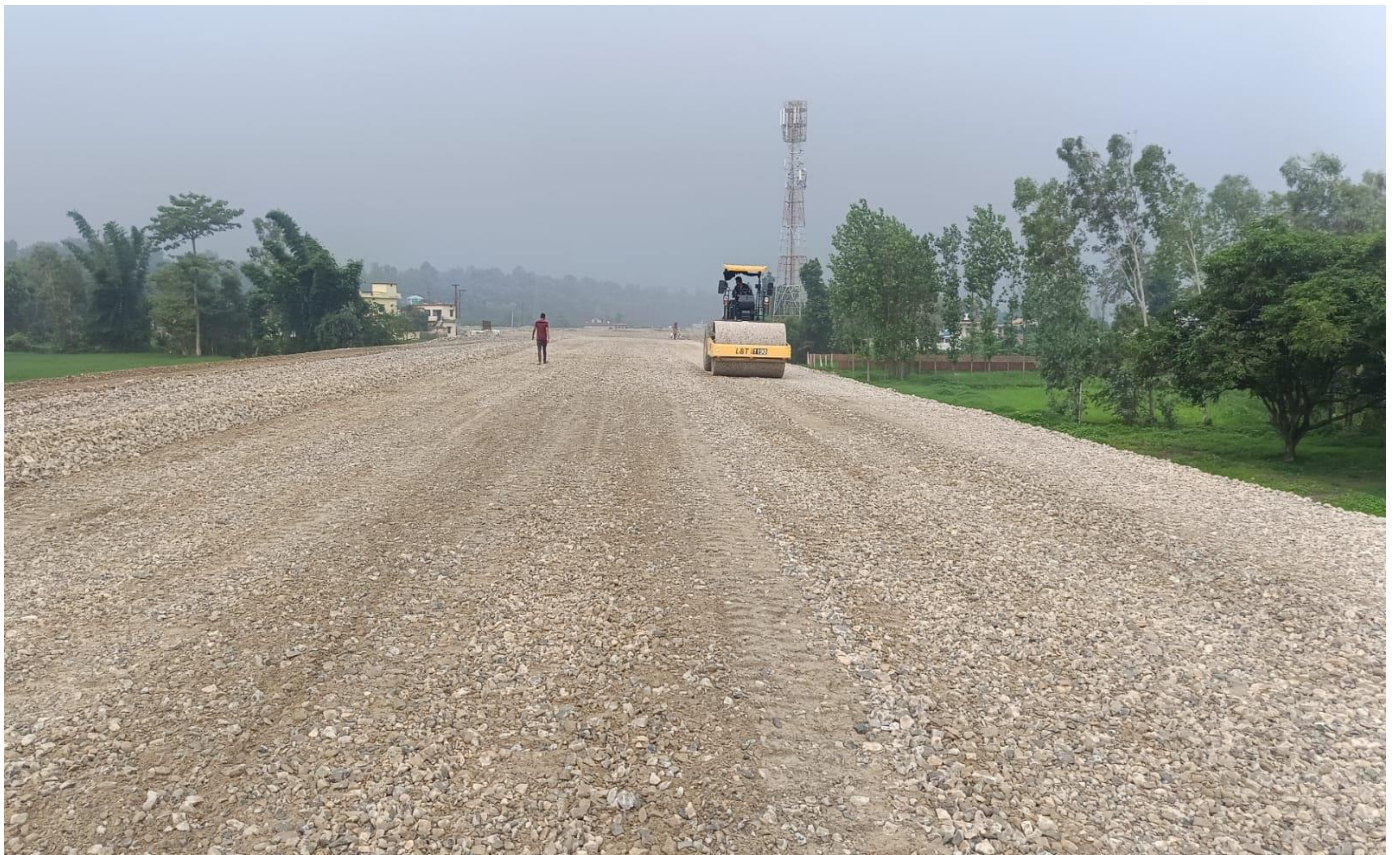
GSB Top Rolling Work in Progress at Ch. 19+100 to 19+280
