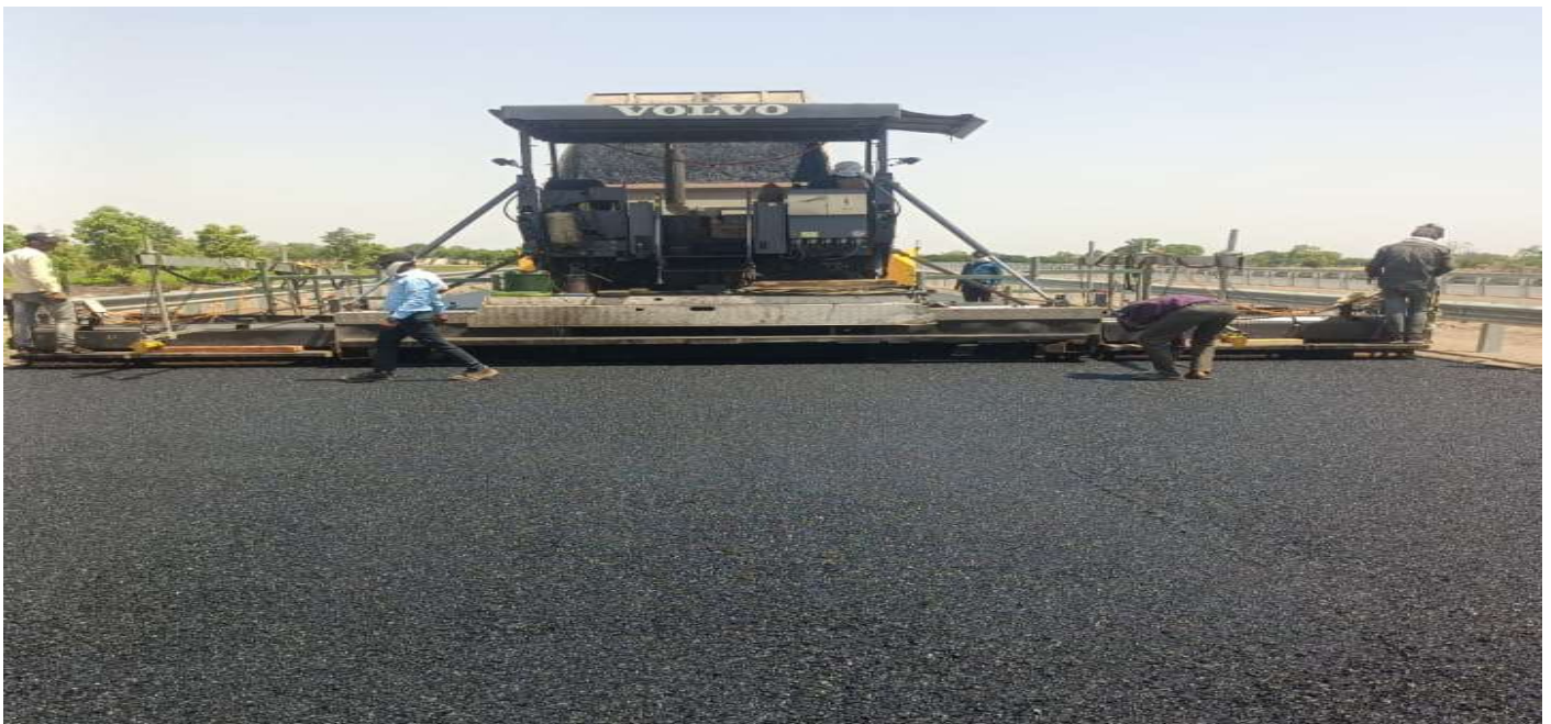
BC laying work in progress at Ch 101230 LHS
