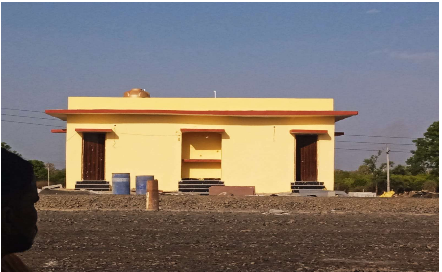
Toilet Block Completed
