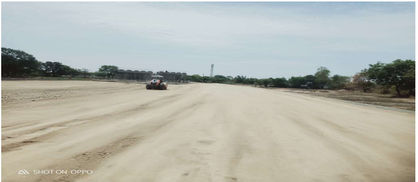
ROB RE BLOCK Rolling work in progress A2 Side
