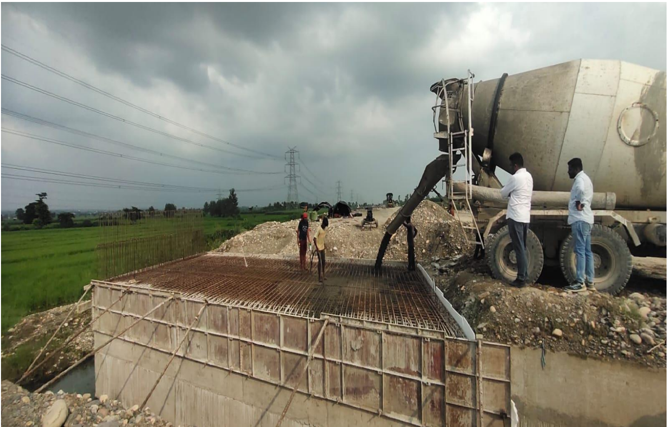
Box Culvert Slab Casting Work in Progress at Ch. 21+108 LHS
