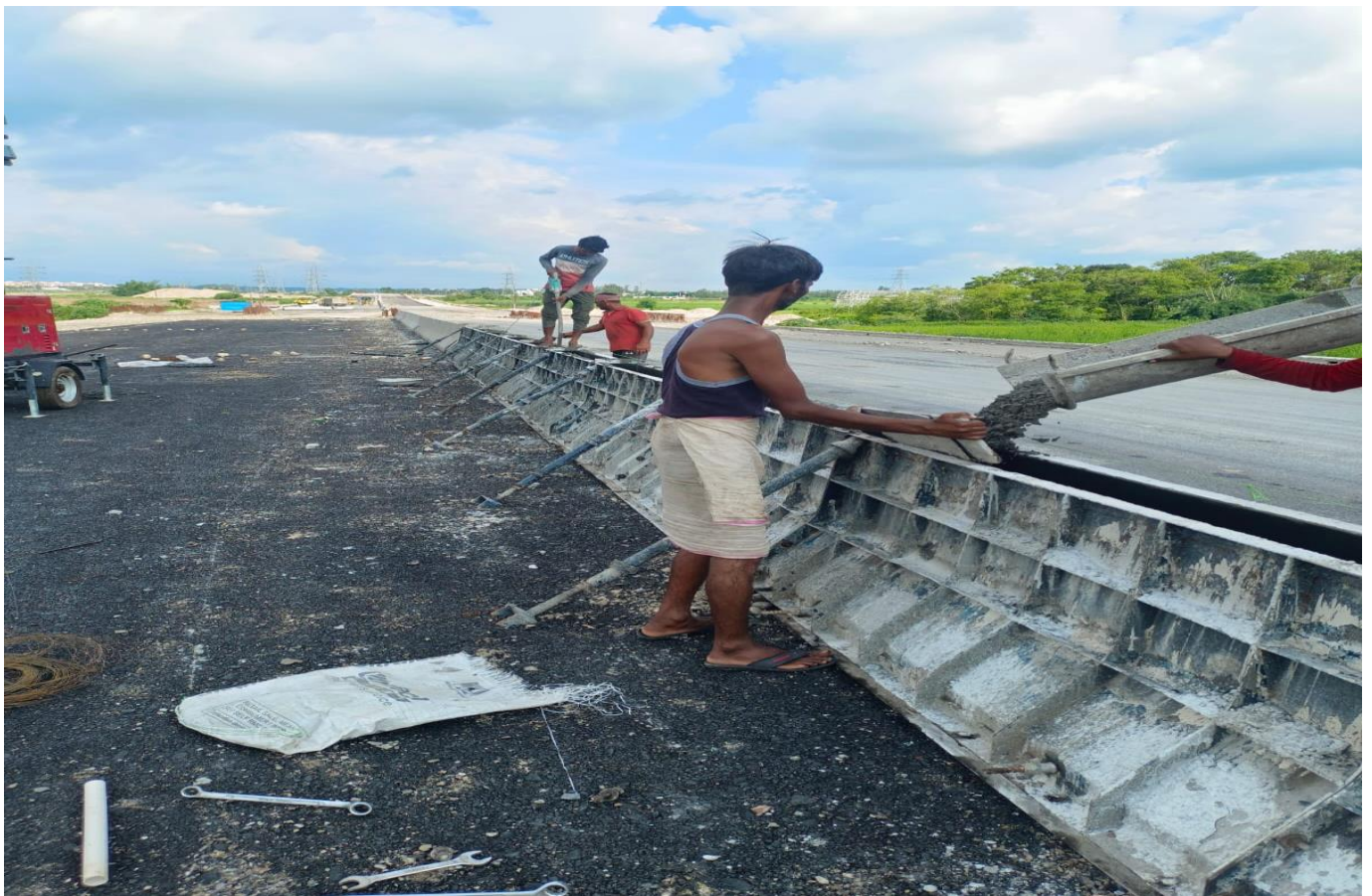
NJCB Casting Work in Progress at CH 29+530 TO 29+550
