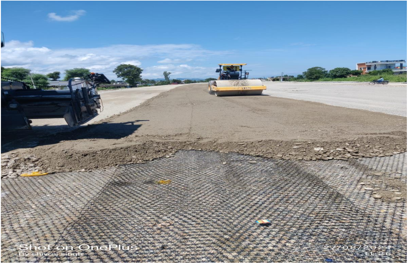
WMM Top Rolling Work in Progress at Ch 29+400
