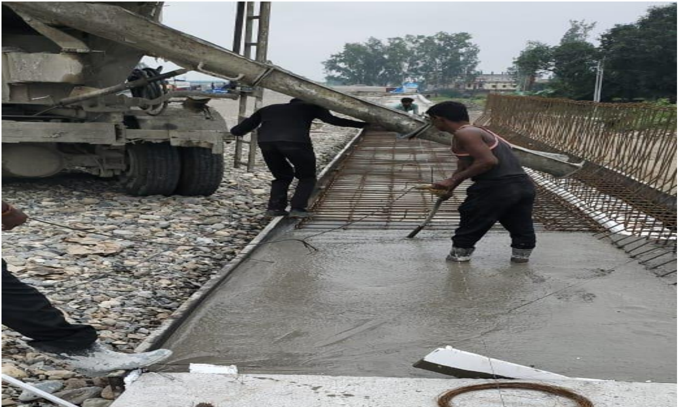
Friction Slab Work in Progress at Ch. 31+253 to 31+273 RHS
