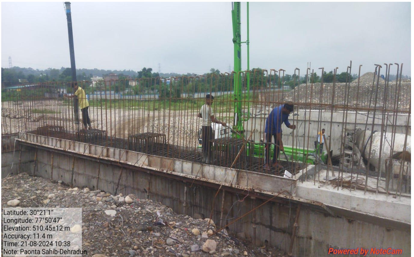
MNB Abutment Cap Casting Work in Progress at Ch. 28+122 RHS
