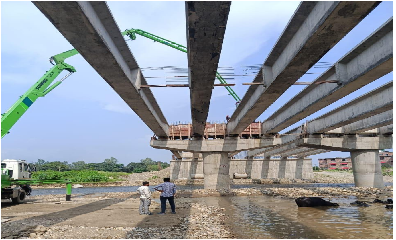
MJB End Cross Girder Casting Work in Progress at Ch. 33+033 LHS
