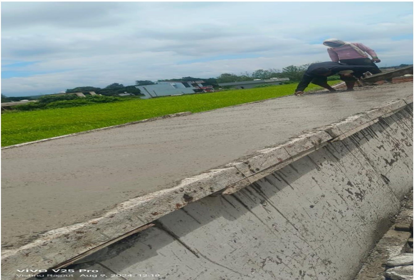
Drain Slab Casting Work In Progress at Ch. 32+533 to 32+545 LHS
