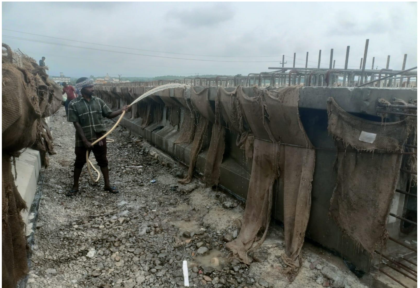
Girder Curing Work in Progress of VUP Ch. 40+063
