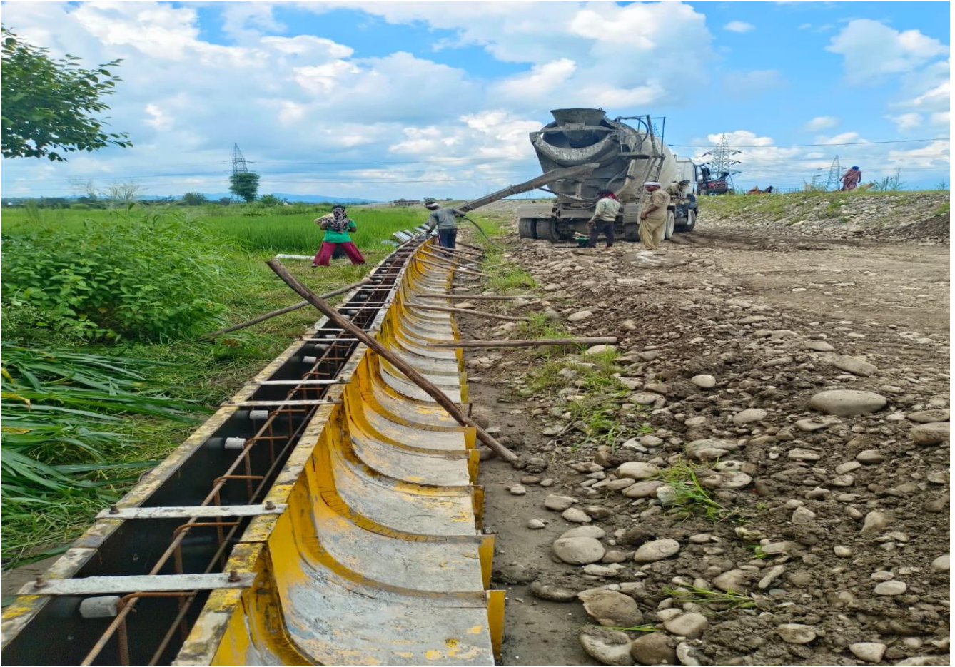
Boundary Wall Casting Work in Progress at Ch. 30+675 to 30+700 RHS
