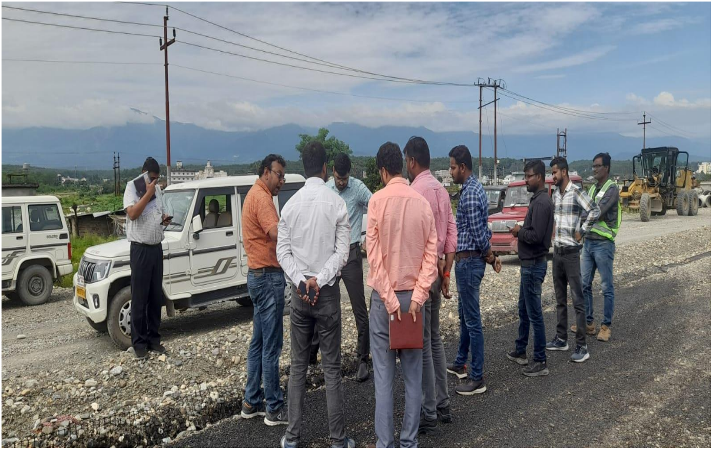
Manager Technical (NHAI) & IE Team Site Visit at Ch 38+200
