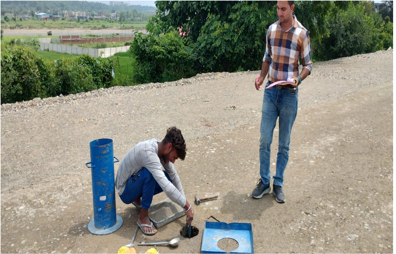
FDD Checking of WMM Top Layer at Ch-30+940 to 31+200 LHS
