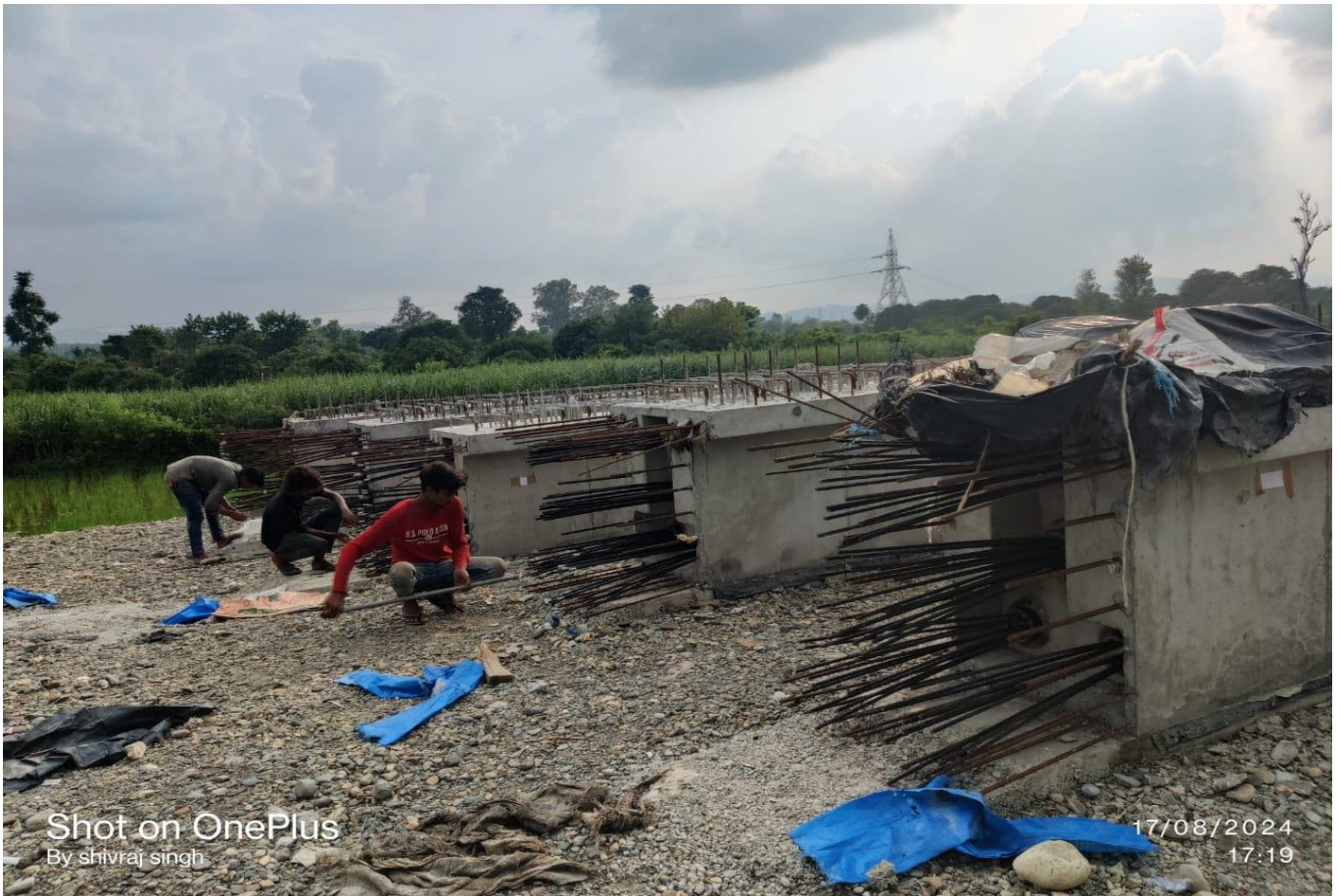
VUP PSC Girder Stressing Work in Progress at Ch. 22+598
