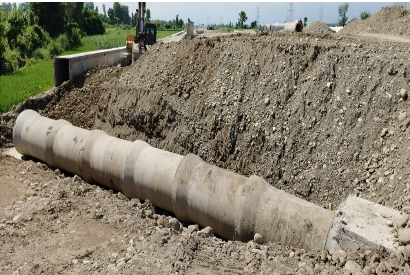
HPC Pipe Laying Work in Progress at Ch. 25+150 RHS
