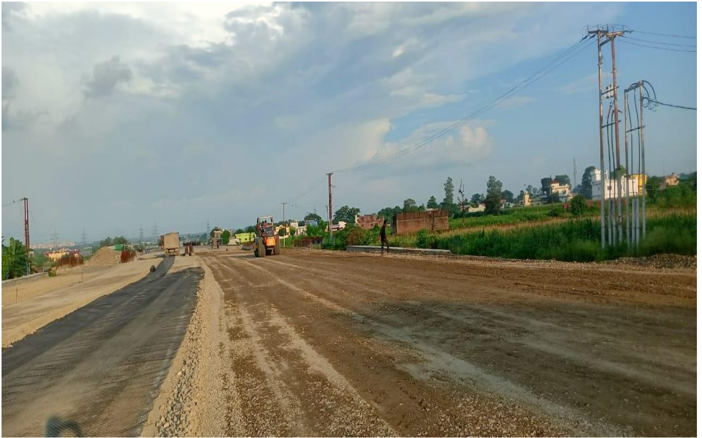
GSB Top Rolling Work in Progress at Ch. 29+020 to 29+160 RHS
