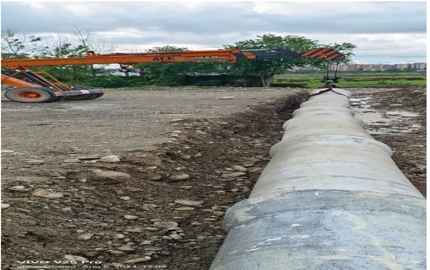
Utility Pipe Laying Work in Progress at Ch. 32+900
