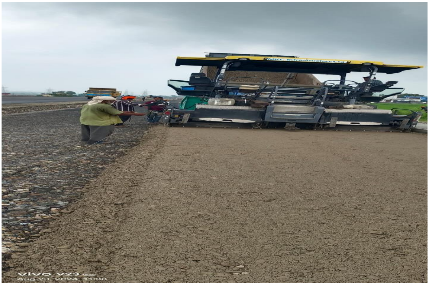
WMM Laying Work in Progress at Ch 29+220 (RHS) Service Road
