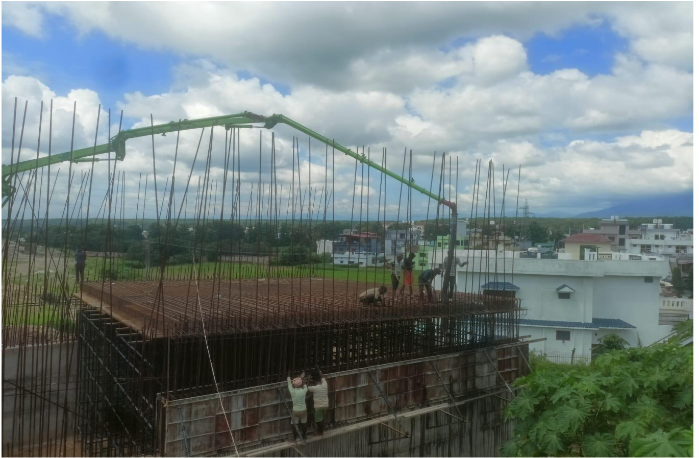
LVUP Wall 4th Lift Casting Work in Progress at Ch. 39+500
