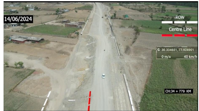
Ch. 34520 to 34770 LHS, MCW & Service Road Work
