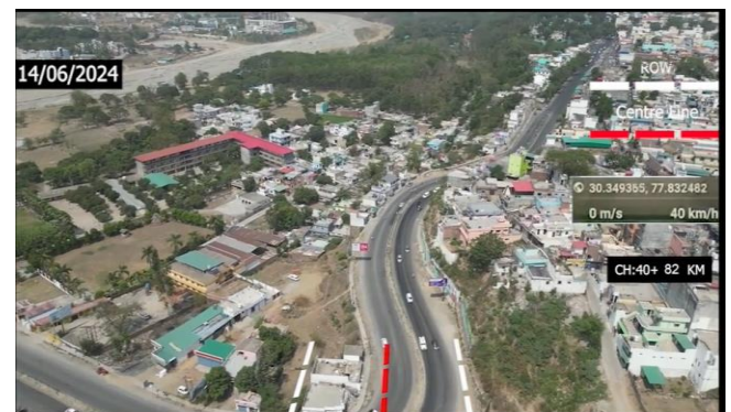
Ch. 40100 to 40350 LHS , Highway Work
