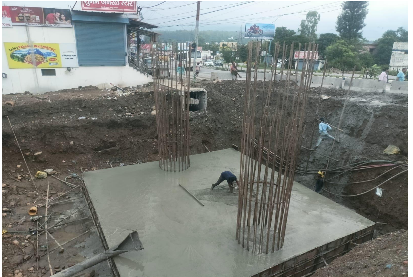
VUP P1 Foundation Casting Work in Progress at Ch 40+063
