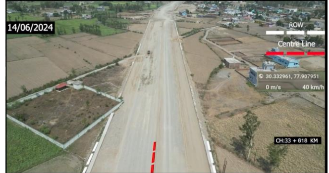
Ch. 33650 to 33680 LHS, Drain & Service Road Work
