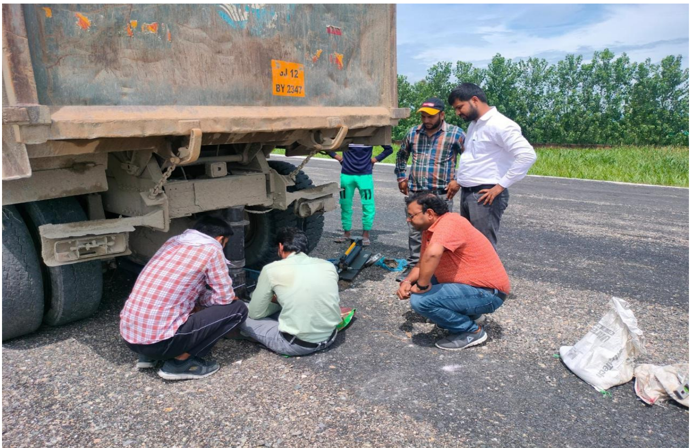
Plate Load Test Going on WMM Top at Ch. 24+090
