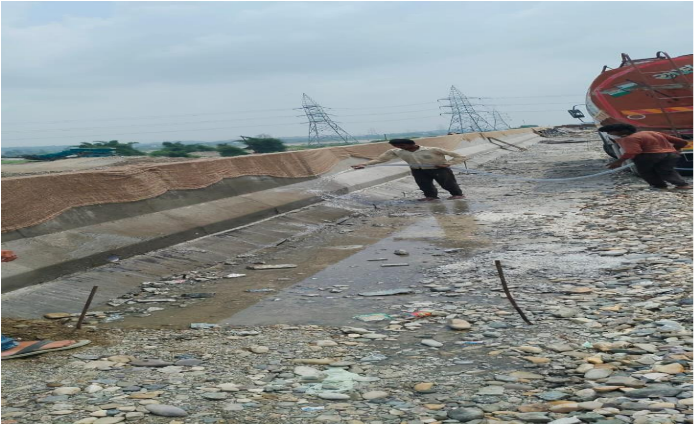
Friction Slab & Crash Barrier Curing Work in Progress at Ch. 30+250 LHS
