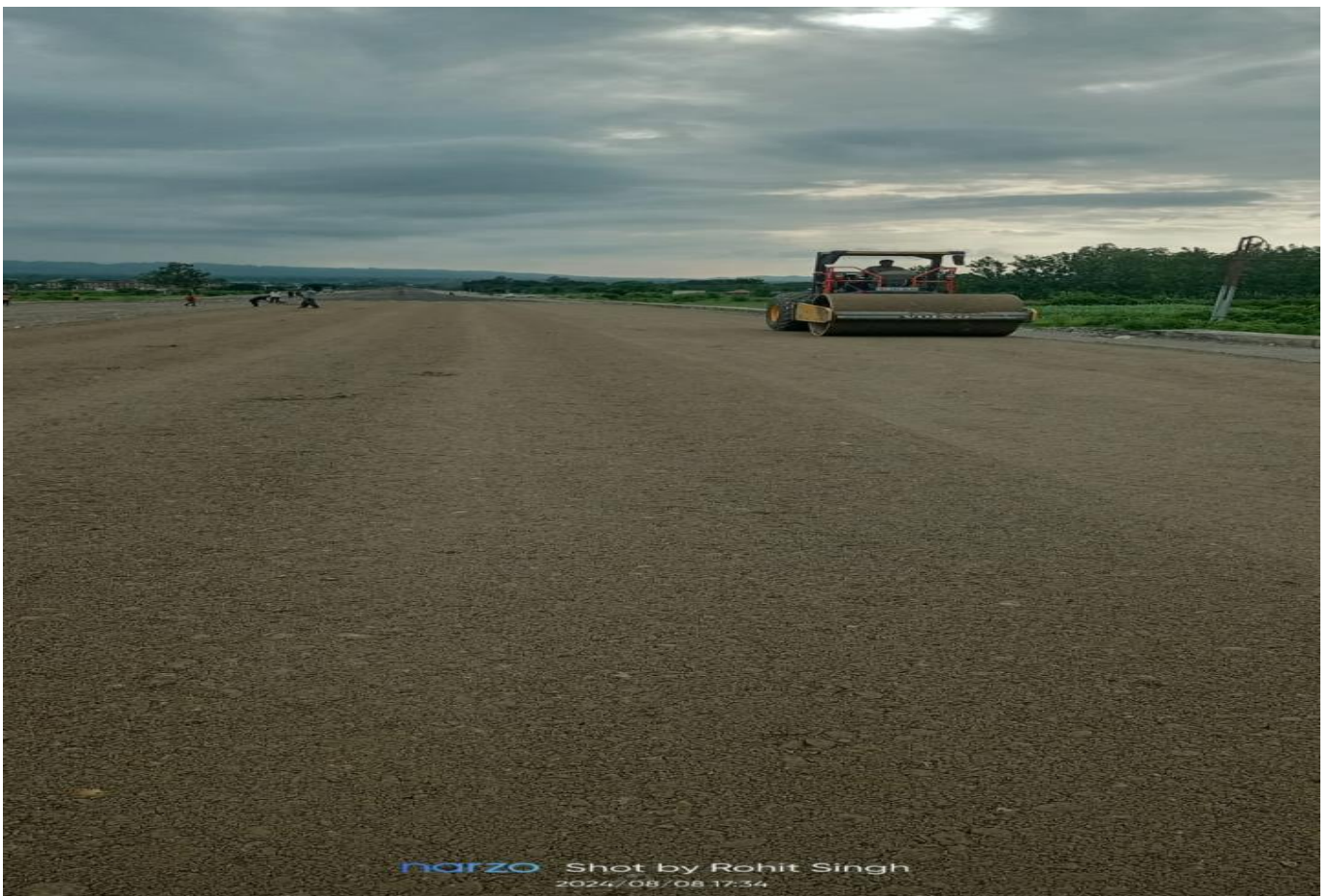
WMM Top Rolling Work in Progress at Ch 33+950 to 34+100 (LHS)
