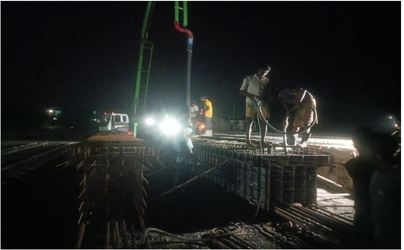
RCC Girder Casting Work in Progress of VUP Ch. 40+063
