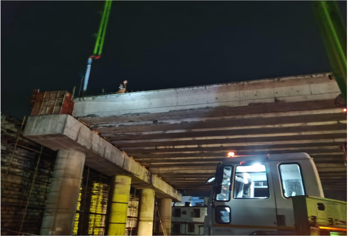
VUP End Cross Girder Casting Work in Progress at Ch. 31+678
