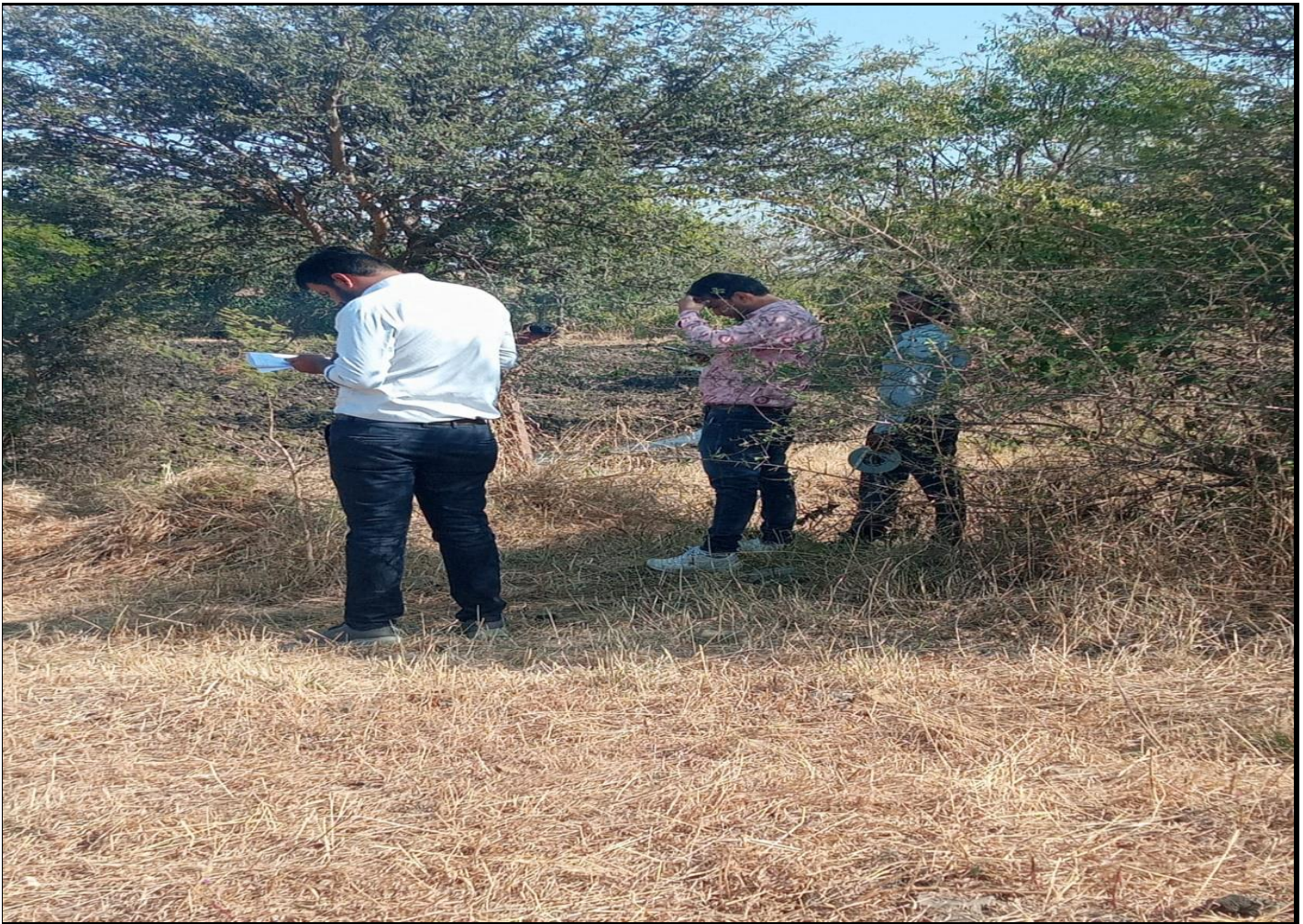
Toll Area ROW Marking at ch-112+800
