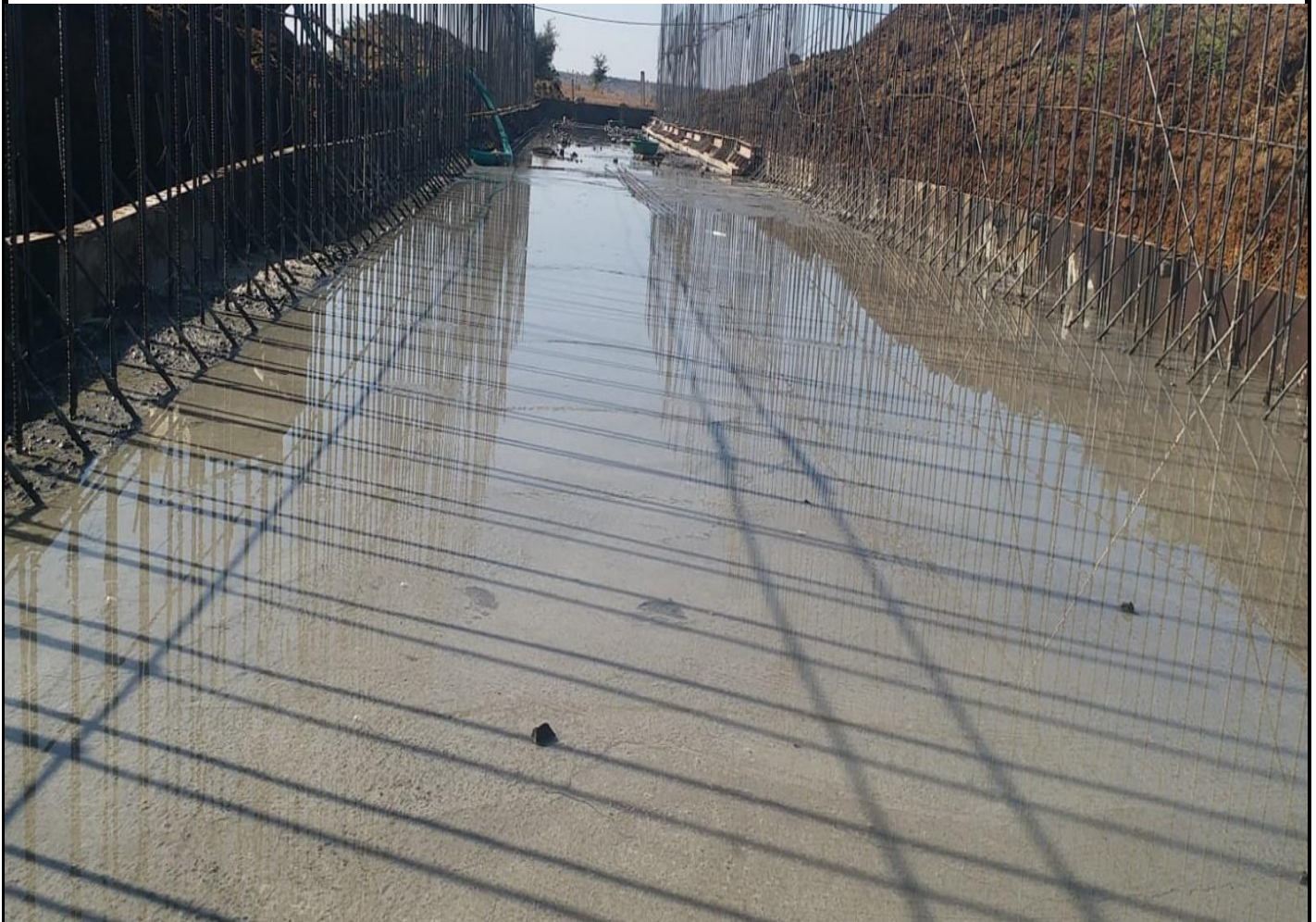
Curing of Bottom Slab
