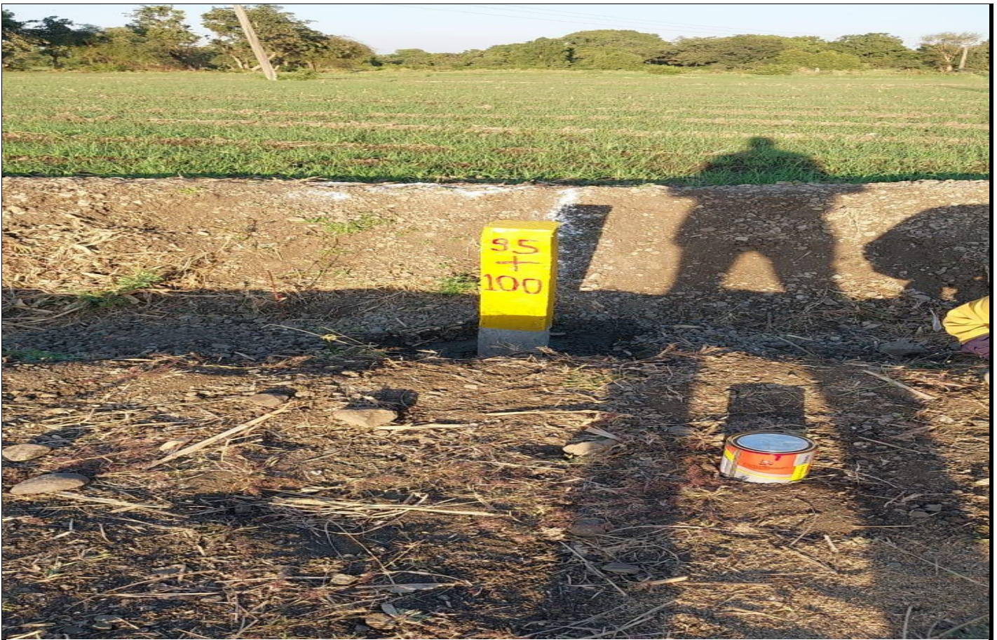
Chainage Pillar Erection
