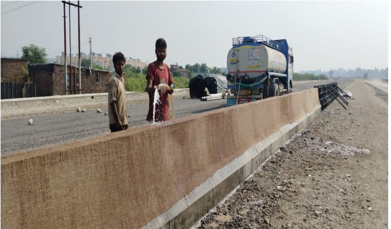
New Jercy Crash Barrier Curing Work in Progress at Ch. 35+400
