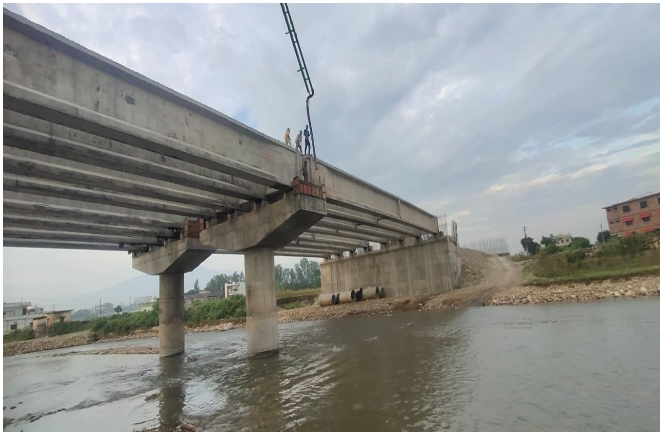
MJB Seismic Restrainer Casting Work in Progress at Ch. 33+033
