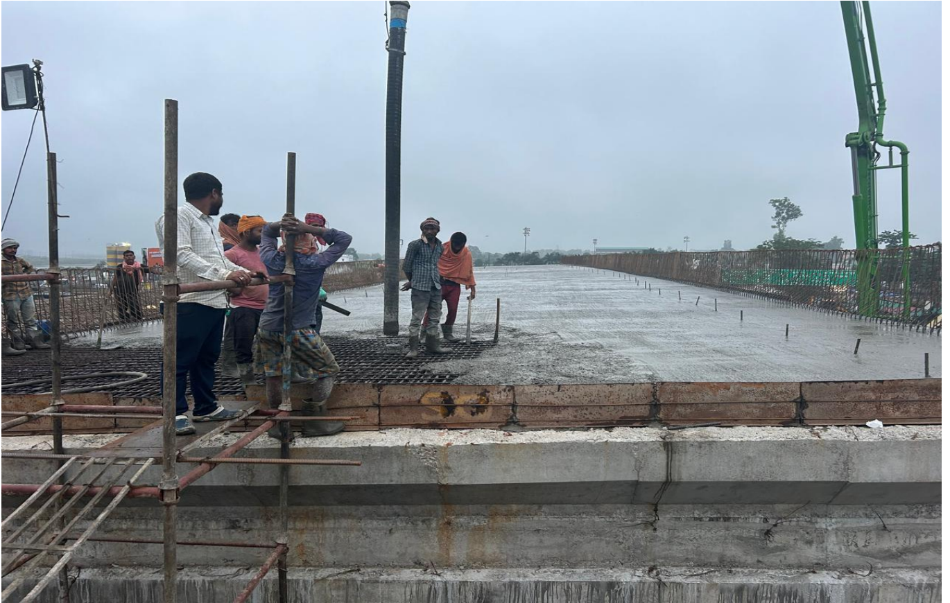
VUP Deck Slab Casting Work in Progress at Ch. 31+678 RHS
