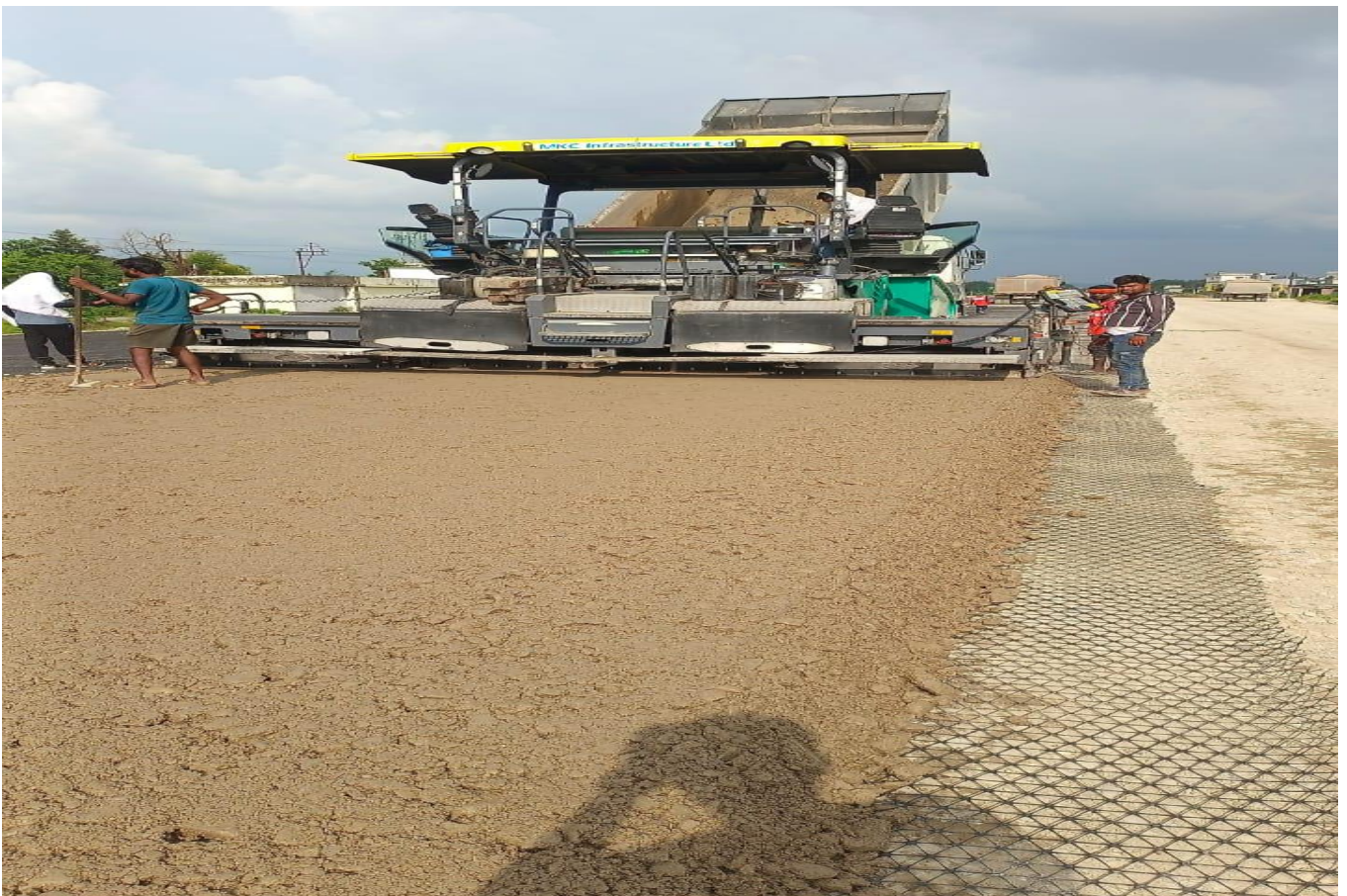
WMM Laying Work in Progress at Ch 36+300 (RHS)
