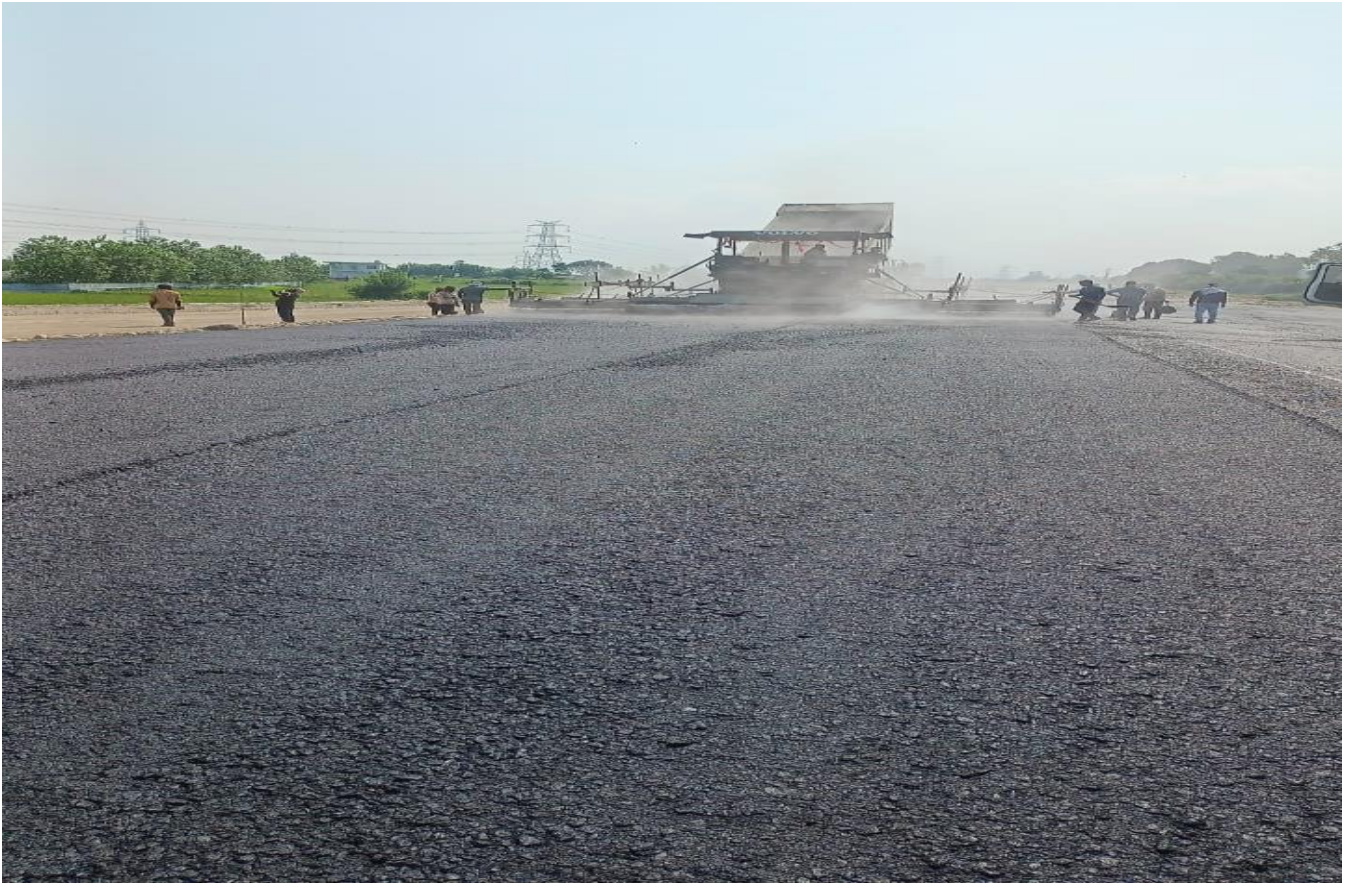
DBM Laying Work in Progress at Ch -24+900
