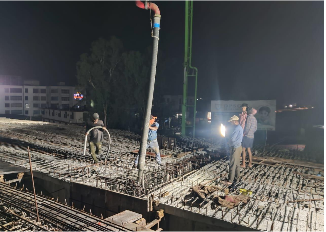
VUP End Cross Girder Casting Work in Progress at Ch. 31+678
