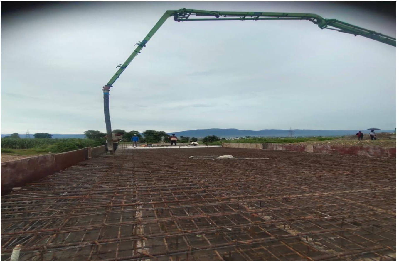
Box Culvert Slab Casting Work in Progress at Ch. 27+400 RHS
