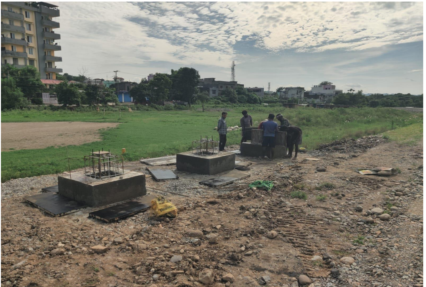
Bus Shelter Foundation Casting Work in Progress at Ch 38+450
