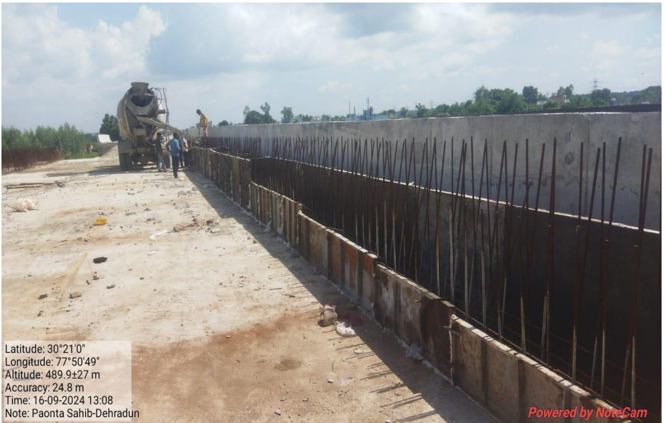
MNB Crash Barrier Kerb Casting Work in Progress at Ch. 28+222
