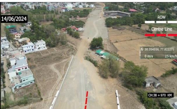
Ch. 39000 to 39120 BHS, Highway Work
