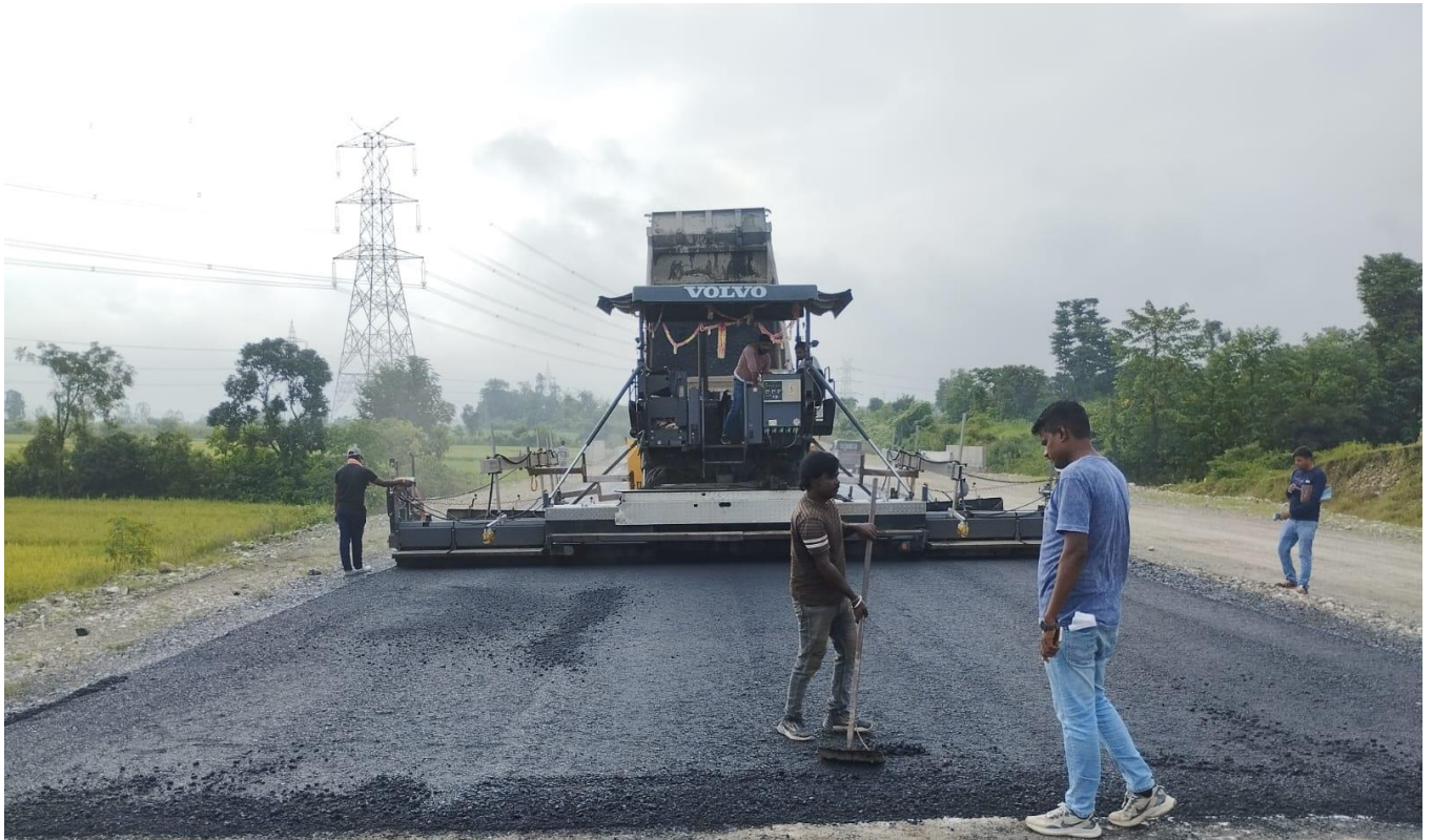
DBM Laying Work in Progress at Ch - 25+740 to 25+950 LHS
