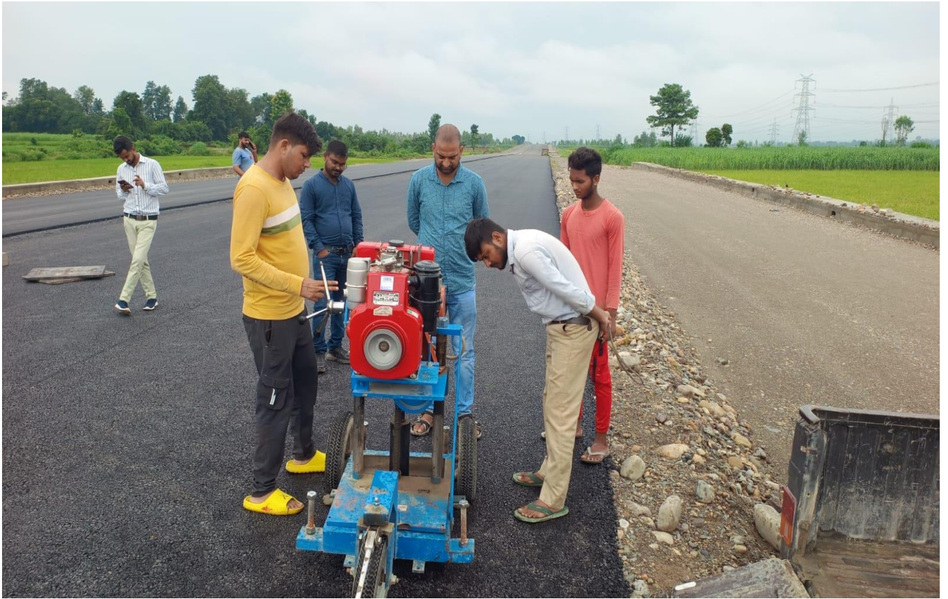
DBM Core Cutting & Thickness Checking by IE Staff at Ch 24+800 LHS
