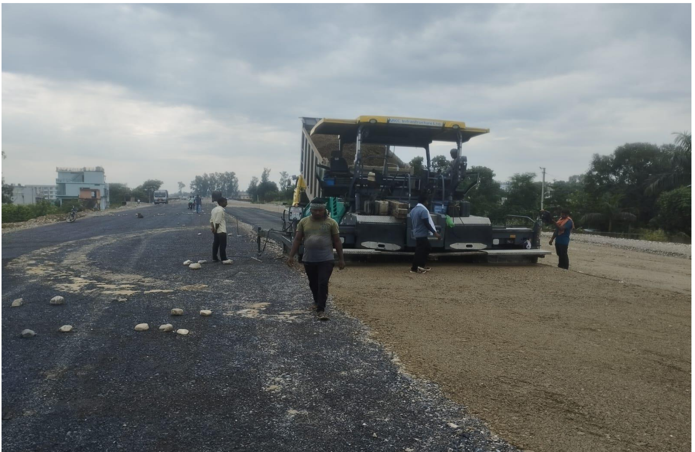
WMM Laying Work in Progress at Ch 31+020 to 31+200 (RHS)
