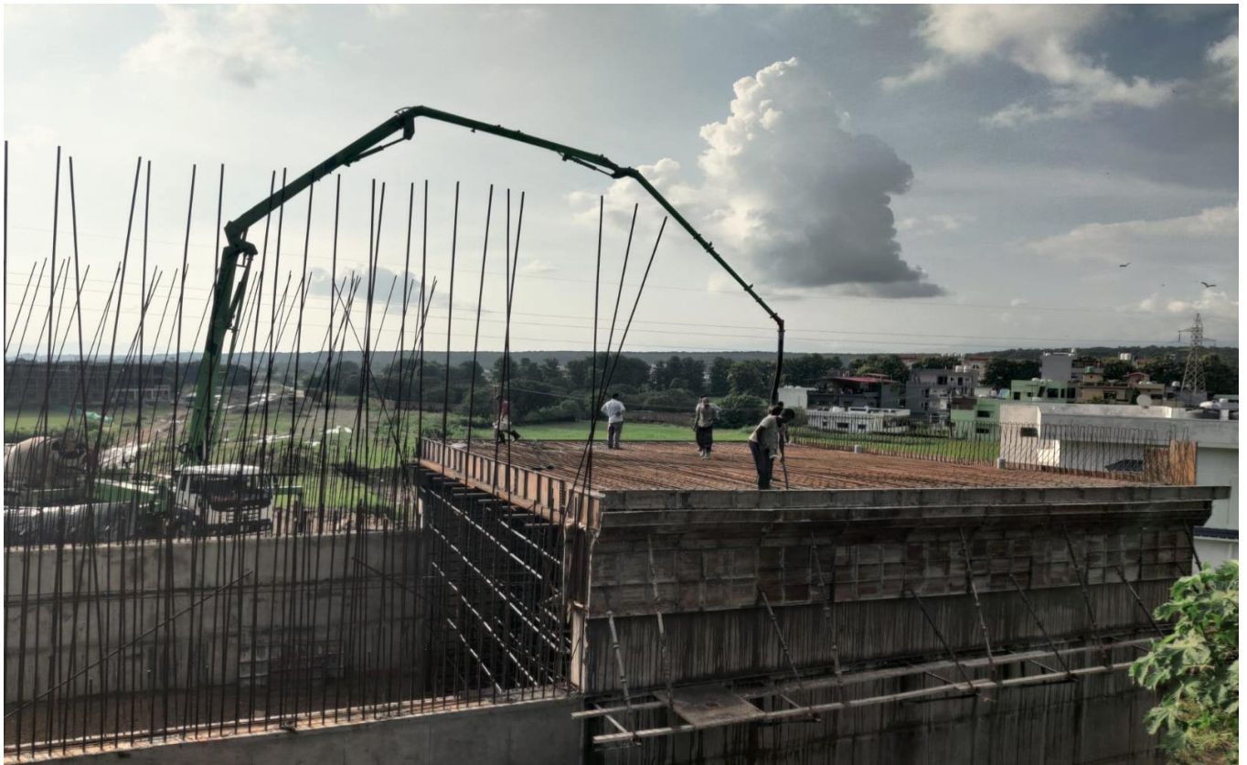
LVUP Slab Casting Work in Progress at Ch. 39+500 LHS
