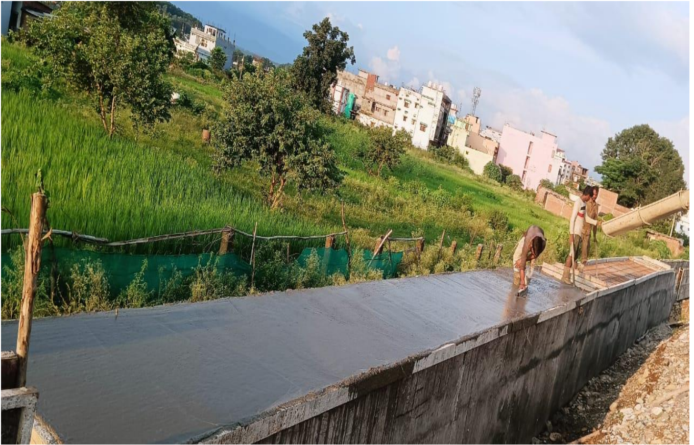
Drain Slab Casting Work in Progress at Ch. 38+870 LHS
