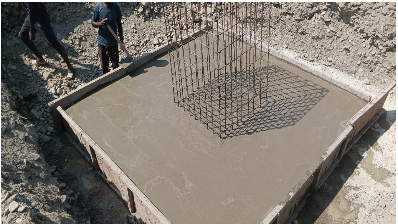
High Mast Foundation Raft Casting Work in Progress at Ch. 38+338
