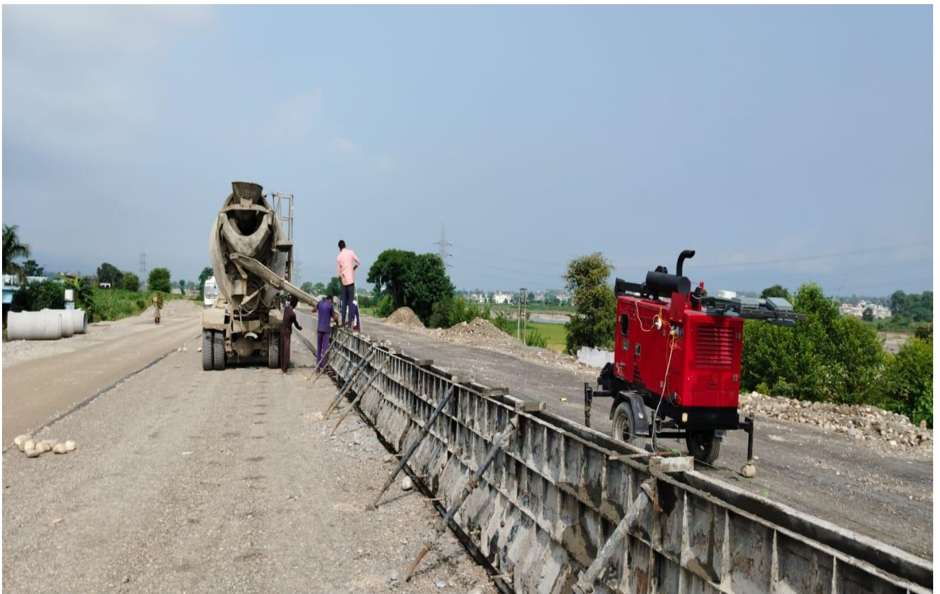
NJCB Casting Work in Progress at CH 31+190
