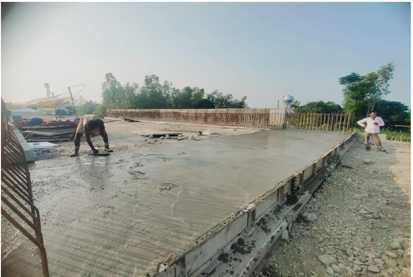
Approach Slab Casting Work in Progress at Ch. 19+297
