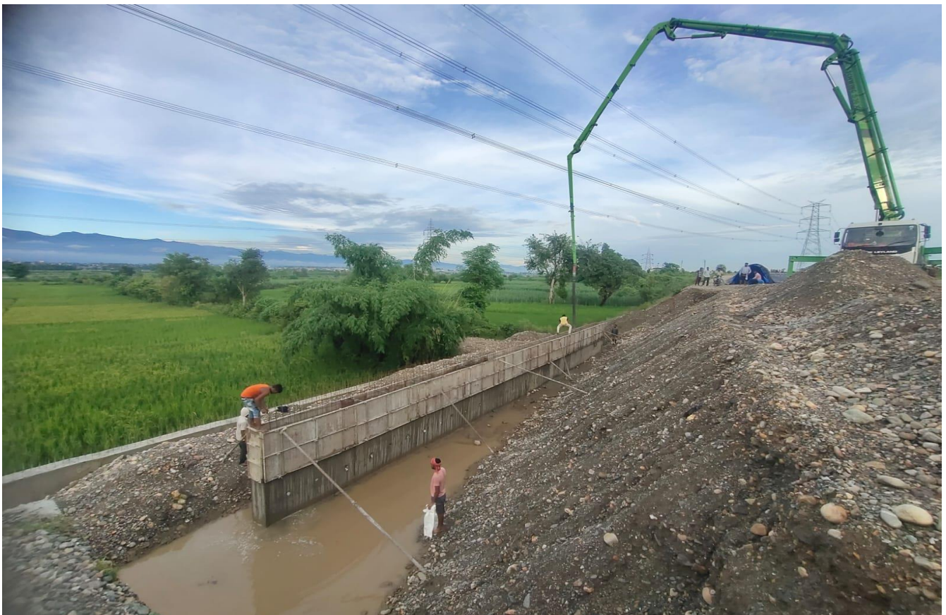
Toe Wall 2nd Lift Pouring Work in Progress at Ch. 25+980 LHS
