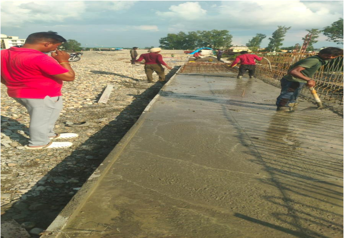
Friction Slab Casting Work in Progress at Ch. 31+333 RHS
