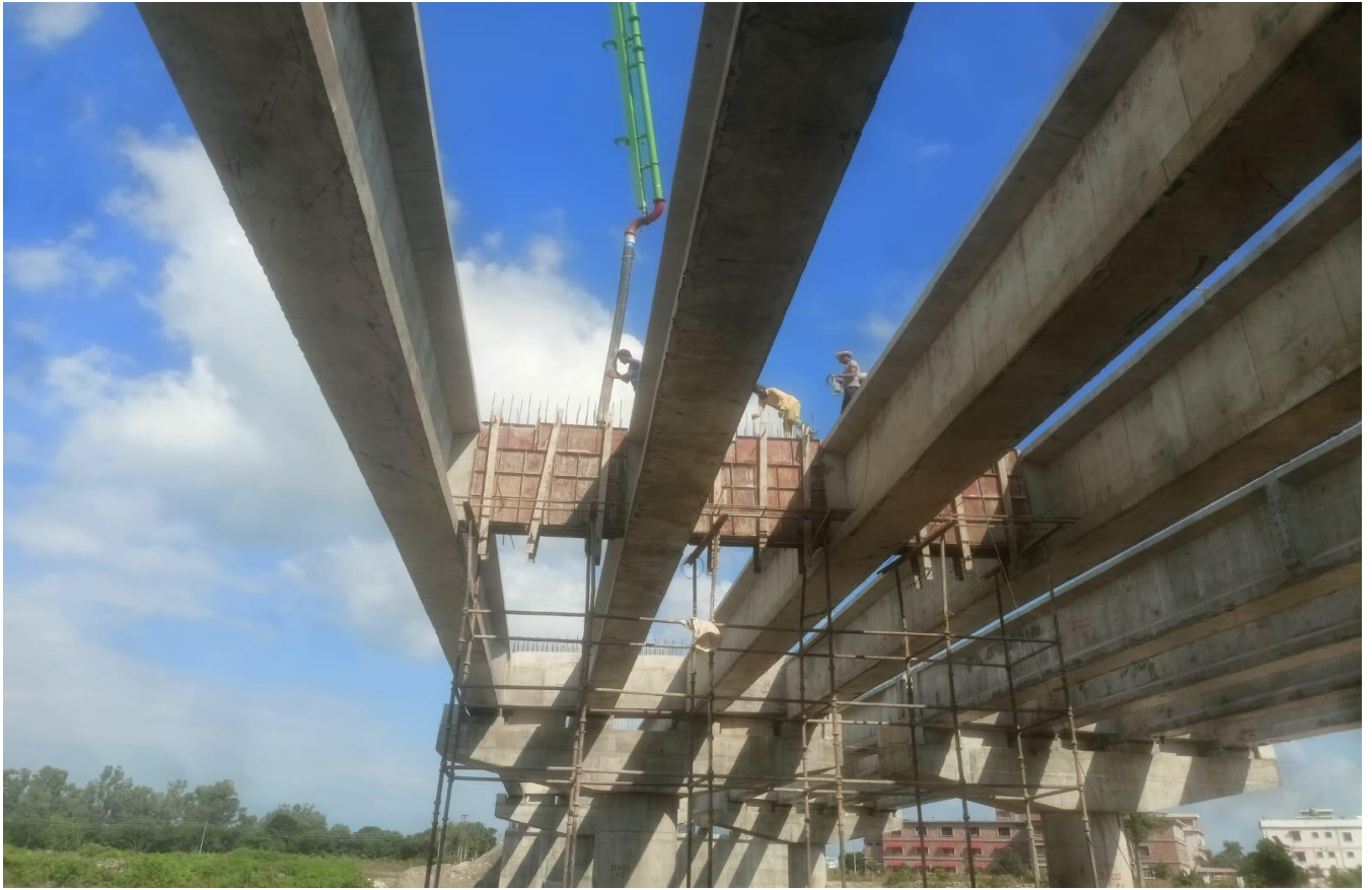
MJB Intermediate Cross Girder Casting Work in Progress at Ch. 33+033 LHS
