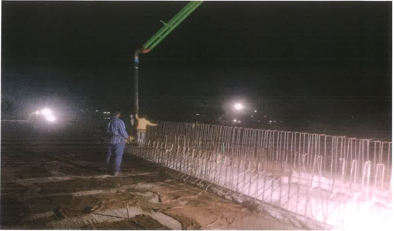
Ch 33+033 MJB RHS parapet footpath kerb casting work in progress
