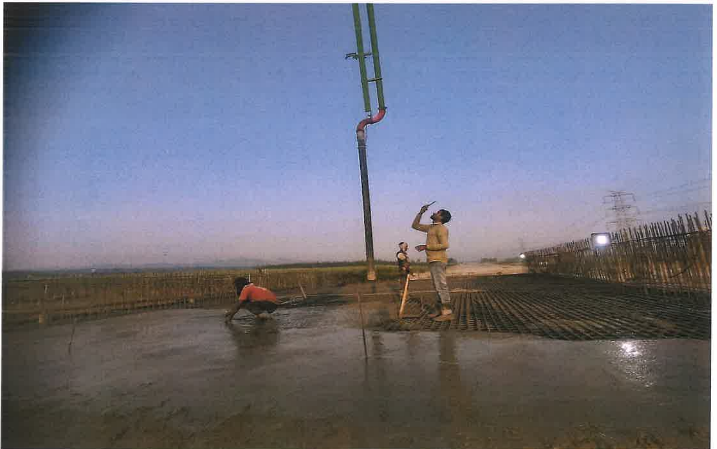
21+610 Slab casting work in progress
