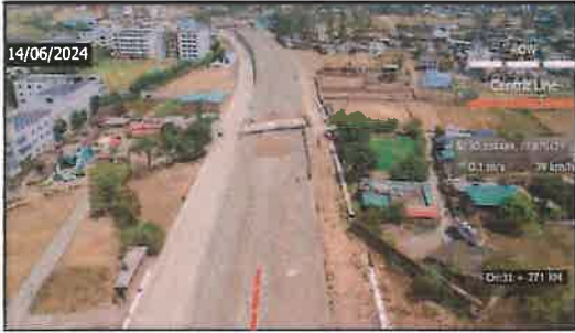
Ch. 31280 to 31300 RHS, Drain & Service Road Work
