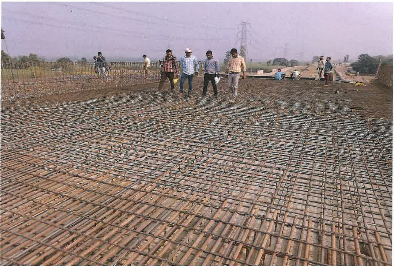
22+598 VUP Deck slab reinforcement binding checking by ABE Sir
