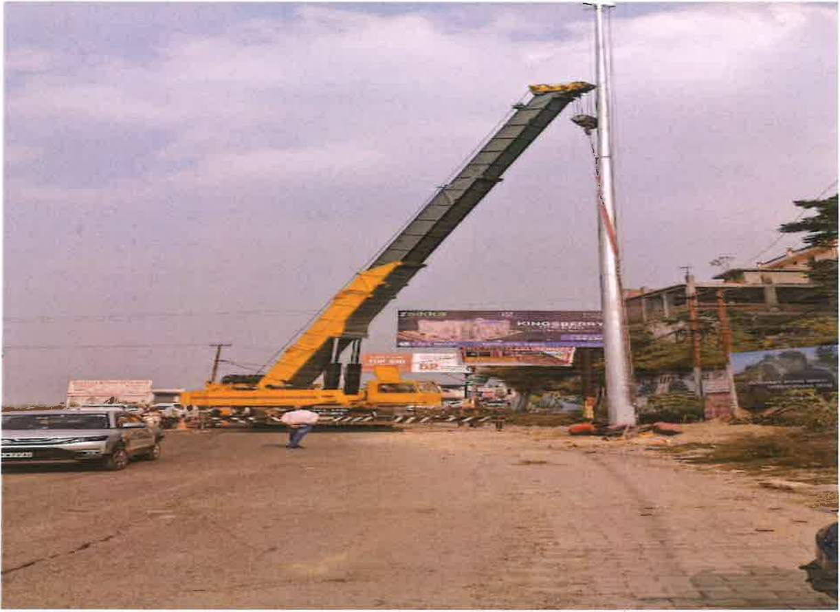
HIGH MAST POLE INSTALLATION WORK IN PROGRESS AT 40+115
