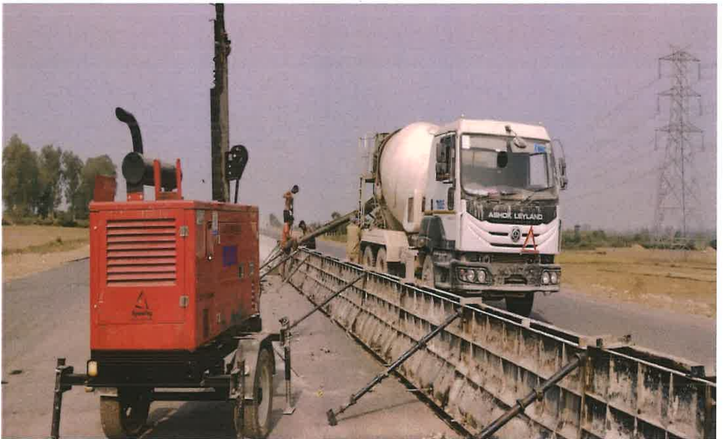
Filter media pouring at Ch 39+500 RE wall A1 side LHS
