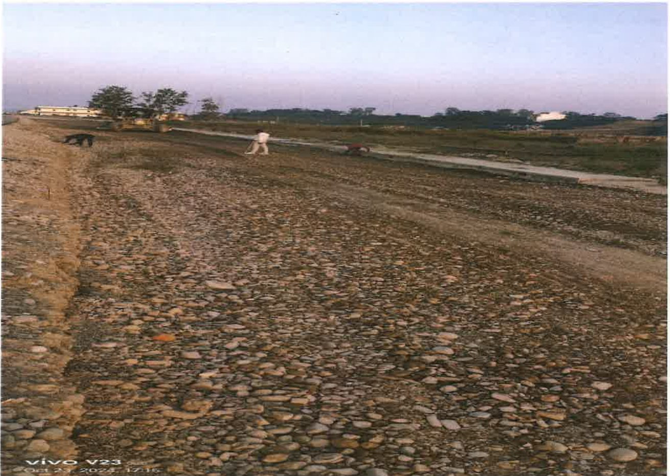
Service Road Gsb preparation in progress at ch35+700 To Ch36+000 (RHS)
