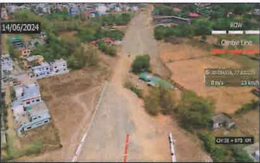
Ch. 39000 to 39120 BHS, Highway Work
