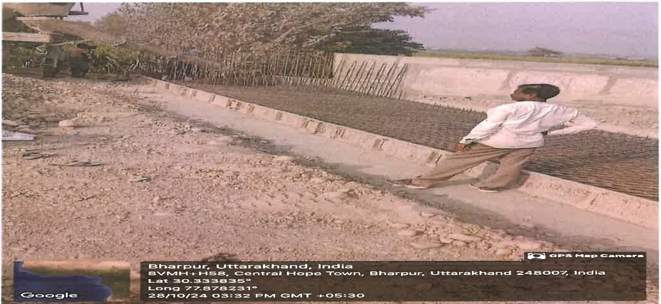
20+820 MNB approach slab casting work in progress LHS
