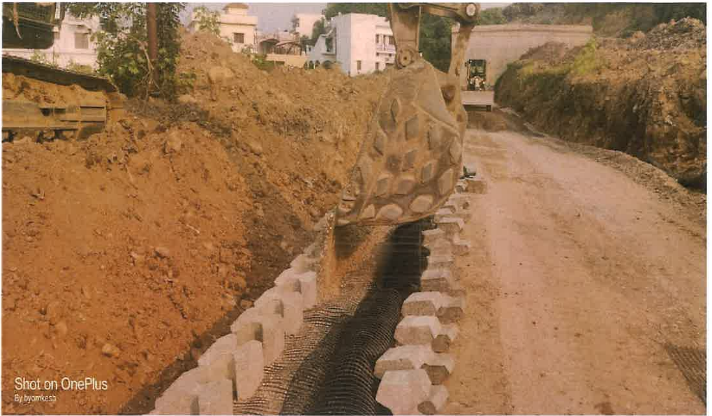
Filter media pouring at Ch 39+500 RE wall A1 side LHS
