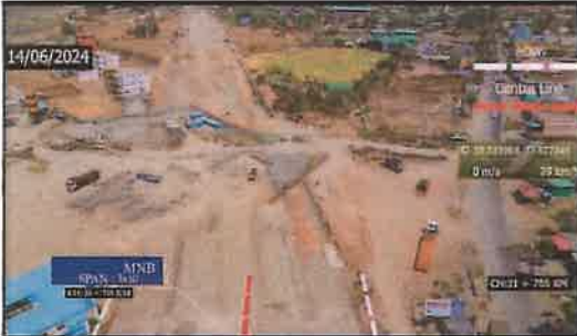
Ch. 31770 to 31850 BHS, Highway Work
