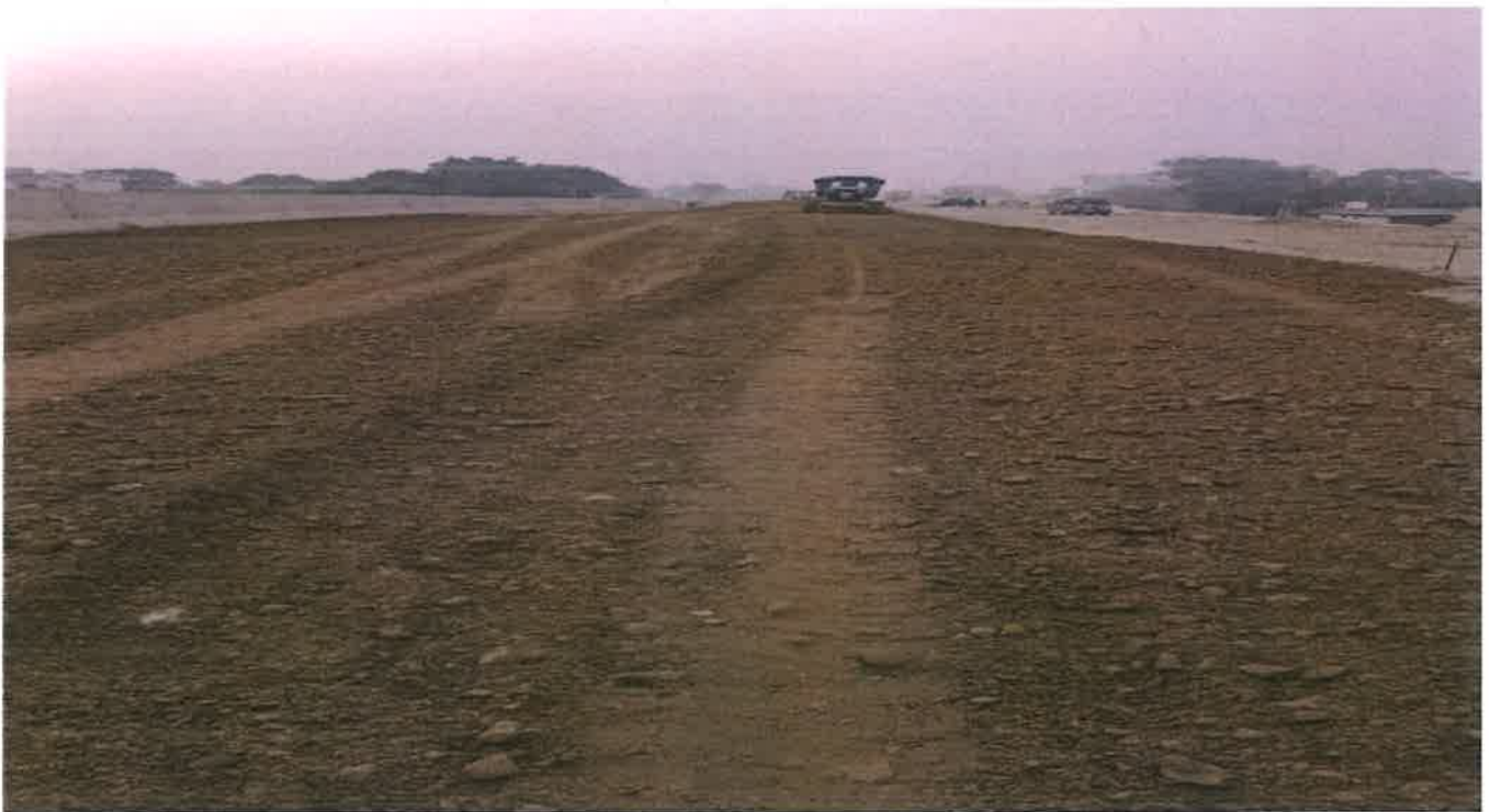
Wmm preparation in progress at ch 31+400
