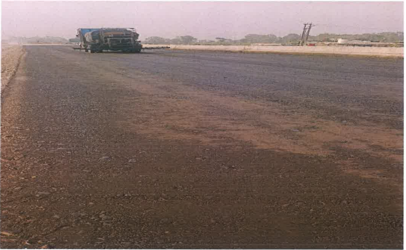
Prime coat spray work in progress at ch34+900 To Ch35+700(RHS)
