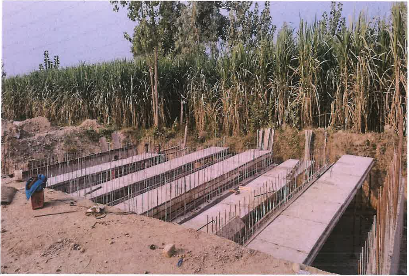
22+554 Box Culvert SR slab staging work in progress.
