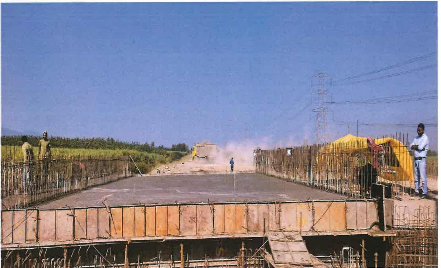
21+610 solid slab casting completed.
