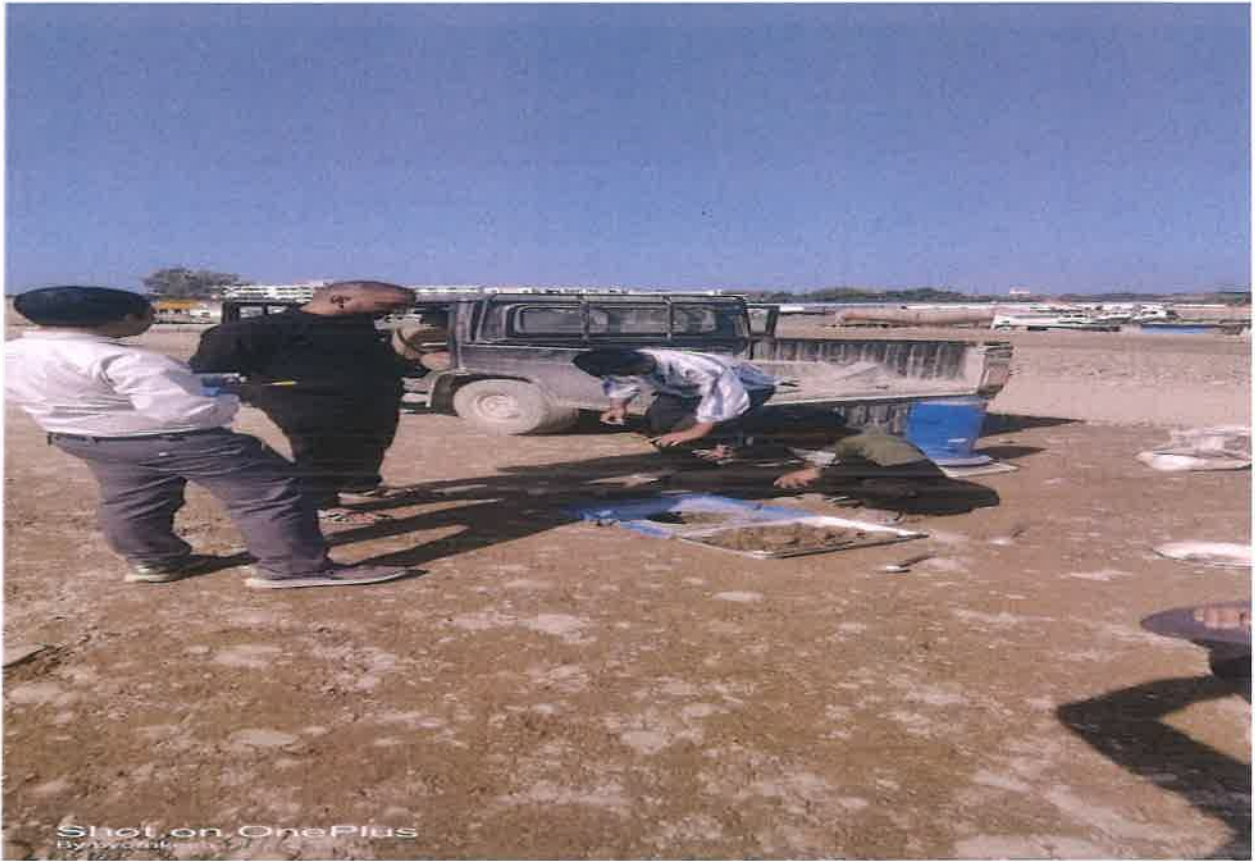
RE wall FDD checking by AQME sir at 31+800 A2 side BHS
