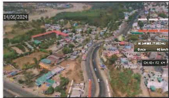
Ch. 40100 to 40350 LHS, Highway Work
