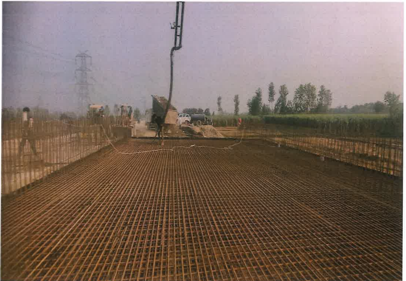
21+610 MNB RHS Solid slab casting work in progress
