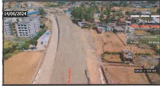
Ch. 31400 to 31480 RHS, Drain & Service Road Work
