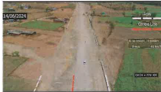
Ch. 34520 to 34770 LHS, MCW & Service Road Work
