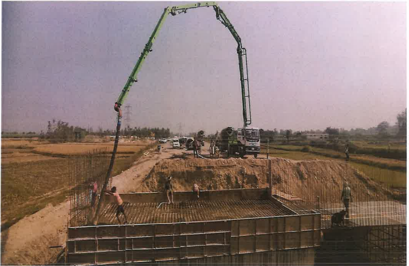
Box culvert slab casting work in progress at Ch 19+890 LHS
