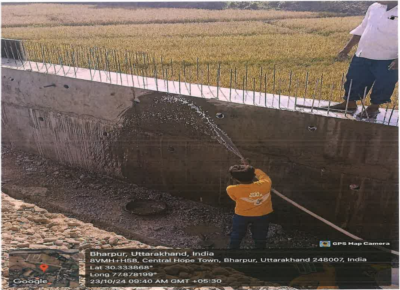
Retaining wall curing work in progress at Ch 32+390 RHS
