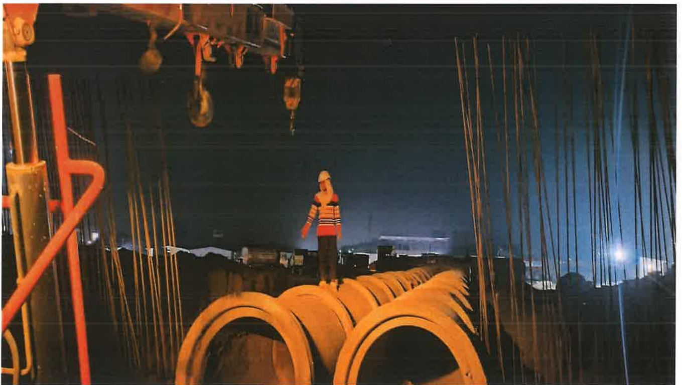
HPC pipe laying at ch 31+830
