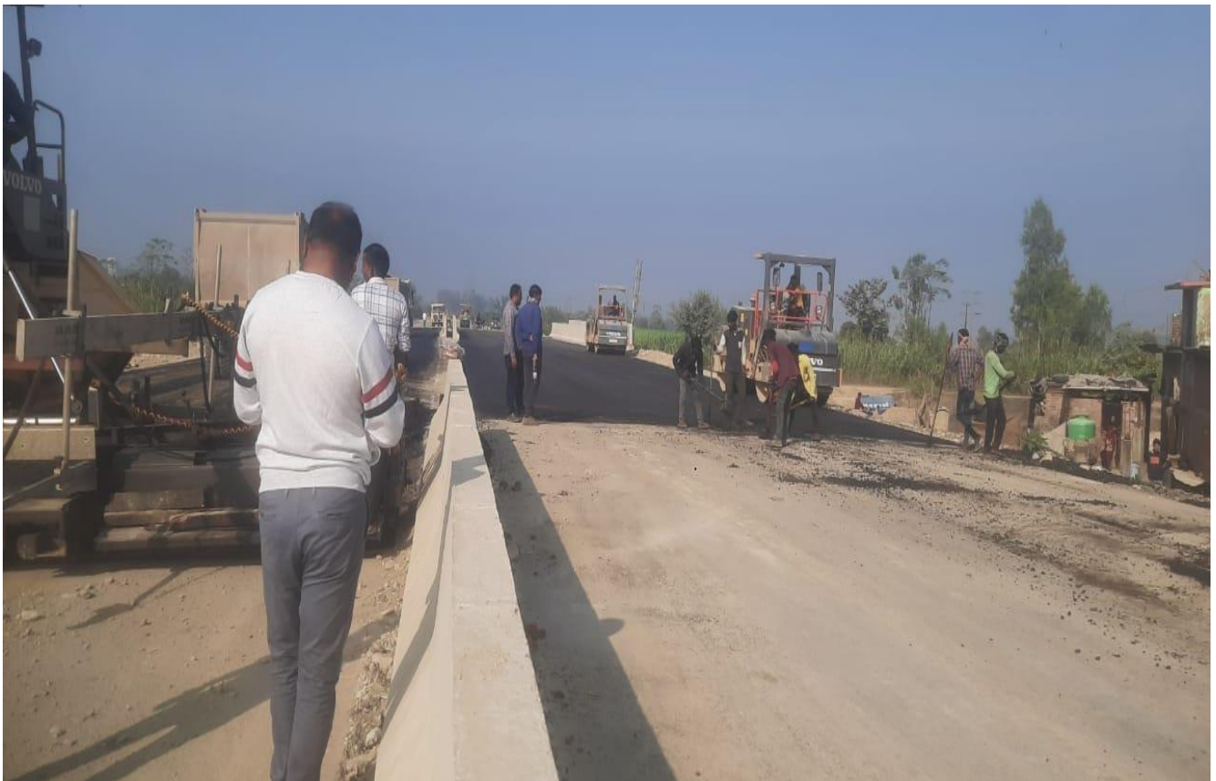
DBM Laying Work in Progress at Ch.27+680 to 27+820 BHS
