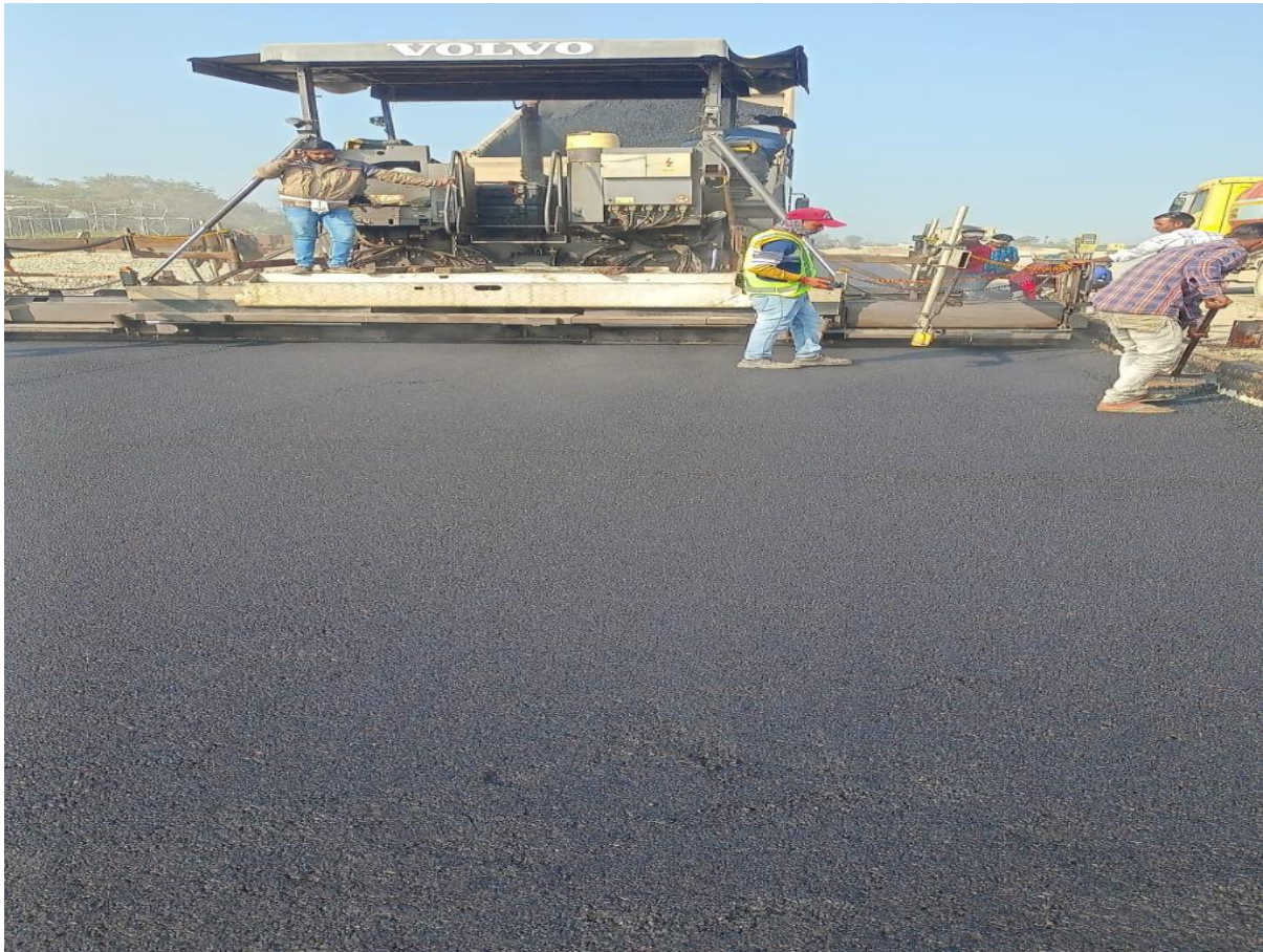
Service Road BC Laying Work in Progress at Ch. 29+800 RHS
