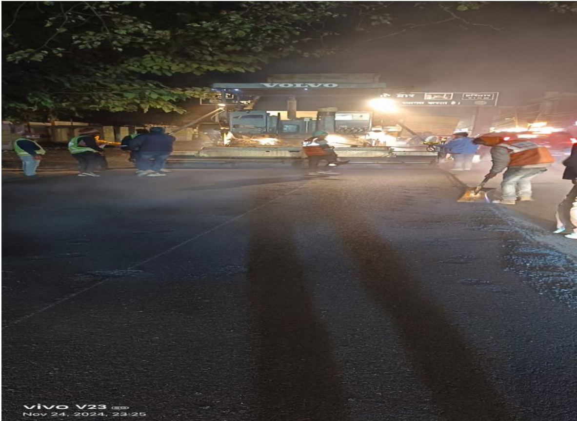
BC Laying Work in Progress at Ch.40+750
