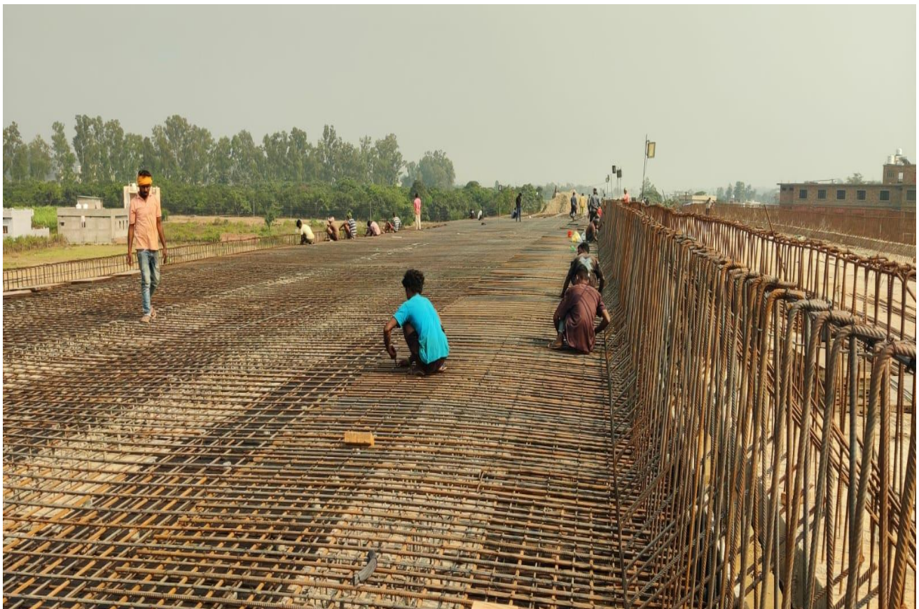
MJB Deck Slab Reinforcement Work in Progress at Ch-33+033(LHS)
