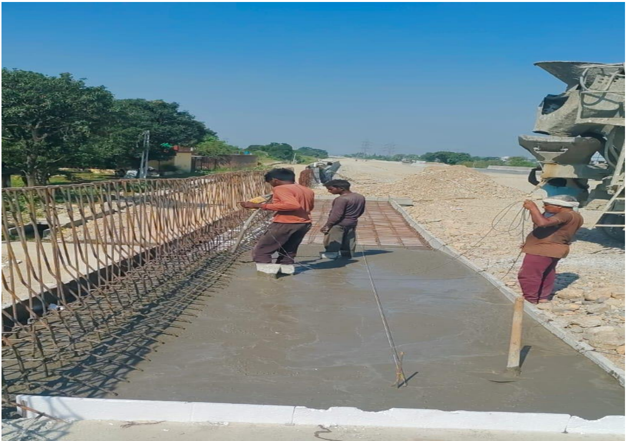
Friction Slab Casting Work in Progress at Ch. 31+370 RHS
