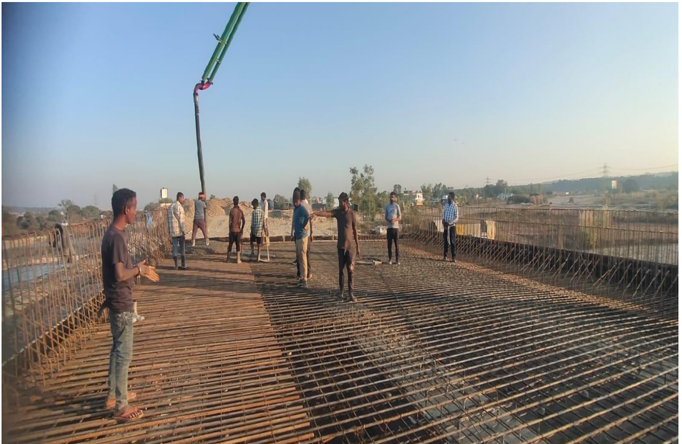
MNB Slab Casting Work in Progress at Ch. 28+122
