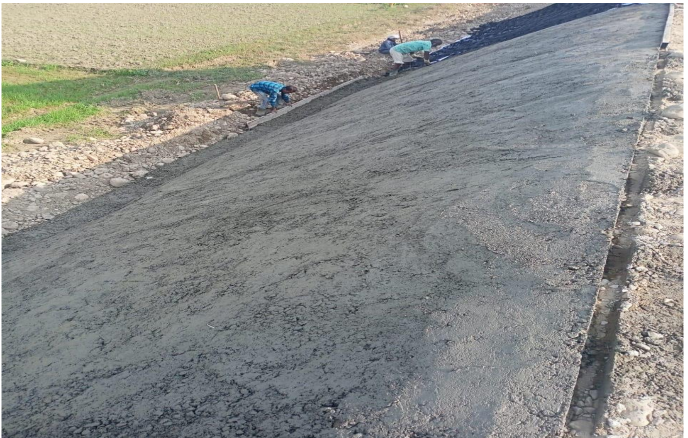
Slope Protection Work in Progress at Ch. 25+850 to 25+880 LHS
