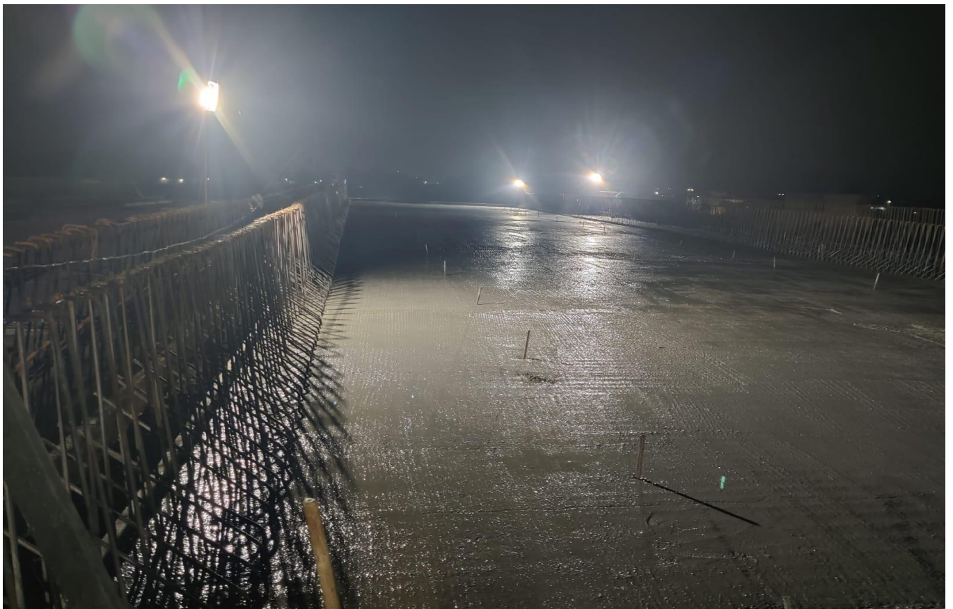
MJB Slab Casting Work is Completed at Ch. 33+033 LHS
