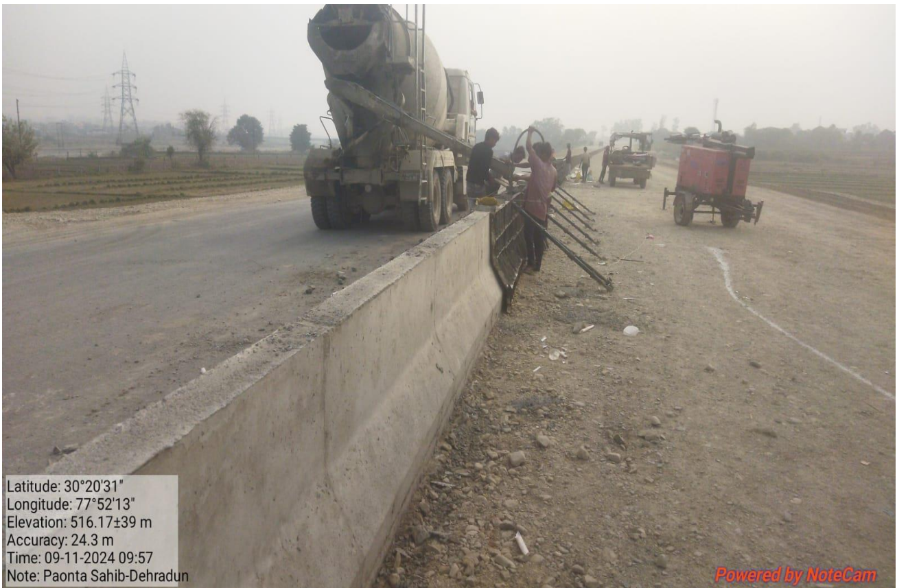
NJCB Casting Work in Progress at Ch. 30+705 to 30+716
