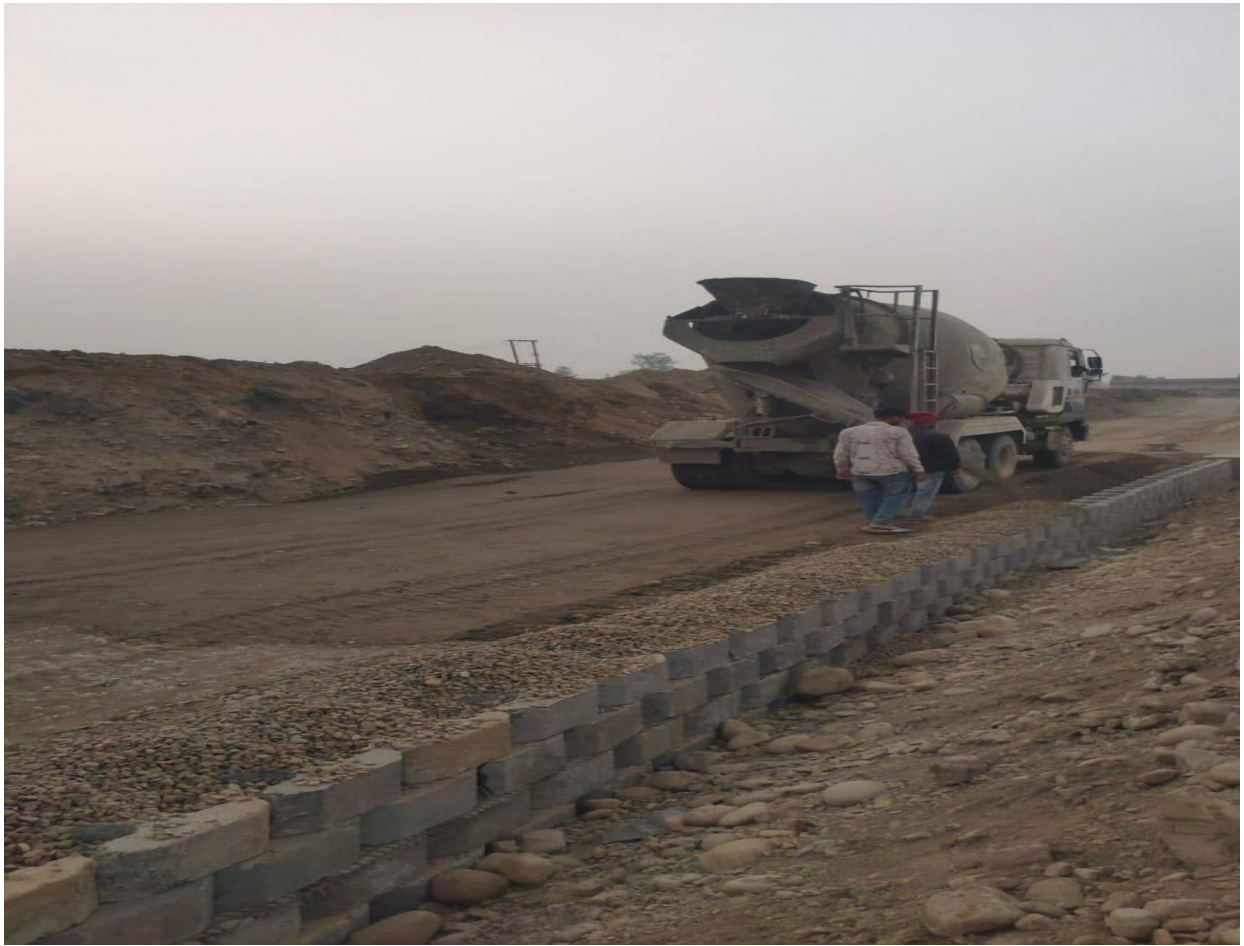
RE Wall Filter Media Pouring Work In Progress at Ch 22+750 LHS
