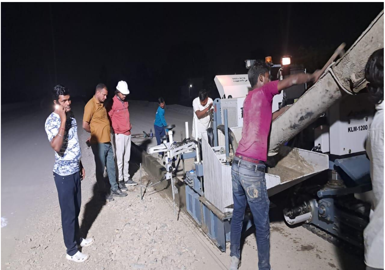
Kerb Laying Work in Progress at Ch. 32+020 to 32+280 RHS Service Road
