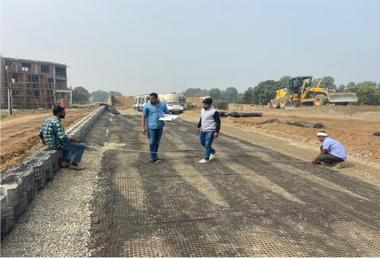
RE Wall Geo Grid Lenth Check by SPS Sir at Ch. 39+500
