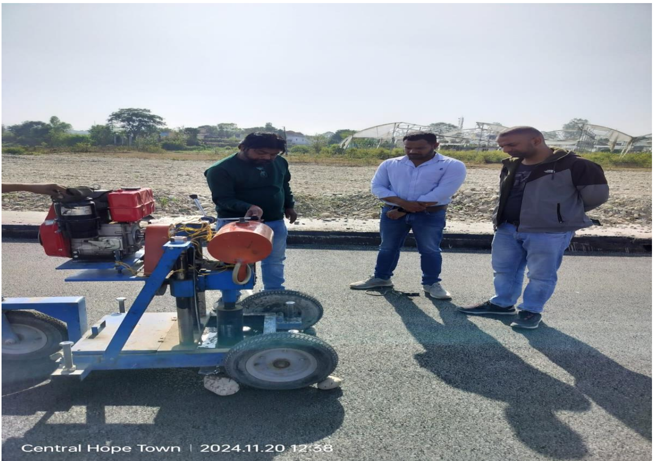
BC Core Cutting with SPS & AQME Sir at Ch. 29+800
