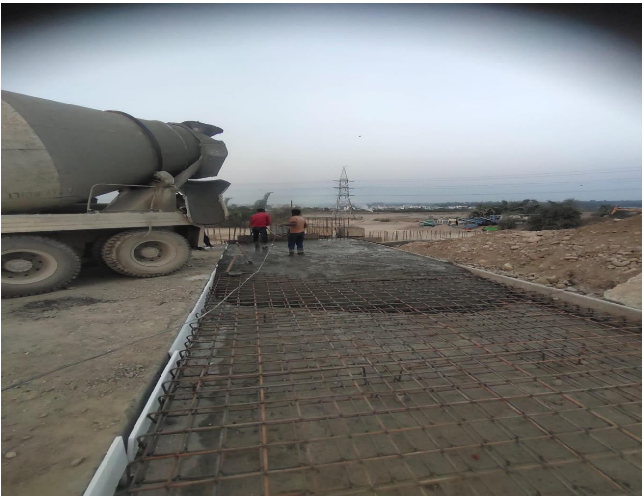
Approach Slab Casting Work in Progress at Ch. 30+259 A2 LHS
