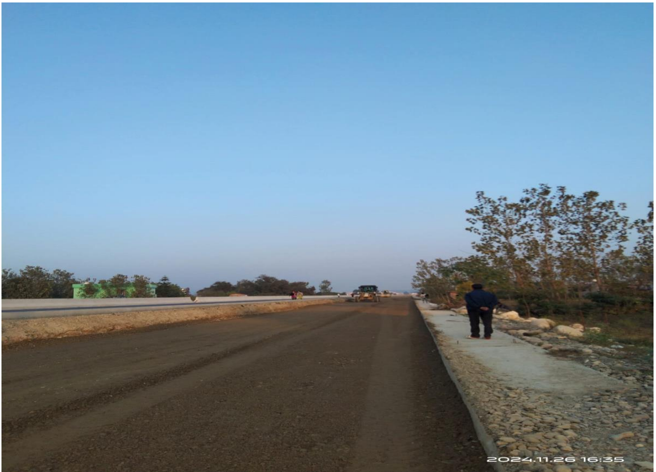
Service Road WMM Rolling Work in Progress at Ch. 36+920 to 37+060
