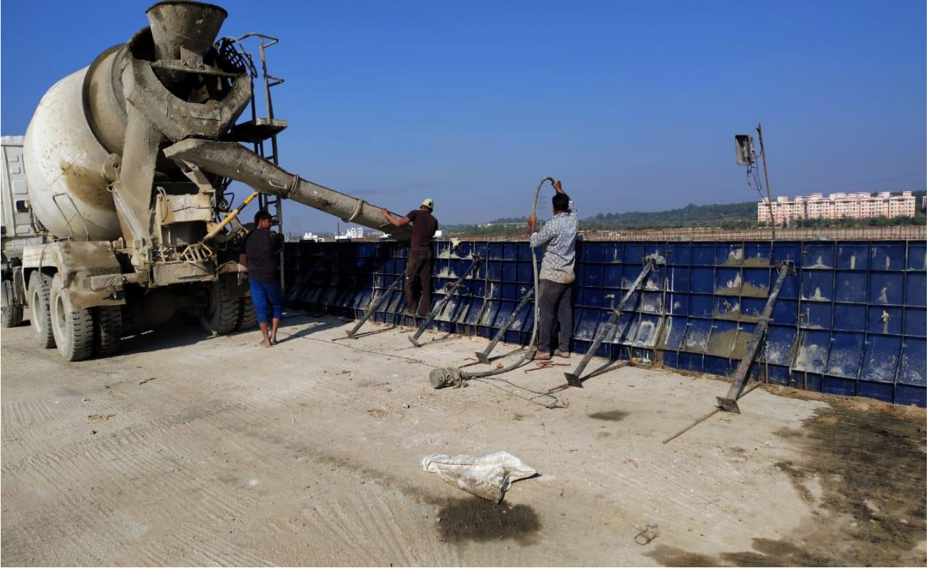
MJB Crash Barrier Casting Work in Progress at Ch. 33+033
