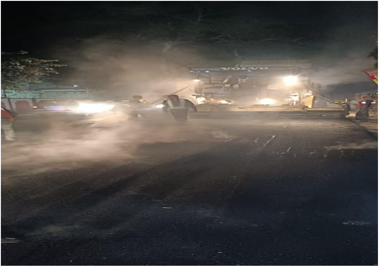
BC Laying Work in Progress at Ch.41+880
