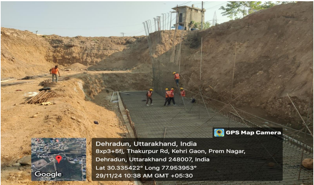
Retaining Wall Reinforcement Work in Progress at Ch. 39+780 to 39+800 RHS
