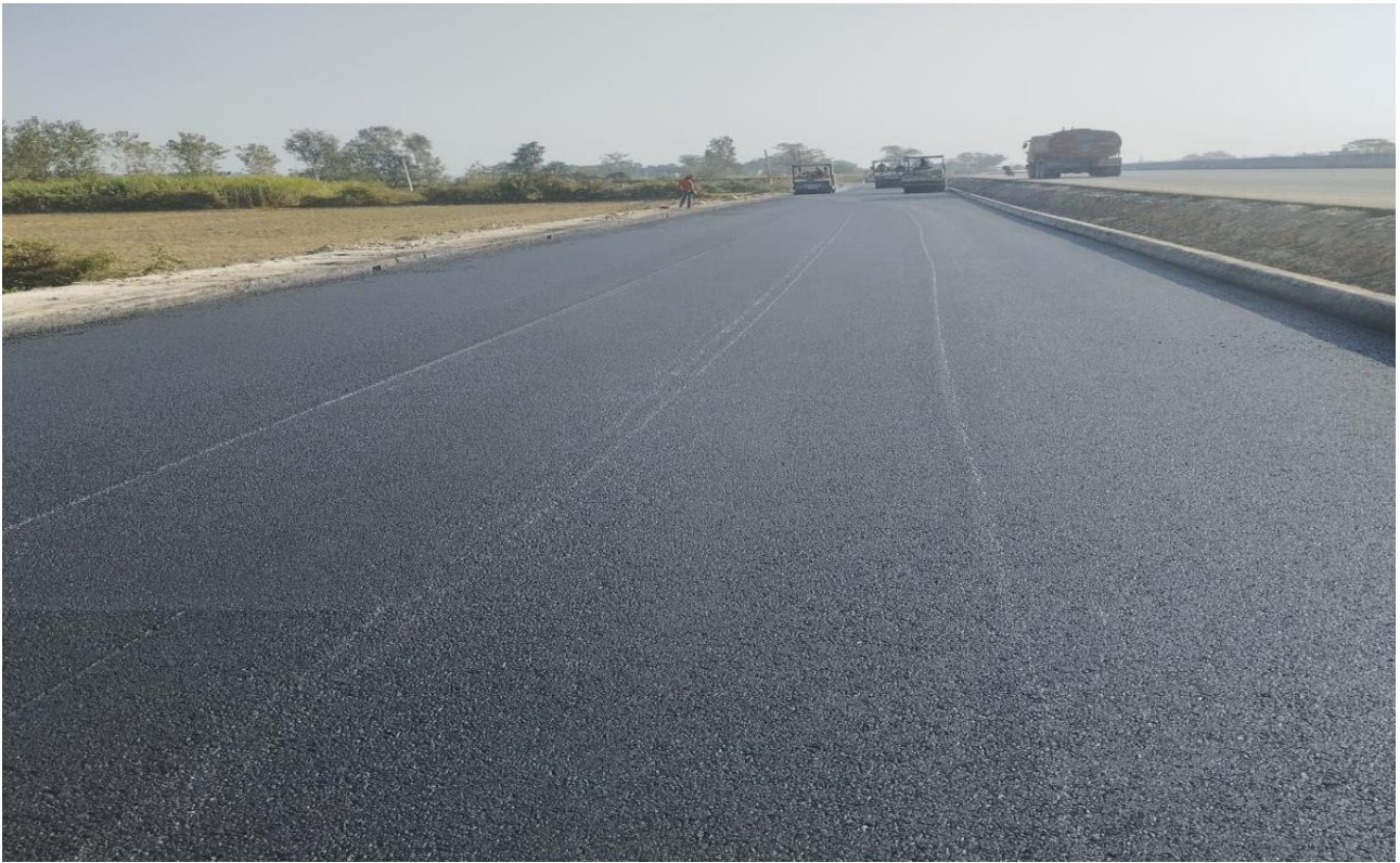
Service Road BC Laying Work in Progress at Ch. 33+320 to 34+040 LHS
