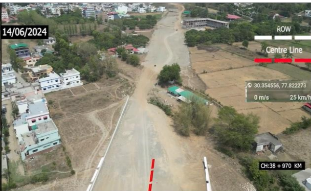
Ch. 39000 to 39120 BHS, Highway Work
