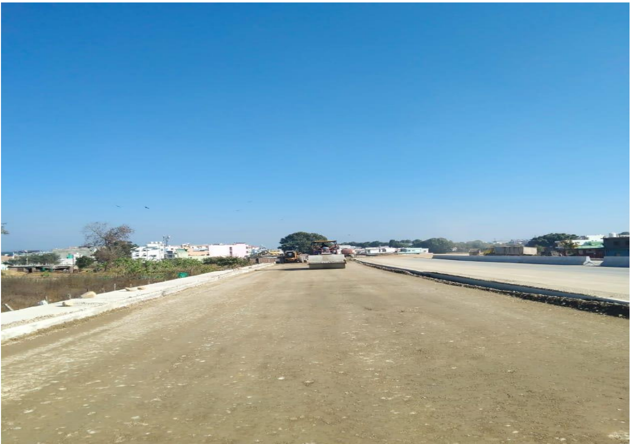
Service Road WMM Rolling Work in Progress at Ch. 38+600 to 38+820 LHS
