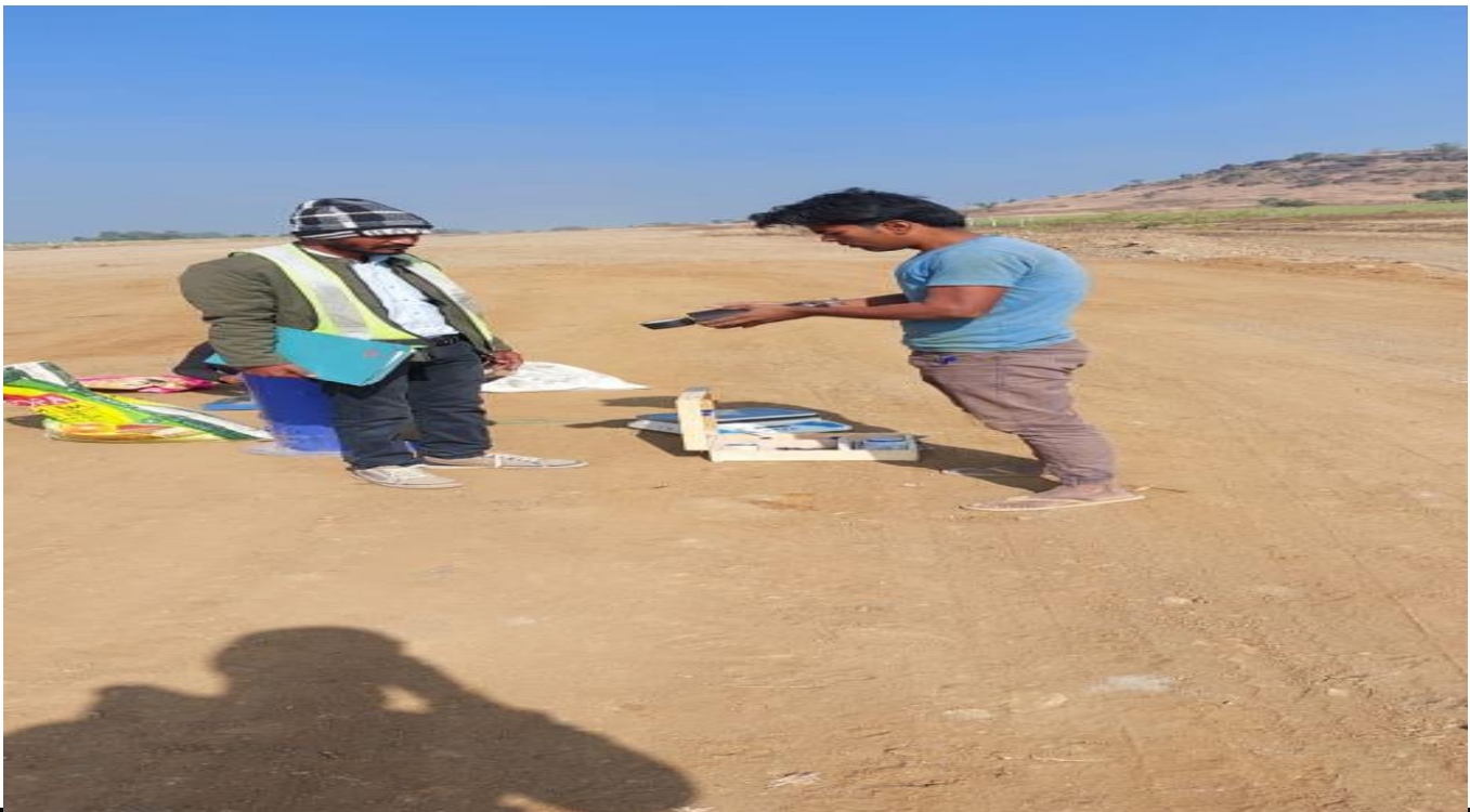
FDD Testing of embankment Layer
