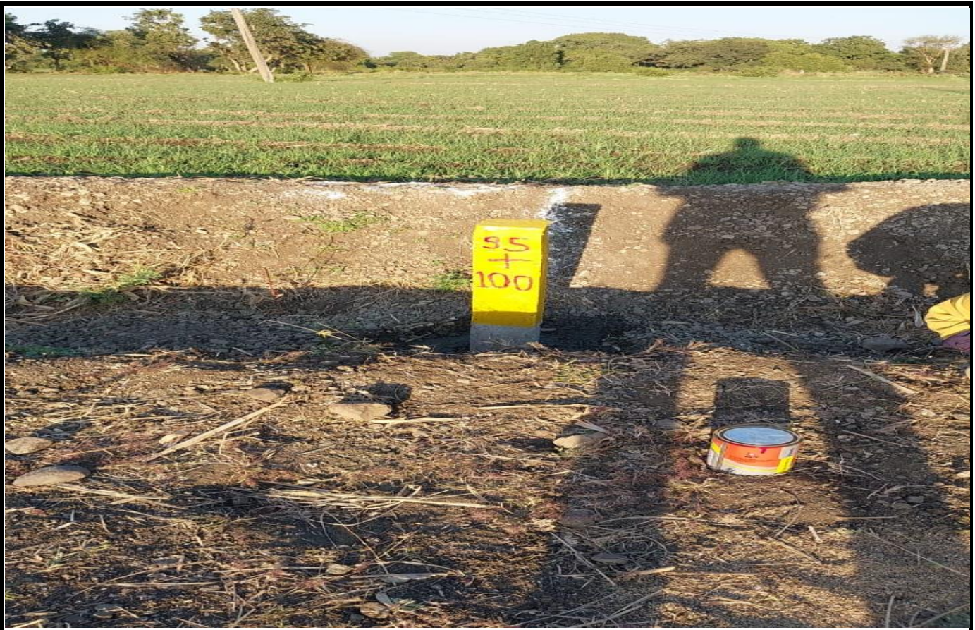
Chainage Pillar Erection
