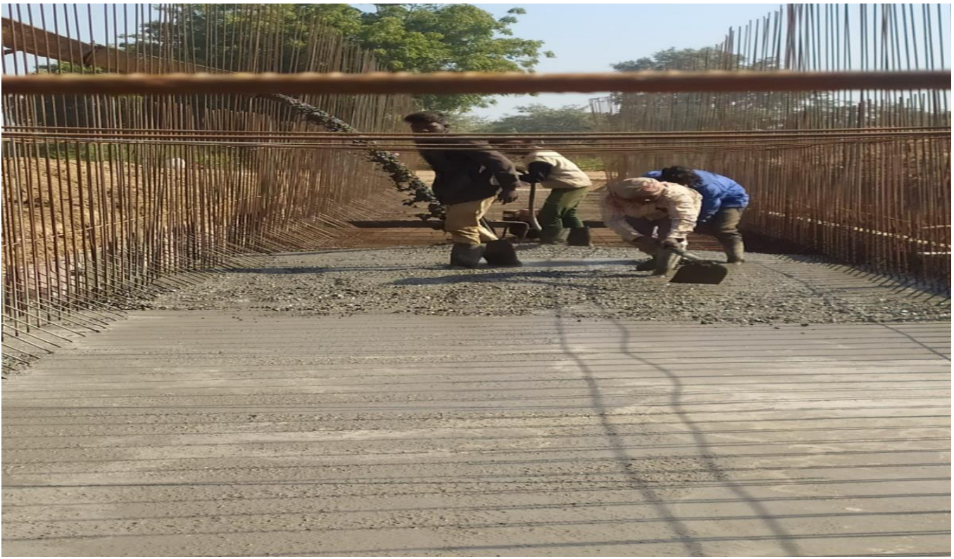
Raft Casting Work in Progress
