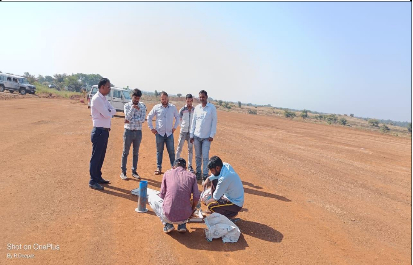
FDD Testing of embankment Layer
