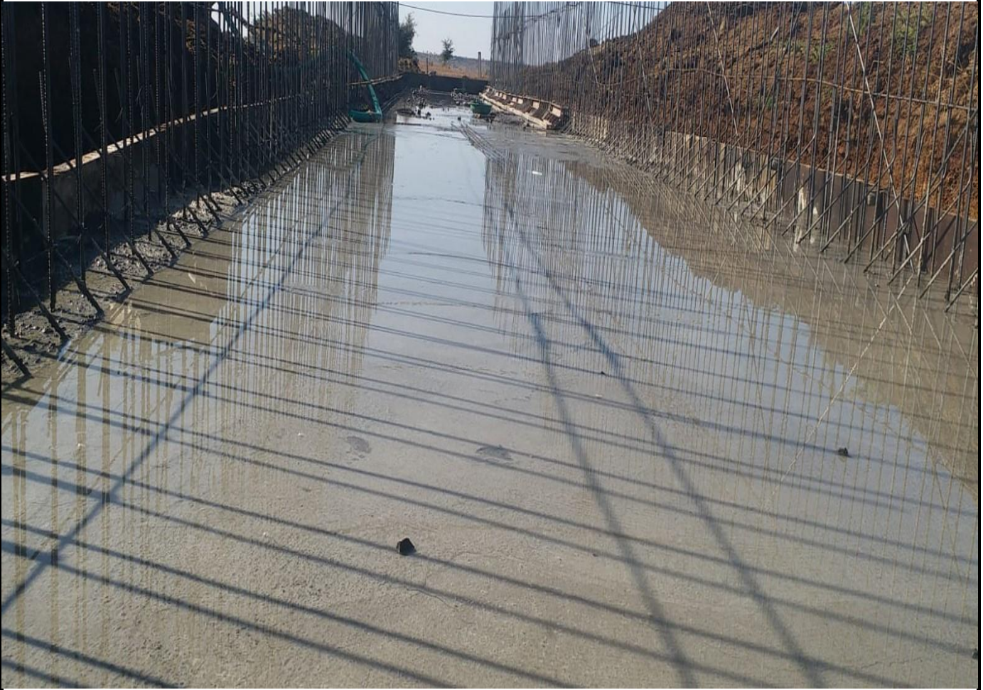
Curing of Bottom Slab
