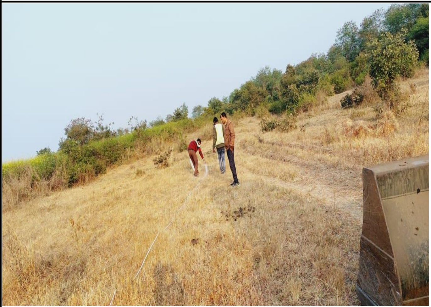
Borrow Area Marking
