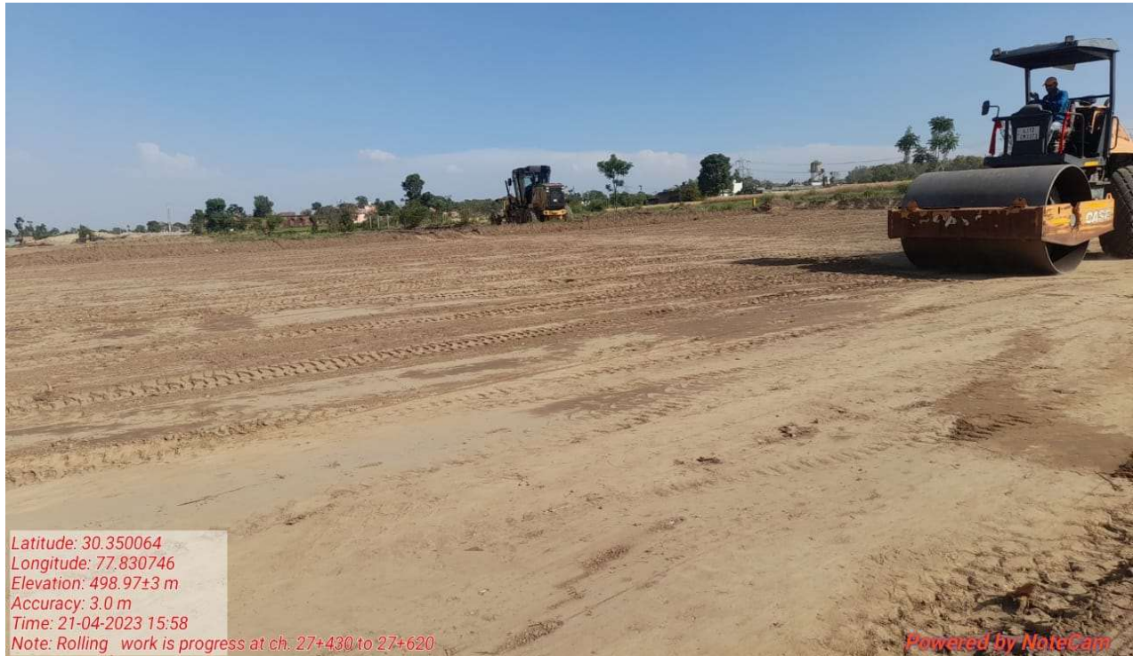
OGI Bed Preparation at Ch 27+430 to 27+620.
