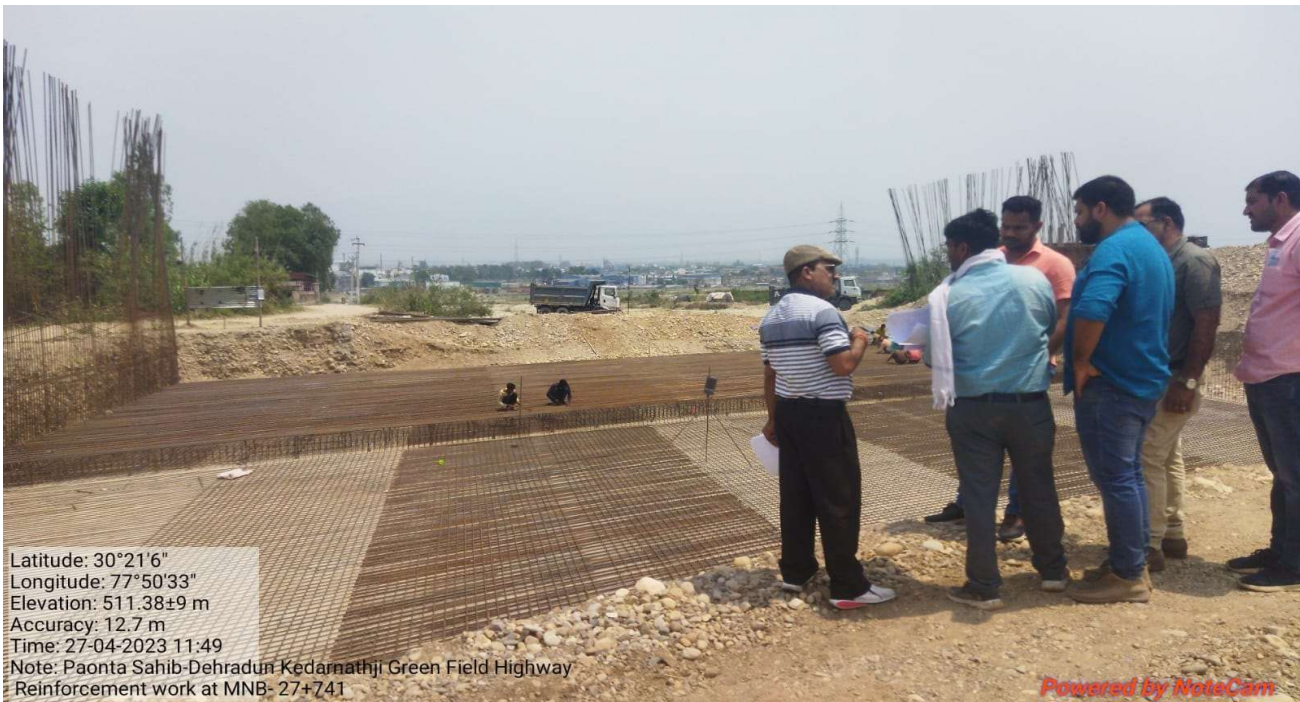
Reinforcement Checking of MNB 27+741 by I.E Team.
