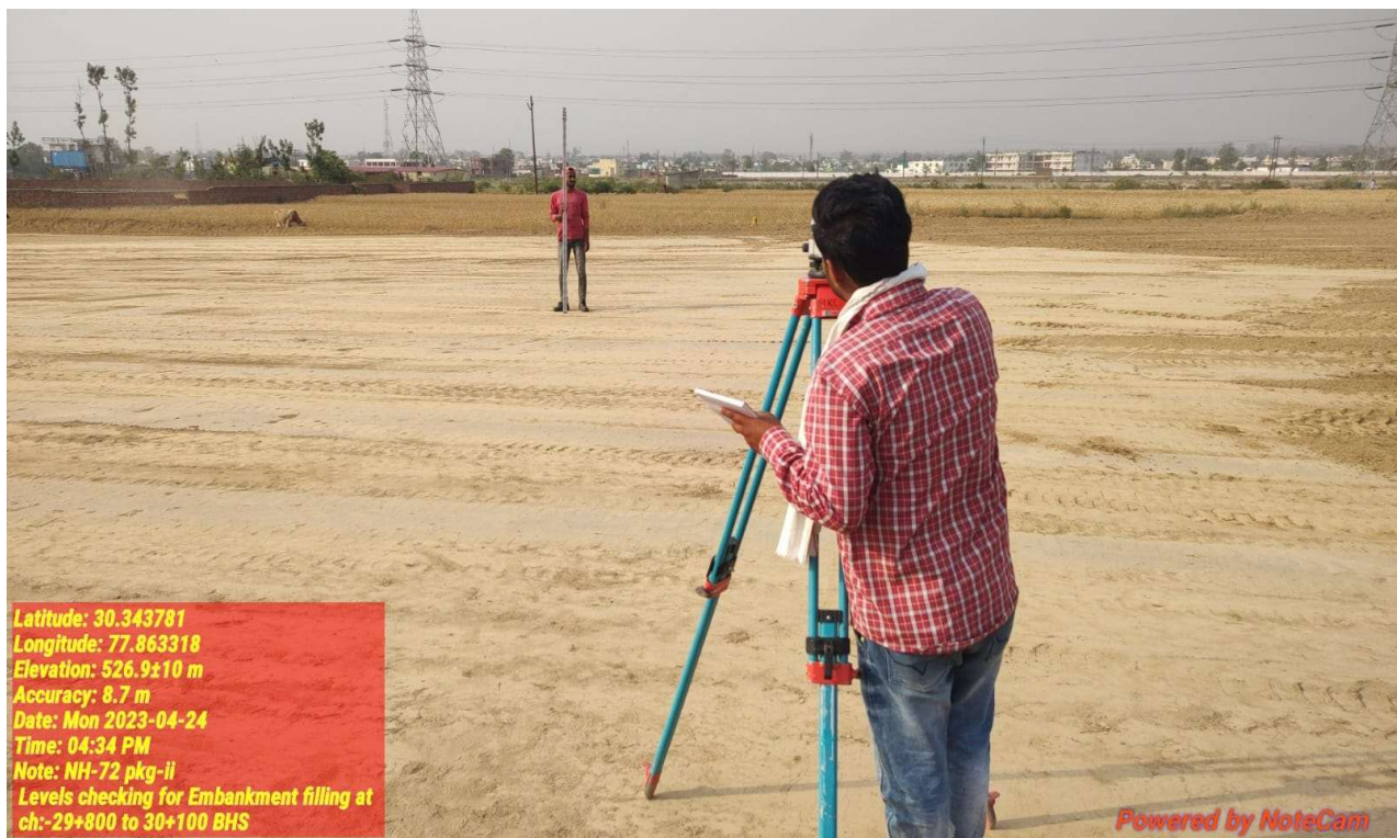
Level Checking for EMB Filling at Ch 29+800 to 30+100.
