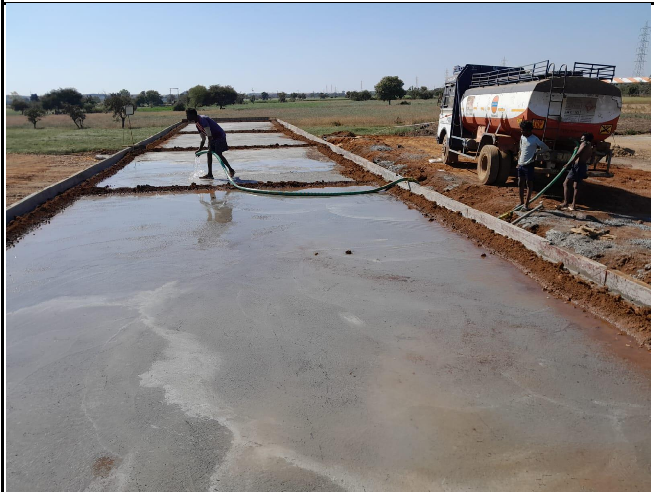
Curing Work in progress
