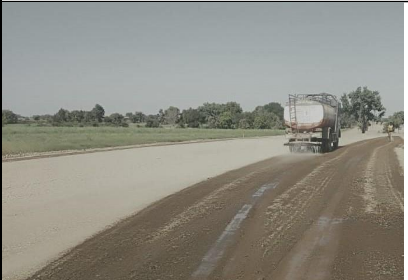
Watering on Embankment Layer
