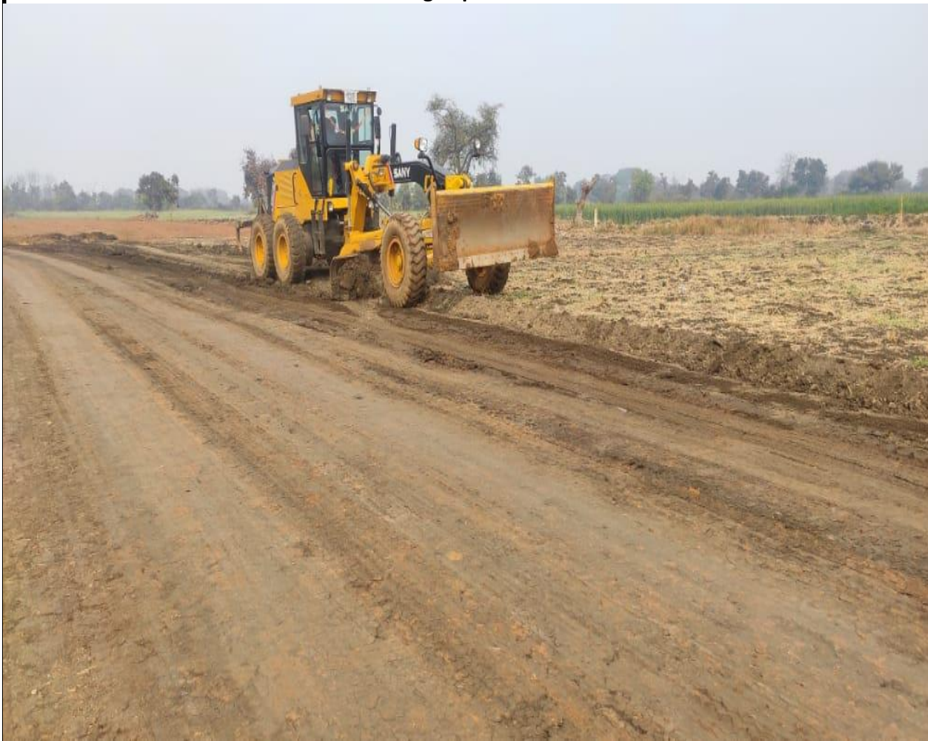
C&G Work in progress
