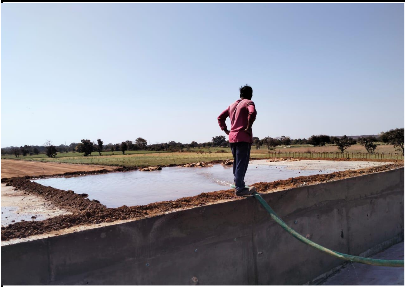
Curing Work in progress
