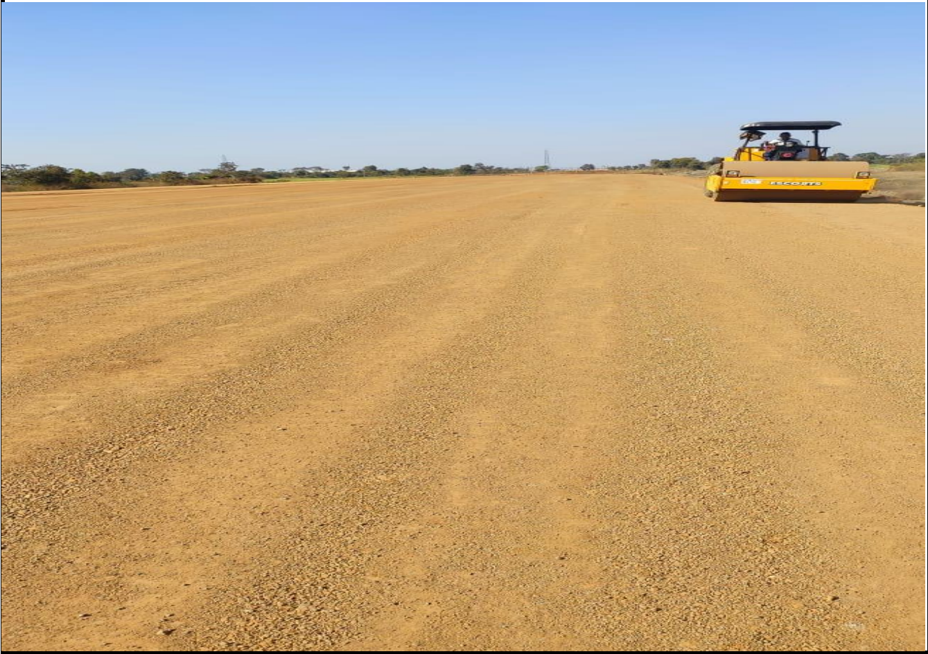
Rolling on Embankment Layer
