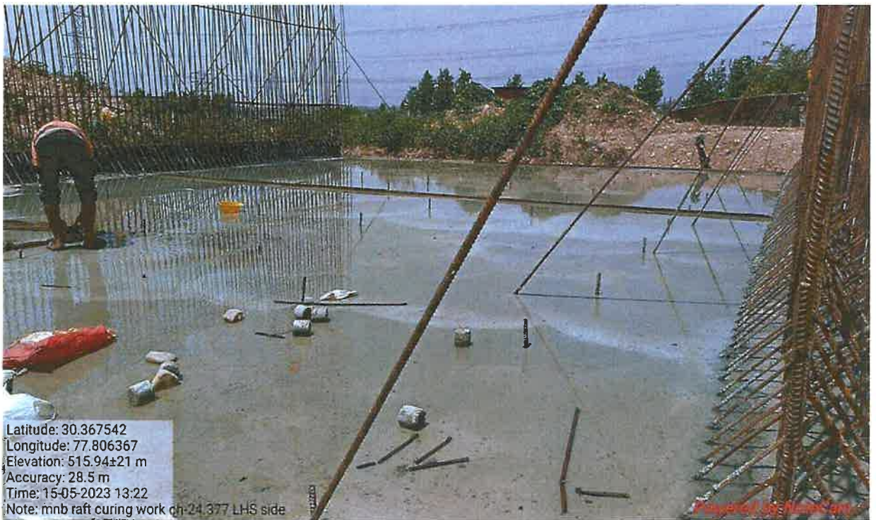
Raft Steel Checking by BE Sir.
