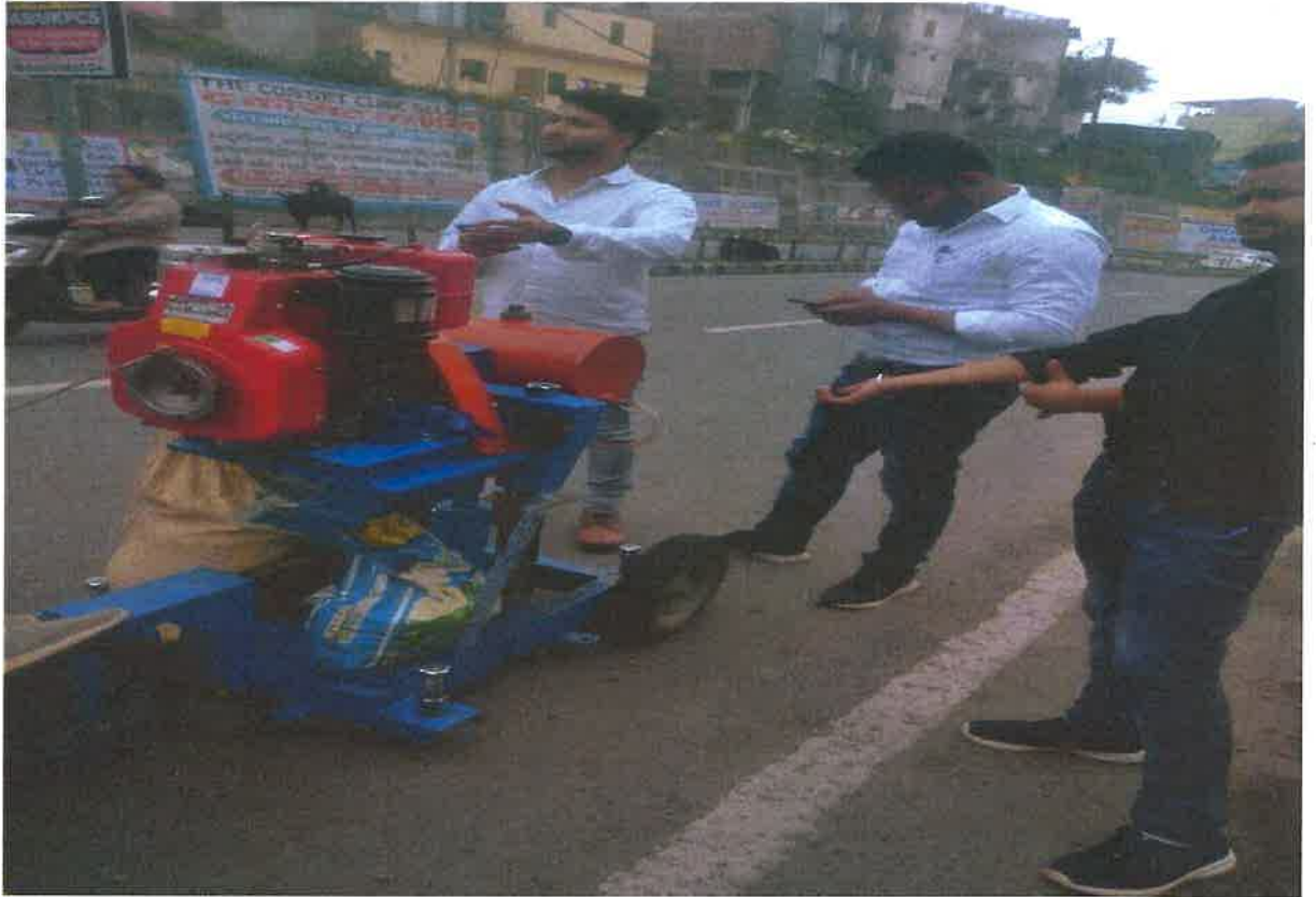
Existing Road Layer Thickness Checking
