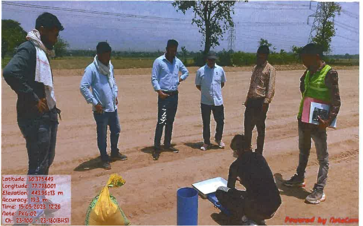
FDD Checking at Ch 23+100 to 23+180.
