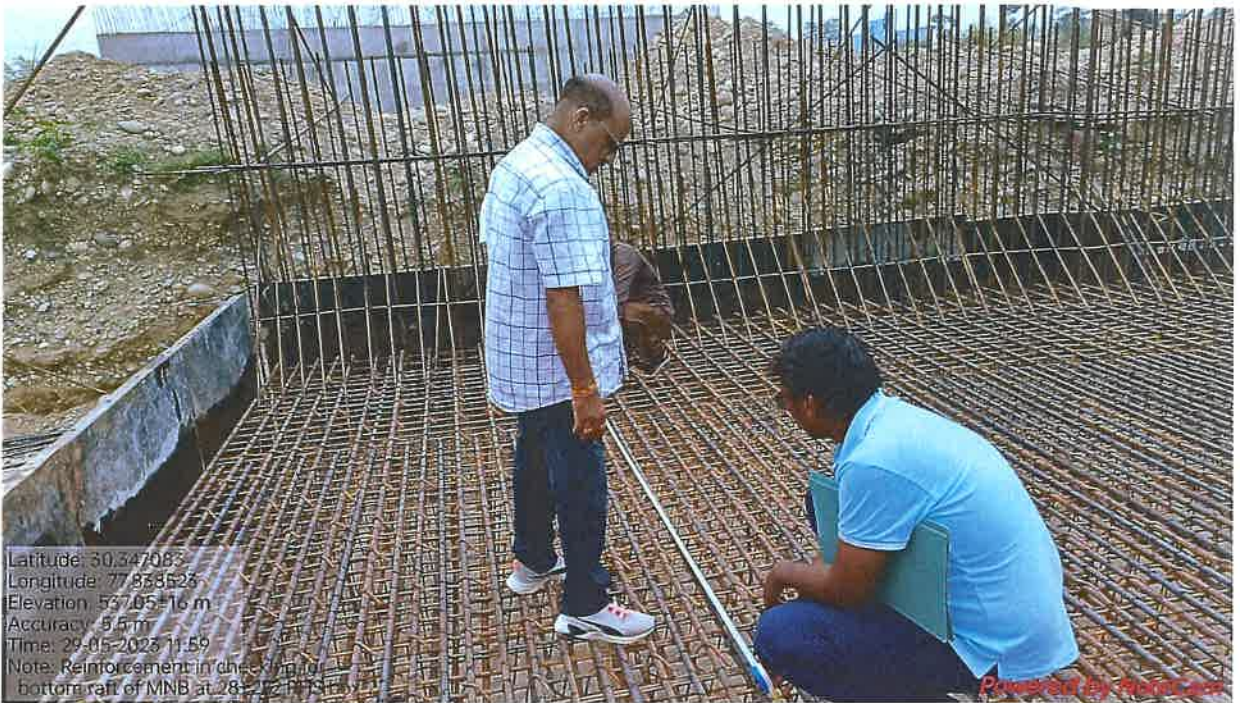
Raft Steel Checking by BE Sir.
