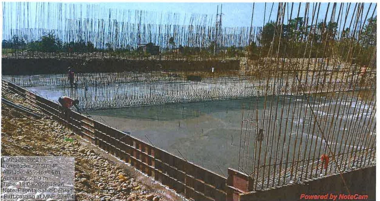
EMB 1st Layer in Progress
