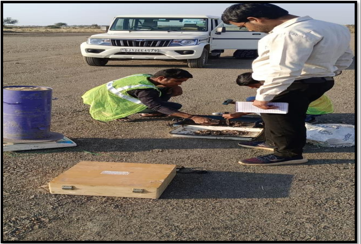
Embankment 6th Layer FDD Checking at Ch. 116+480 to 116+520 RHS
