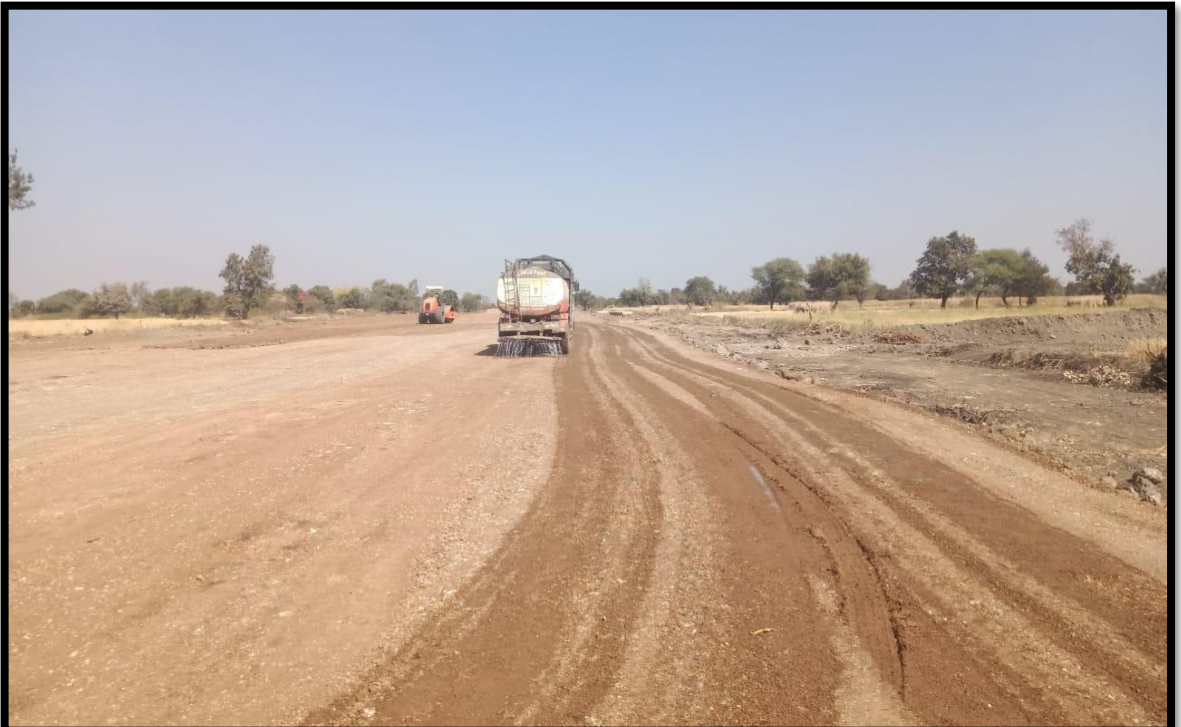
Watering on Embankment Layer at Ch. 91+800 to 92+100
