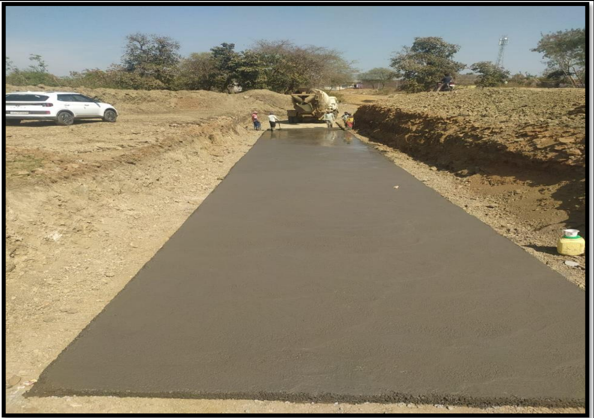
Box Culvert PCC Work in Progress
