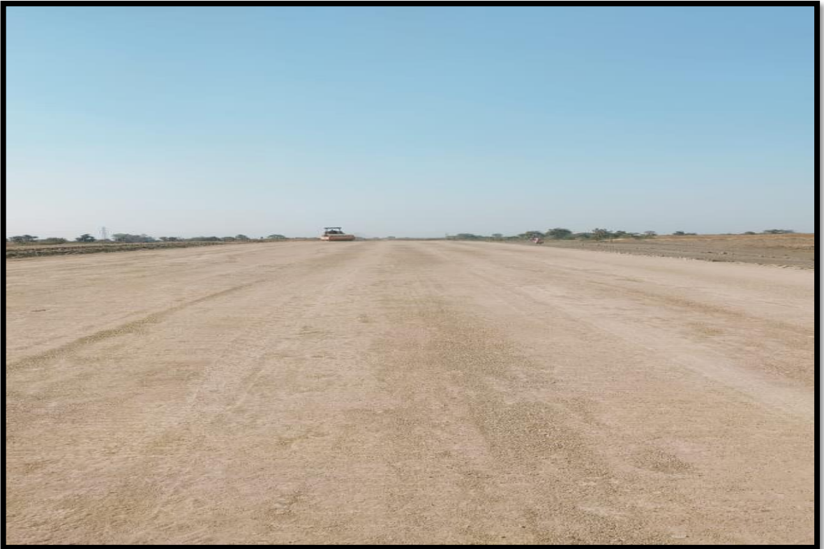
Sub-Grade Top at ch. 97+800 To 98+540 BHS
