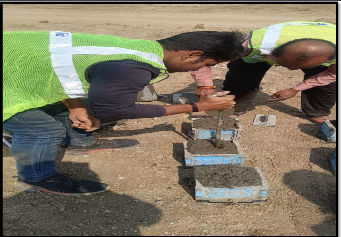
Cube Test at Ch. 117+240 BHS
