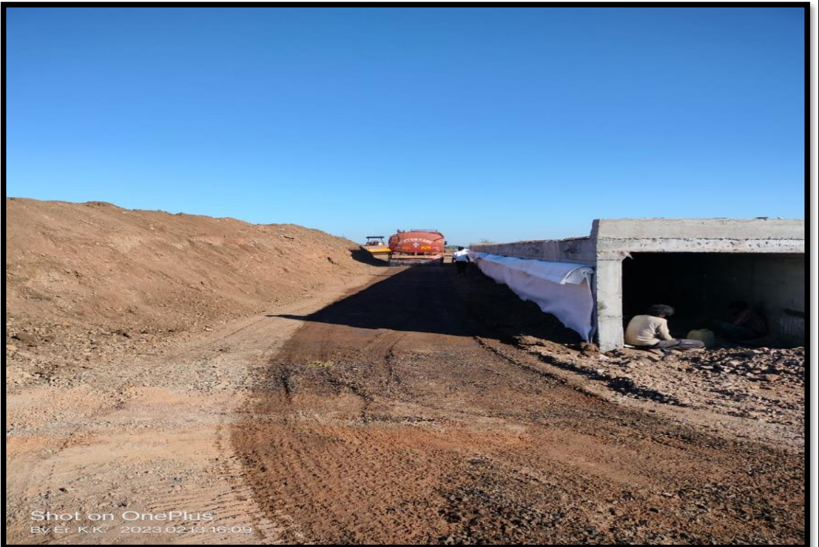
Back Filling Work in Box Culvert at ch. 106+650
