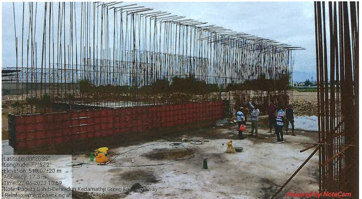
Wall Reinforcement Checking MNB 30.300.
