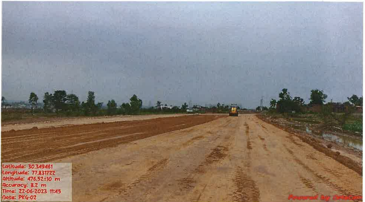
EMB 3rd Layer Rolling work at Ch 27.540 to 27.600
