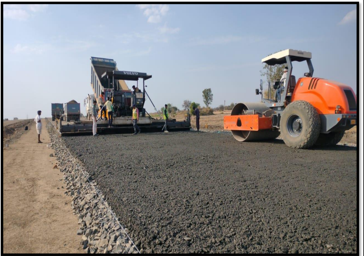
WMM Laying at Site
