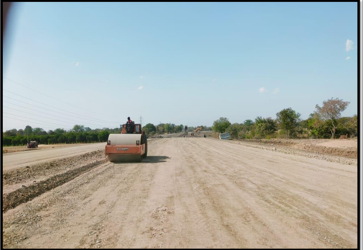
Sub-Grade Top Rolling Work in Progress
