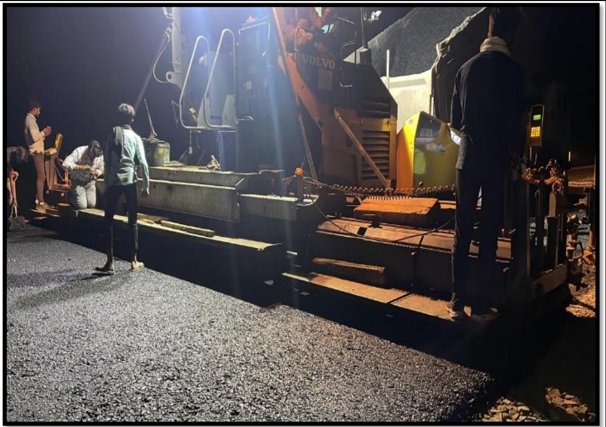
DBM Work in Progress at Site at Ch. 97+000 to 97+300 RHS
