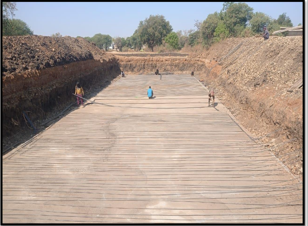
MNB 108+513 Raft Reinforcement Work in Progress
