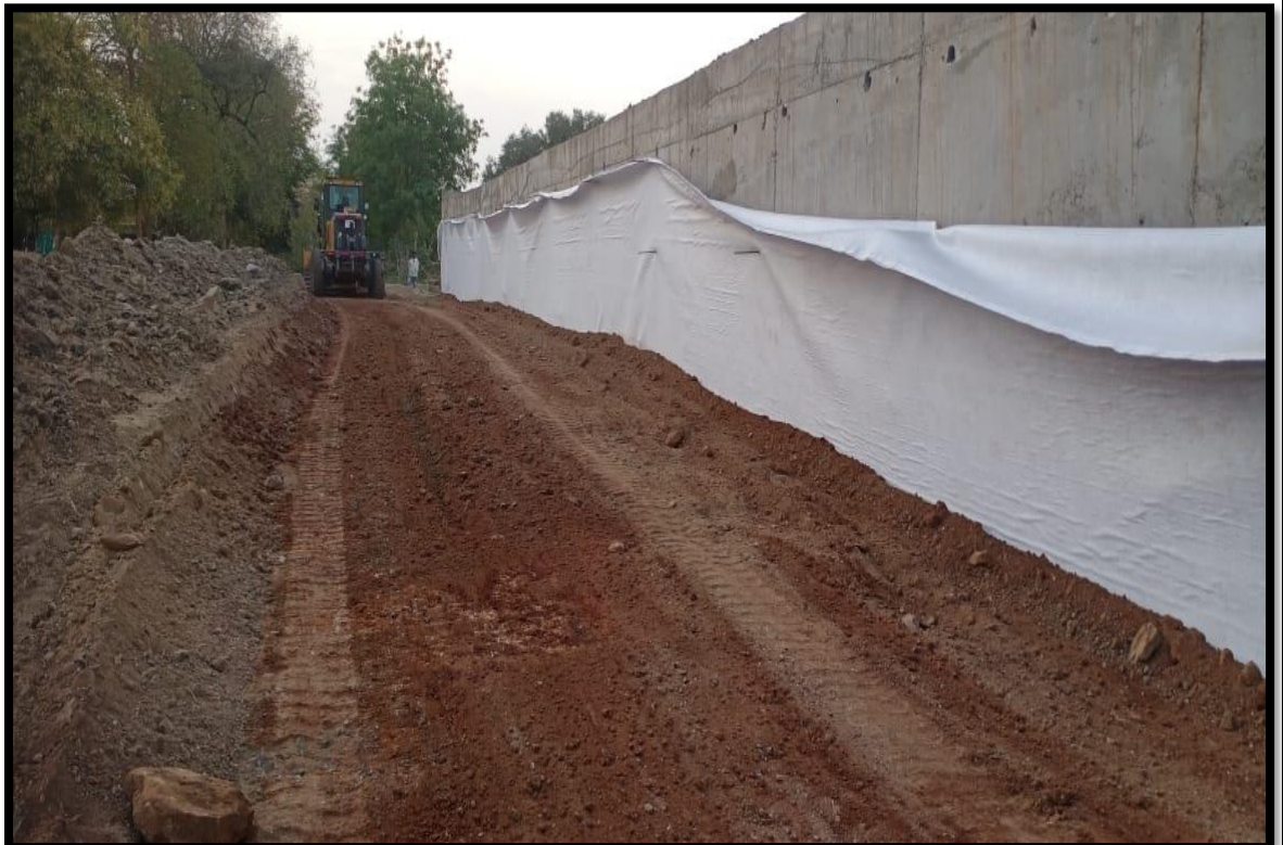
Box Culvert Backfilling Work in Progress at various locations
