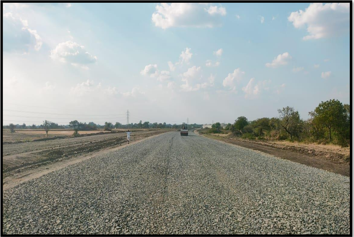
GSB Work in Progress
