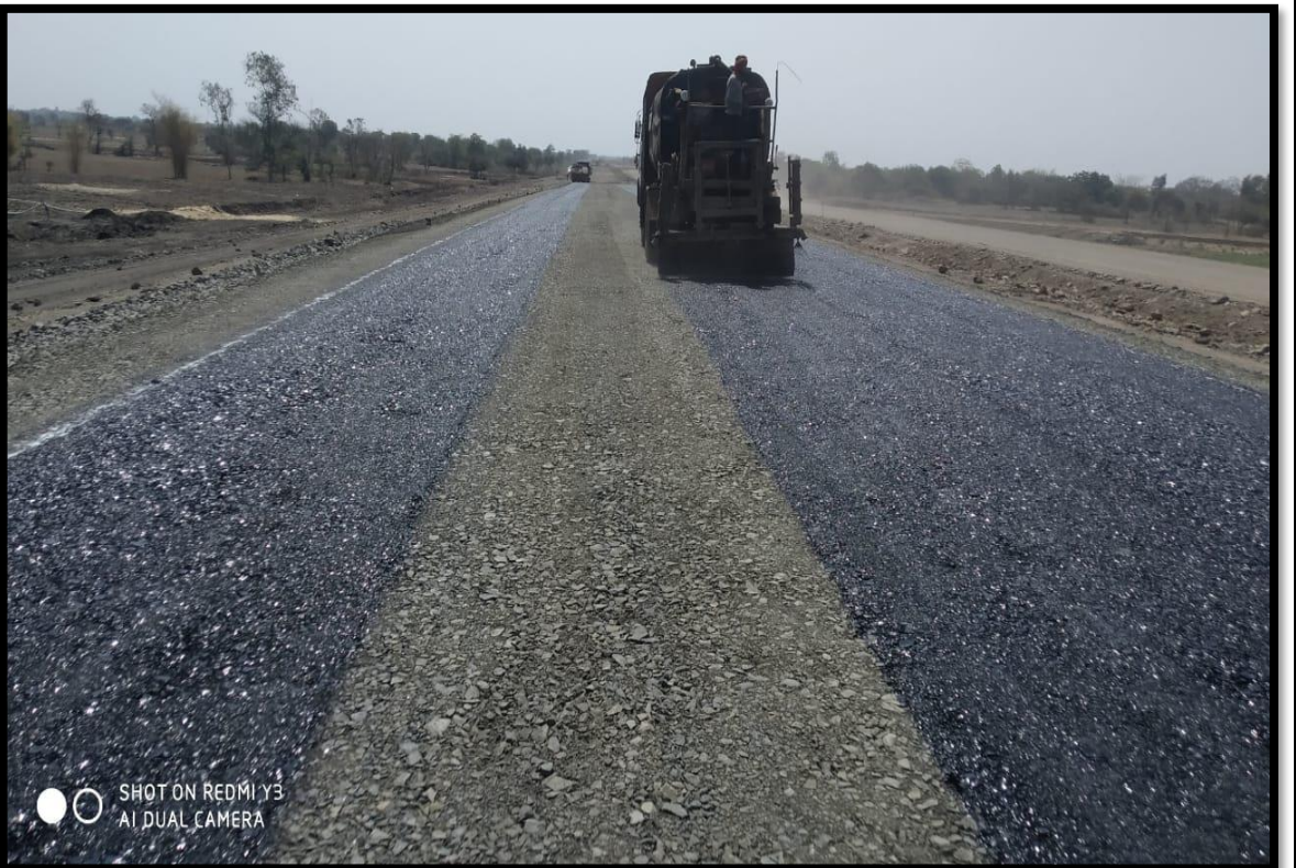
Emulsion spraying at WMM Top
