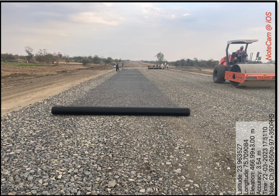
Geo-Grade Laying Work in Progress
