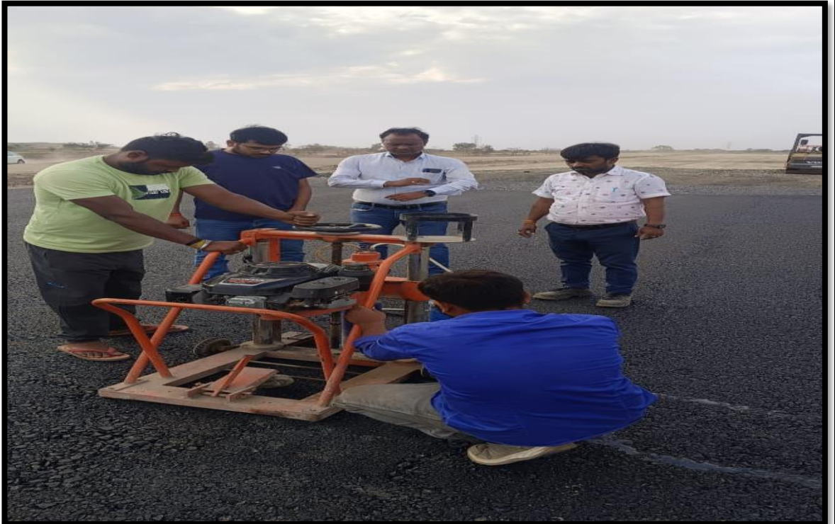
DBM Grade-II Core cutting at Ch. 97+070 to 97+270 RHS
