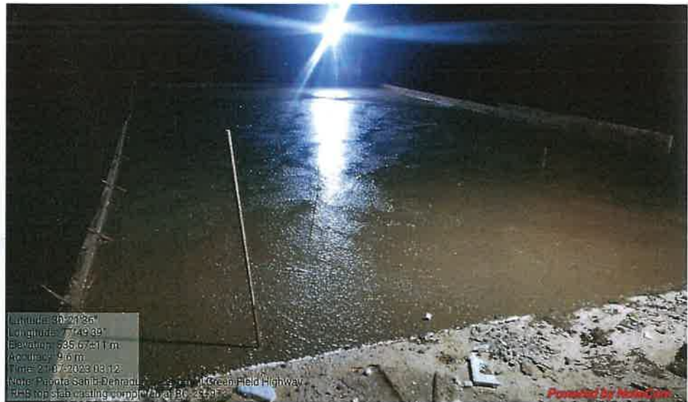
Box Culvert 25.973 Top Slab Casting
