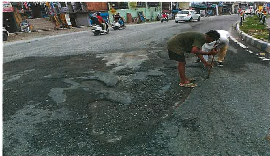
Existing Road Repairing work near Ch 40.100.
