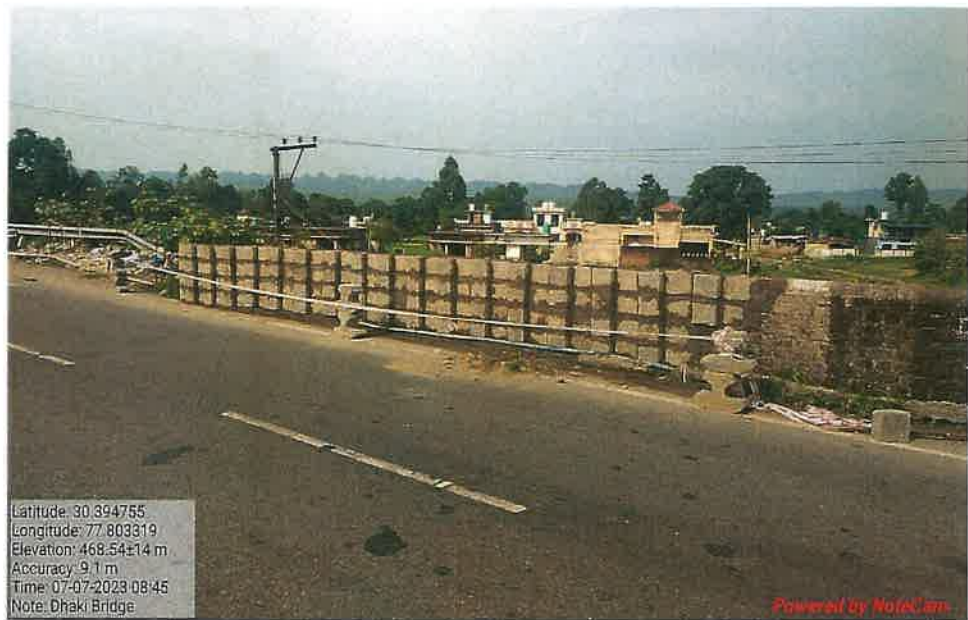
Existing Dhaki Bridge Repairing
