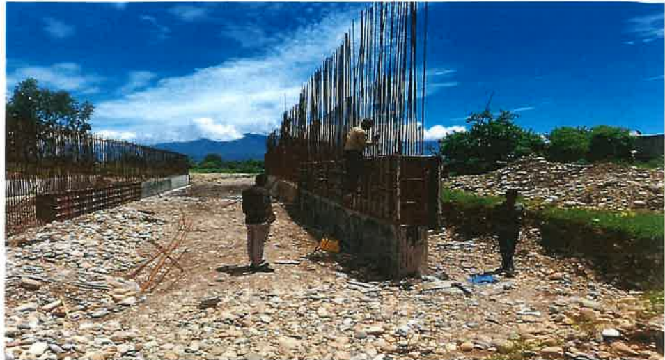
MNB wall 1st Lift Checking by ABE.
