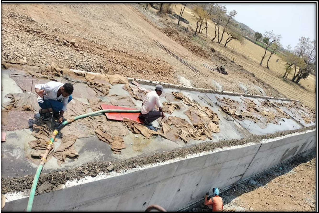
Box Culvert Curing Work
