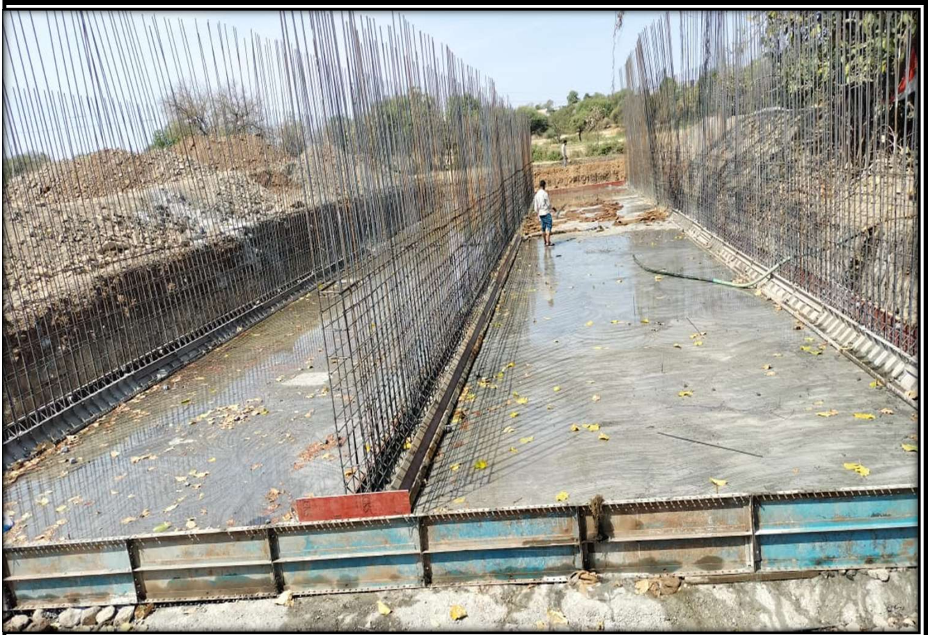
MNB Raft Foundation Curing
