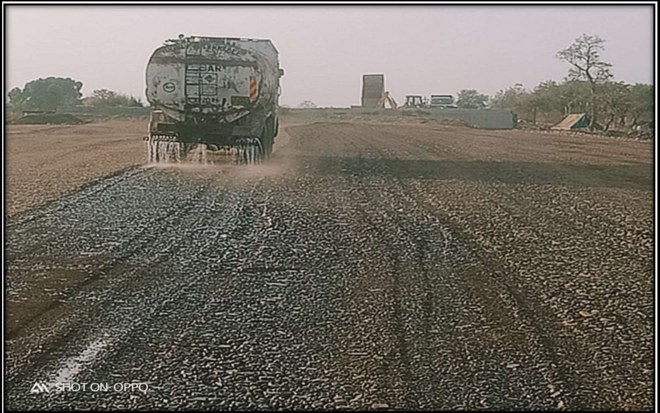
Embankment 4th layer watering in progress
