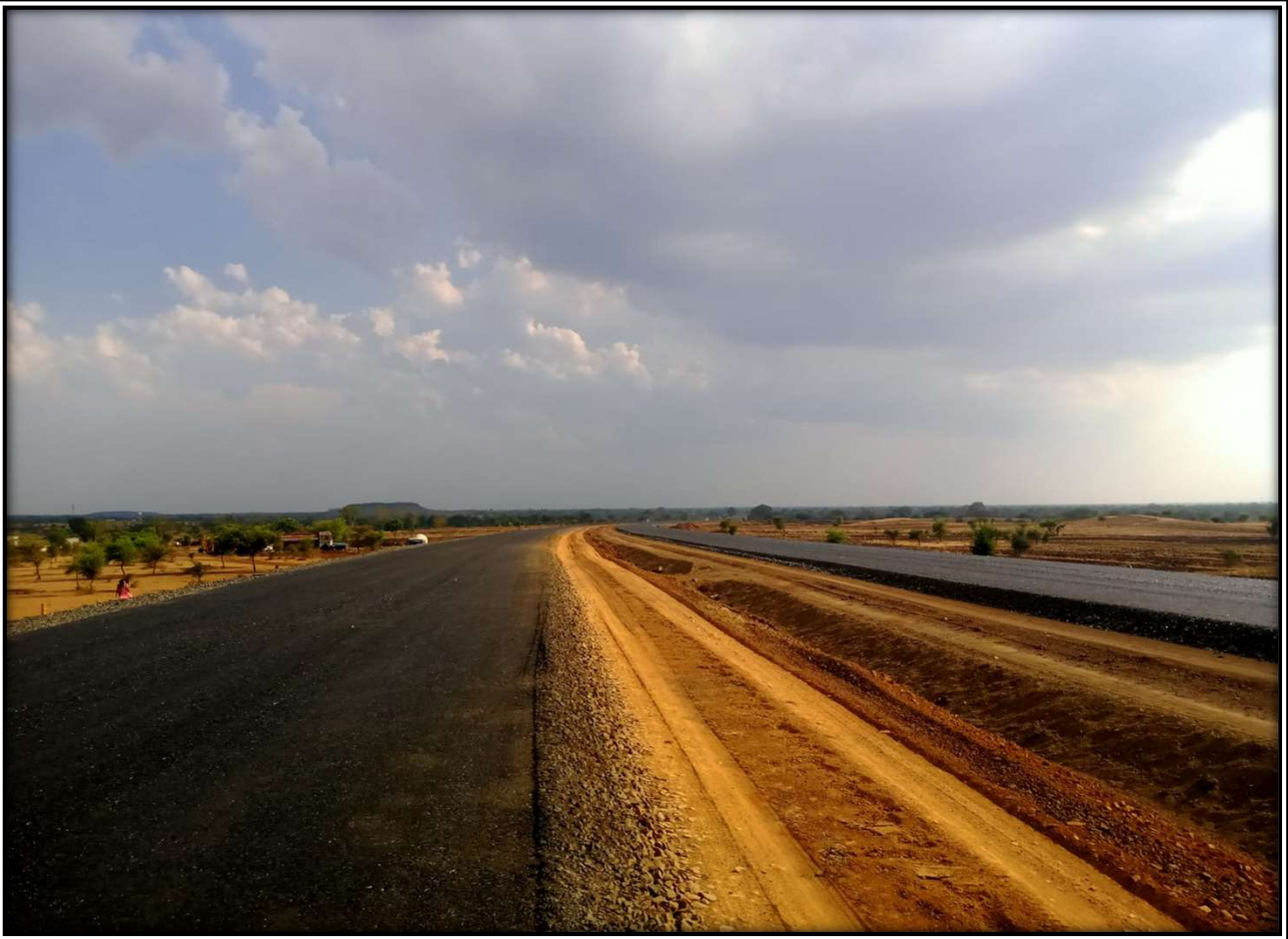
Prime coat spraying on WMM Top
