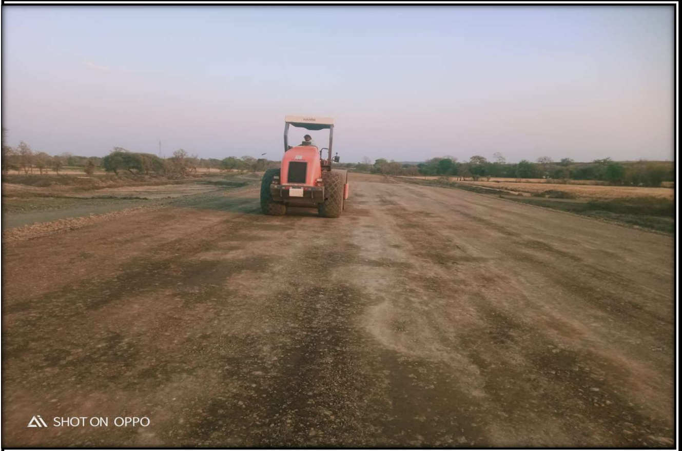
Sub-Grade work in Progress
