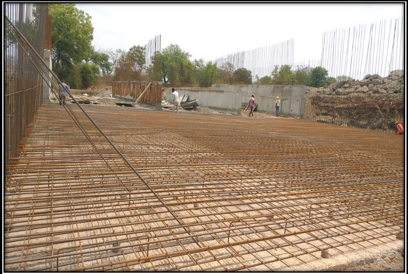
MNB Reinforcement Steel progress work
