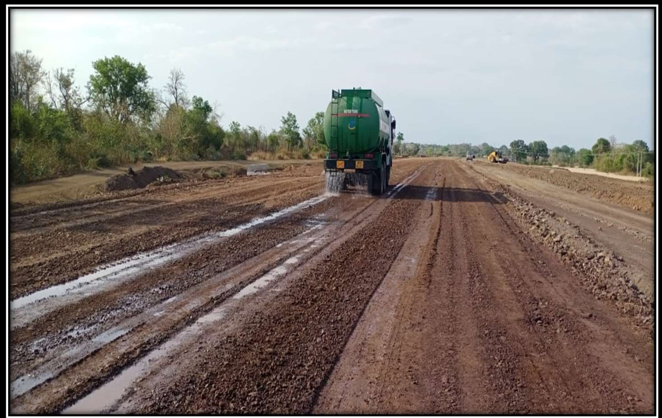
Watering subgrade top
