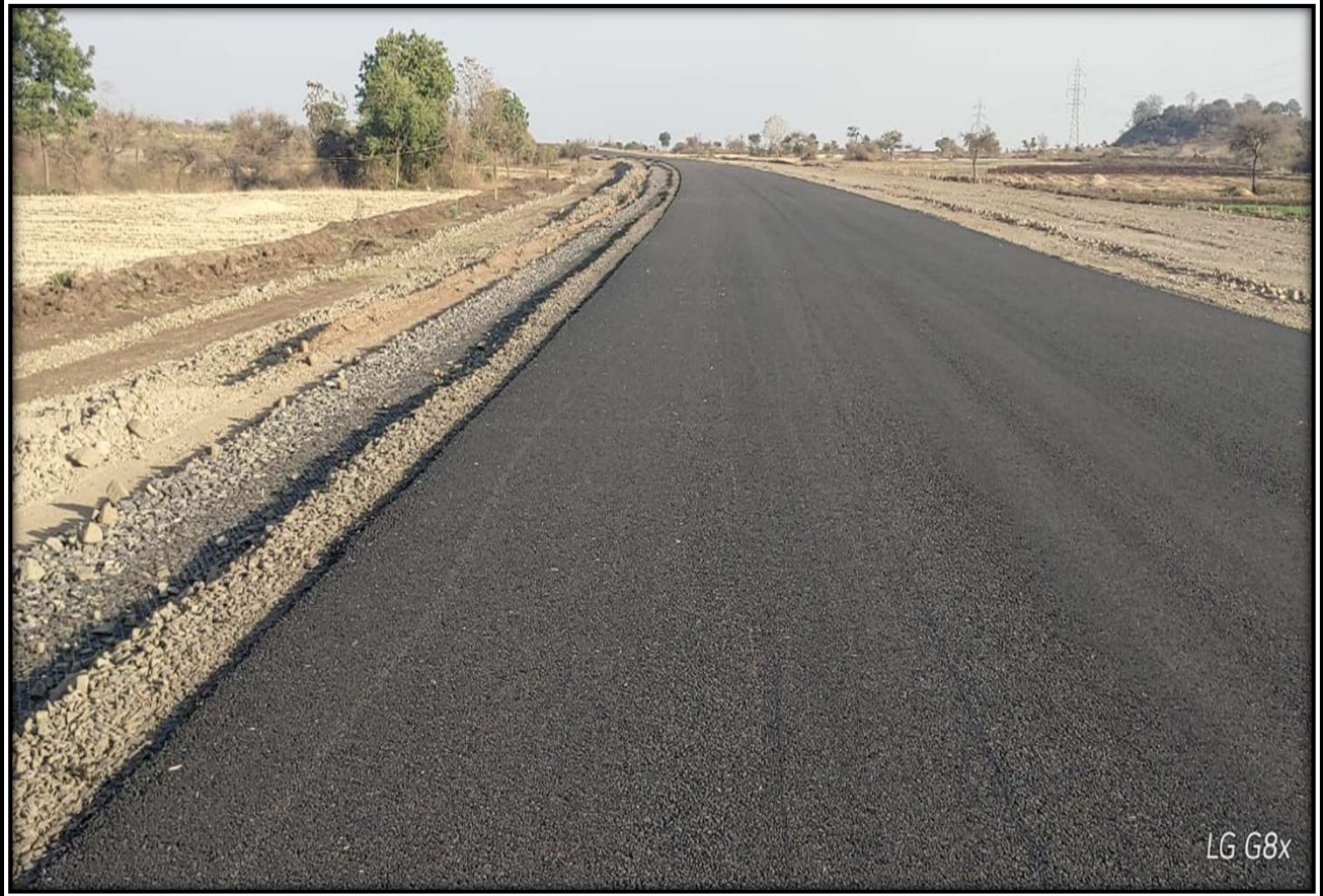
DBM Laying 98+000 To 97+500 RHS
