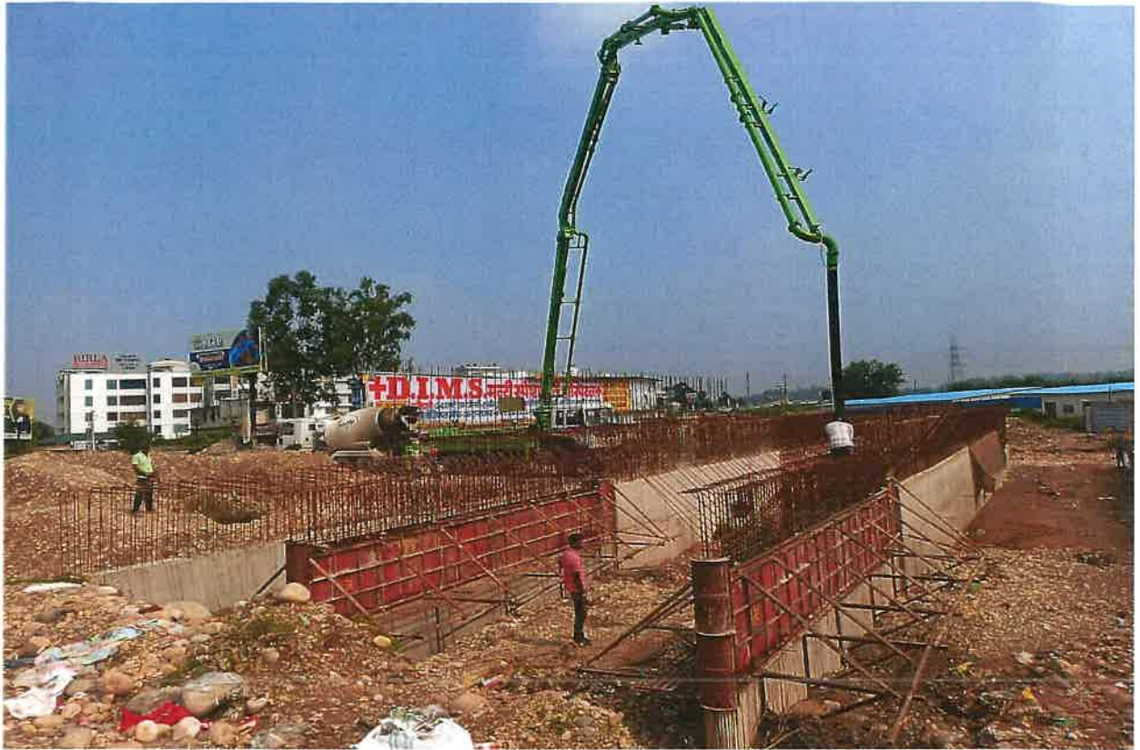
MNB Wall Casting at Ch.31+745
