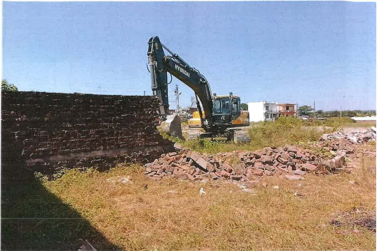
Dismantling of Obstruct Buildings from Aligment
