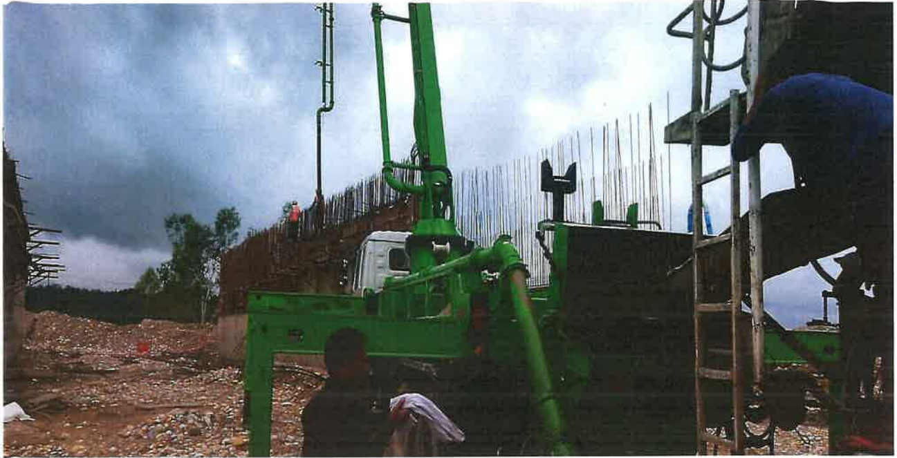
MNB Wall Casting at Ch.28+222
