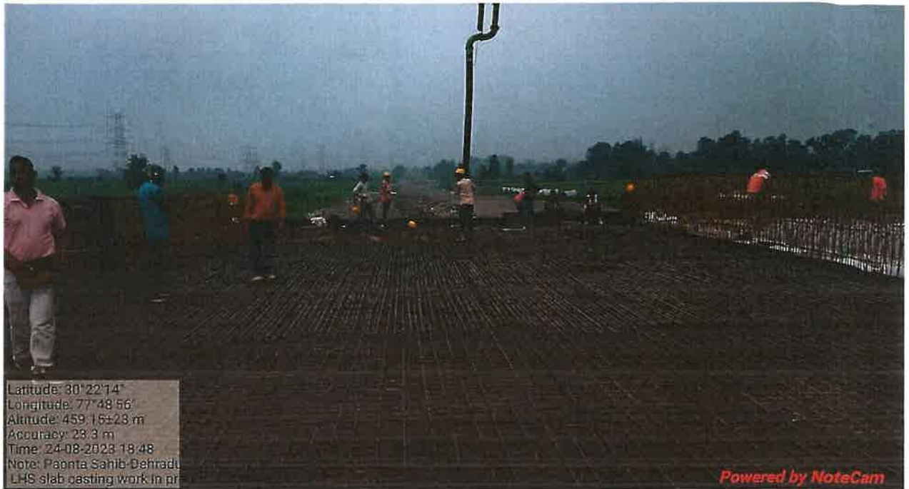
Top Slab Casting Work of MNB at Ch. 24+377
