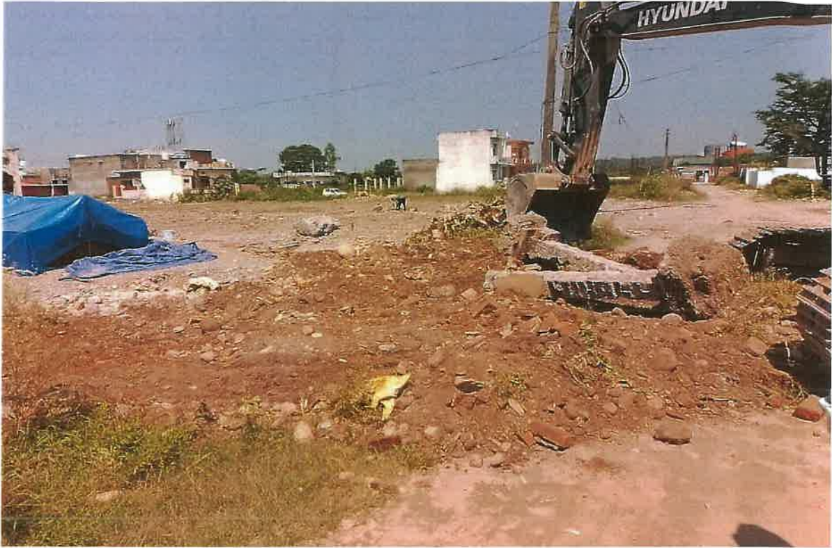
Dismantling of Obstruct Buildings from Aligment
