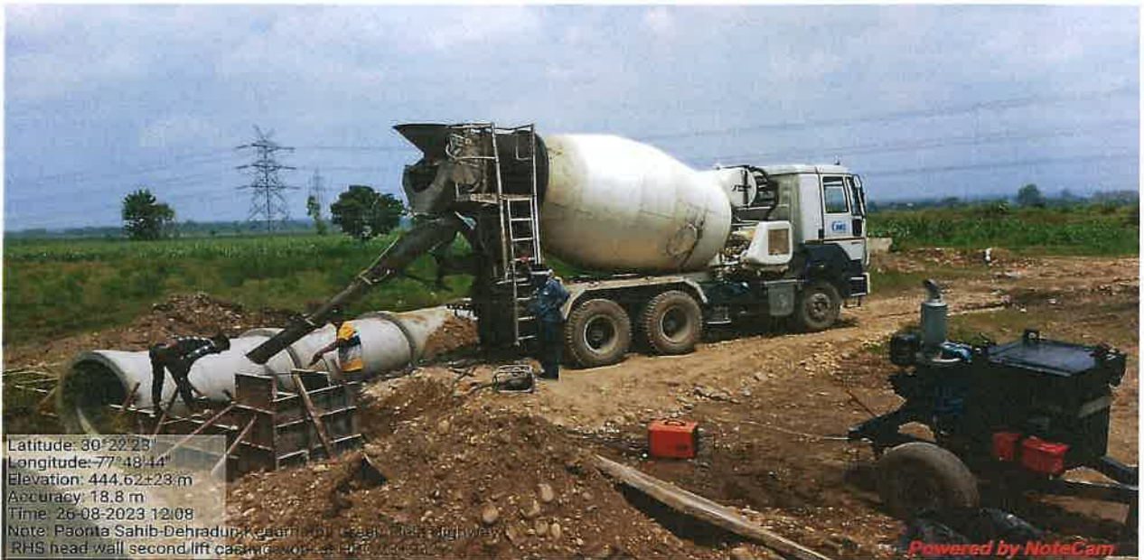
Head Wall Concrete Pouring Work of HPC at Ch. 23+932
