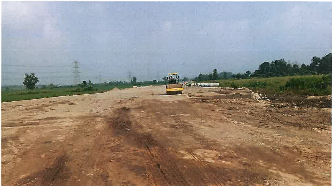
Embankment Bed Rolling Work in Progress at Ch. 24+400
