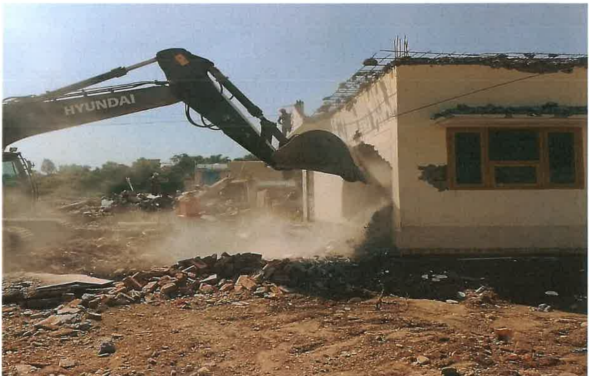
Dismantling of Obstruct Buildings from Aligment
