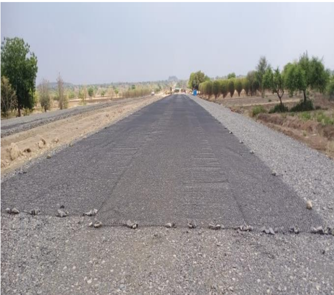
Geogrid Laying at Ch- 101+930 to 102+200
