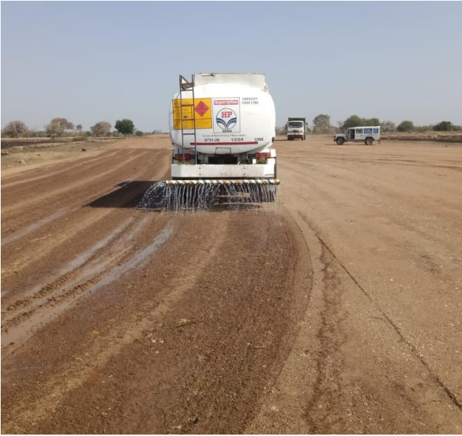
Sub Grade Laying at Ch- 97+680 to 98+520
