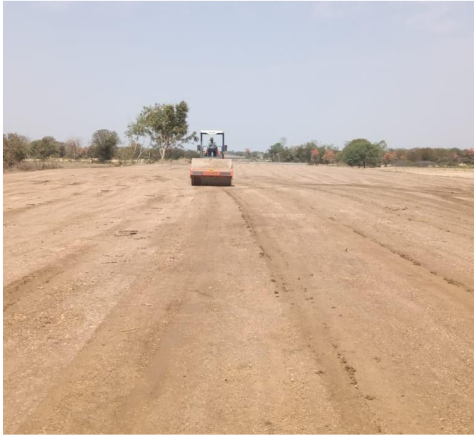
Sub Grade at Ch- 98+870 to 99+060
