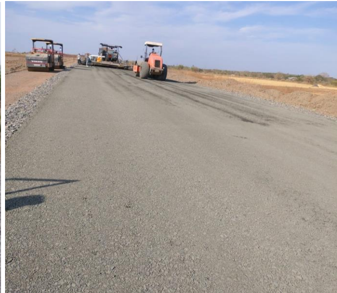
WMM Laying at Ch- 106+540 to 106+650
