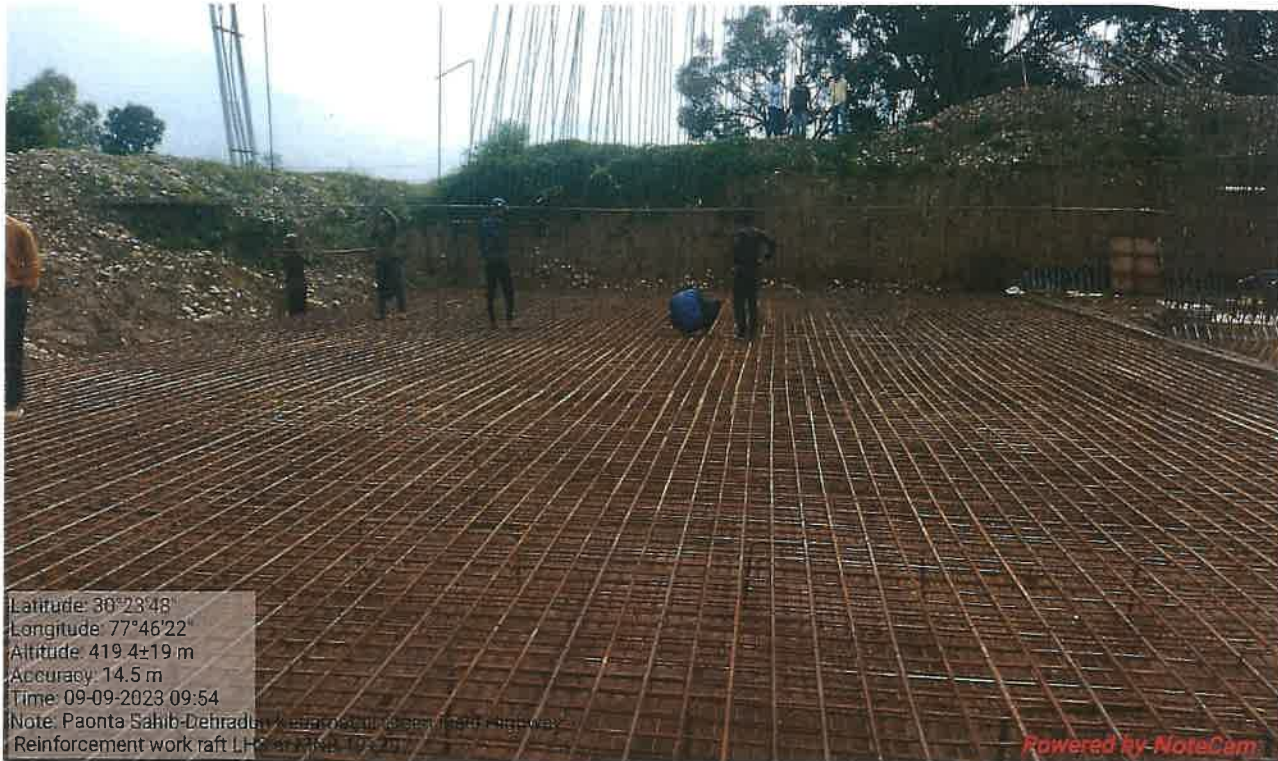
Raft Reinforcement Work of MNB at Ch. 19+297
