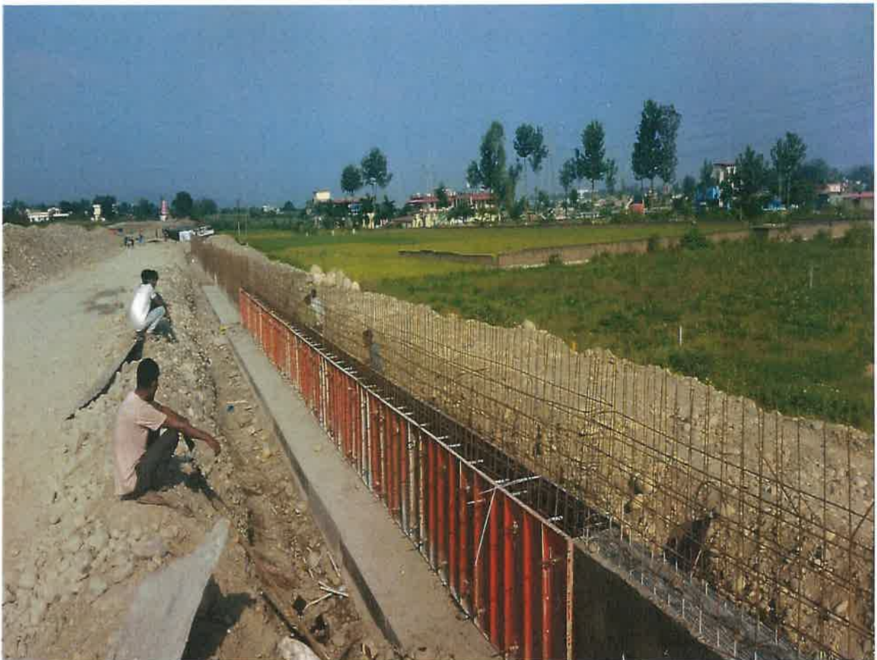
Toe Wall Reinforcement & Shuttering Work in Progress at Ch. 29+940
