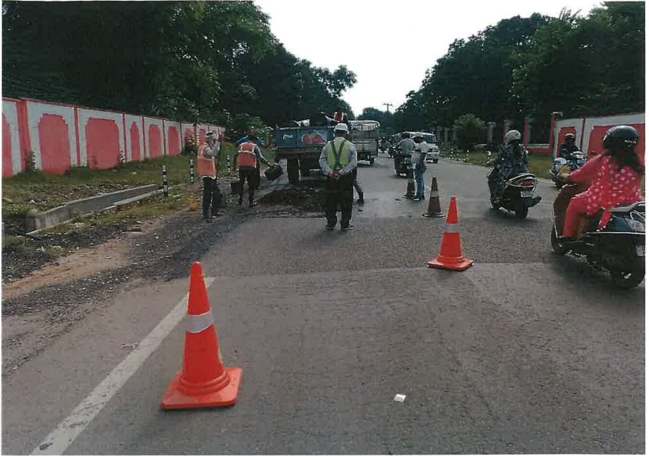
Patch Work at Ch.44+200
