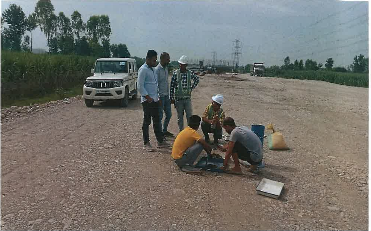
FDD Checking of Embankment Bed at Ch. 21+900
