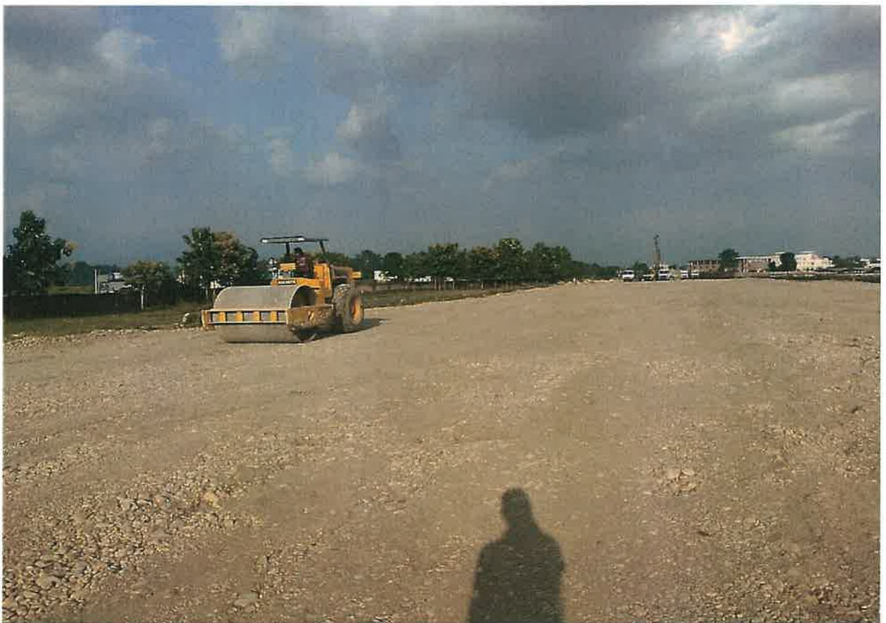
Embankment Bed Compaction Work in Progress at Ch.32+850
