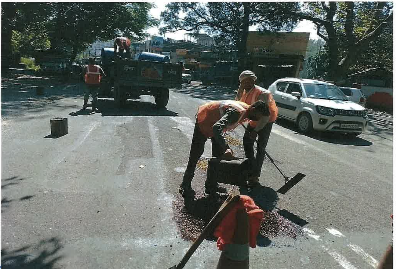
Patch Work at Ch.42+650
