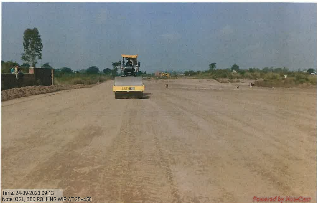
OGL Bed Rolling Work in Progress at Ch.35+450
