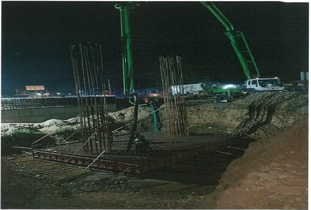
VUP Raft Pouring Work in Progress at Ch. 31+671
