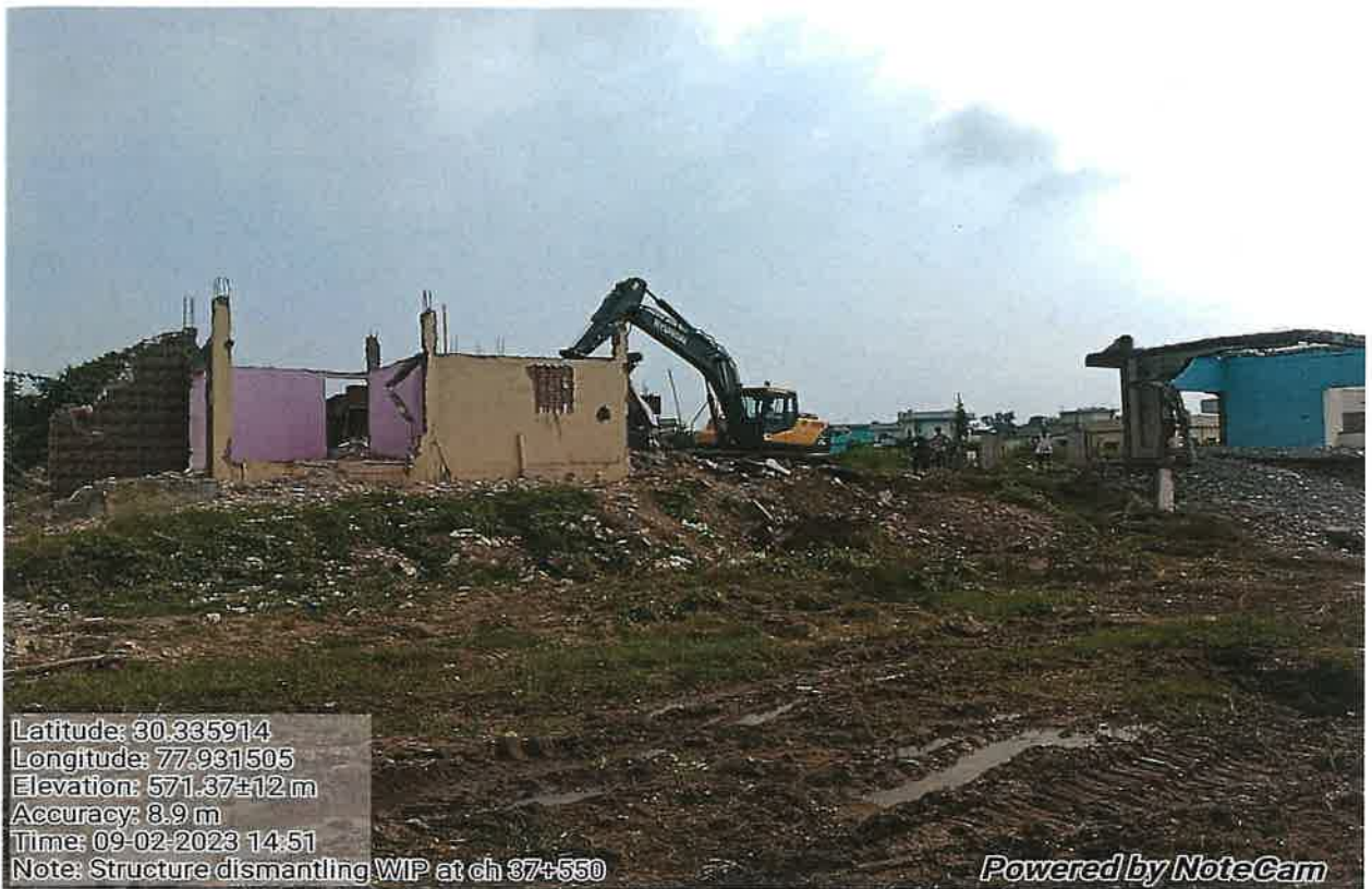
Dismantling of Obstruct Buildings from Alignment at Ch. 37+550
