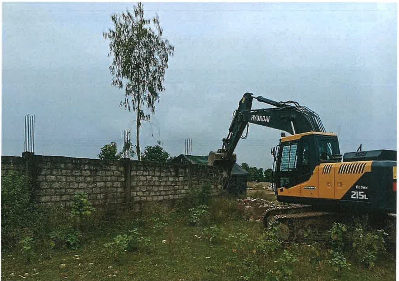
Dismantling of Obstruct Buildings from Alignment
