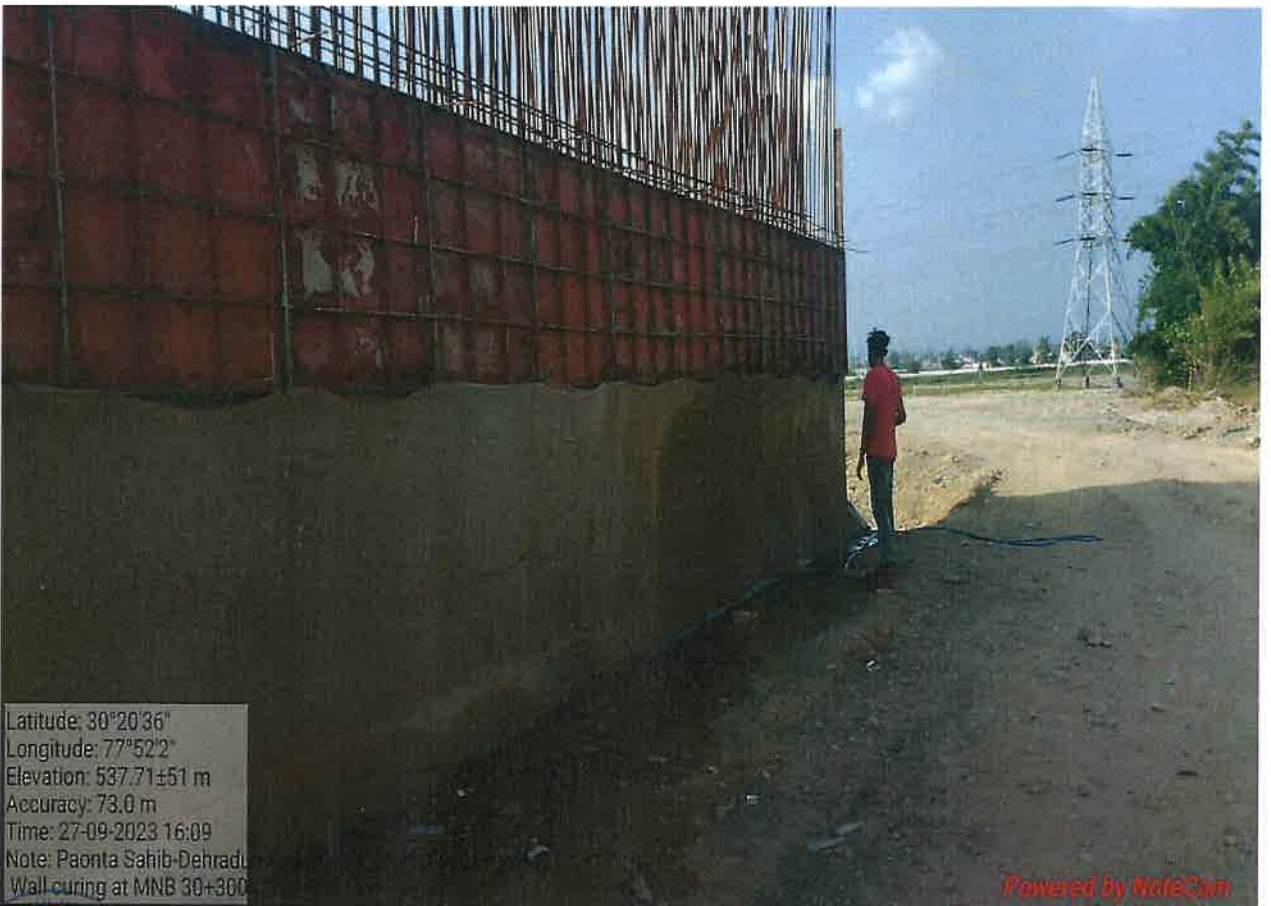
MNB Wall Curing Work in Progress at Ch. 30+300
