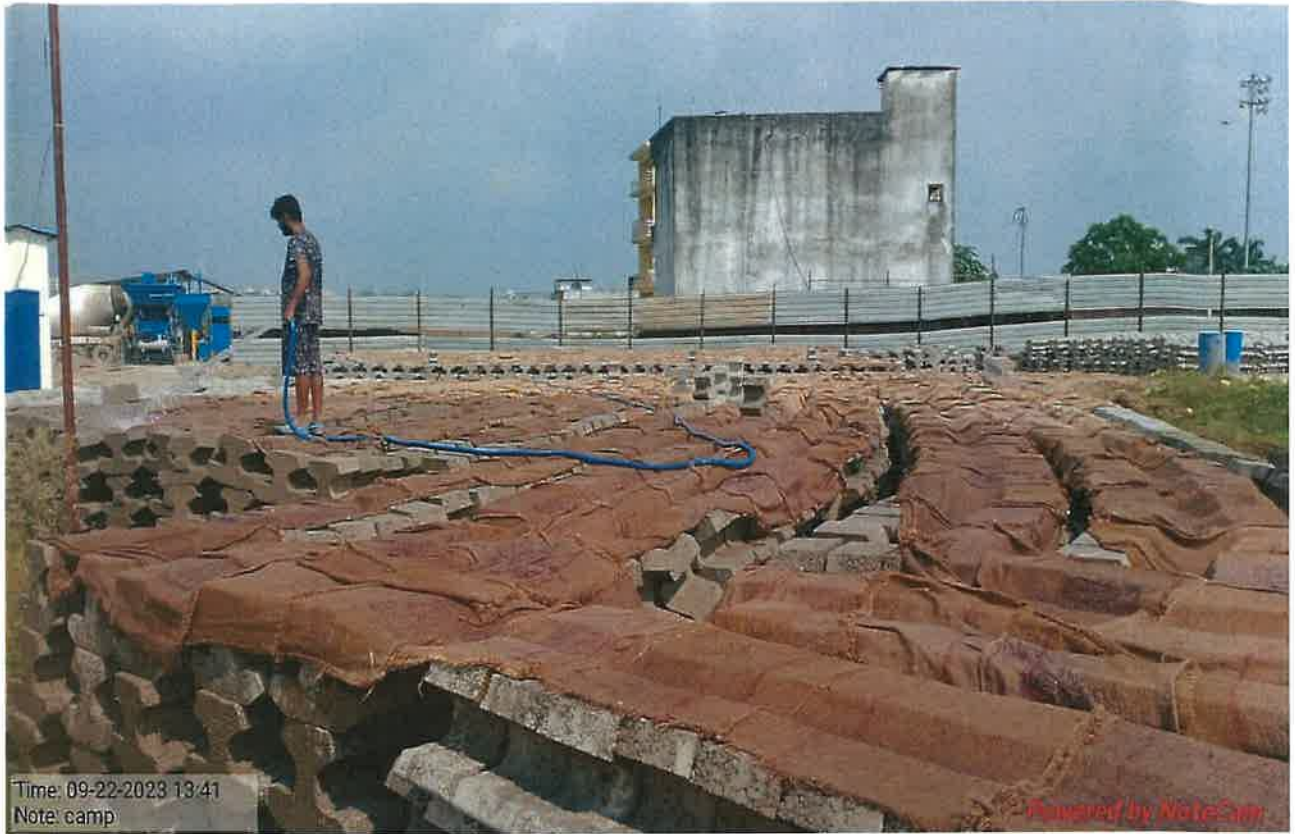
RE Block Curing Work in Progress
