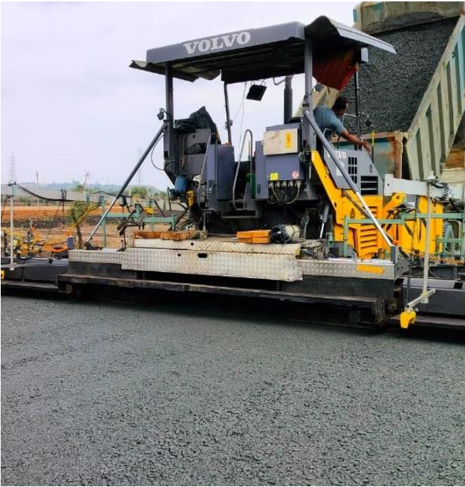
DBM Laying at Ch- 107+080 to 107+480
