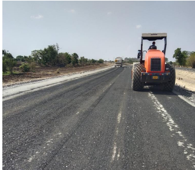
WMM 1 st Laying at Ch- 99+000
