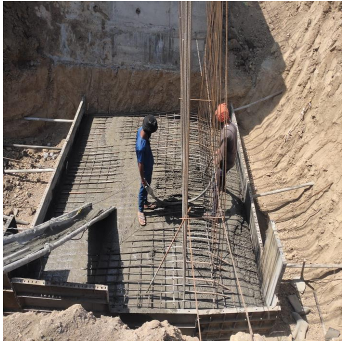
Retaing Wall Raft WIP at 99+345
