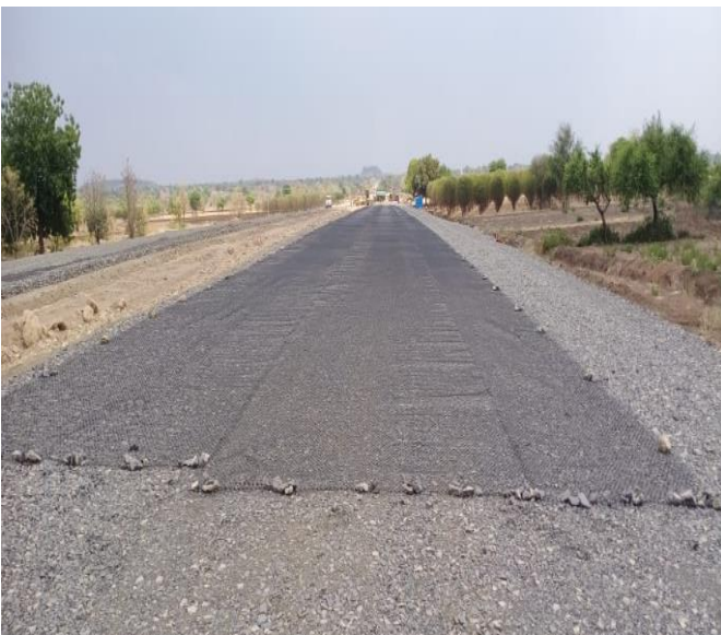
Geogrid Laying at Ch- 101+050 to 101+440
