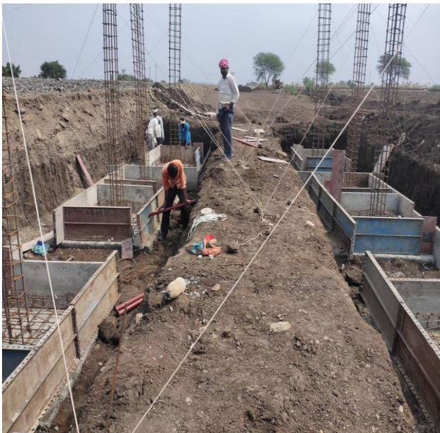
Toilet Block Foundation at Ch- 102+200
