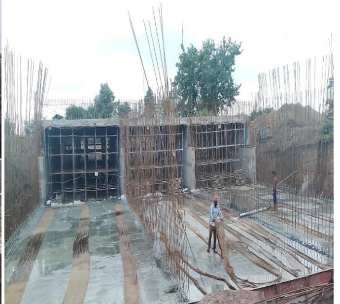
MNB RHS Raft Curing WIP at Ch- 104+251
