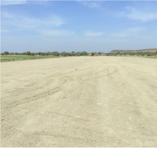
Sub Grade Top at Ch- 128+700 to 128+750
