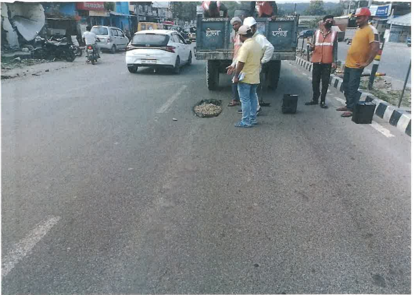
Patch Work is Going on
