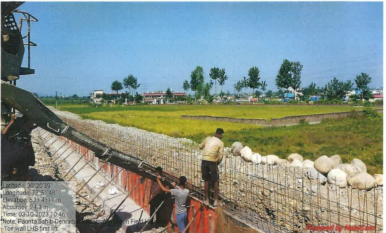
Toe Wall Concreting Work in Progress at Ch. 29+900
