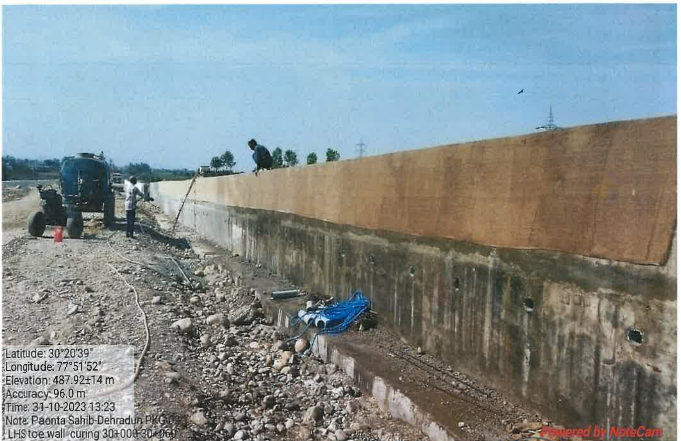
Toe Wall Curing Work in Progress at Ch. 30+030
