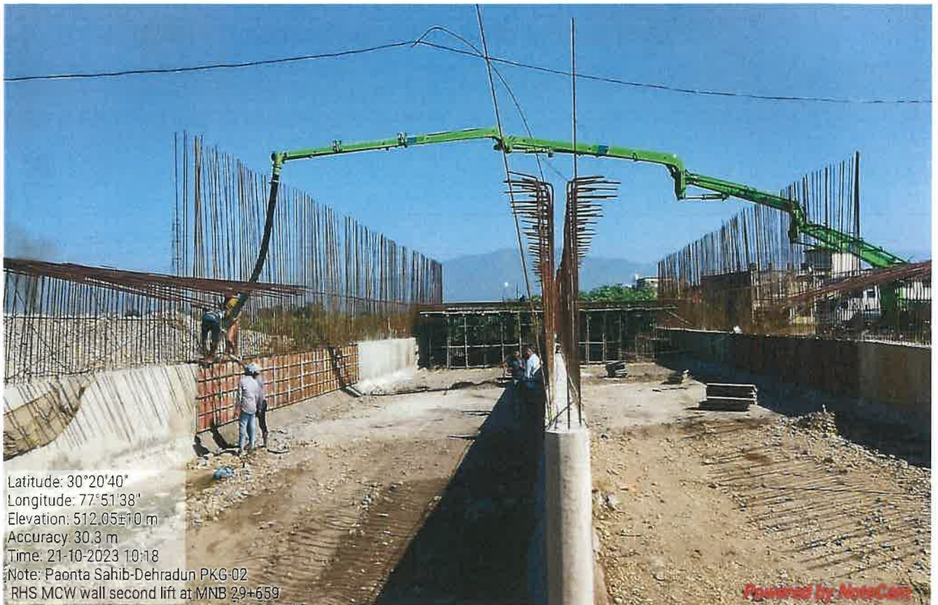
MNB Wall Concrete Pouring Work in Progress at Ch. 29+659
