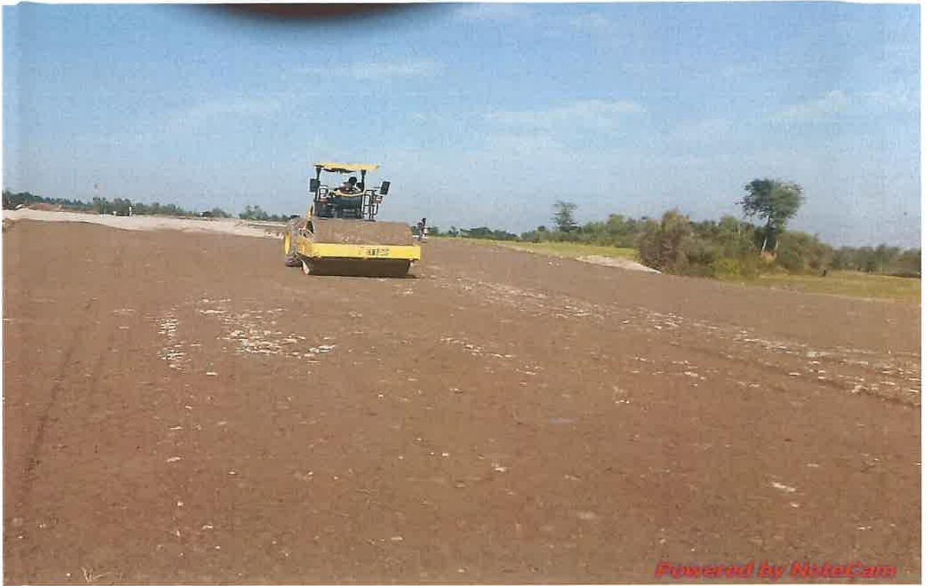
EMB Rolling Work in Progress at Ch. 19+800
