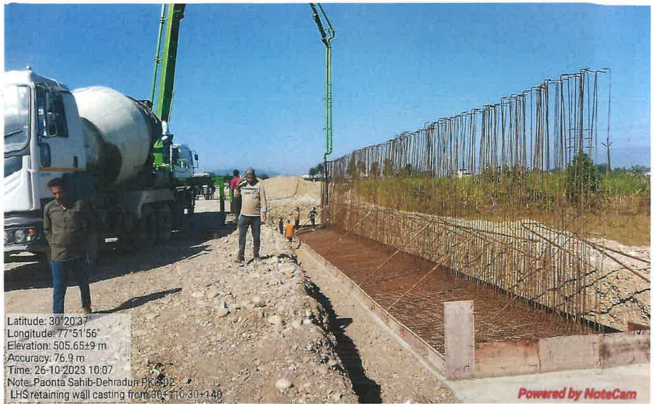
Retaining Wall Raft Concreting Work in Progress at Ch. 30+110
