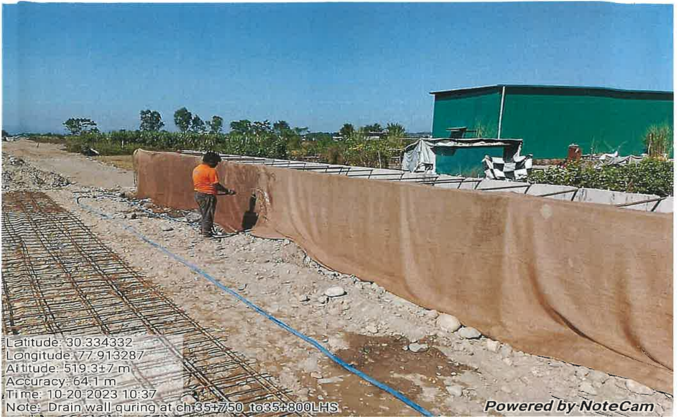
Drain Wall Curing work in Progress at Ch. 35+750
