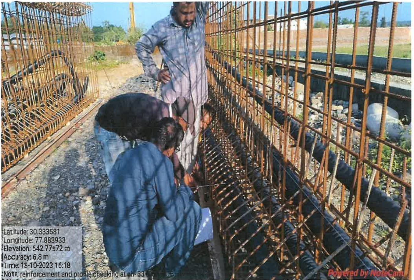
Girder Reinforcement & Profile Checking of MJB at Ch. 33+033
