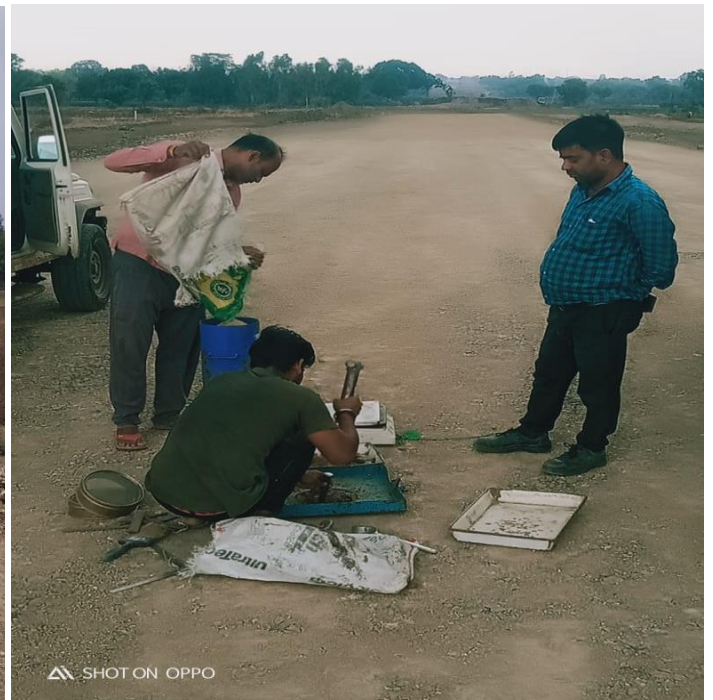
Sub Grade Top FDD Checking at Ch-129+800
