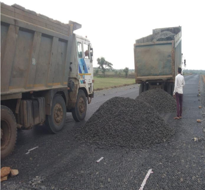
WMM DUMPING at Ch- 115+260 TO 115+480
