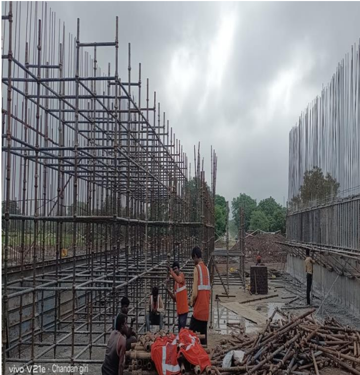
Staging WIP at Ch- 94+058
