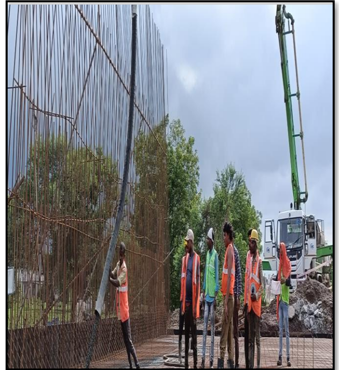
VUP Raft Concrete Pouring at Ch- 95+058
