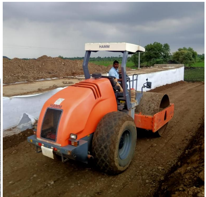
Backfilling at Ch- 122+350 (BHS)
