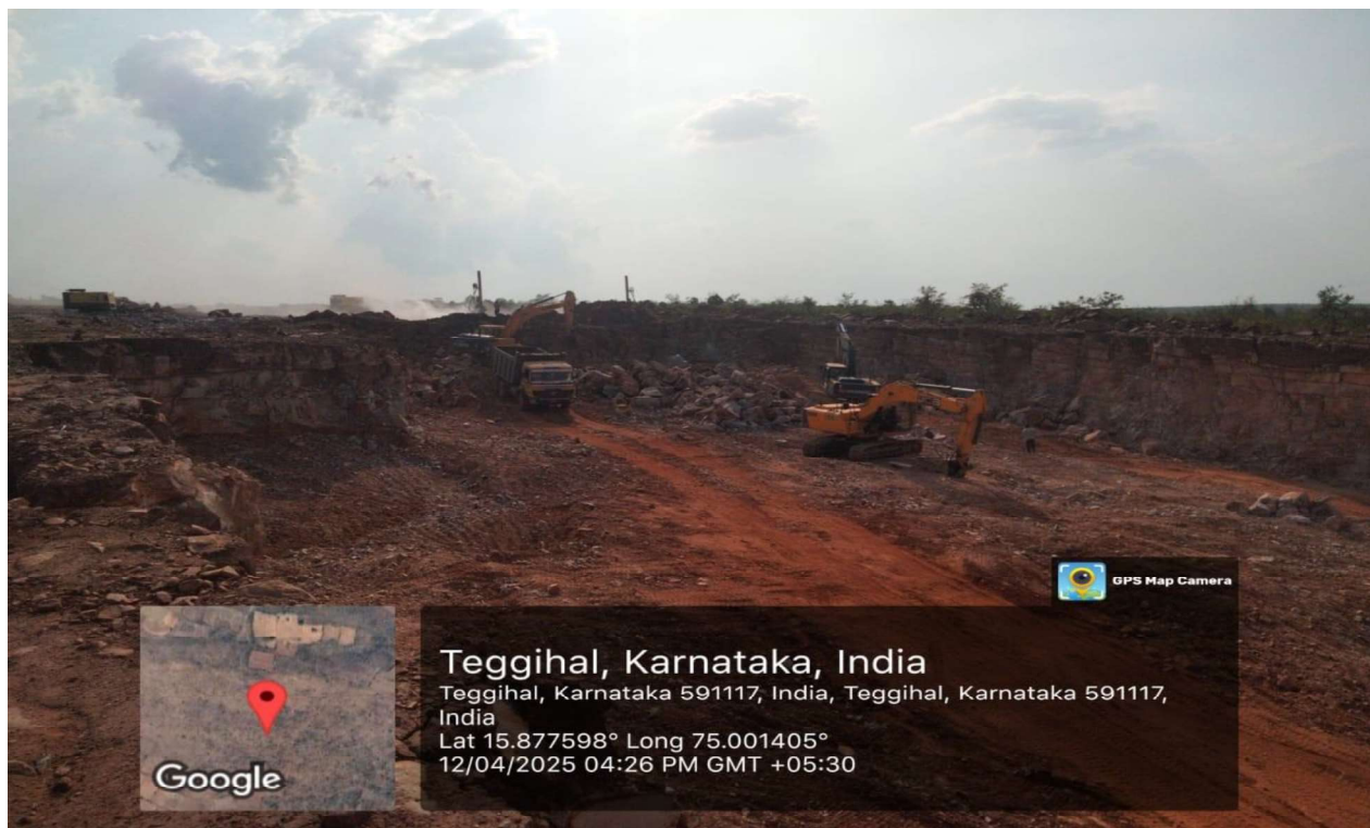
Plate 8 MCW Hard rock excavation work in progress at chainage 46+900
