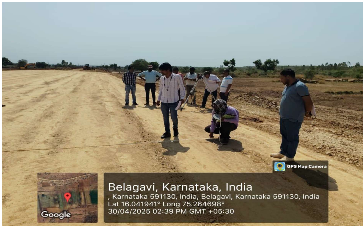
Plate 3 Joint Site Inspection along with IE In progress at Chainage 82+000
