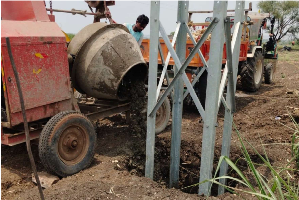
Plate 5 Tower Foundation Casting work in Progress at Chainage 60+800
