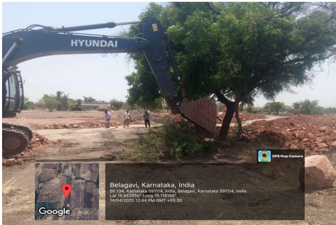
Plate 6 tree felling in progress at Chainage 54+200
