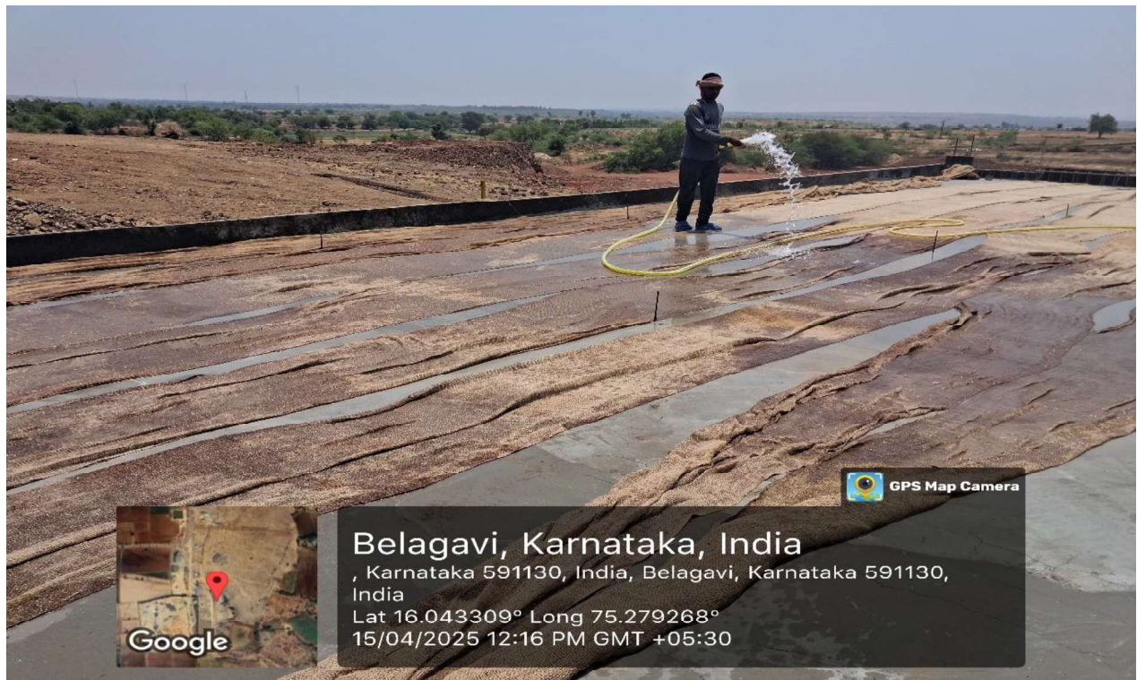
Plate 9 Box Culvert Slab curing work in Progress at Ch. 83+570
