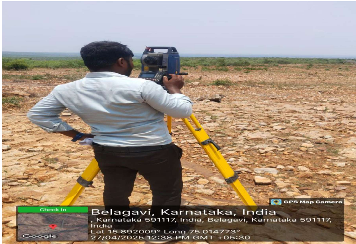
Plate 1 RoW layout marking in progress at chainage 49+500
