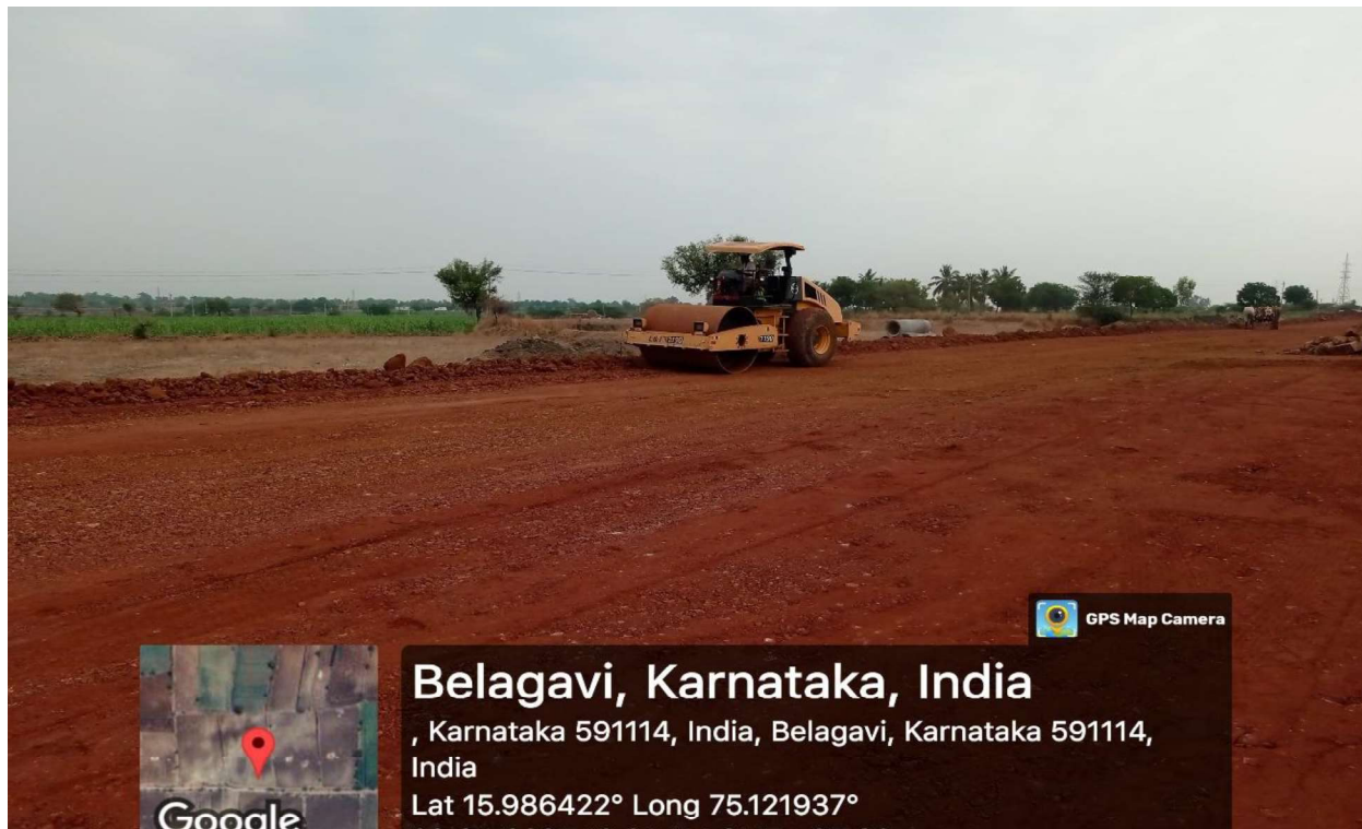
Plate 7 Embankment 2 nd layer Compaction work in progress at Chainage 65+800
