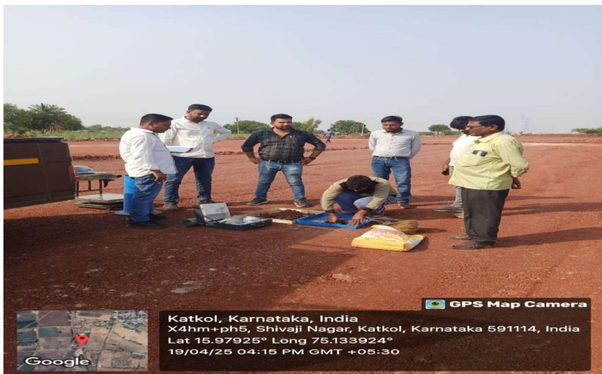
Plate 4 Earth Work Compaction Testin in Progress at Chainage 65+050
