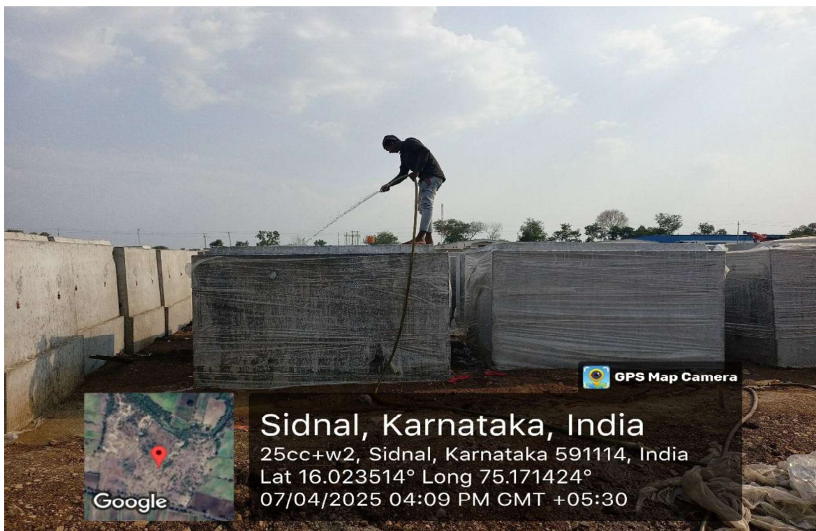
Plate 2 Pre-cast Box Culvert Segment Curing in Progress at Base Camp Casting Yard
