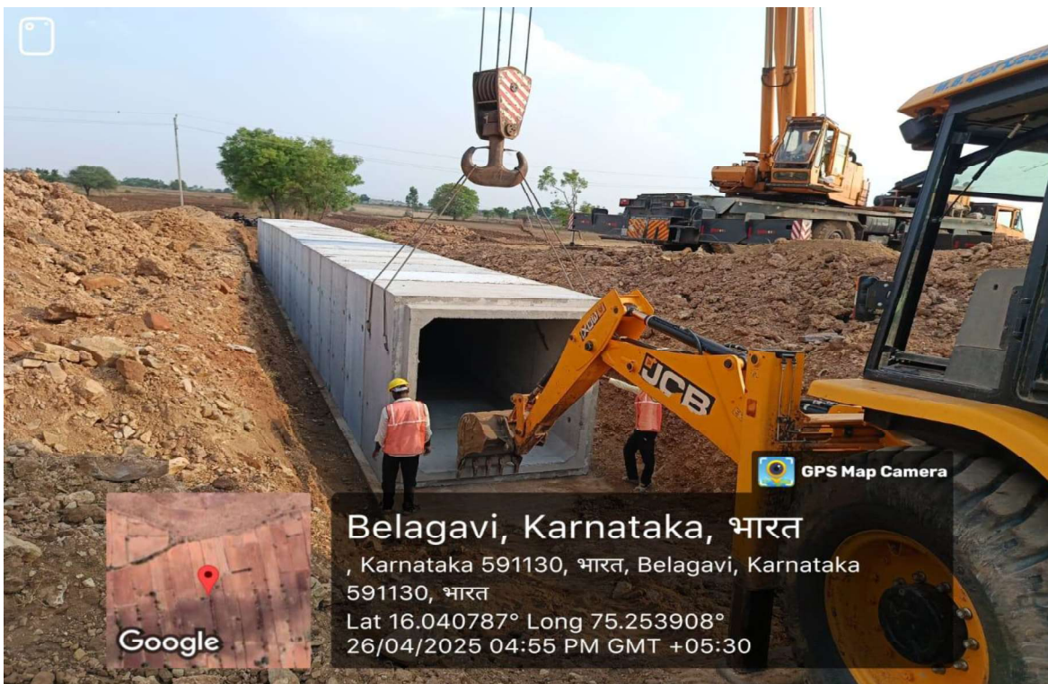
Plate 12 Pre-cast Box Culvert segment erection in progress at Ch. 80+235
