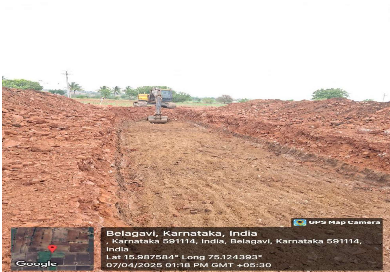
Plate 10 Box Culvert foundation Excavation work in Progress at Ch. 80 +300
