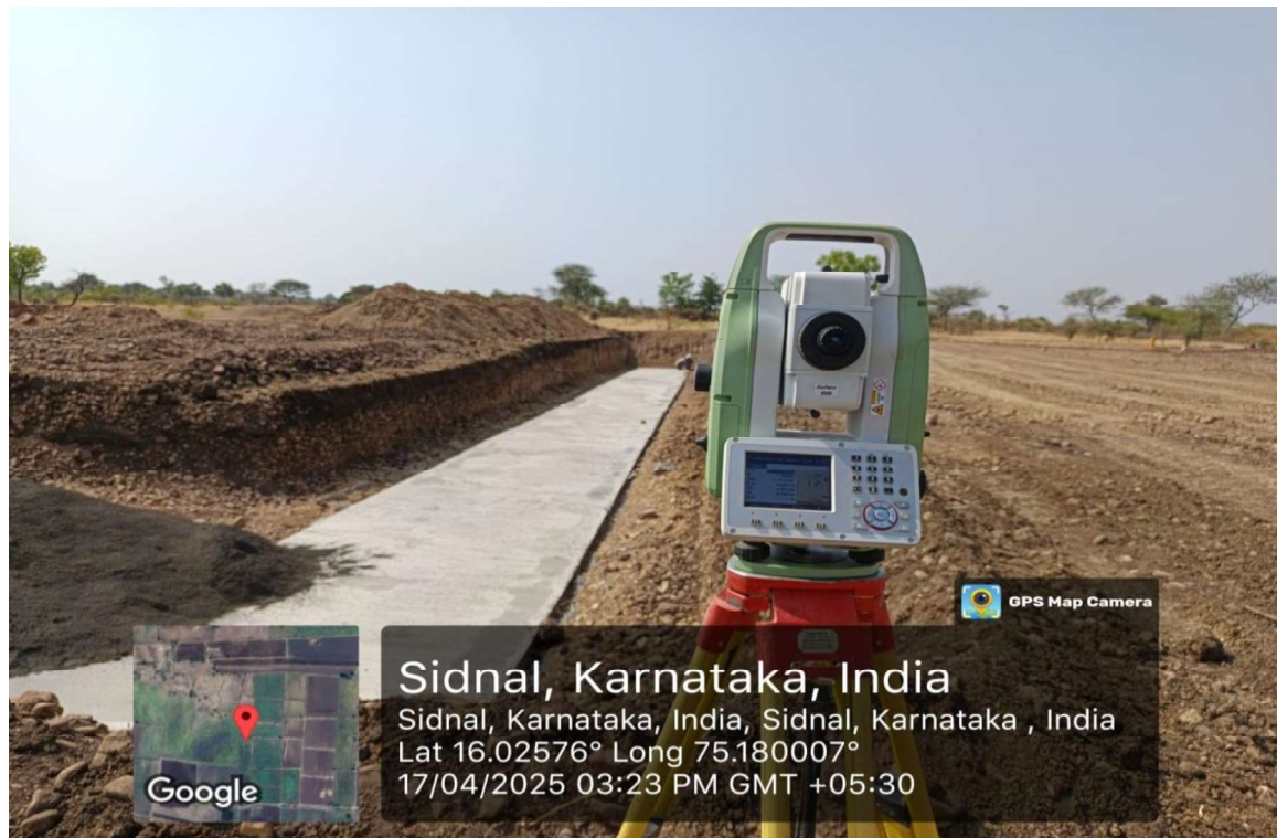
Plate 13 Pre-cast Box Culvert segment erection layout in progress at Chainage 71+800
