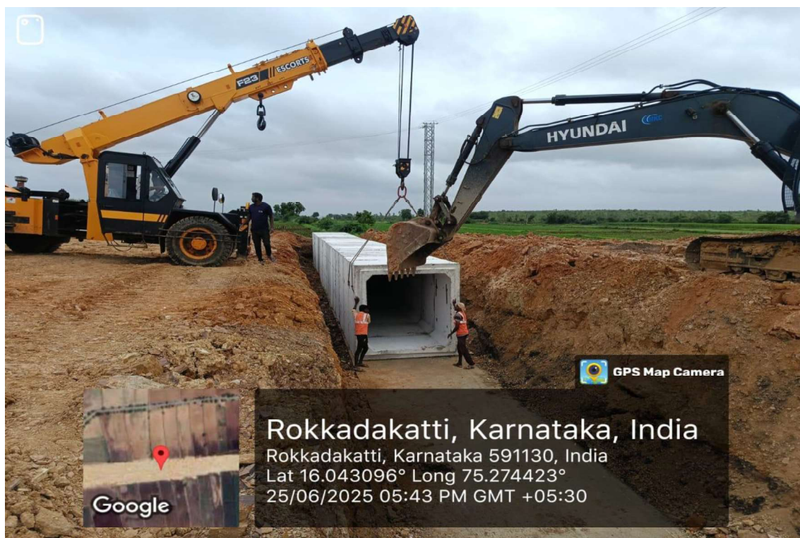
Plate 5 Pre-cast Box Culvert Segment Erection Work in Progress at Ch. 83+052
