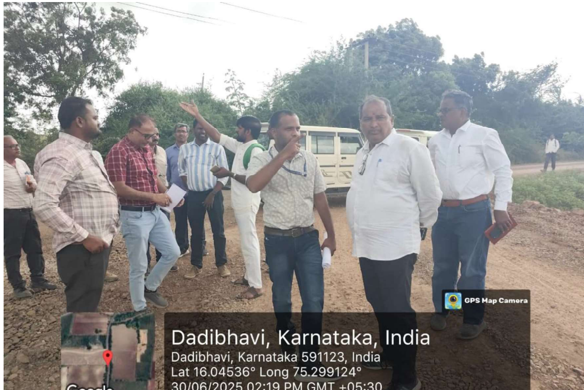
Plate 8 Monthly Site Inspection in Progress at Ch. 77+900
