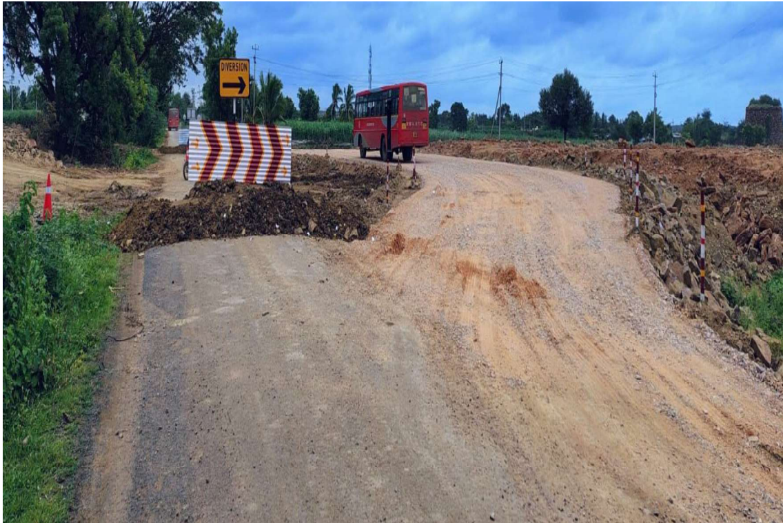
Plate 6 Diversion Work in Progress for Constructing LVUP at Ch. 78+700
