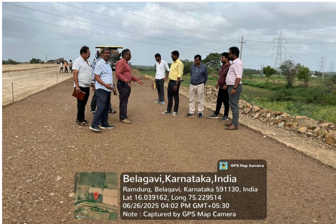
Plate 5 CTSB Laying Work in Progress at Ch. 78+700
