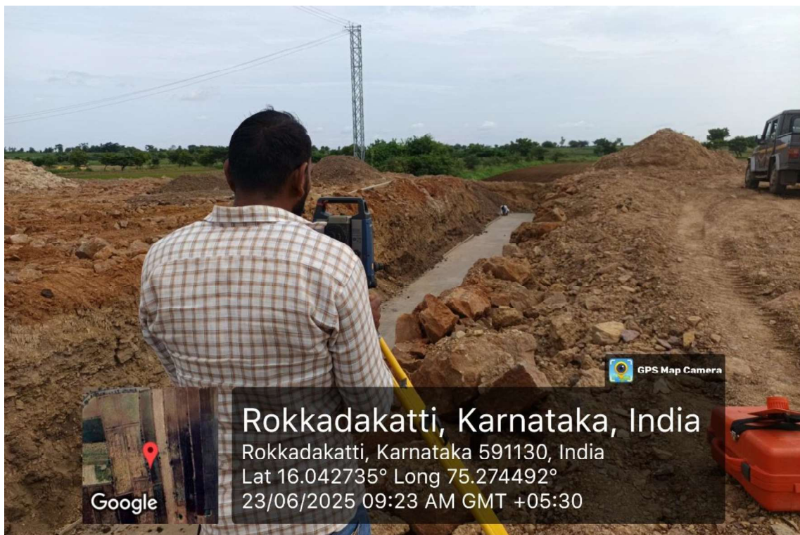
Plate 2 Pre-cast Box Culvert Segment Erection layout work in Progress at Ch. 83+052
