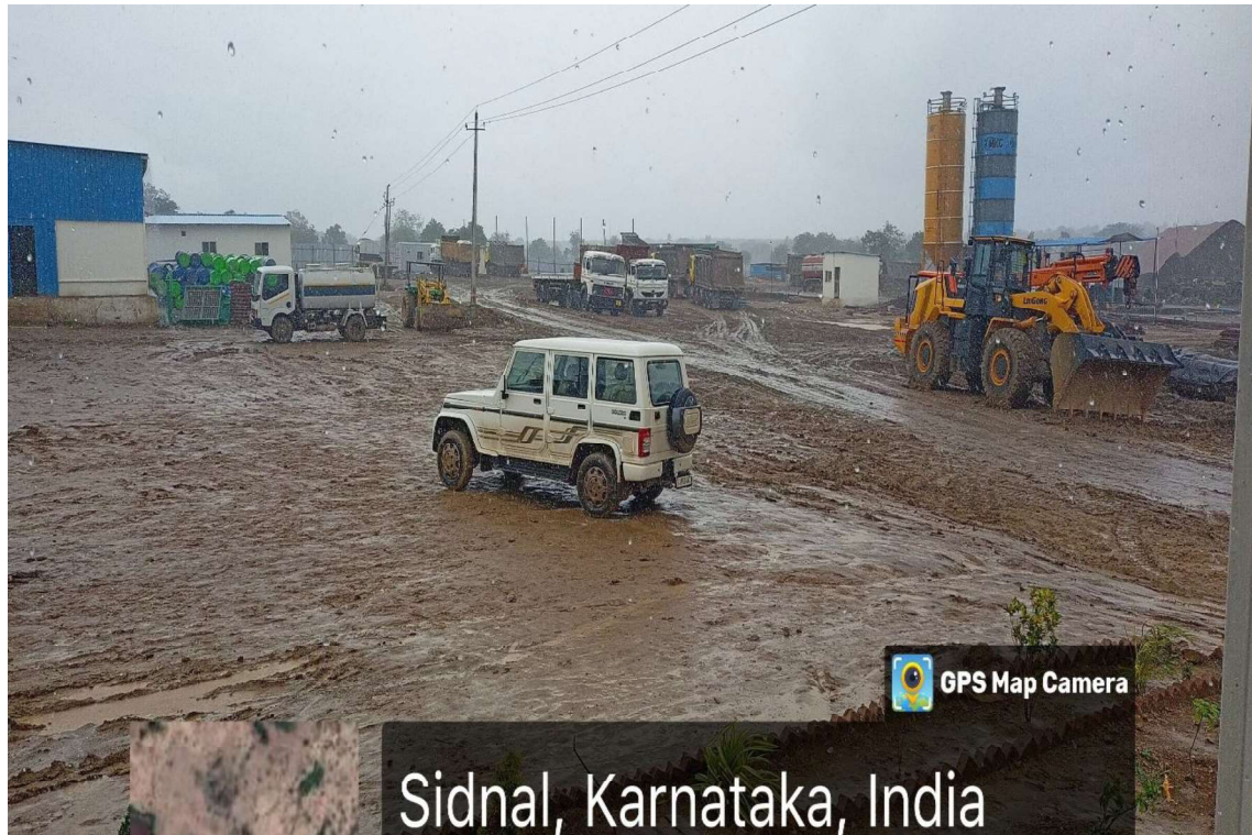
Plate 12 Rain Affecting pre-cast Construction Work at Base Camp
