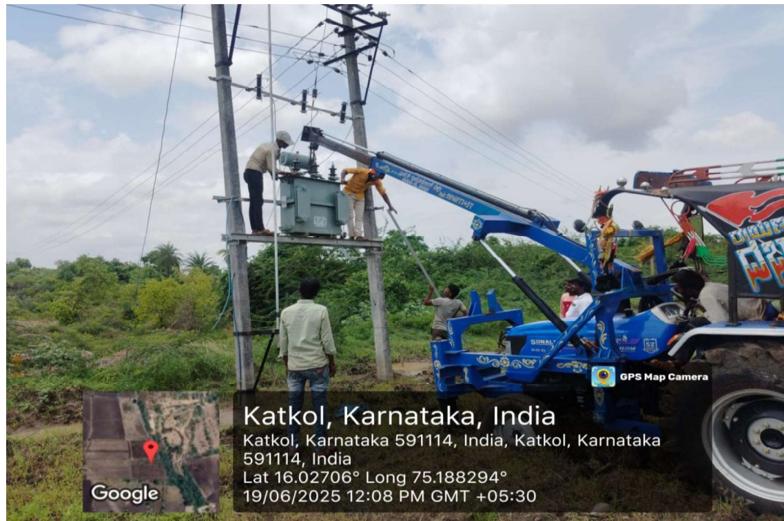
Plate 3 Electrical Utility Work DTC installation Work in Progress at Ch. 73+370
