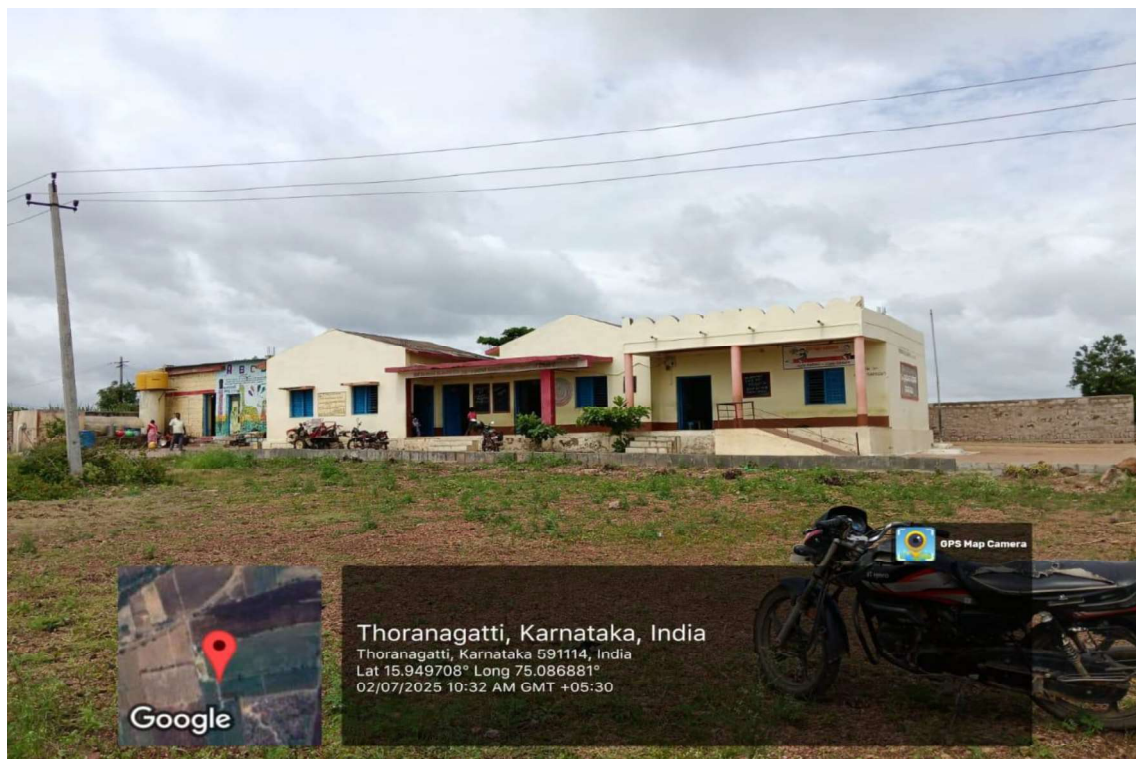
Plate 16 Village School Lies with in Row at Ch. 59+300
