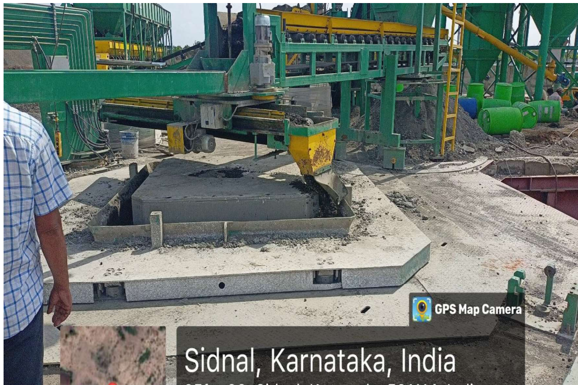
Plate 11 Pre-cast Box Culvert Segment Casting Work in Progress at Base Camp
