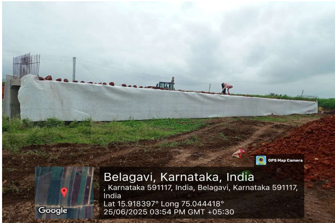
Plate 10 Geo-composite fixing Work in Progress at Ch. 53+550
