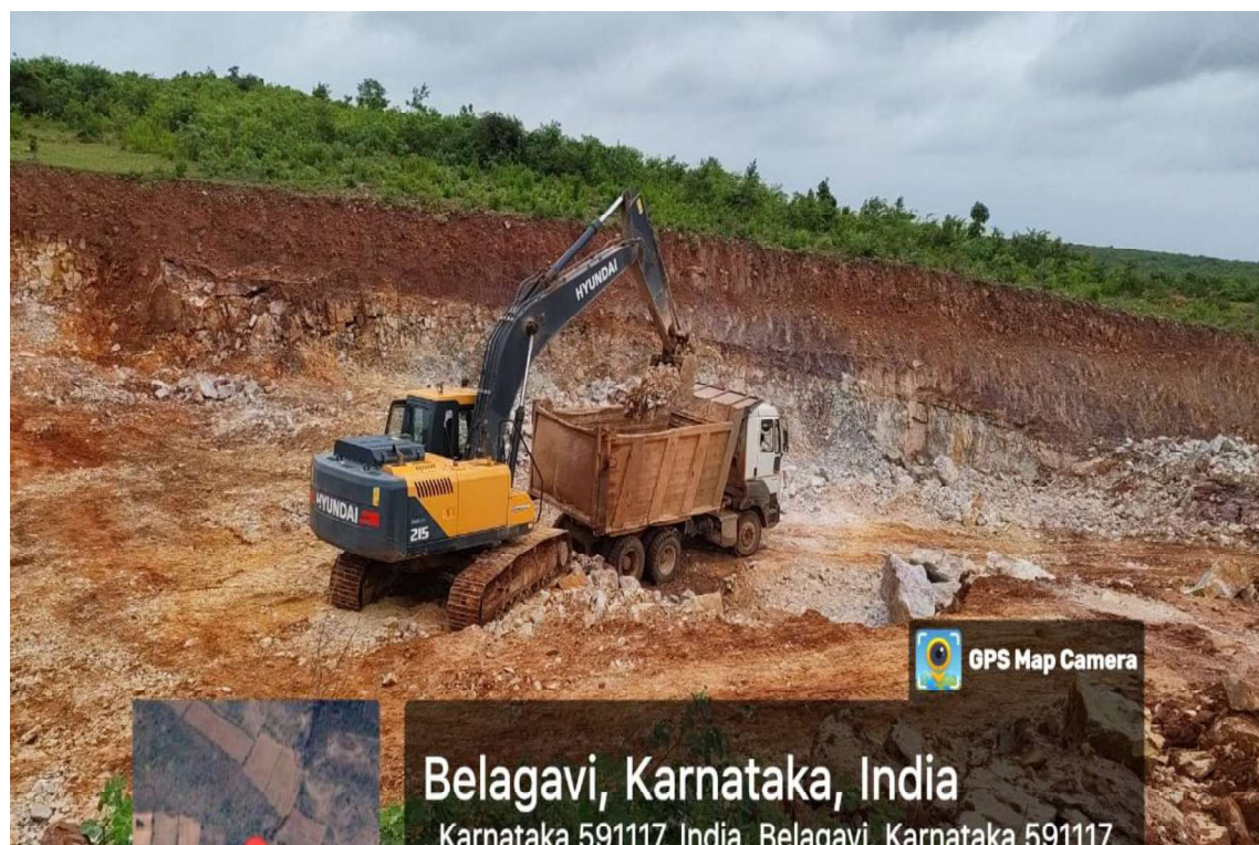
Plate 4 Main Carriageway Hard Rock Excavation Work in Progress at Ch. 47+250
