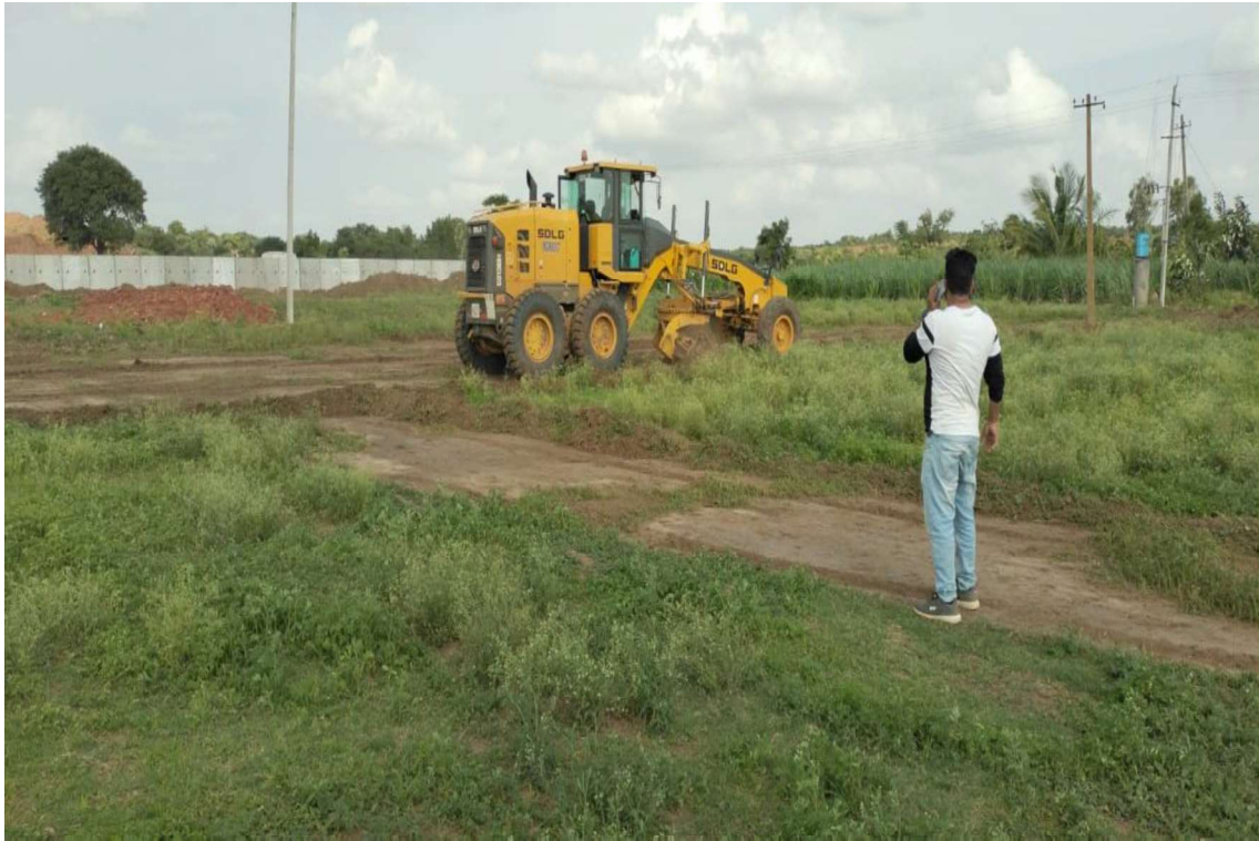
Plate 1 C & G Work in Progress at Ch. 79+300
