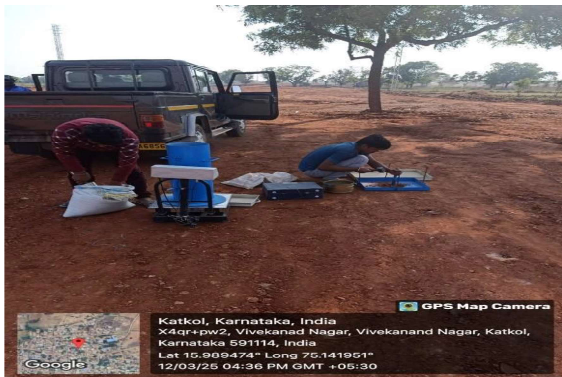
Plate 6 Field Dry Density Checking at Ch. 66+800
