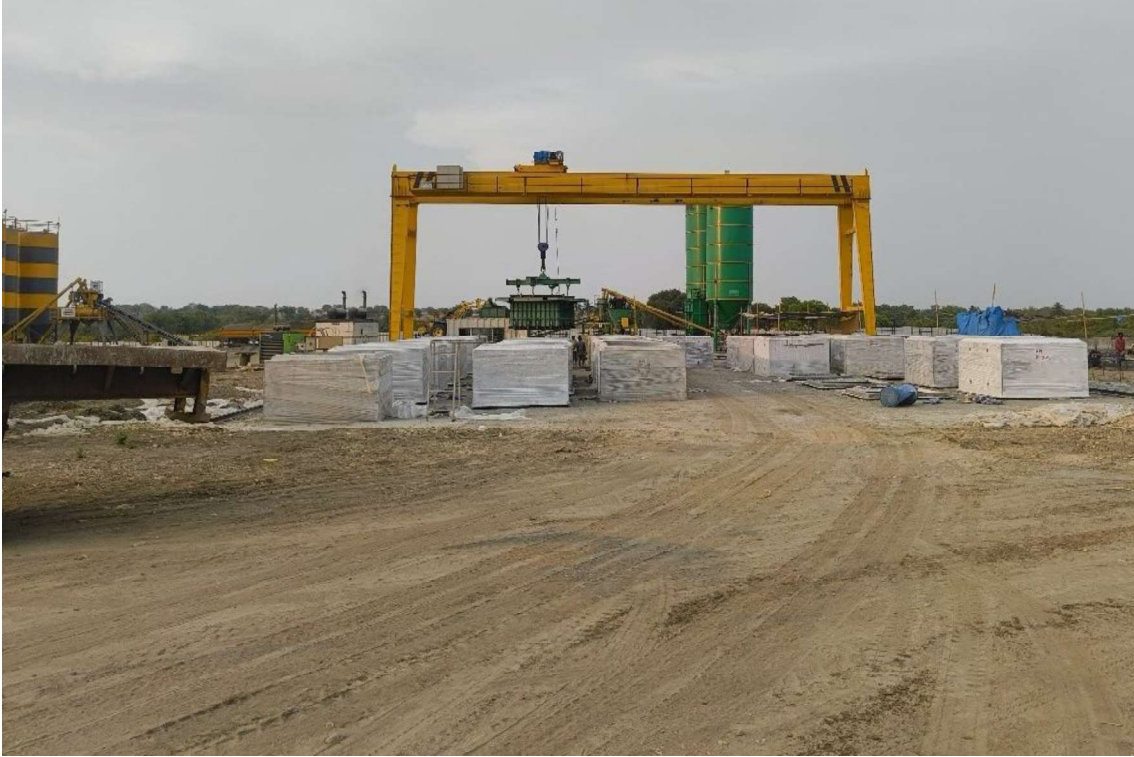
Plate 7 Pre-cast Box Culvert Segment Casting Unit
