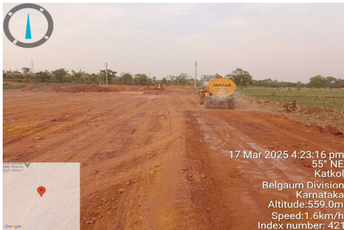
Plate 10 Embankment 3 rd Layer Soil Filling in Progress at Ch. 65+200
