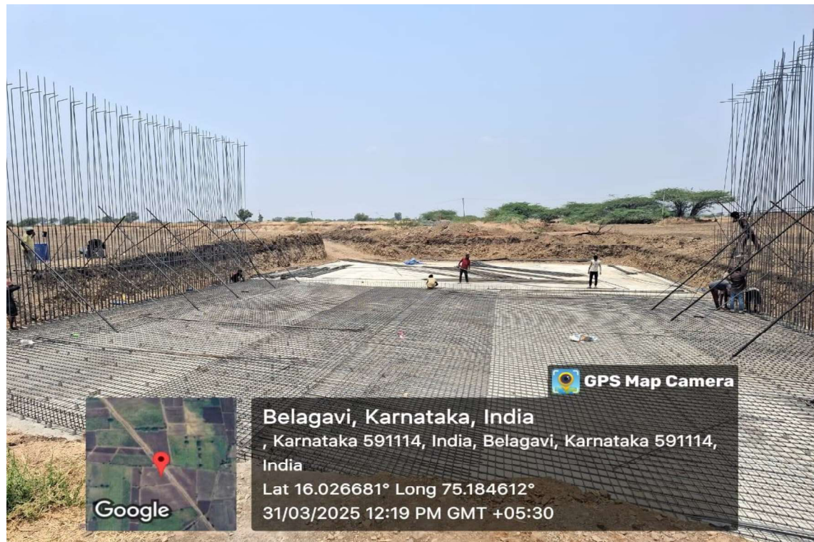
Plate 9 Reinforcement Binding for MNB Raft at Ch. 72+969
