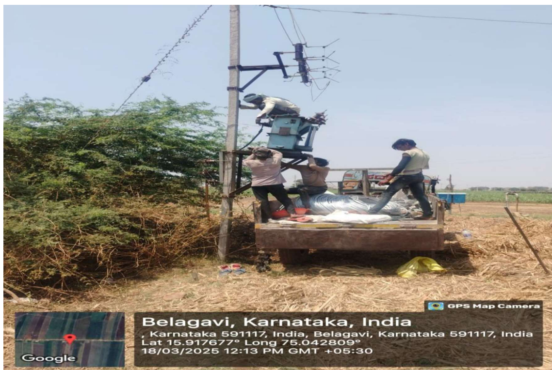
Plate 12 Utility Shifting at Ch. 65+400
