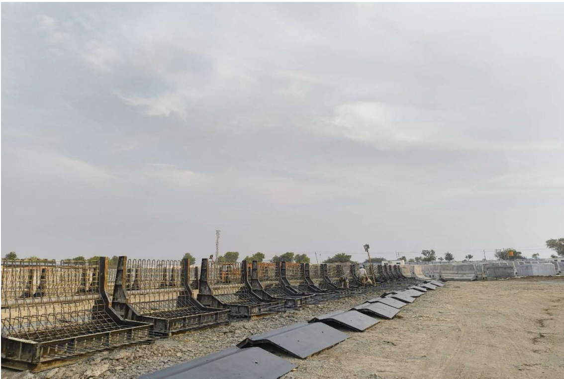
Plate 8 Pre-cast Friction Slab with Crash Barrier Casting
