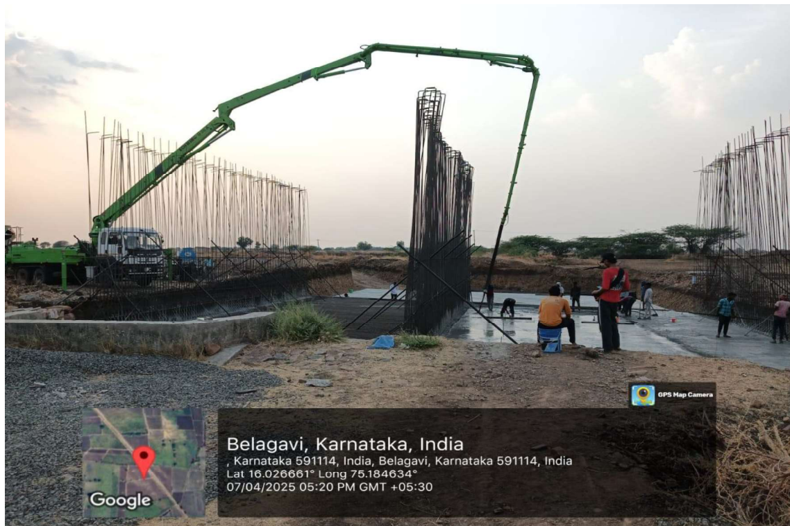
Plate 11 MNB RHS Raft Concrete Pouring at Ch.72+969
