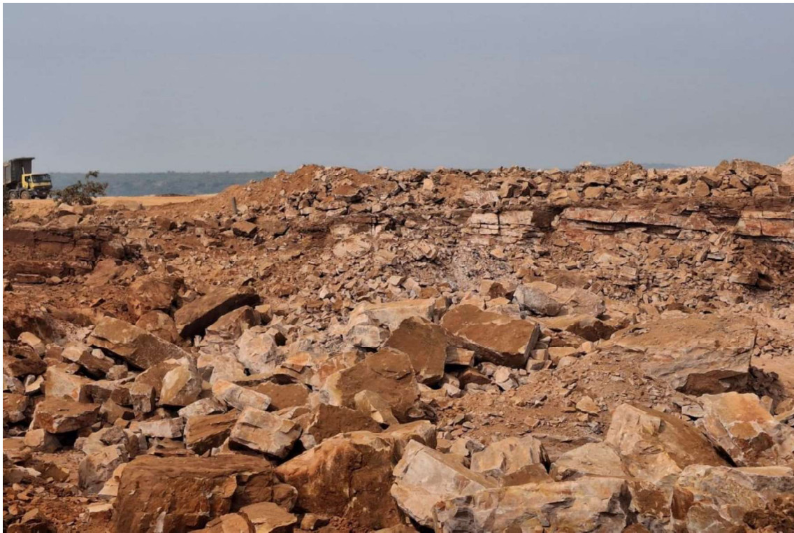
Plate 4 Main Carriageway Hard Rock Excavation at Ch. 46+900
