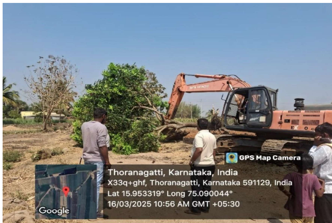
Plate 2 Tree Cutting at Ch. 54+250
