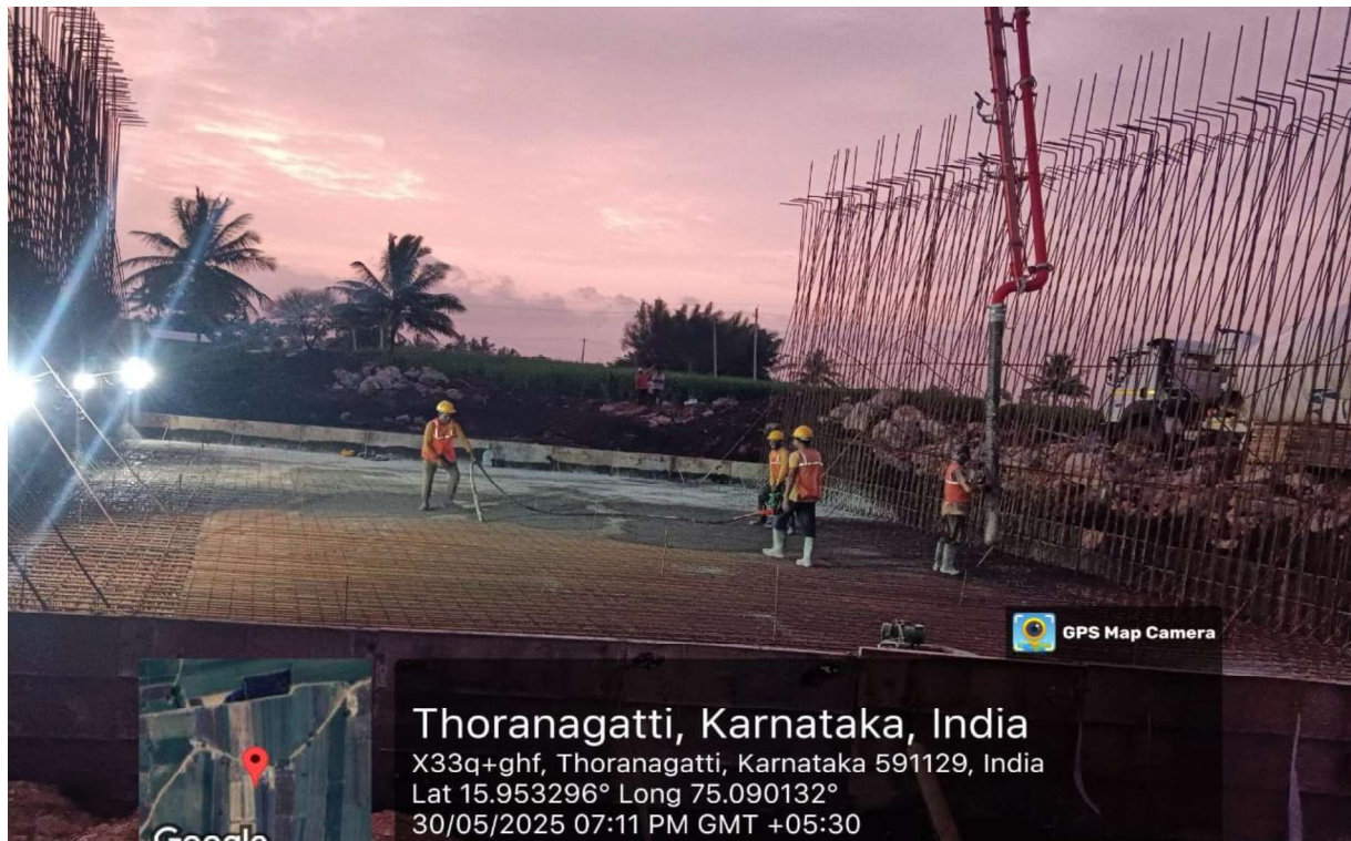
Plate 5 LVUP Foundation Casting Work in Progress at Ch. 59+827
