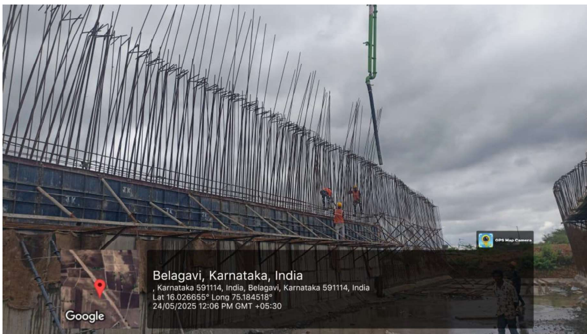
Plate 2 MNB Sub-Structure 3 rd Lift Casting work in progress at Ch. 72+969
