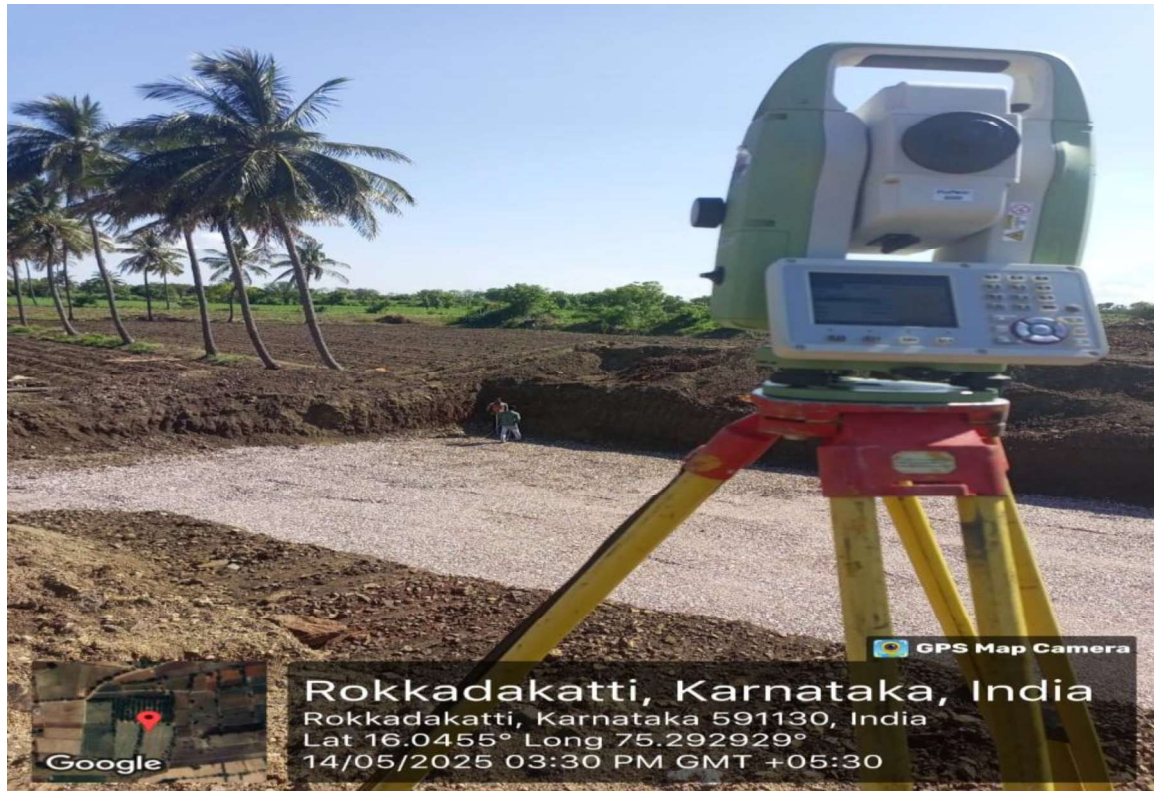
Plate 1 MNB Foundation PCC layout marking in progress at Ch. 85+026
