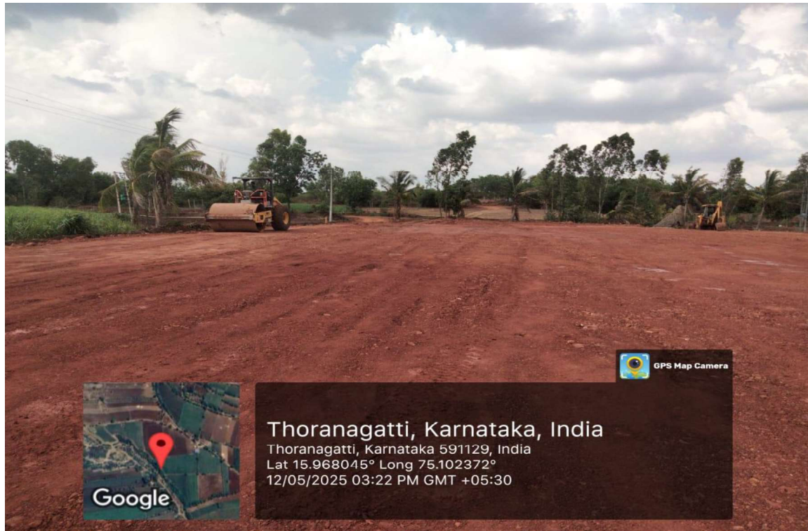
Plate 13 Embankment Layer Compaction Work in Progress at Ch. 61+900
