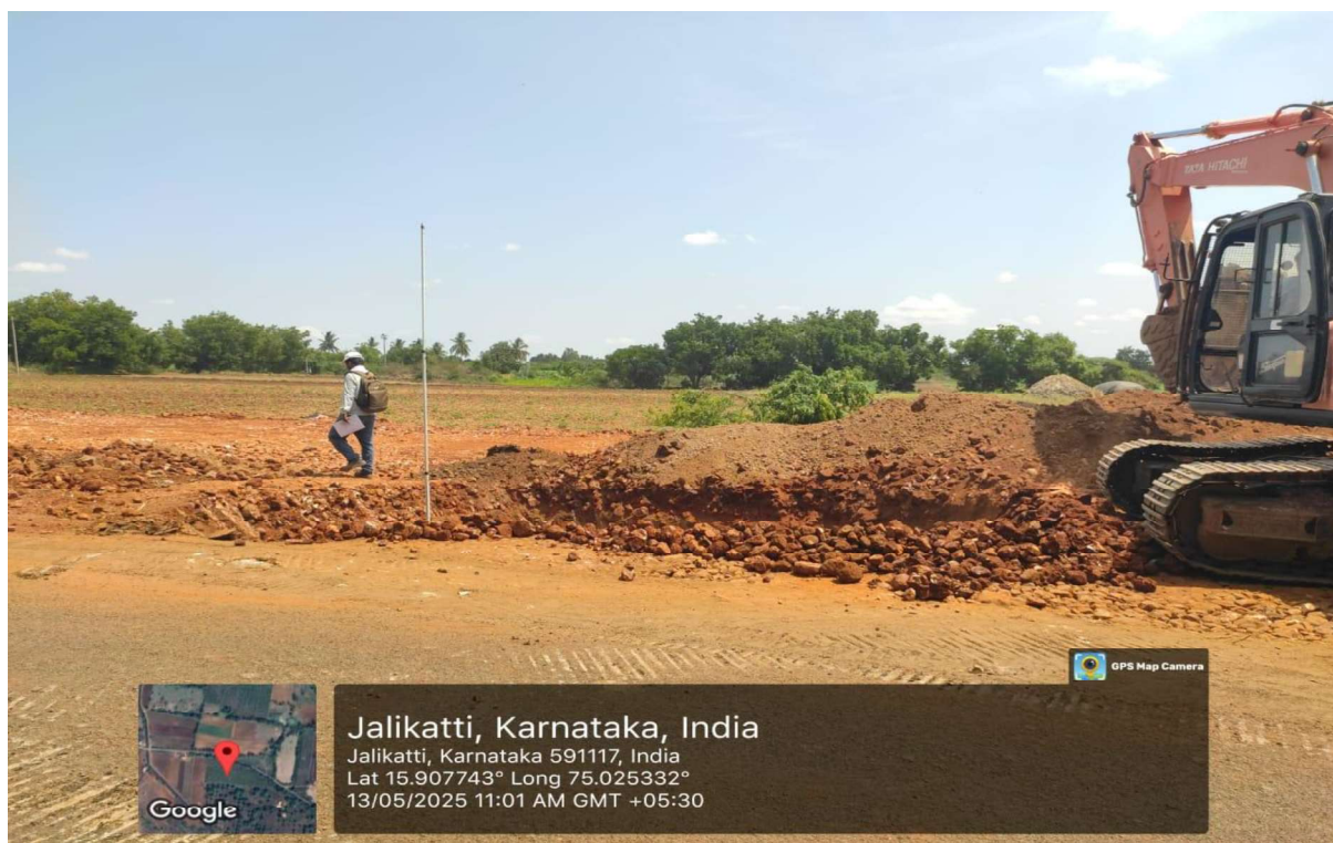
Plate 6 Excavation for LVUP Foundation in Progress at Ch. 51+200
