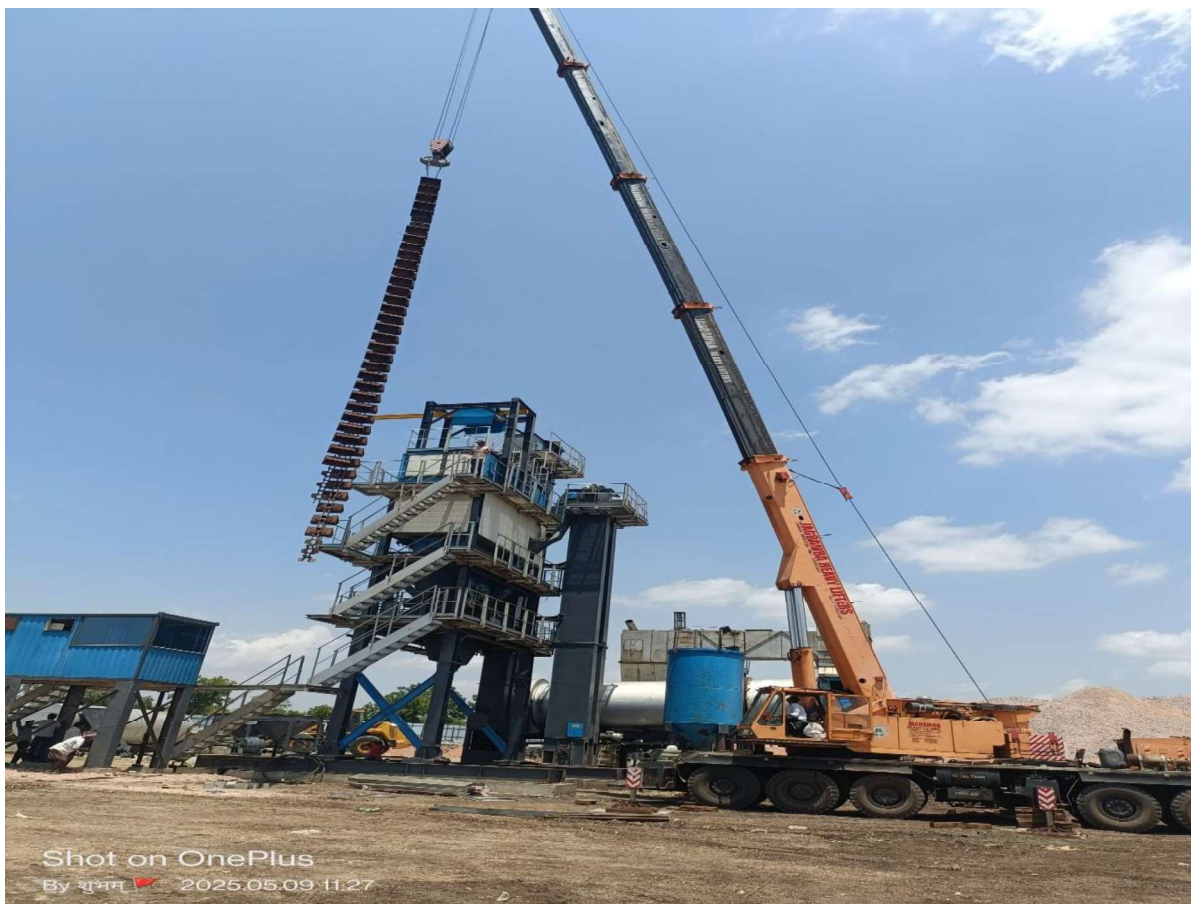
Plate 14 HM Plant Work in Progress at Base Camp
