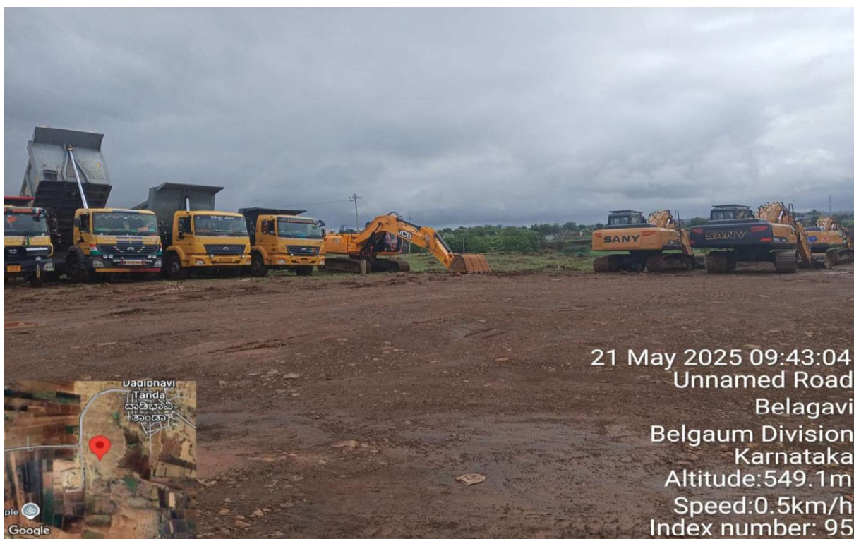
Plate 12 Highway Work Getting Hindered due to Heavy Rain & Bad Weather at Ch. 67+500
