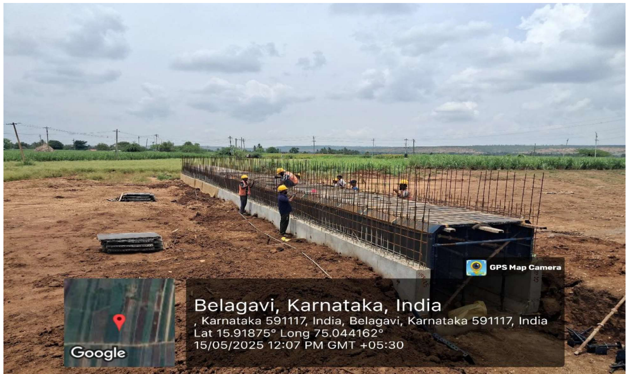
Plate 9 Box Culvert Slab Reinforcement Work in Progress at Ch. 53+532
