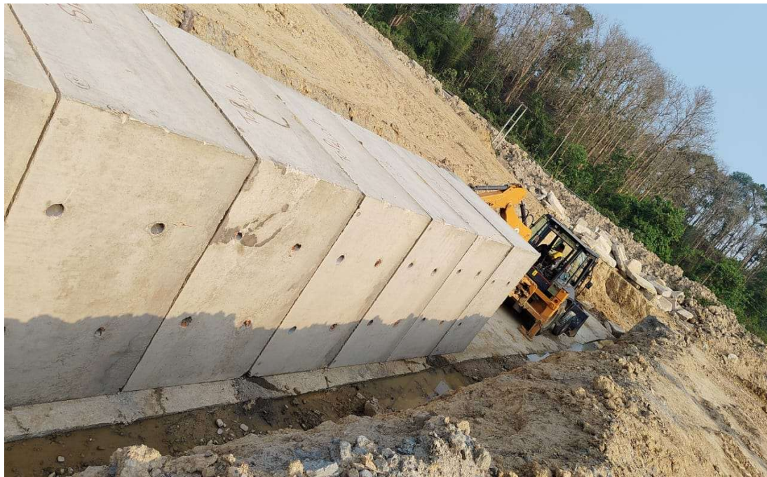
Pre-cast Box-Culvert Erection work at ch-101+535
