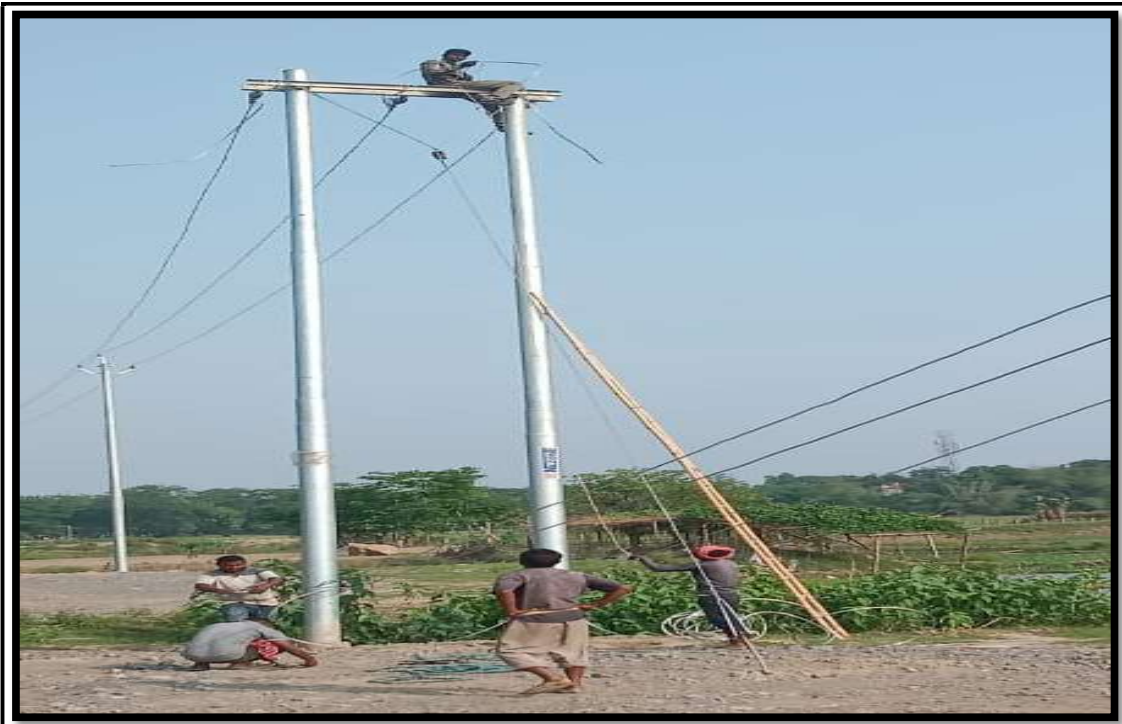
Electric Pole Shifting in progress
