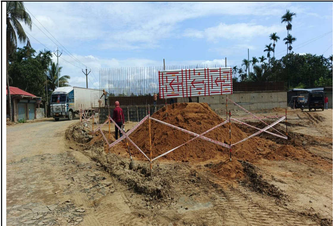
Diversion and Safety Barricading 92+250
