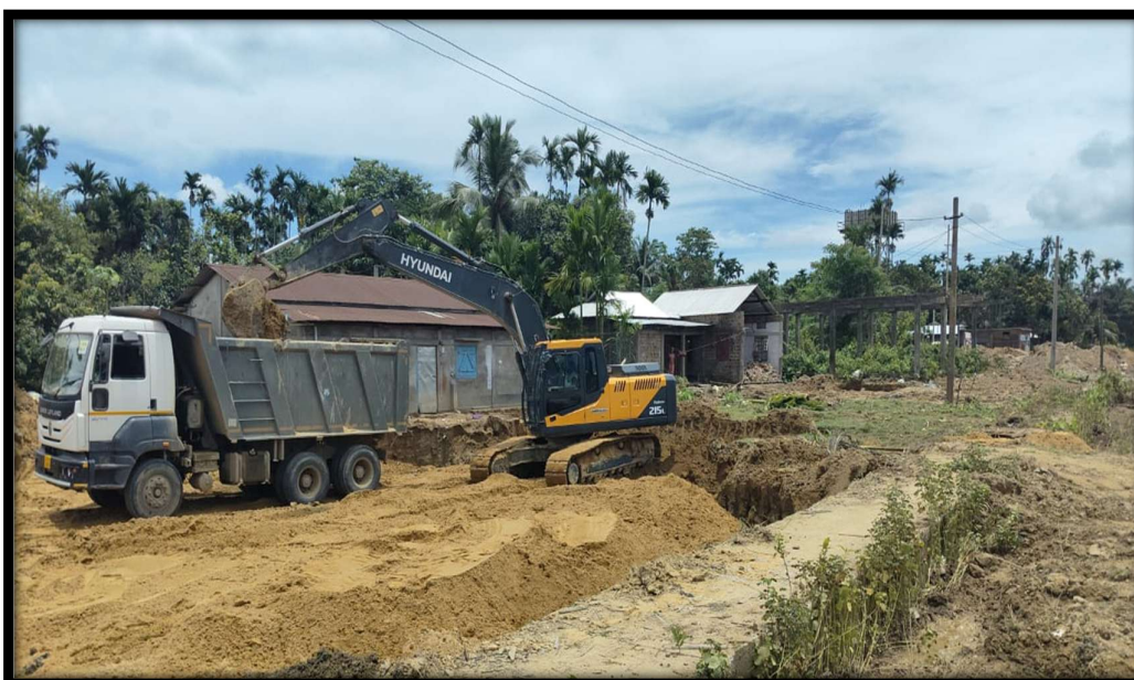
Unsuitable soil removing work at chainage-192+180
