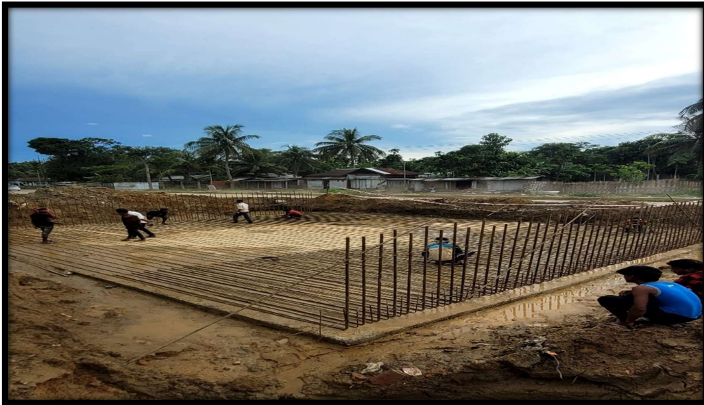
Reinforcement Placing at chainage 92+248 (LVUP)
