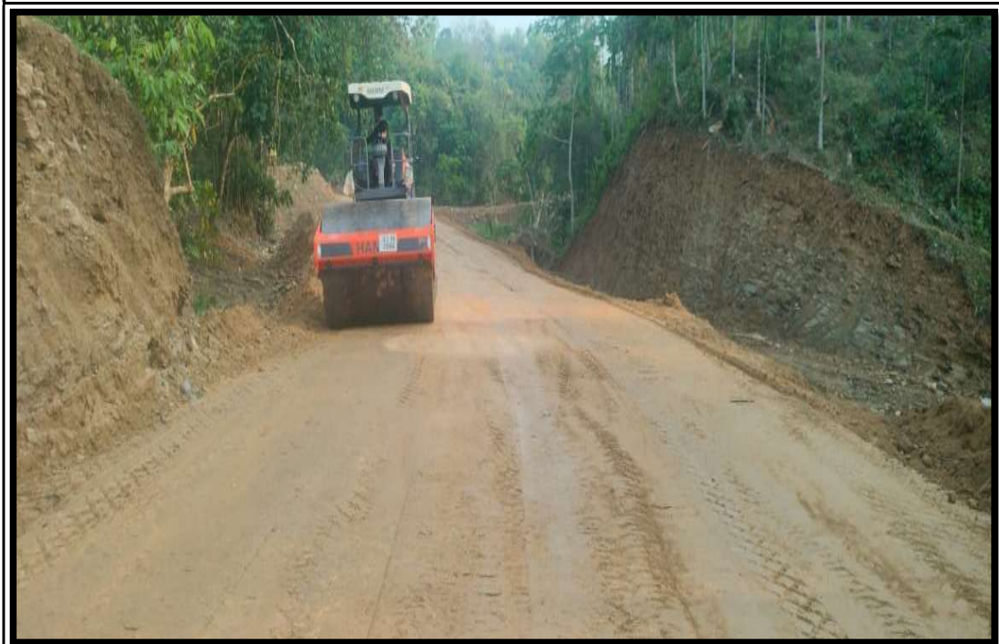
Rolling in progress in Embankment Layer (Ch. 4+350 to 4+520)
