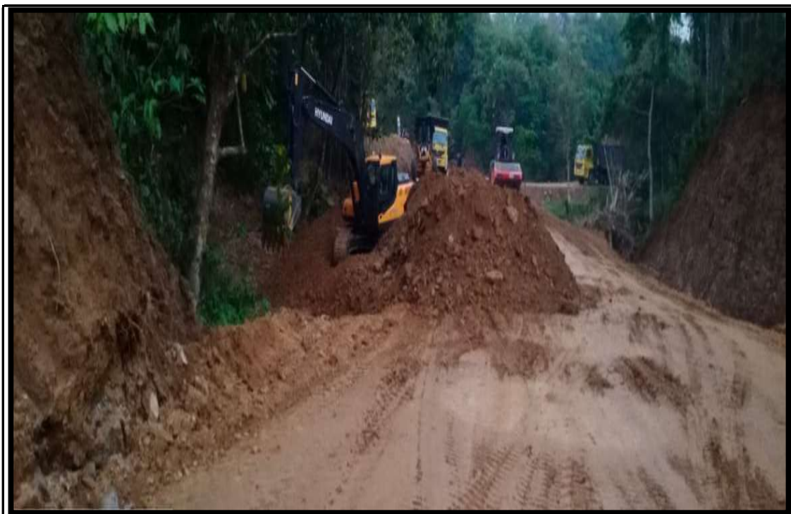
Soil Dumping in Embankment Layer (Ch. 4+450 to 4+500)
