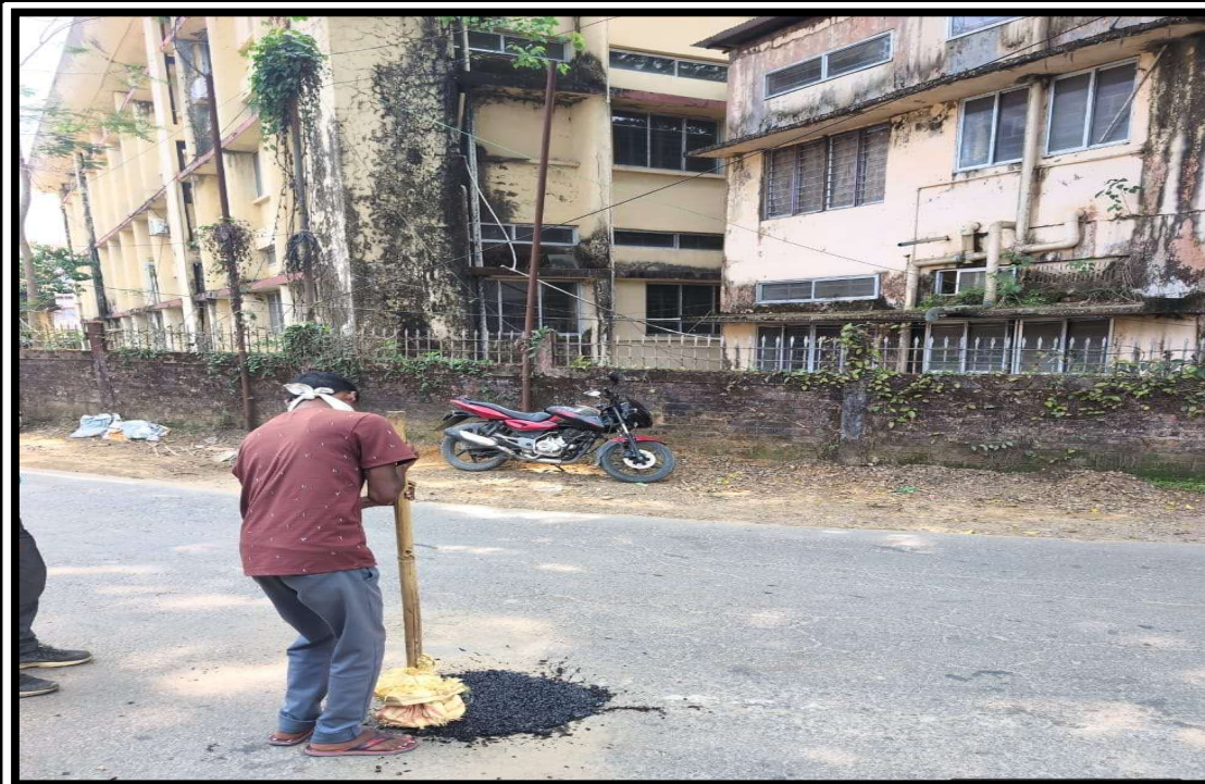
Pot Hole repair in progress
