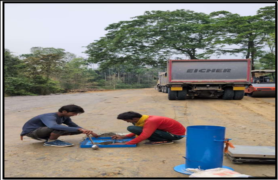
FDD Testing in Embankment Layer
