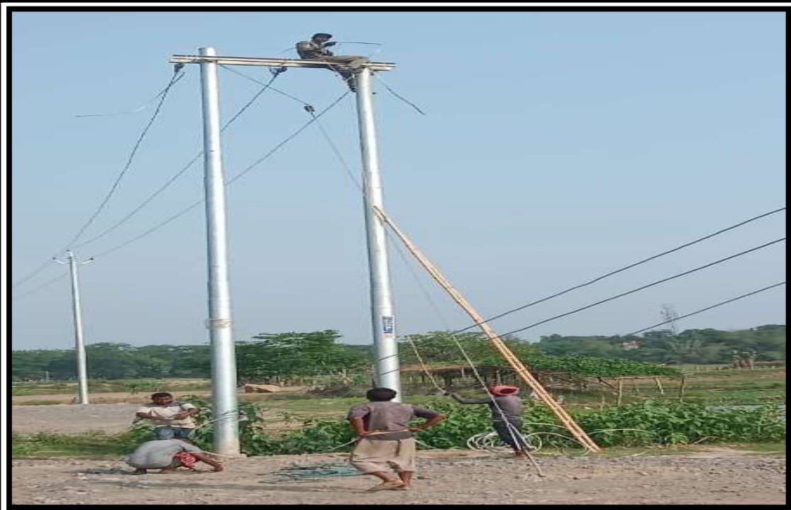
Electric Pole Shifting in progress
