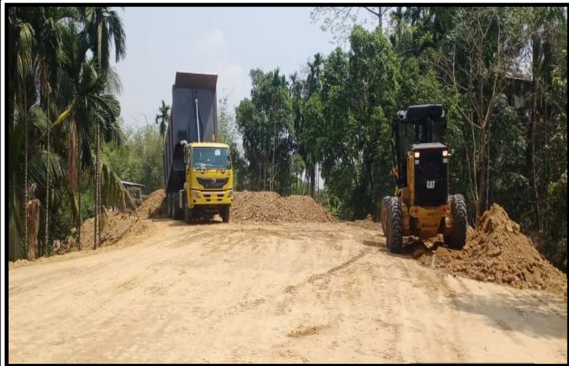
Soil Dumping in Embankment Layer in progress
