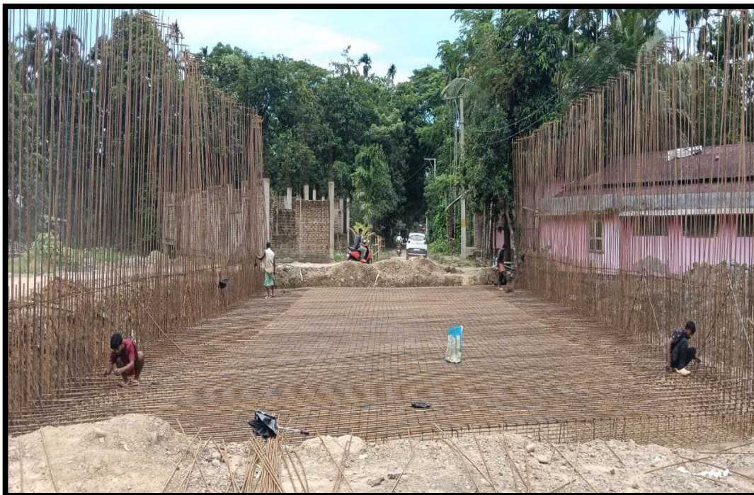
Concrete work in Progress for Raft Chng 04+212
