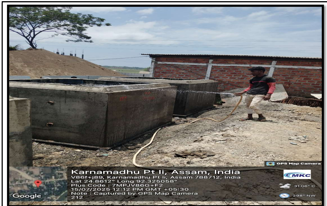
Box Culvert segment curing in Progress
