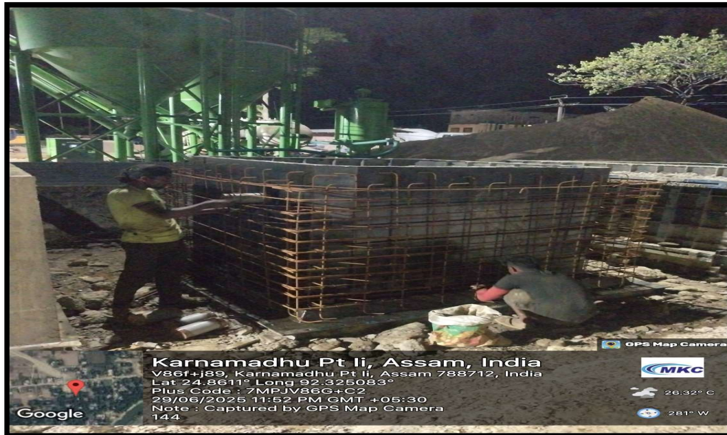
Reinforcement work in Progress for Box Culvert
