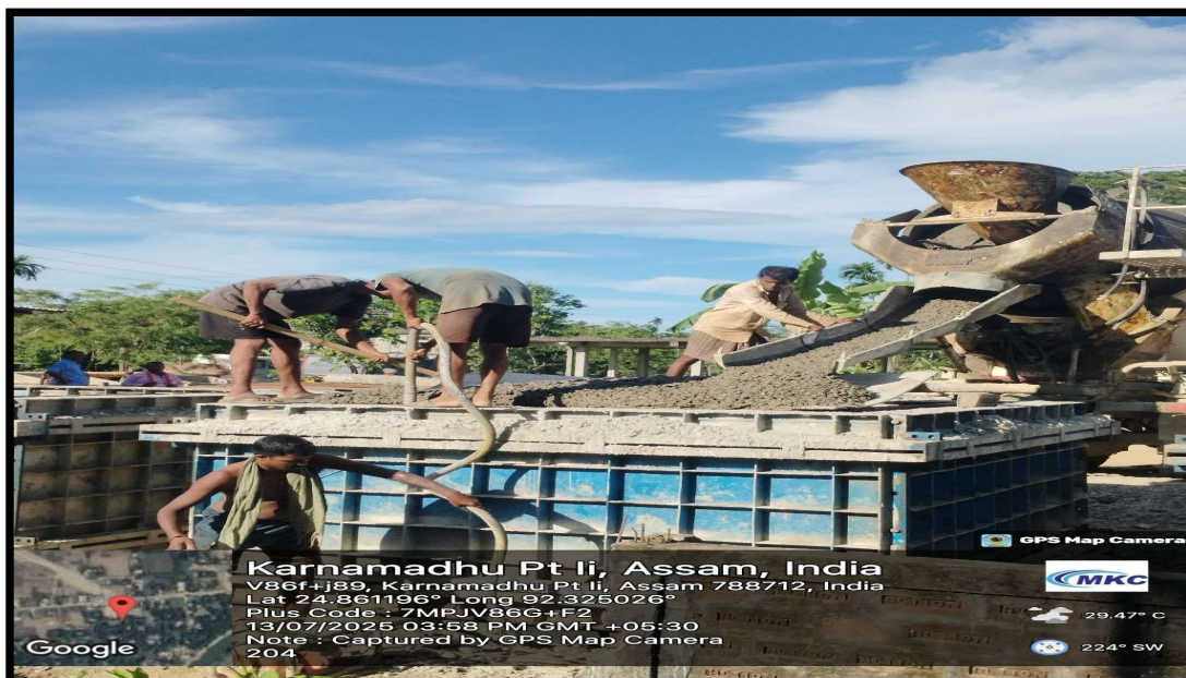
Concrete Pouring of Pre-cast Box-culvert Segment
