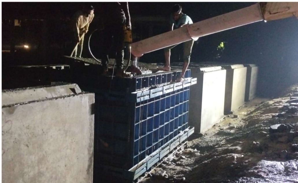
Concrete Pouring of Pre-cast Box-culvert Segment
