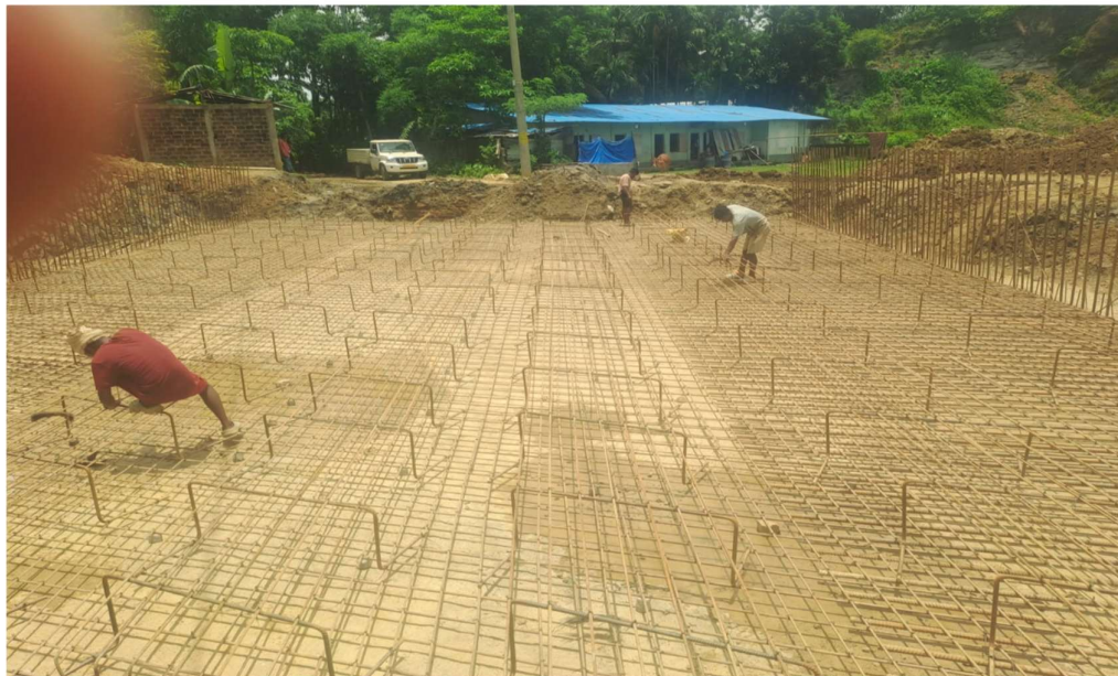
Reinforcement work in Progress at 4+212 (LVUP) BHS
