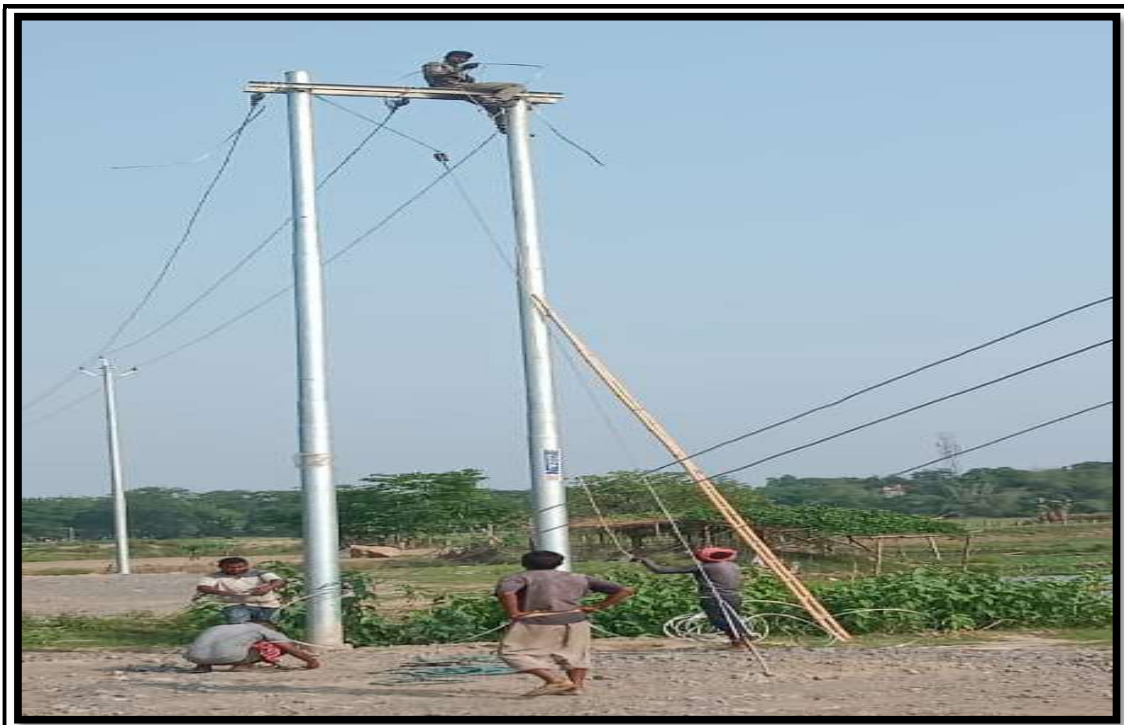
Electric Pole Shifting in progress
