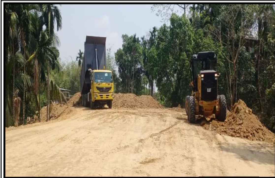
Soil Dumping in Embankment Layer in progress
