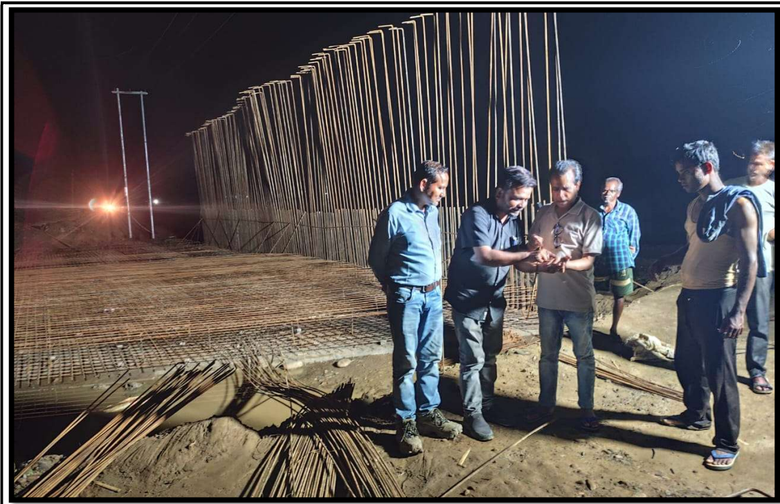
TL sir site visit at ch-10+098 (LVUP)
