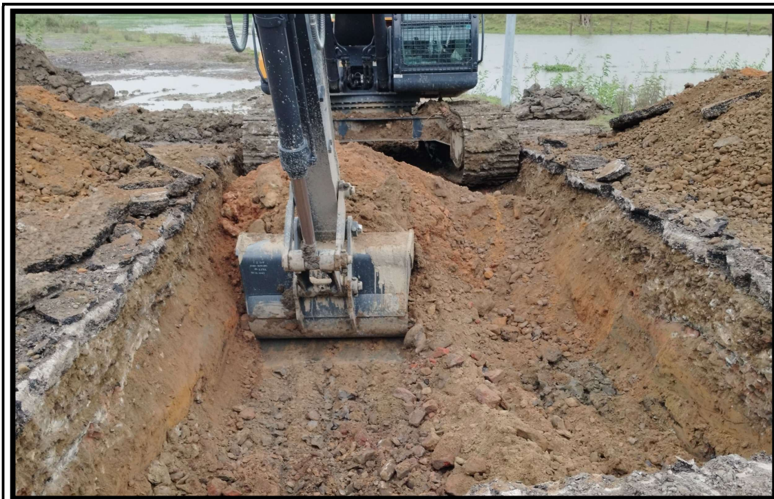
Box Culvert Excavation in Progress 13+065 LHS
