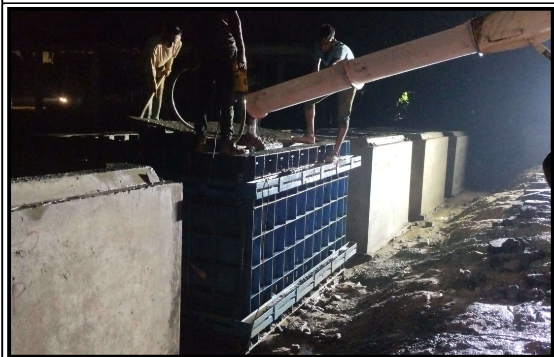
Concrete Pouring of Pre-cast Box-culvert Segment
