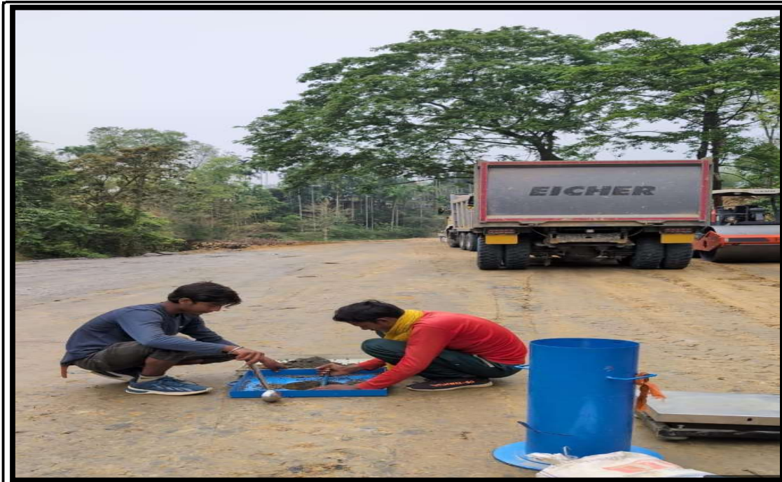
FDD Testing in Embankment Layer
