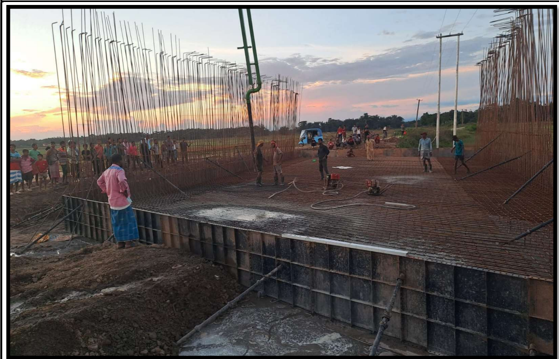
Concrete Work in Progress at CH-10+098 LHS
