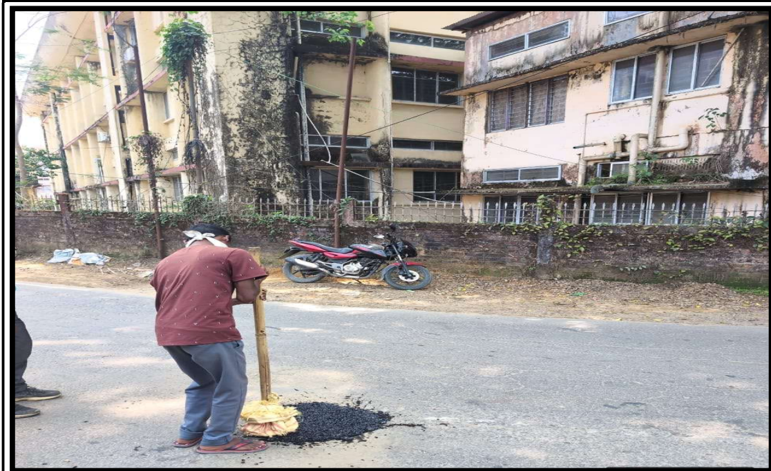
Pot Hole repair in progress
