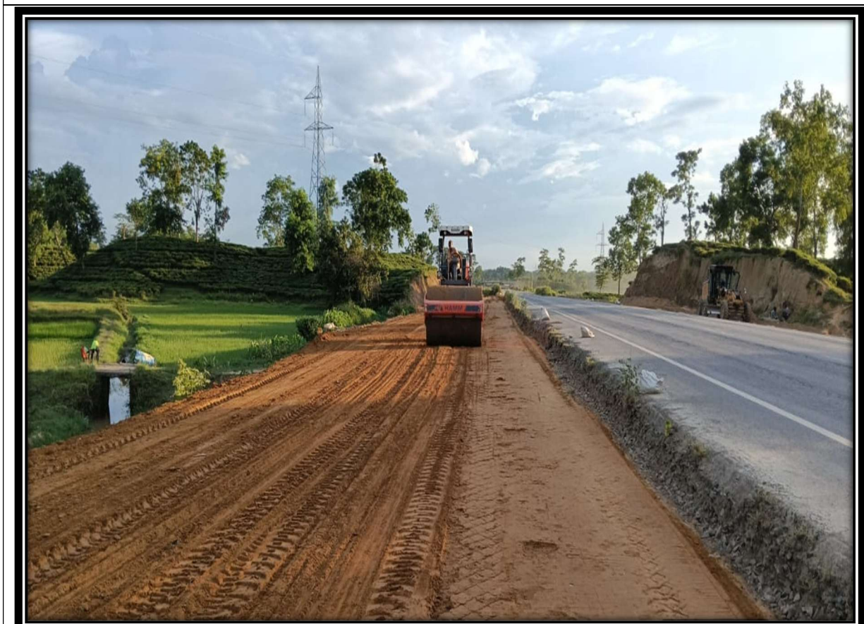
Preparation of sub-grade top at chainage-98+100
