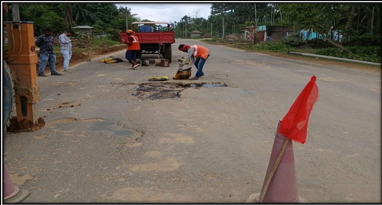
Pot hole filling work at chainage-94+000
