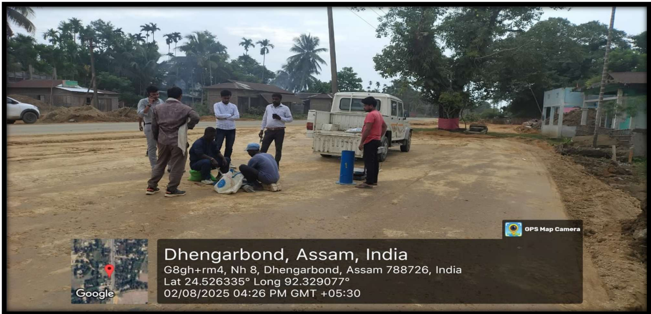
FDD checking at chainage-92+400
