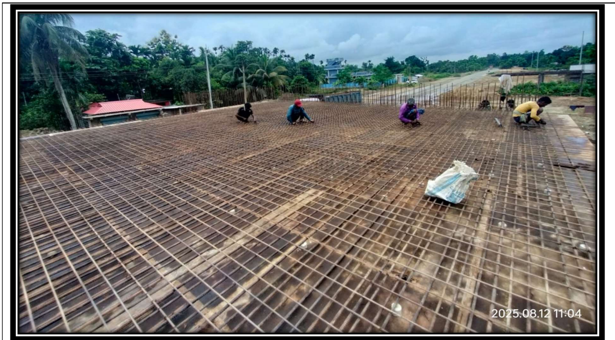
Steel placing and fixing work at ch-92+248(LVUP)
