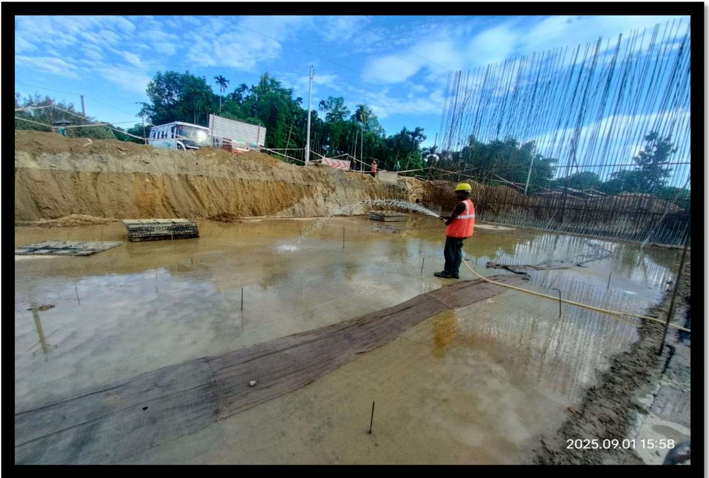
Curing work at chainage-100+290(VUP)
