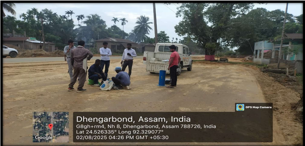
FDD checking at chainage-92+400
