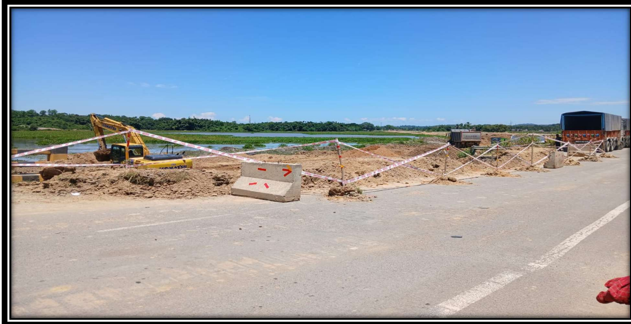
Excavation work at ch-97+102(MNB)
