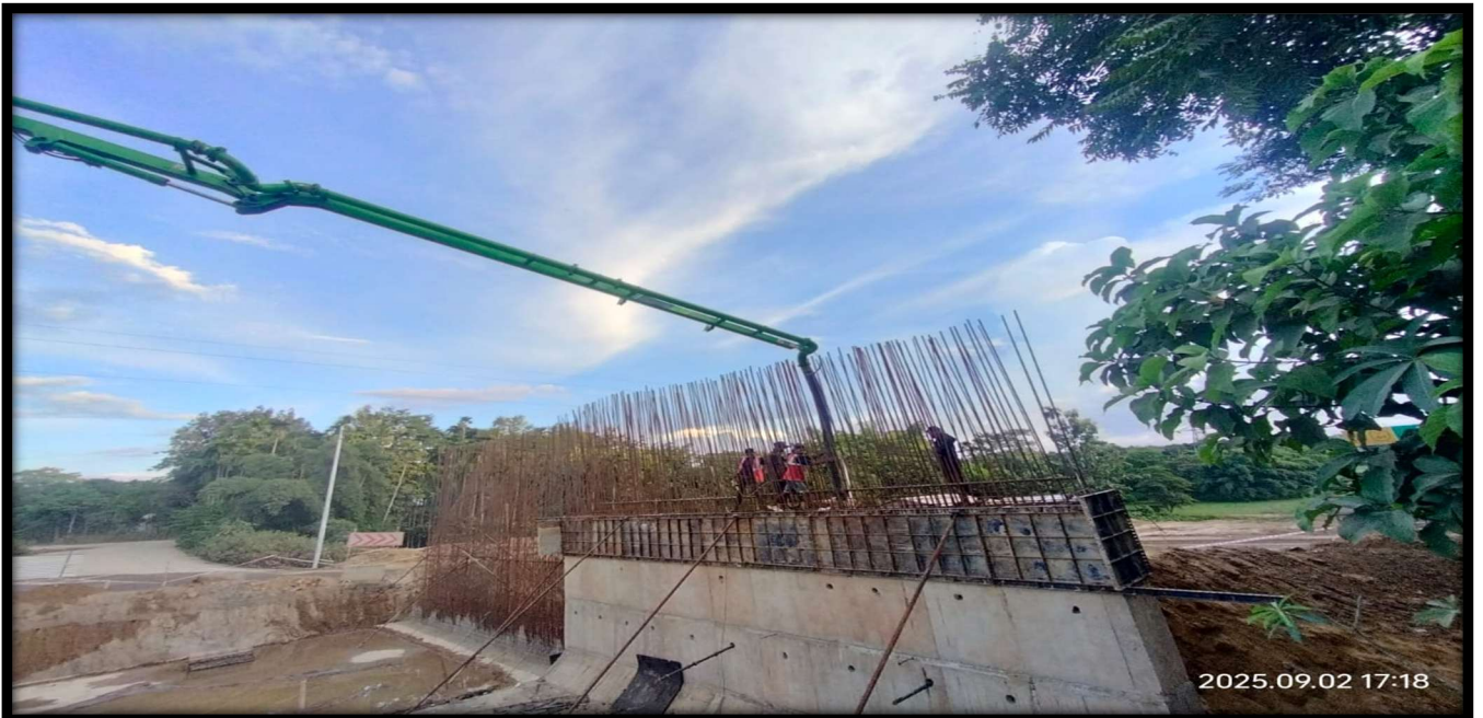
Concrete pouring at chainage-100+290 (VUP)
