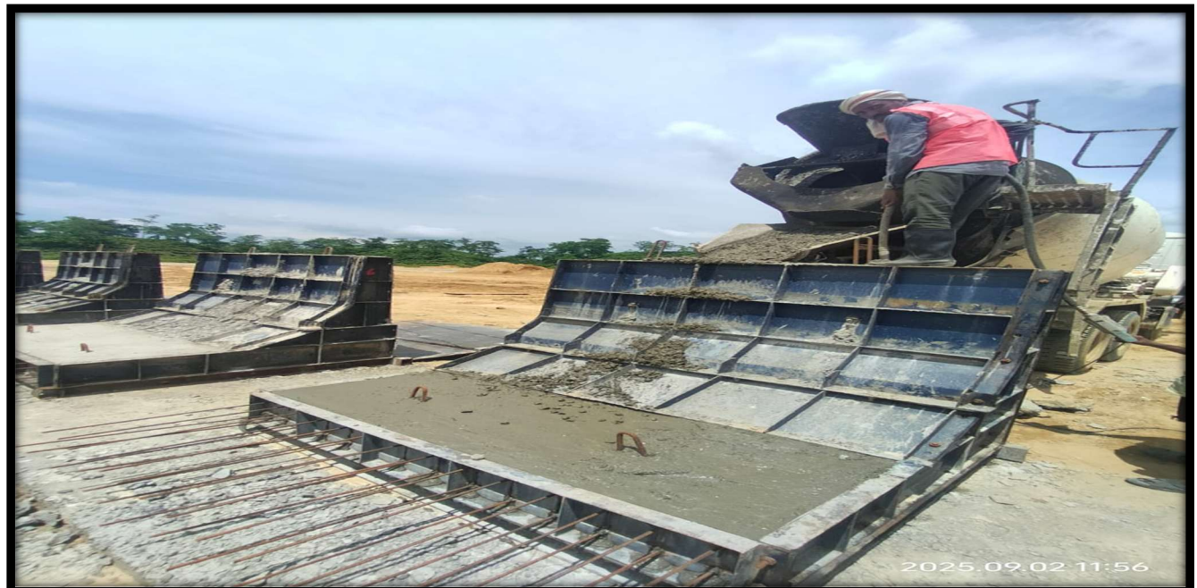
FSCB Casting work
