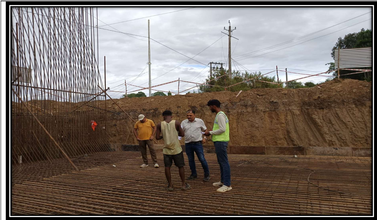
Reinforcement and formwork of checking at ch-100+290(VUP)
