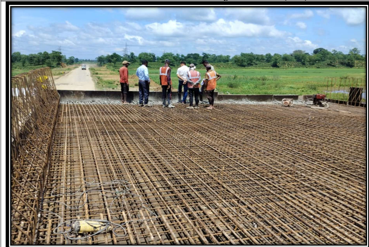
Reinforcement and formwork checking of ch-98+587(LVUP)
